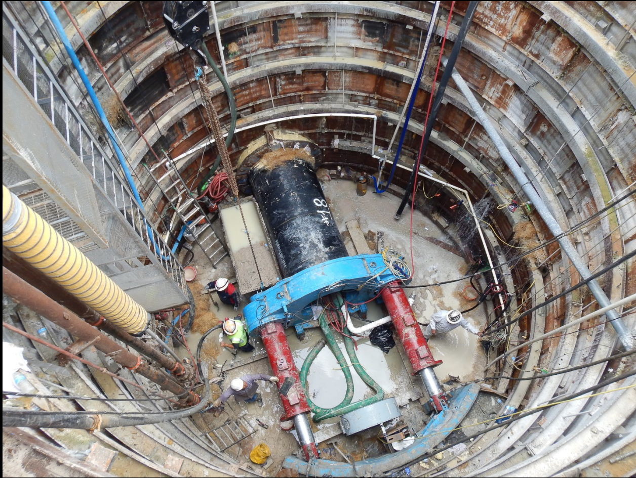
Bore Pit and Tunneling Bore Machine installation for Woodlands Waterway crossing
