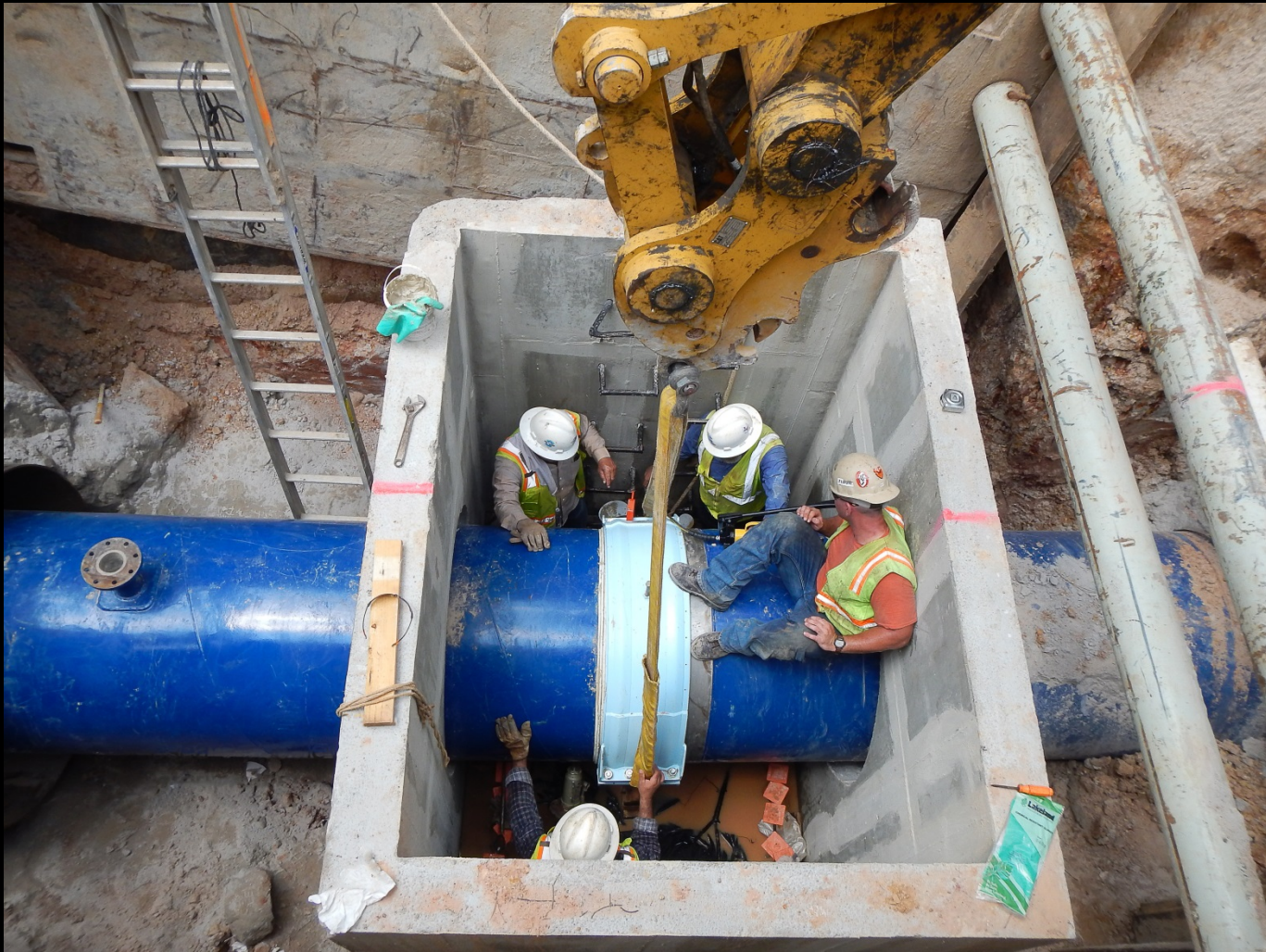
Expansion joint installation at Big Barn fault crossing
