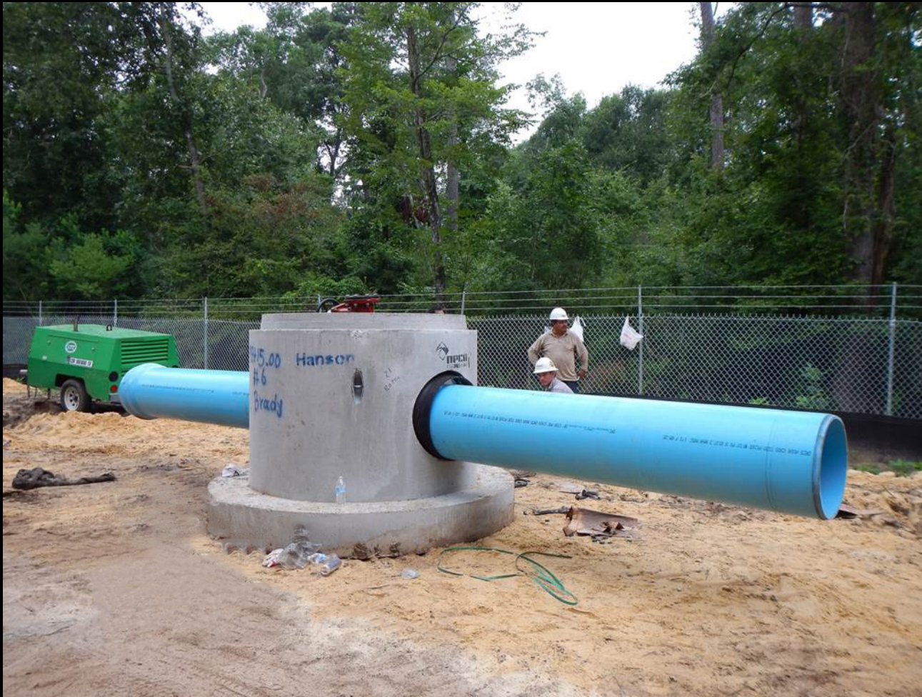
Manhole installation preparation along Silver Springs Road
