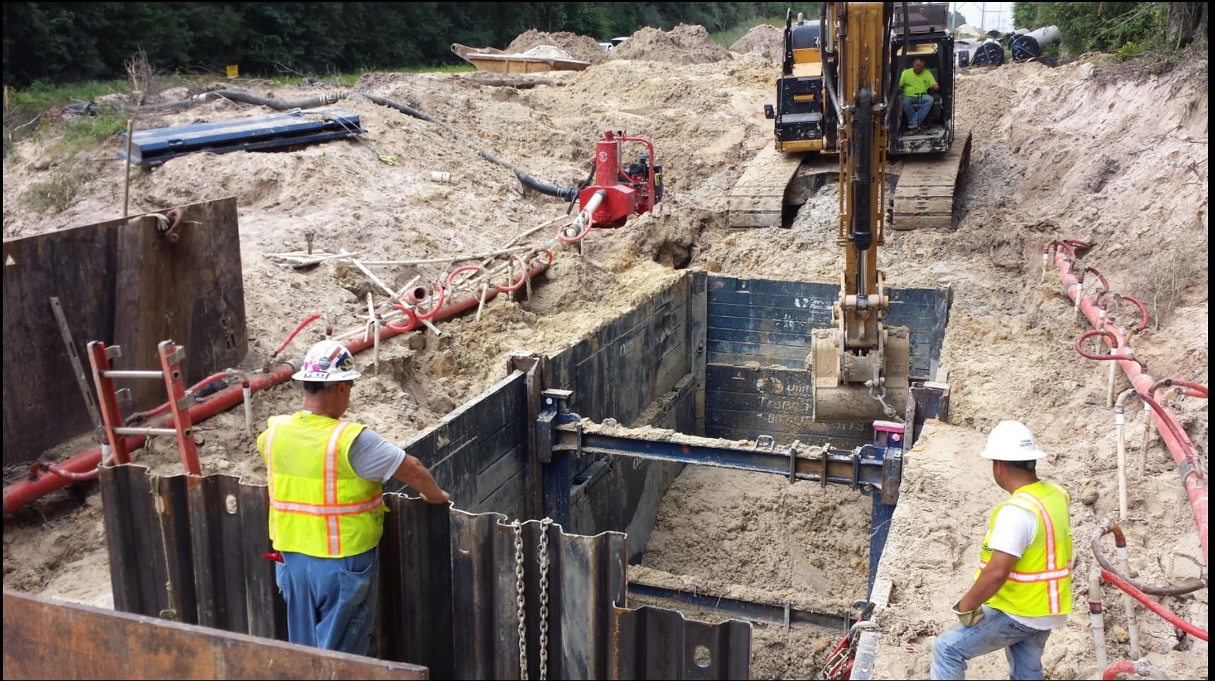
Tunnel bore pit installation along Entergy corridor
