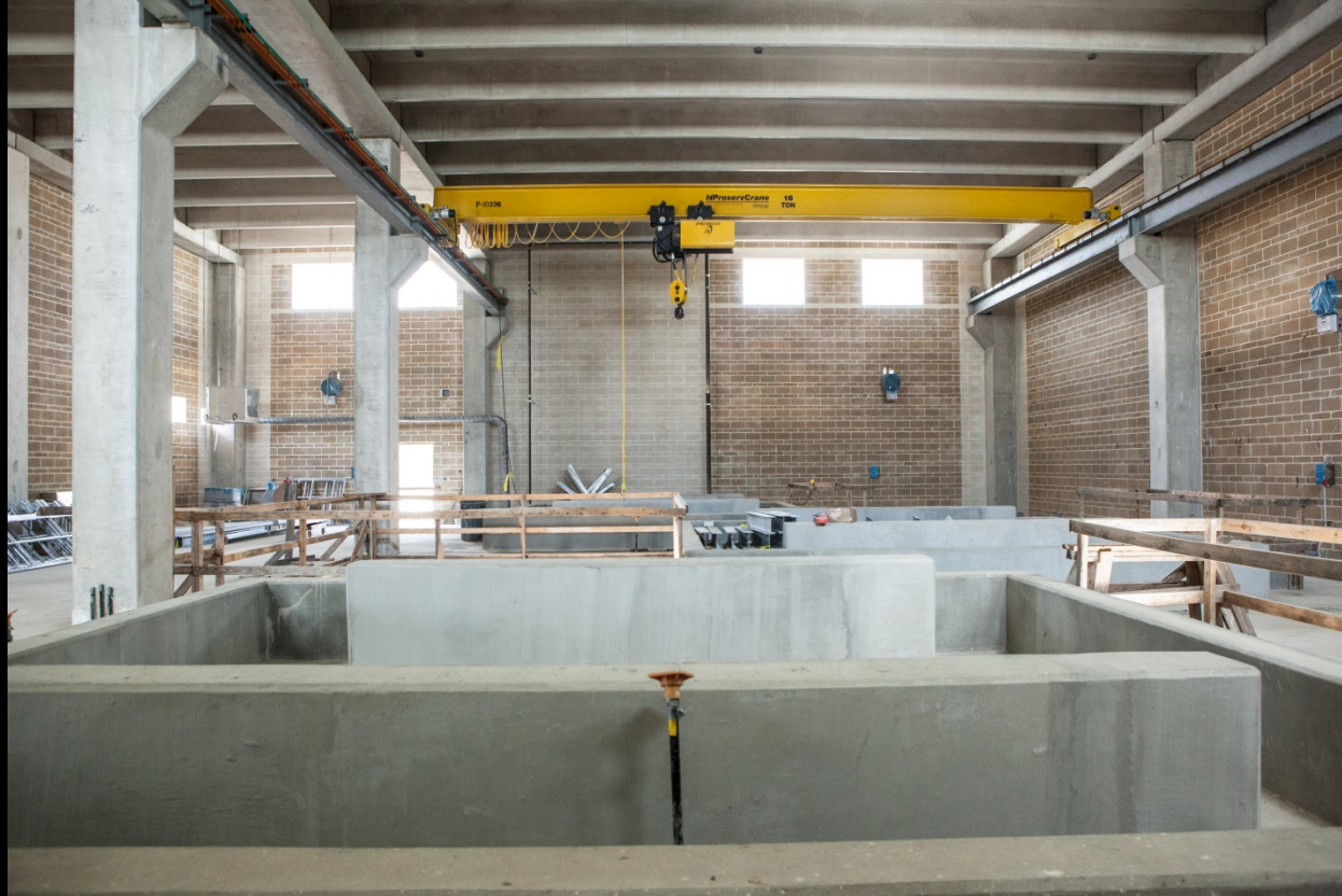
Dewatering Building – Pedestal for belt filter press
