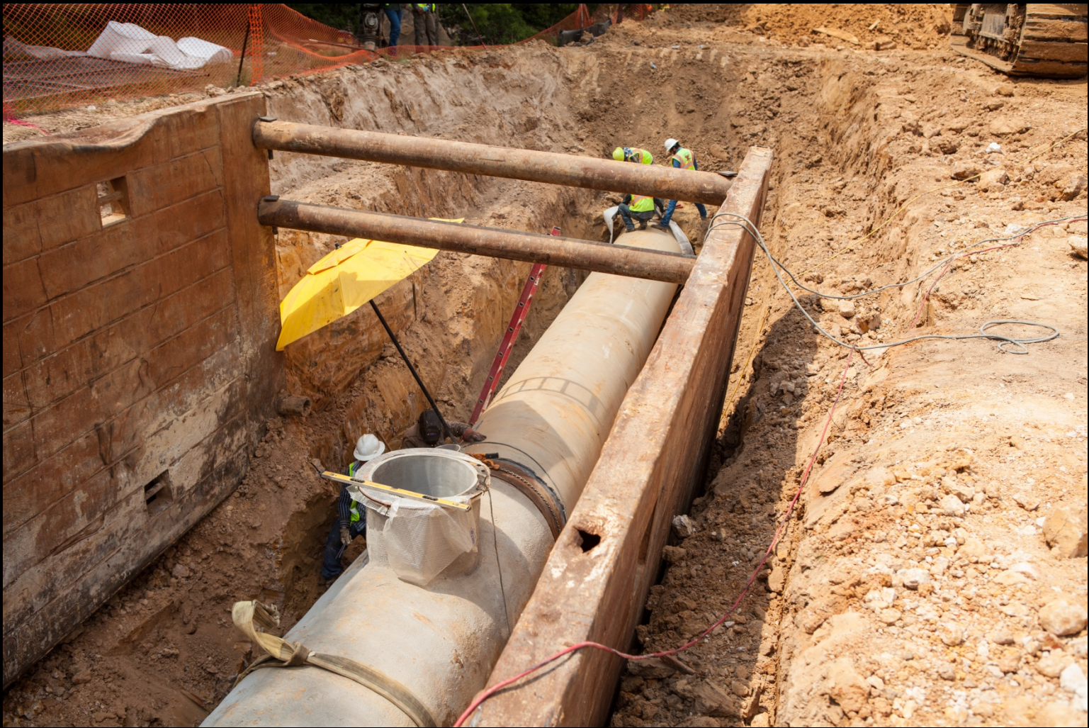
54-inch pipe installation along Sendera Ranch Road
