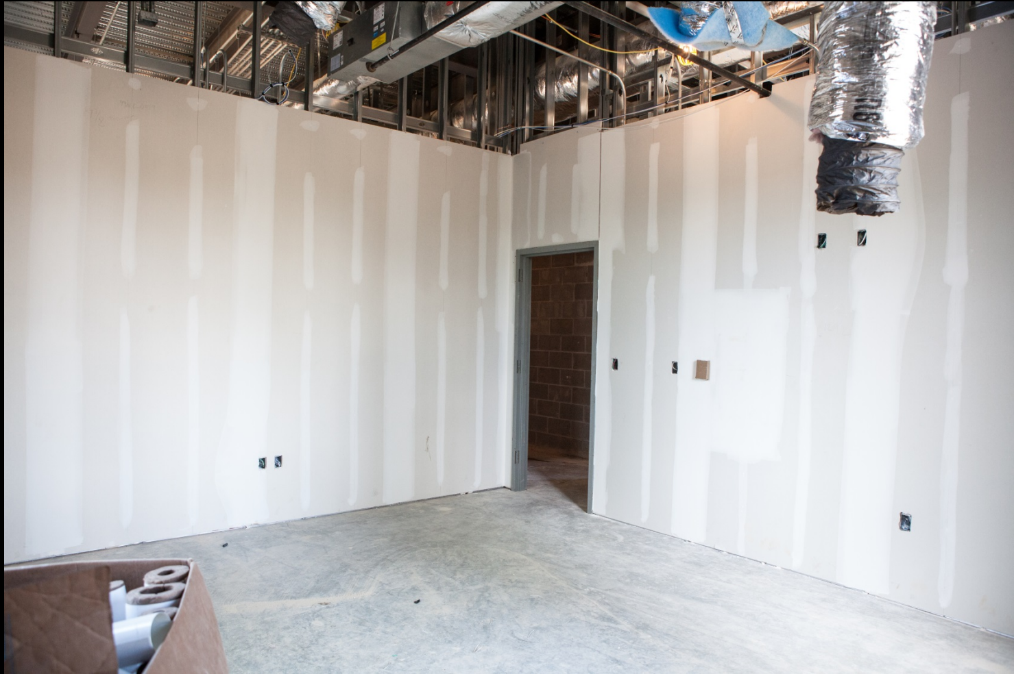
Operations Building – Drywall installation and finishing
