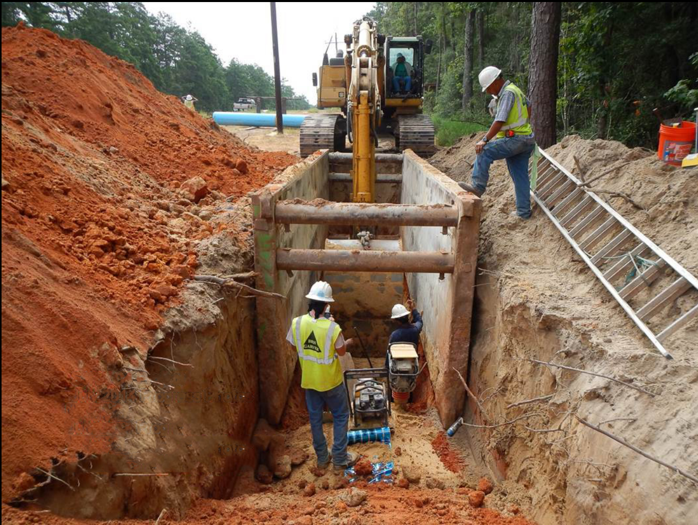
20-inch waterline installation along FM 830
