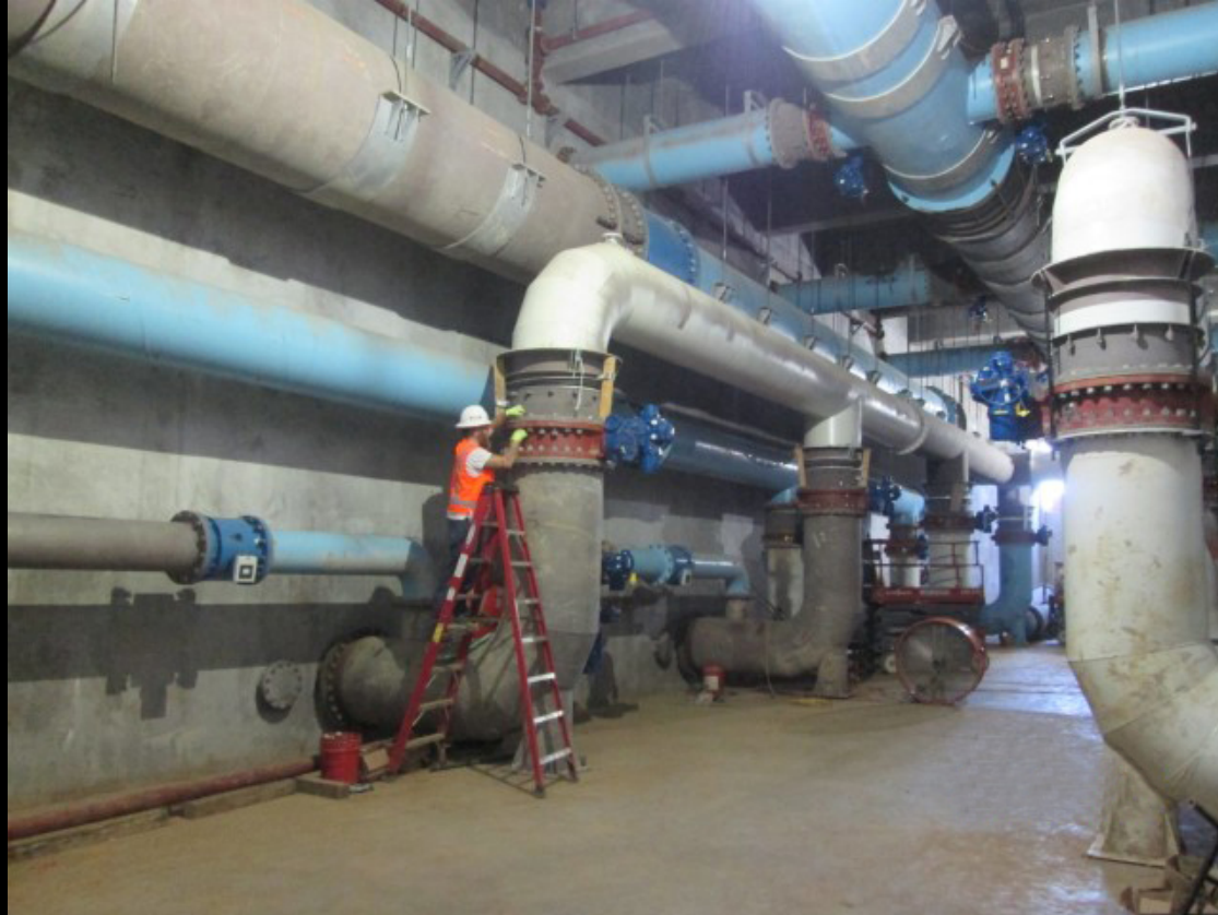
Granulated Activated Carbon – Carbon contactor process piping installation
