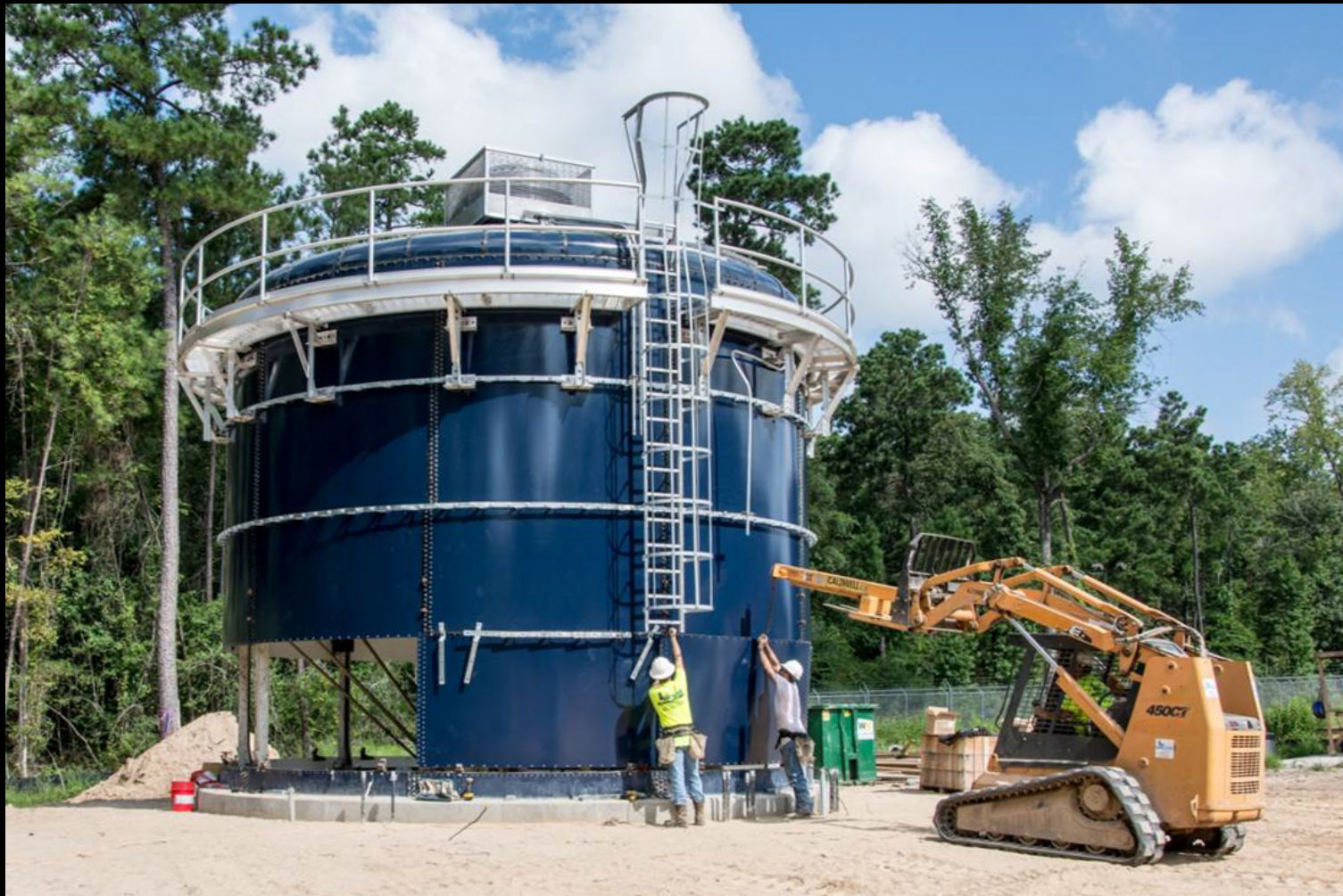
Standpipe tank panel installation
