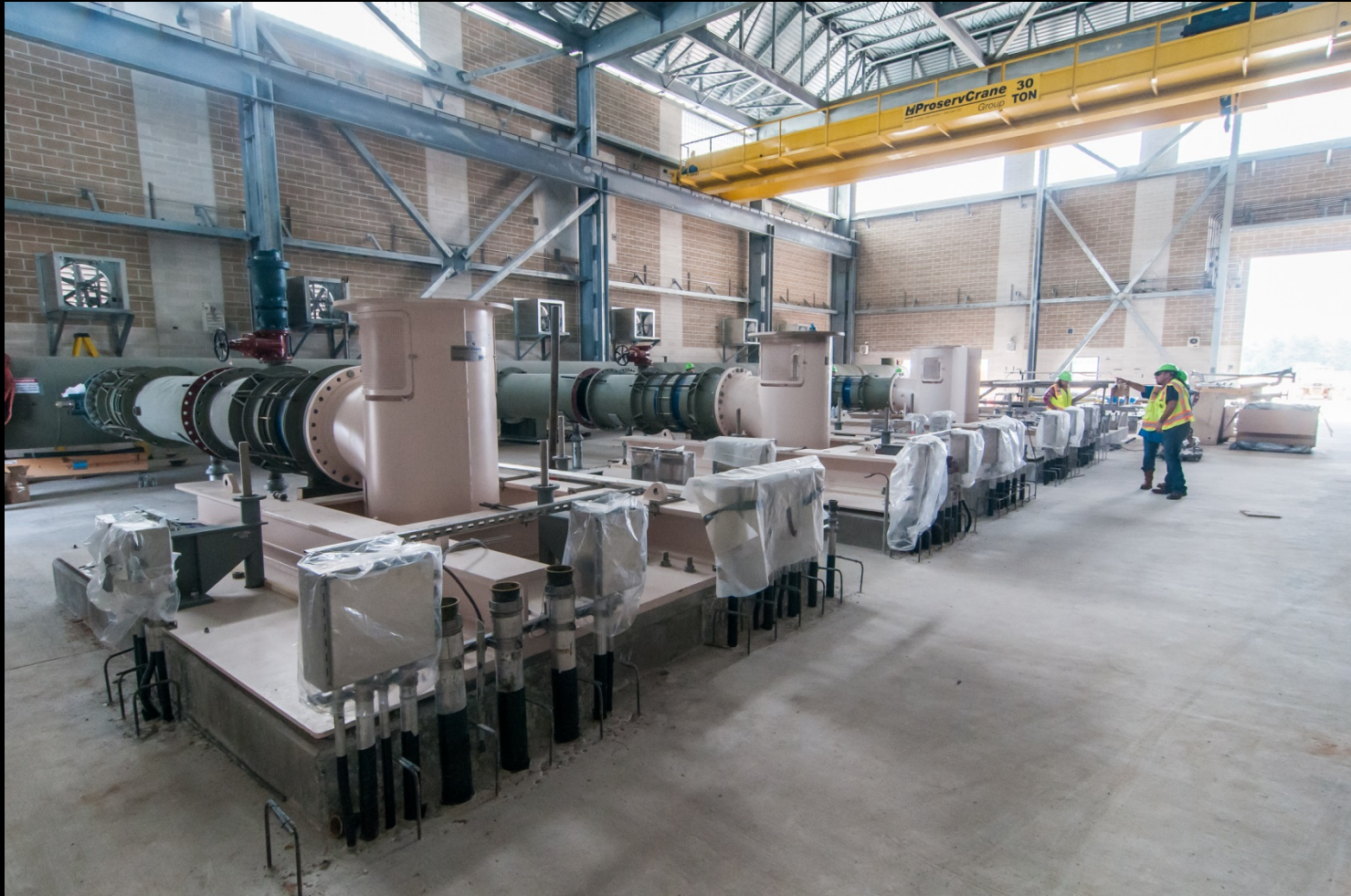
Raw Water Intake & Pump Station – Pump assembly and slide gate installation
