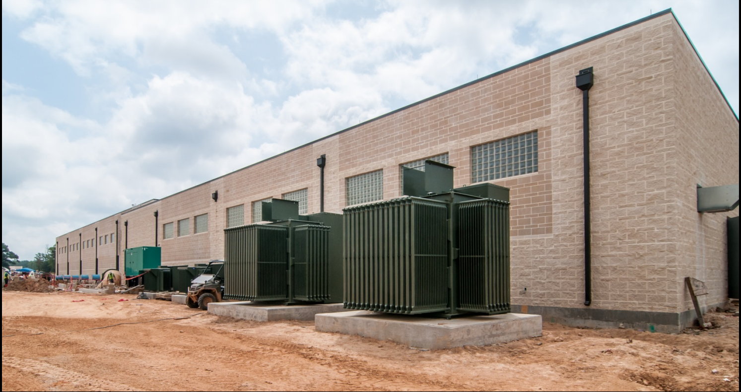
High Service Pump Station – Transformer installation (12470V:4160V)
