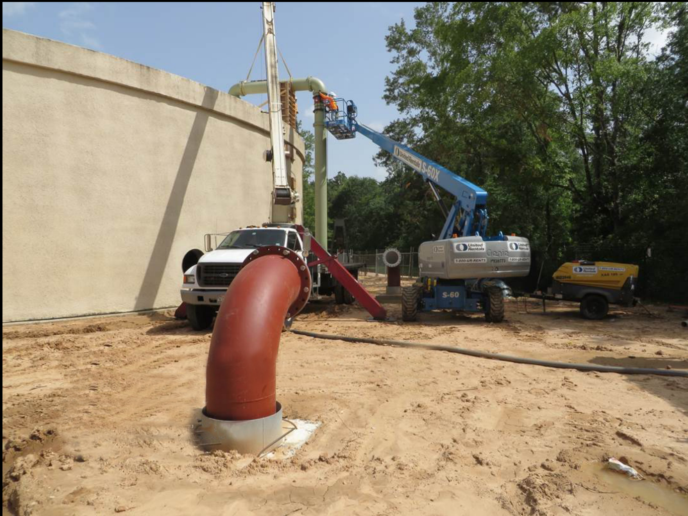
Riser pipe installation at Woodlands Water Plant No. 1
