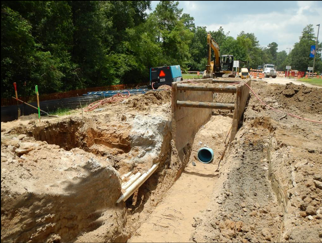
20-inch pipe installation along Grogans Mill Road
