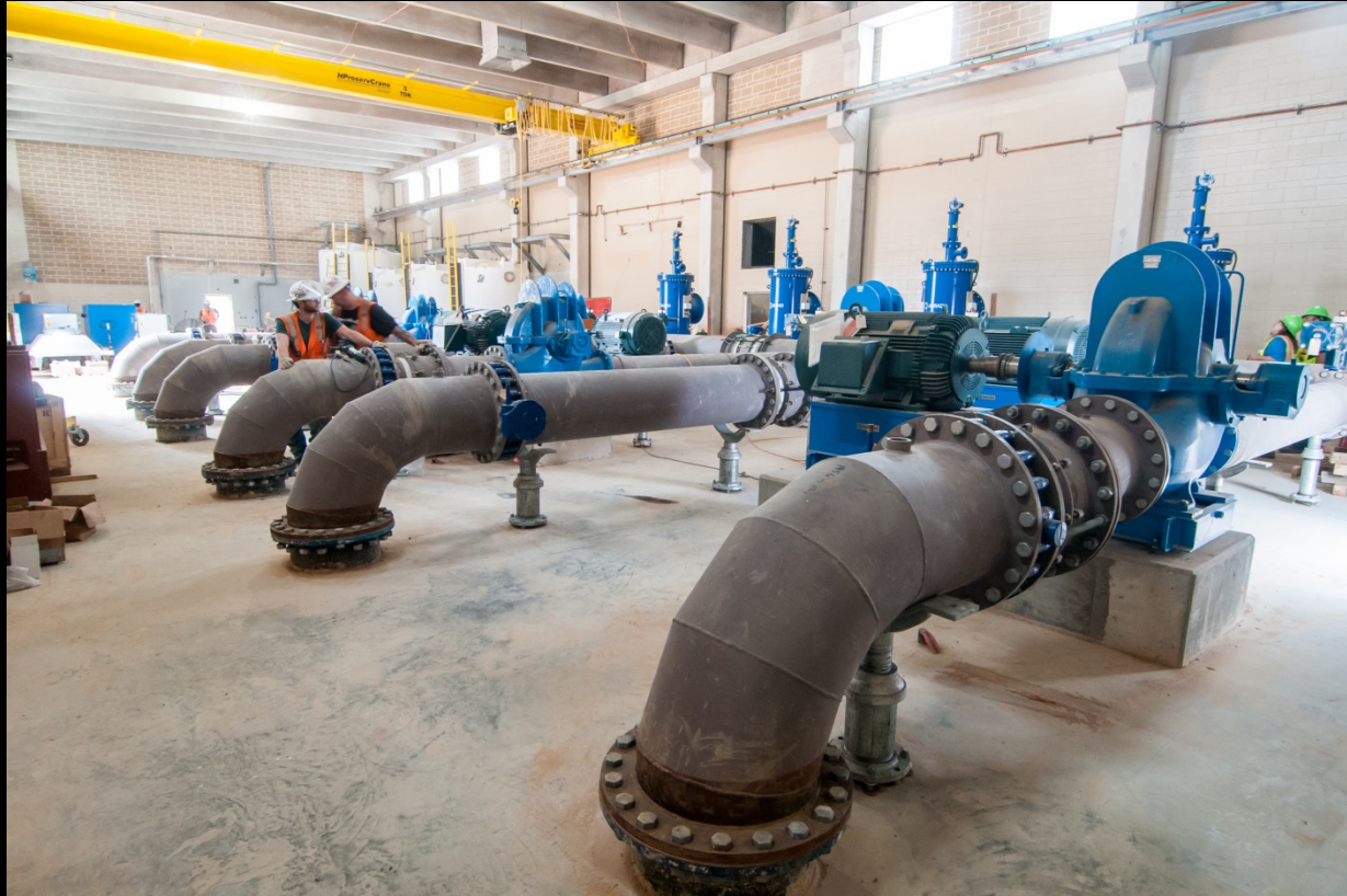
Membrane Building – Feed pump and piping installation
