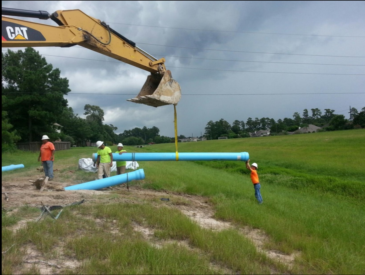
12-inch waterline installation along Montgomery County Drainage District No. 6
