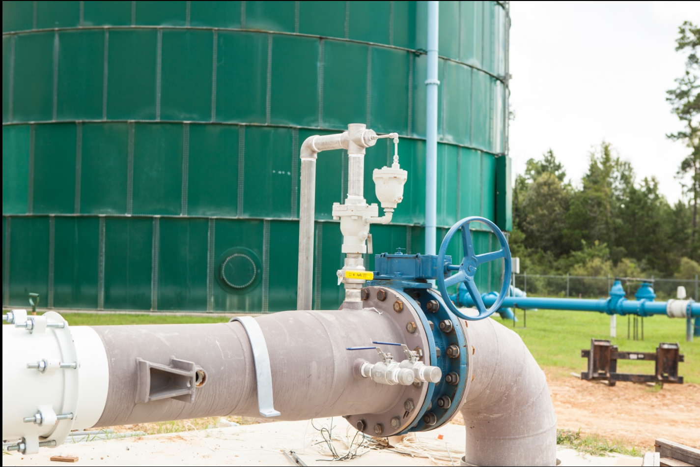
Flow Control Pressure Station assembly at Conroe Water Plant No. 20
