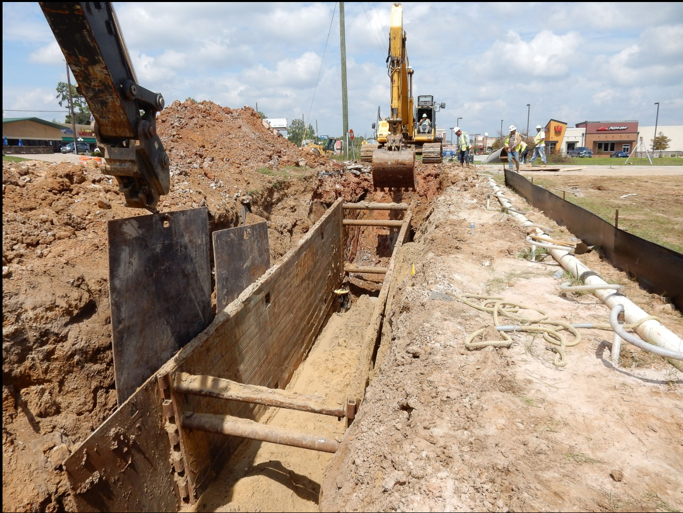
54-inch open-cut pipe installation along FM 2978 south of FM 1488
