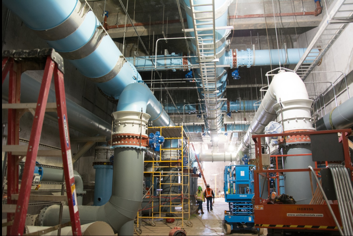
Granulated Activated Carbon Building – Piping and instrumentation installation
