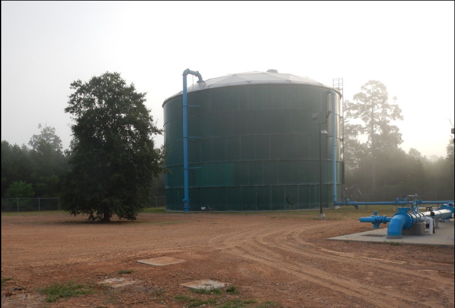
Site restoration at Conroe Water Plant No. 20
