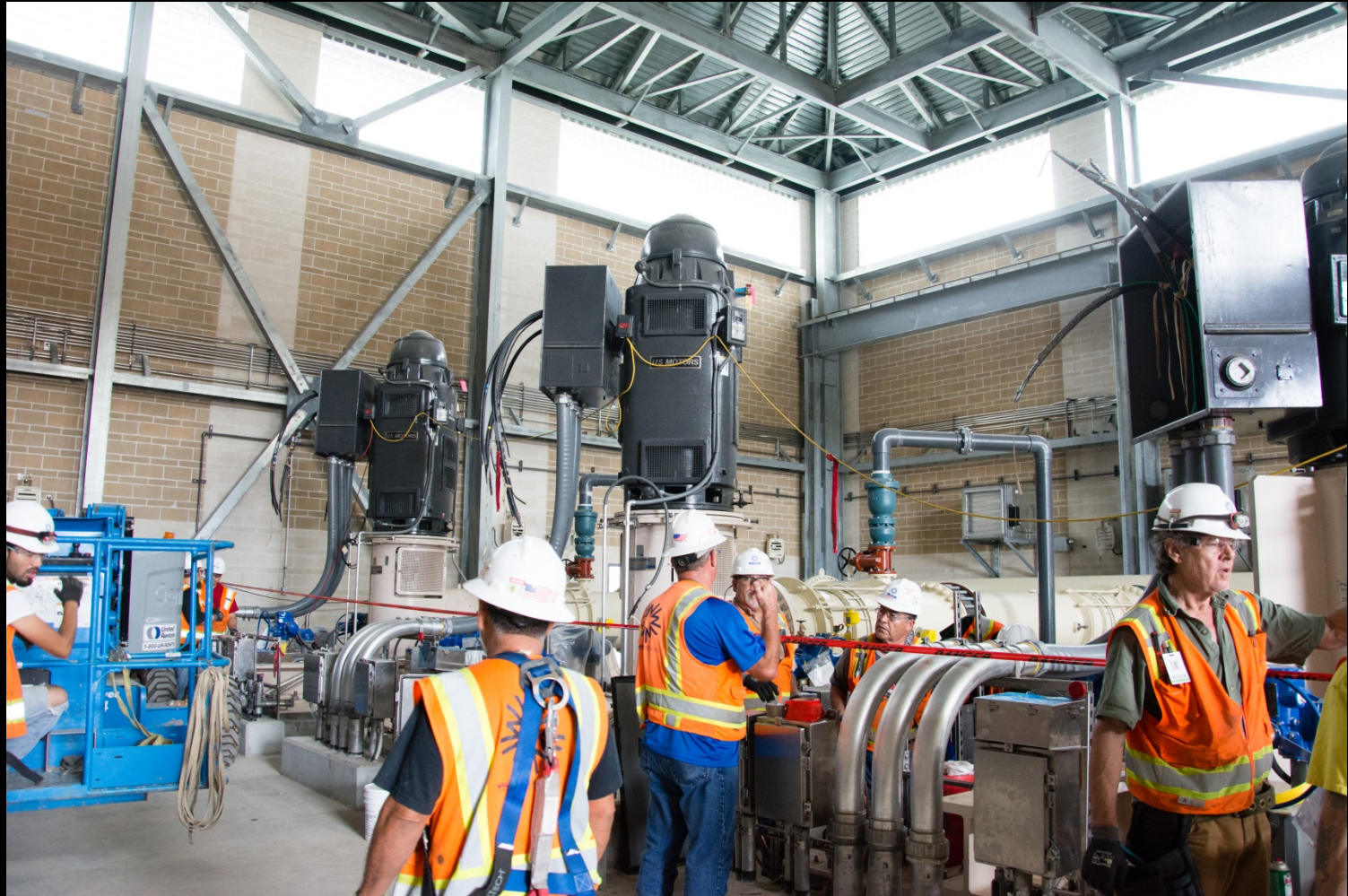
Raw Water Intake & Pump Station – Pump motor installation
