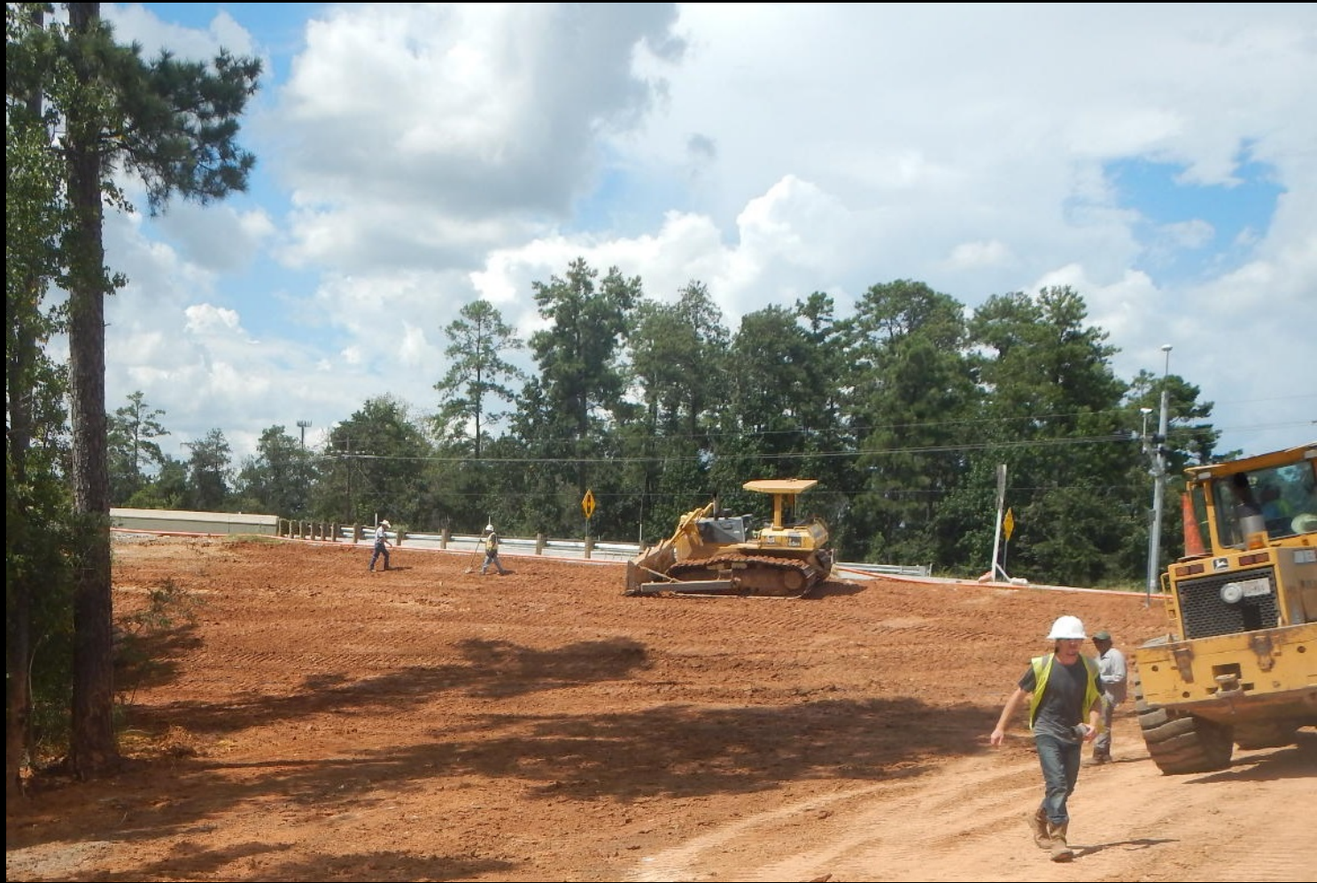
Site restoration along FM 830 at I-45
