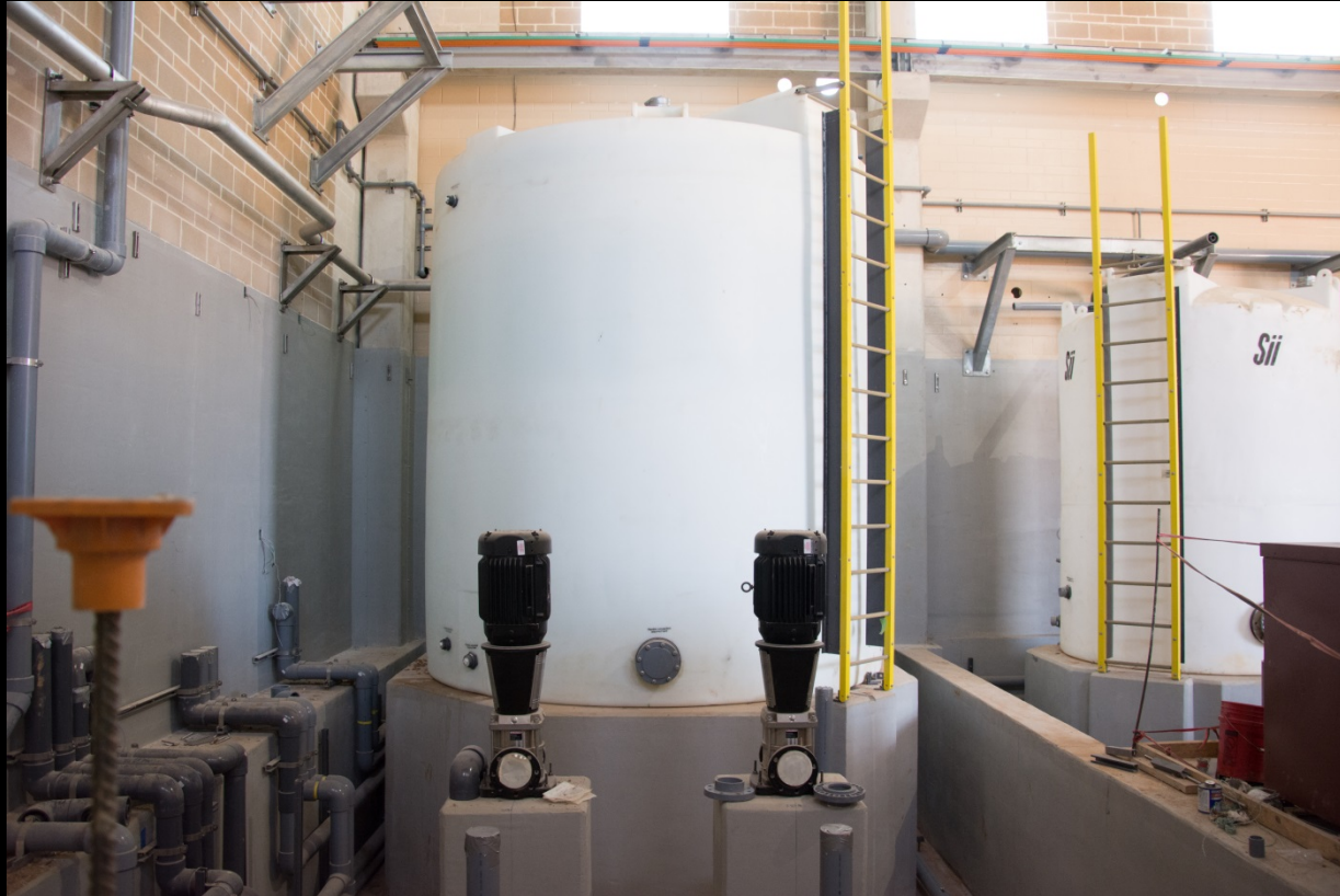
Membrane Building – Chemical storage tank and feed pumps
