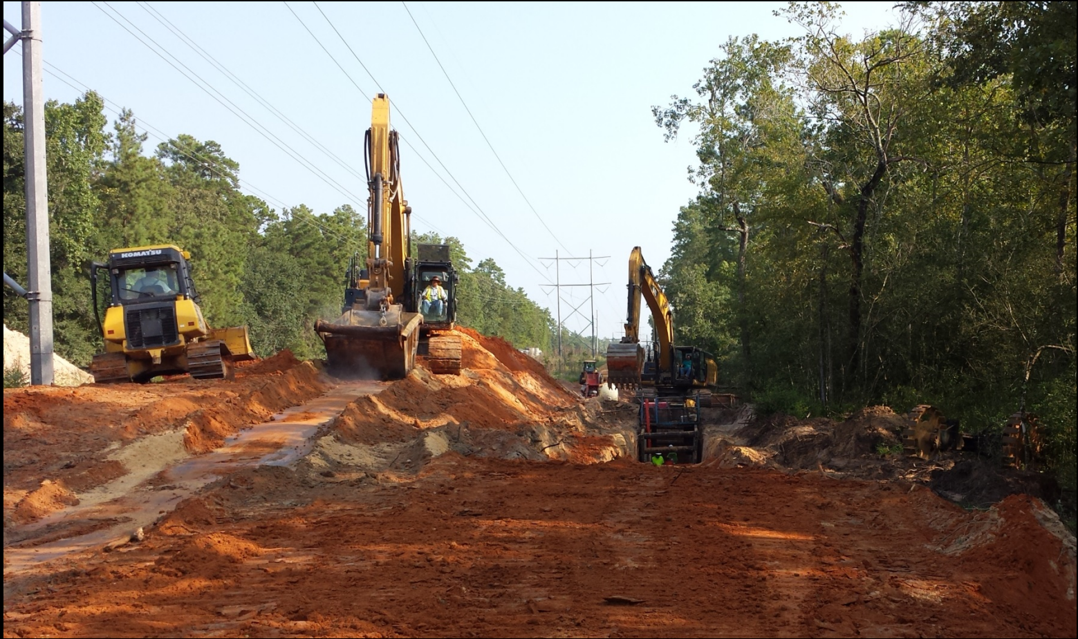
36-inch open-cut pipe installation along Entergy Corridor
