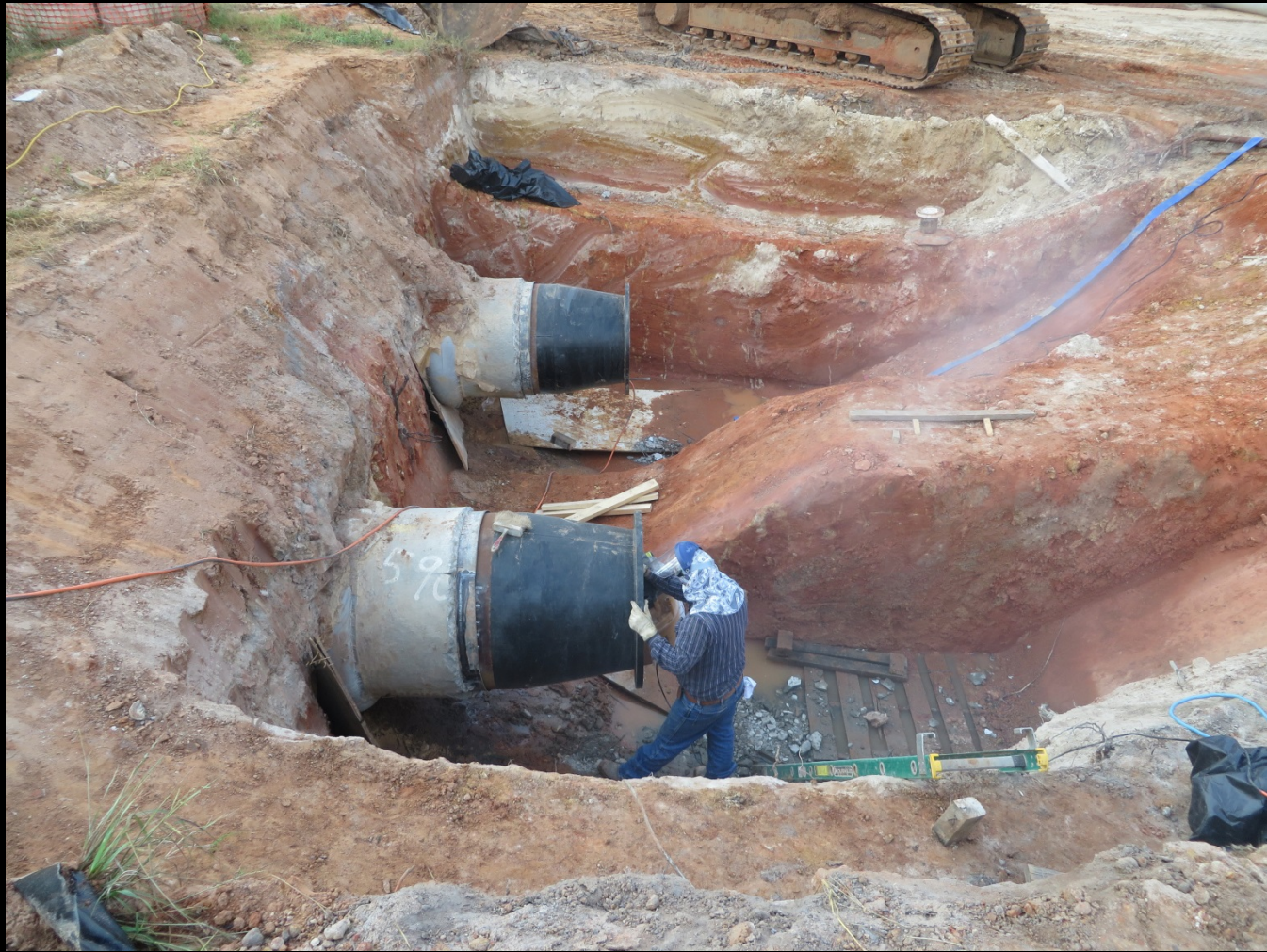
36-inch x 30-inch pipe reducer connections to Standpipe
