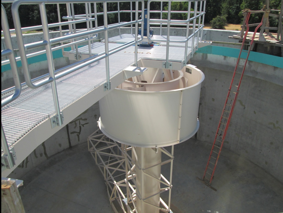
Sludge Thickeners – Stilling well and catwalk installation
