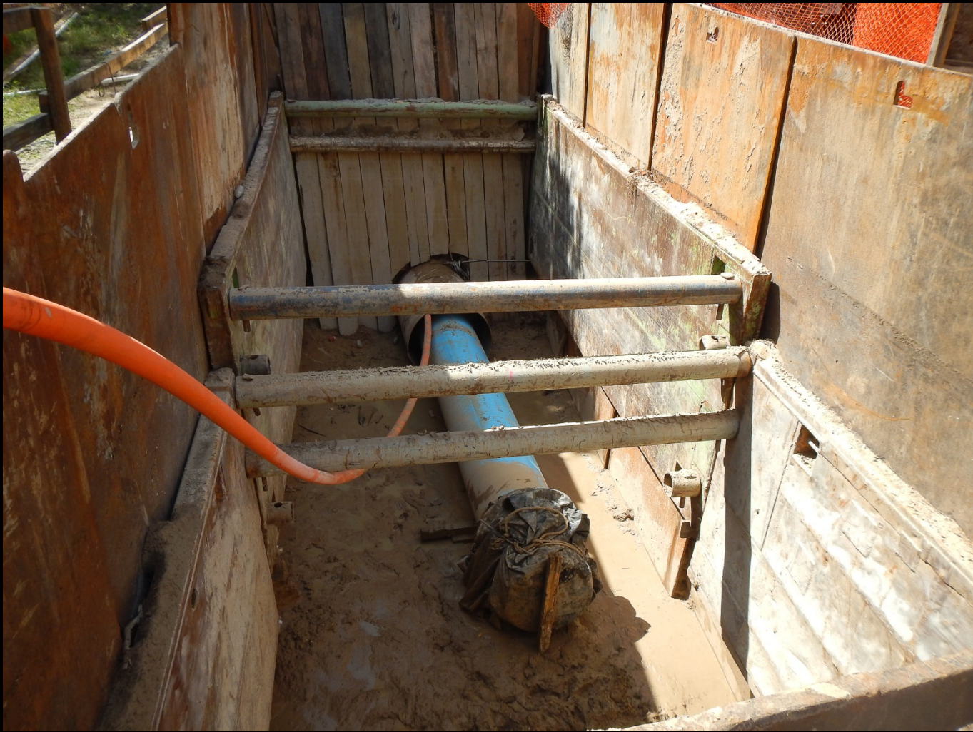
30-inch pipe and fiber optic conduit installation along Research Forest Dr.
