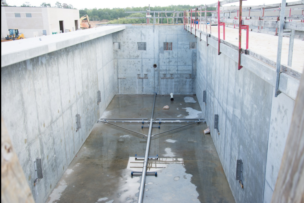
Pretreatment – Hoseless Sludge Collection System installation
