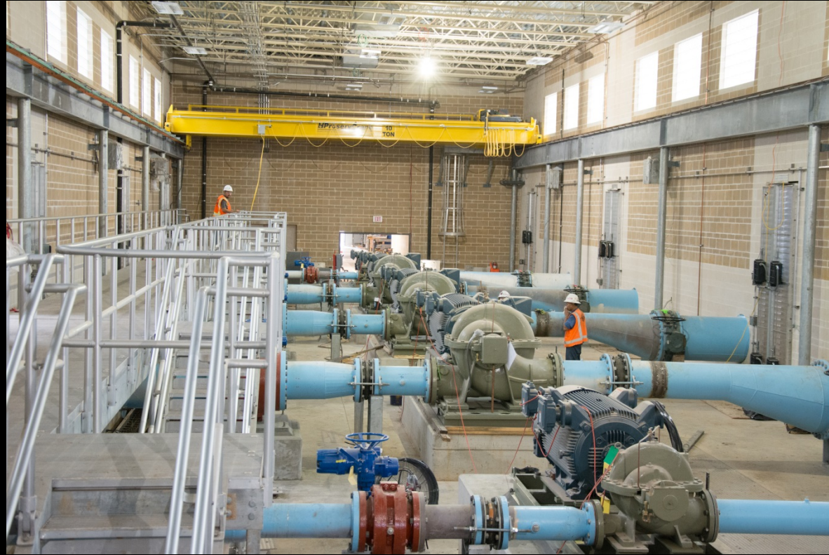
High Service Pump Station – Pump and motor assemblies
