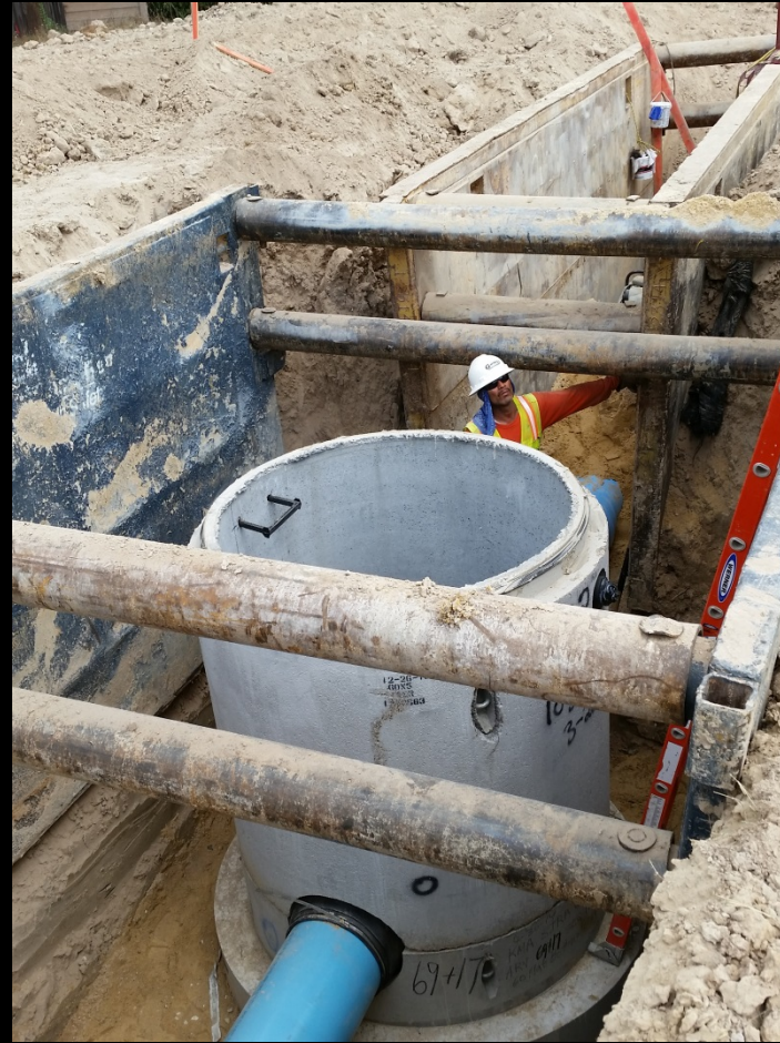
Air Vacuum Relief Valve Manhole installation
