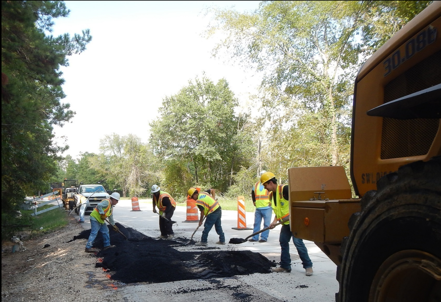
Asphalt shoulder restoration along Grogans Mill Road at Evergreen Circle
