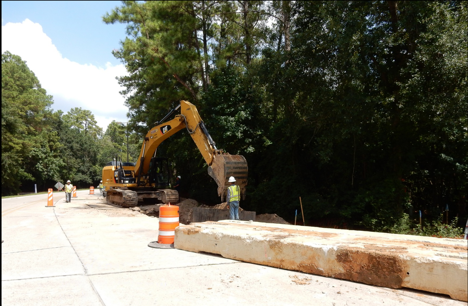
24-inch open-cut pipe installation along South Millbend Dr.
