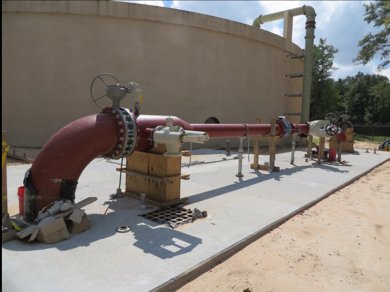
Flow Control Pressure Station at Woodlands Water Plant No. 1
