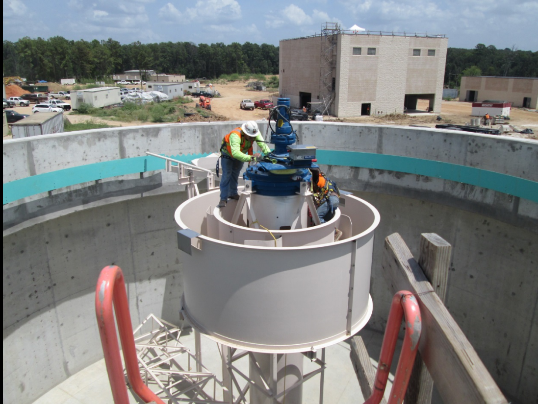
Sludge Thickeners – Installation of mechanical equipment
