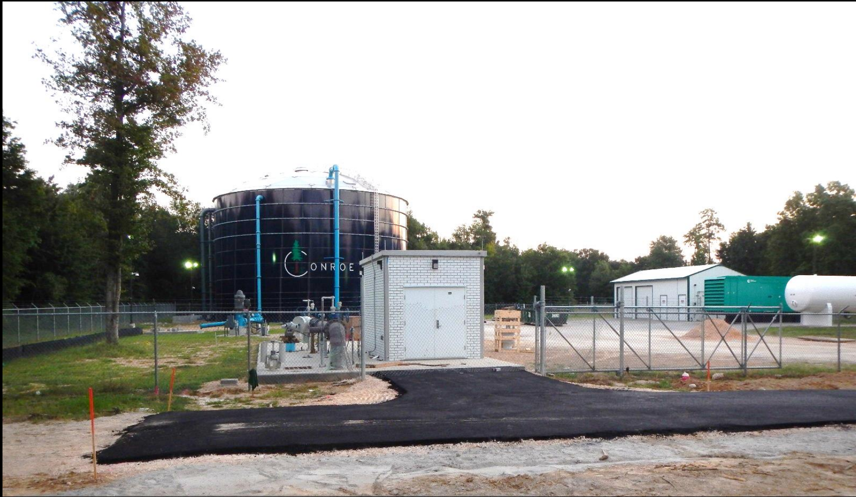
Site work at Conroe Water Plant No. 22
