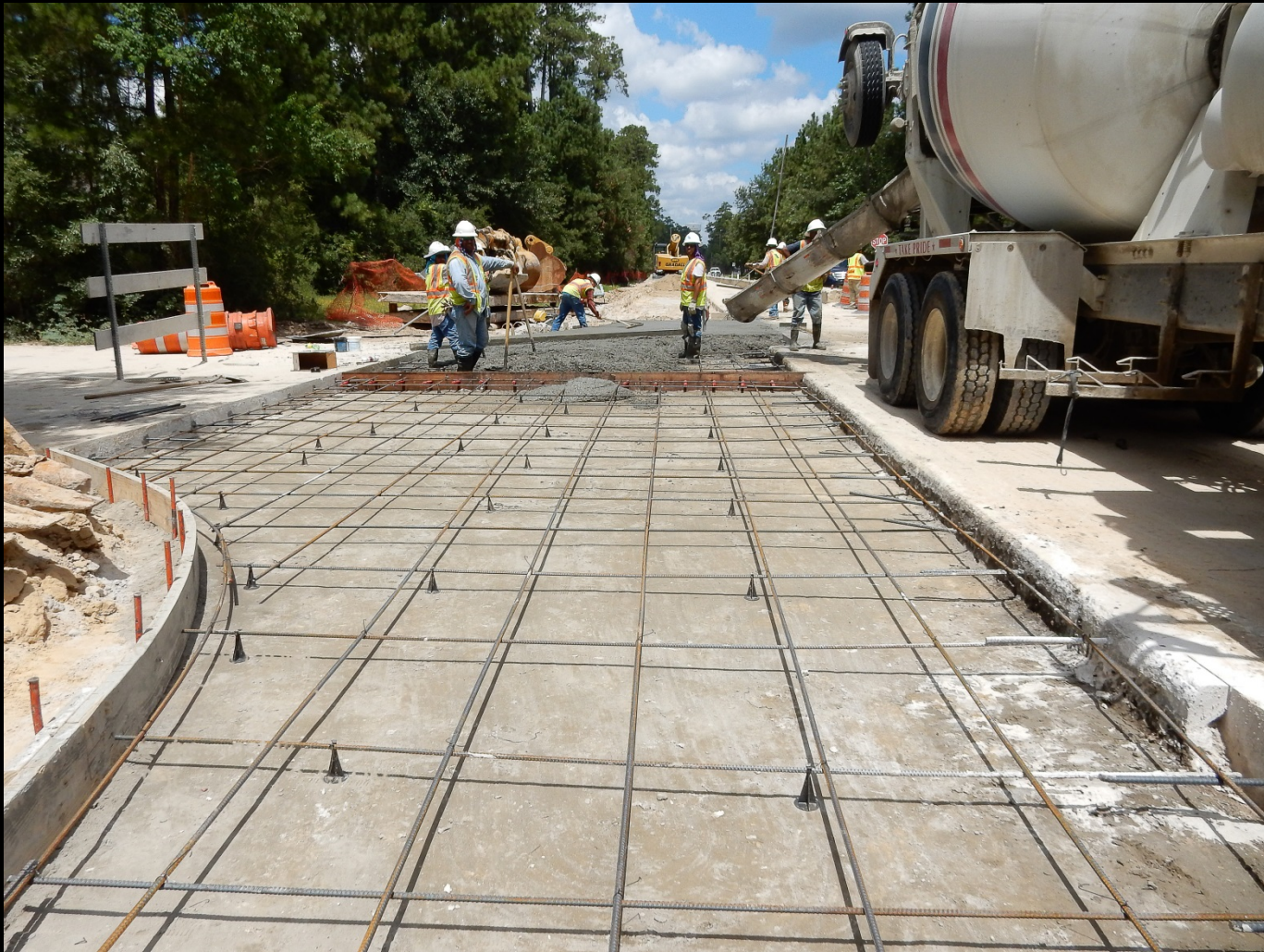
Pavement restoration along Research Forest
