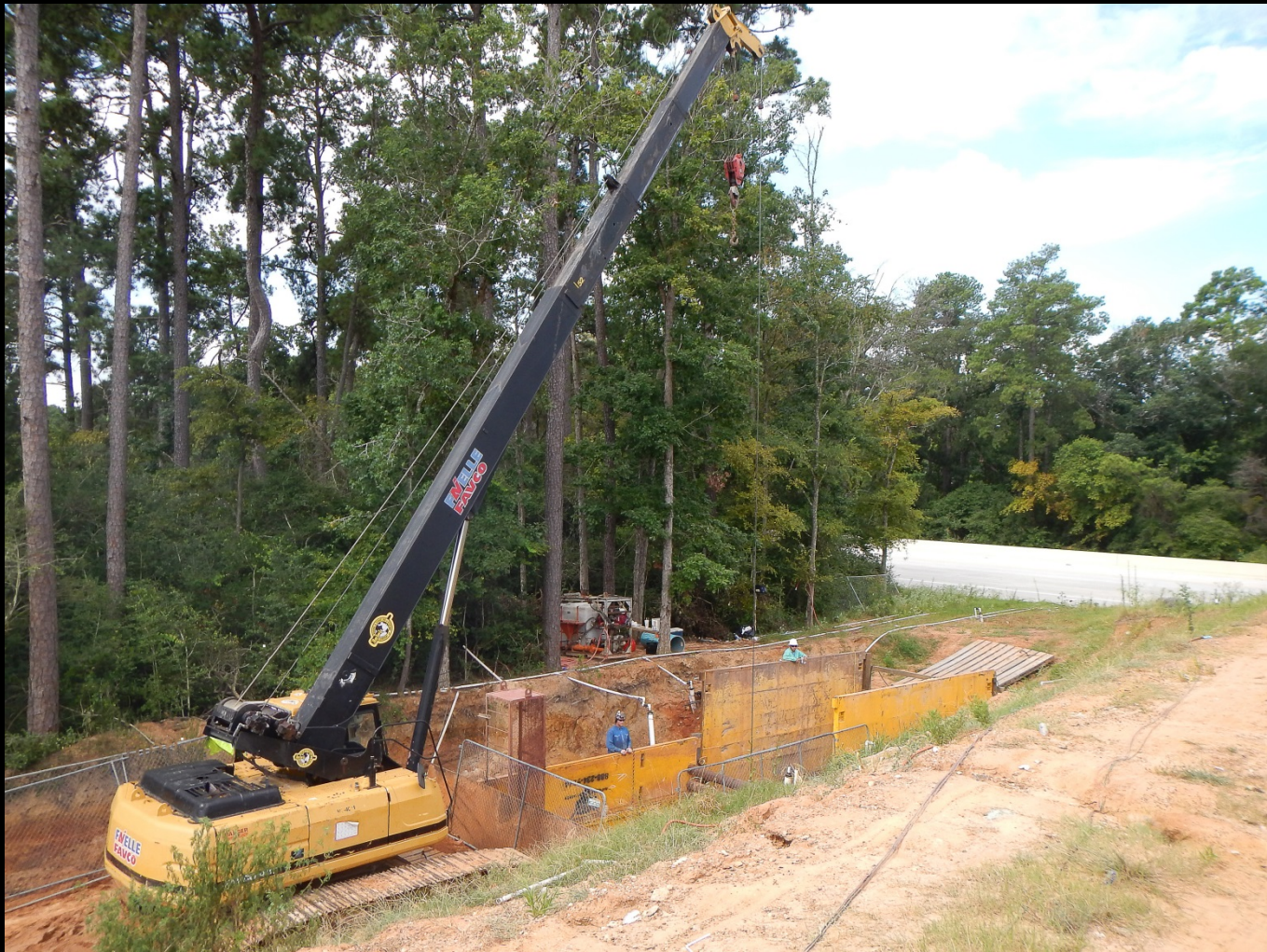
Tunnel operation for 20-inch waterline installation under I-45
