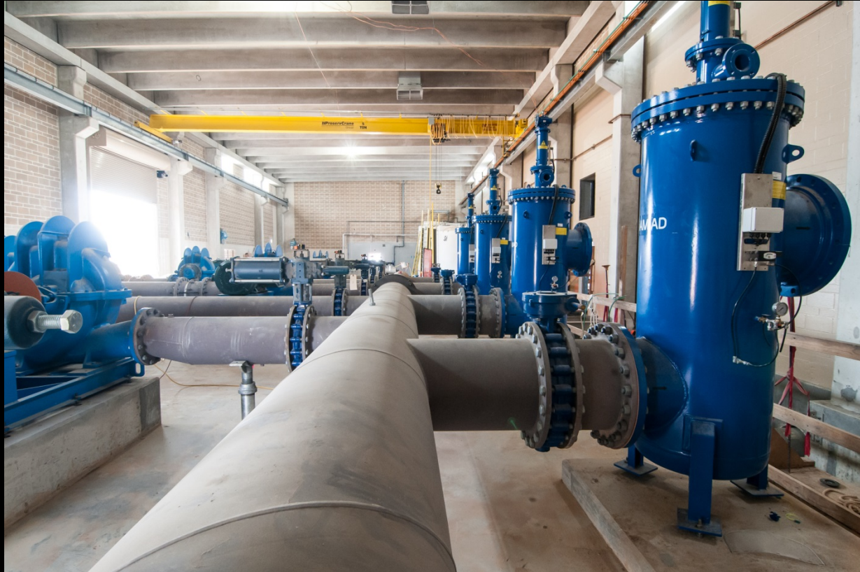
Membrane Building – Supply header and strainer installation
