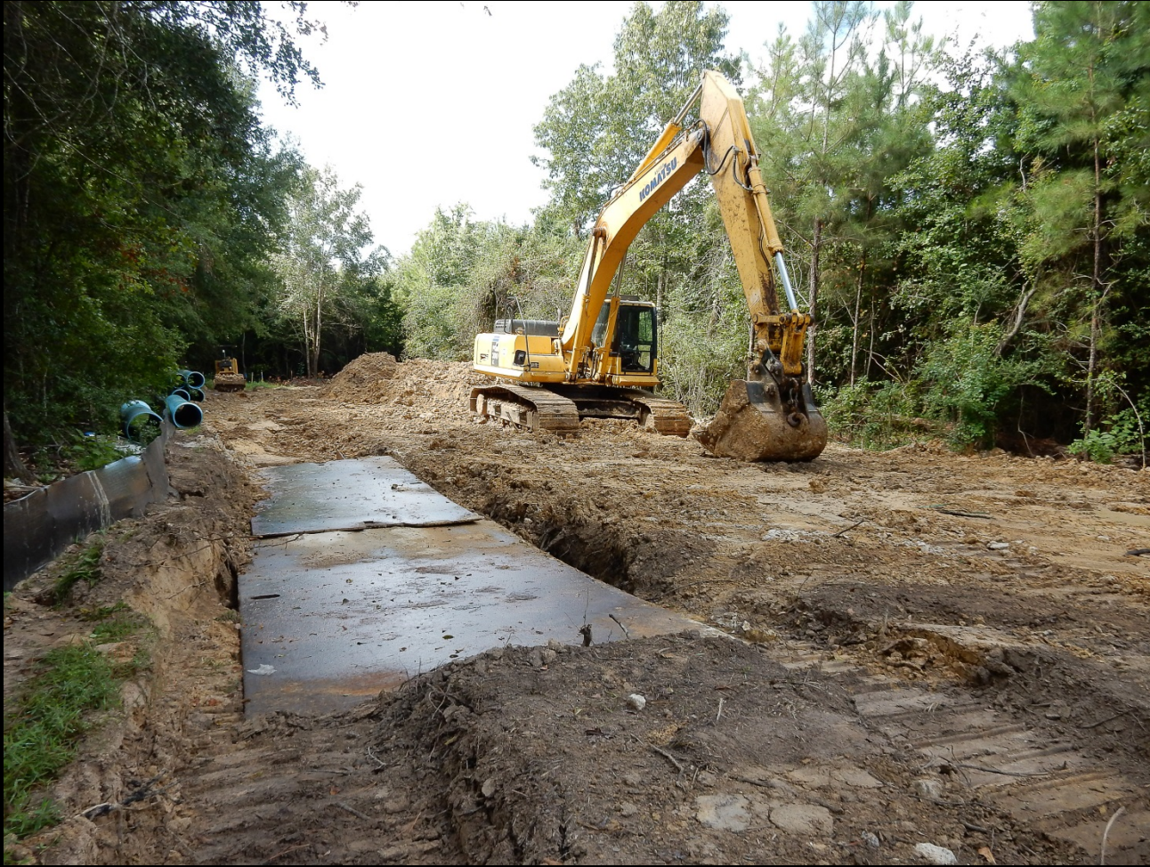
Open cut pipe installation adjacent to Union Pacific Railroad property
