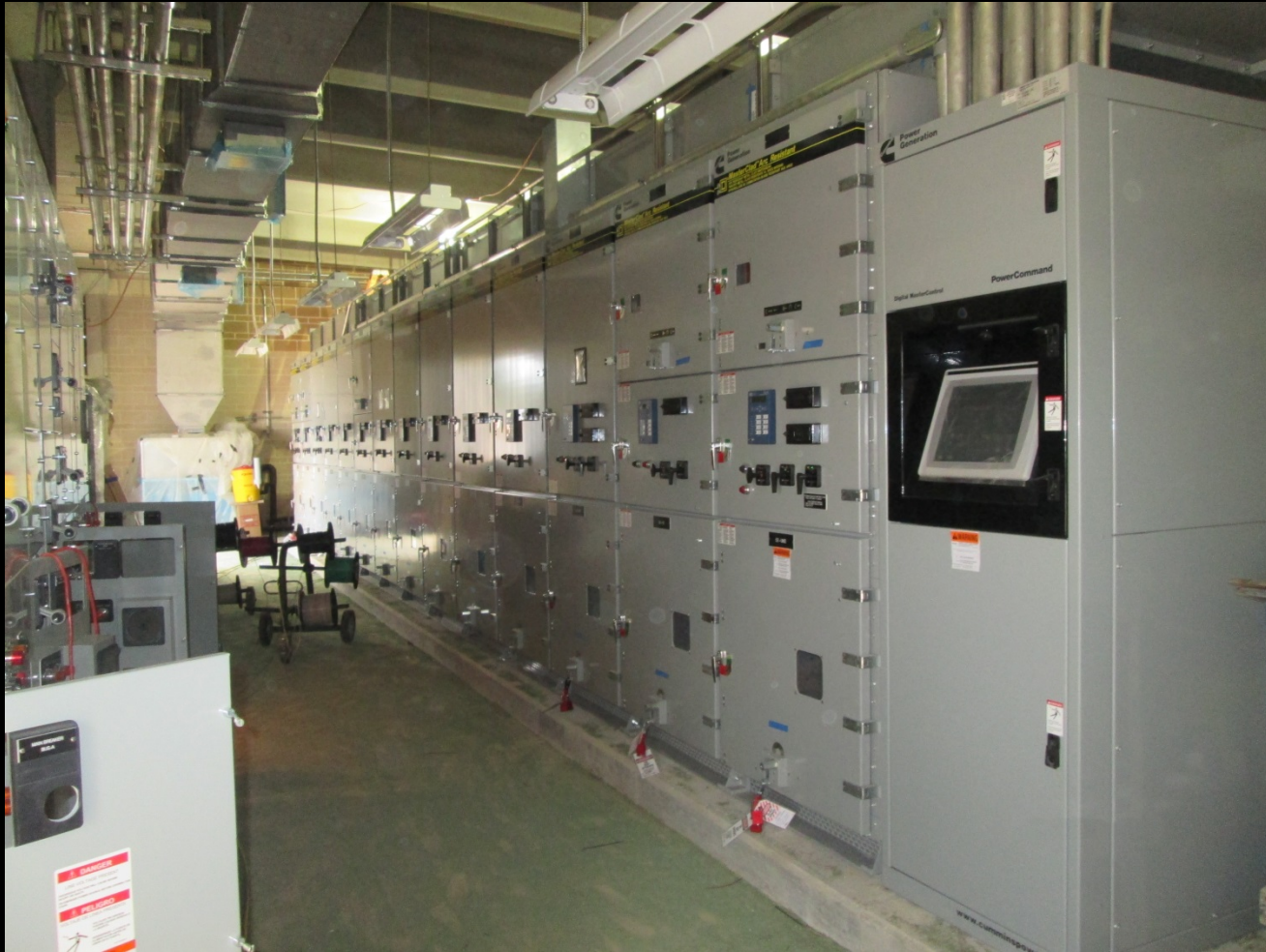
Electrical Building – Paralleling switch gear installation
