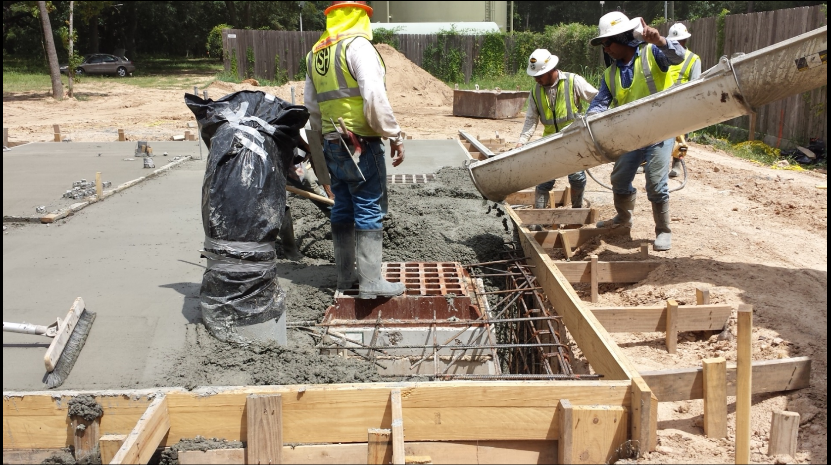
Flow Control Pressure Slab installation at Woodlands Water Plant No. 1
