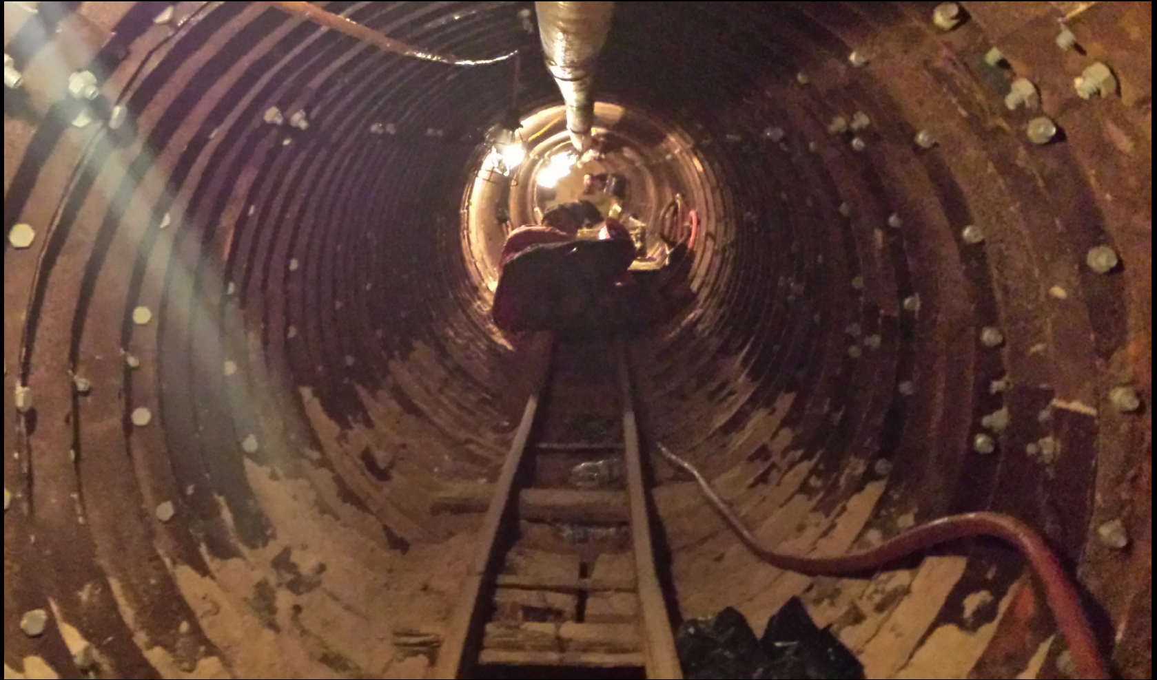
Interior view of 52-inch steel liner tunnel under I-45
