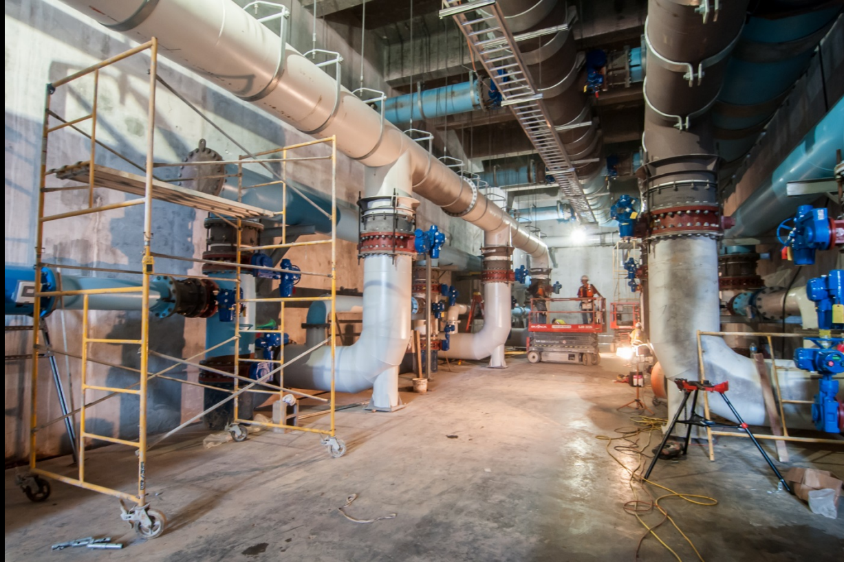
Granulated Activated Carbon Building – Process water piping installation
