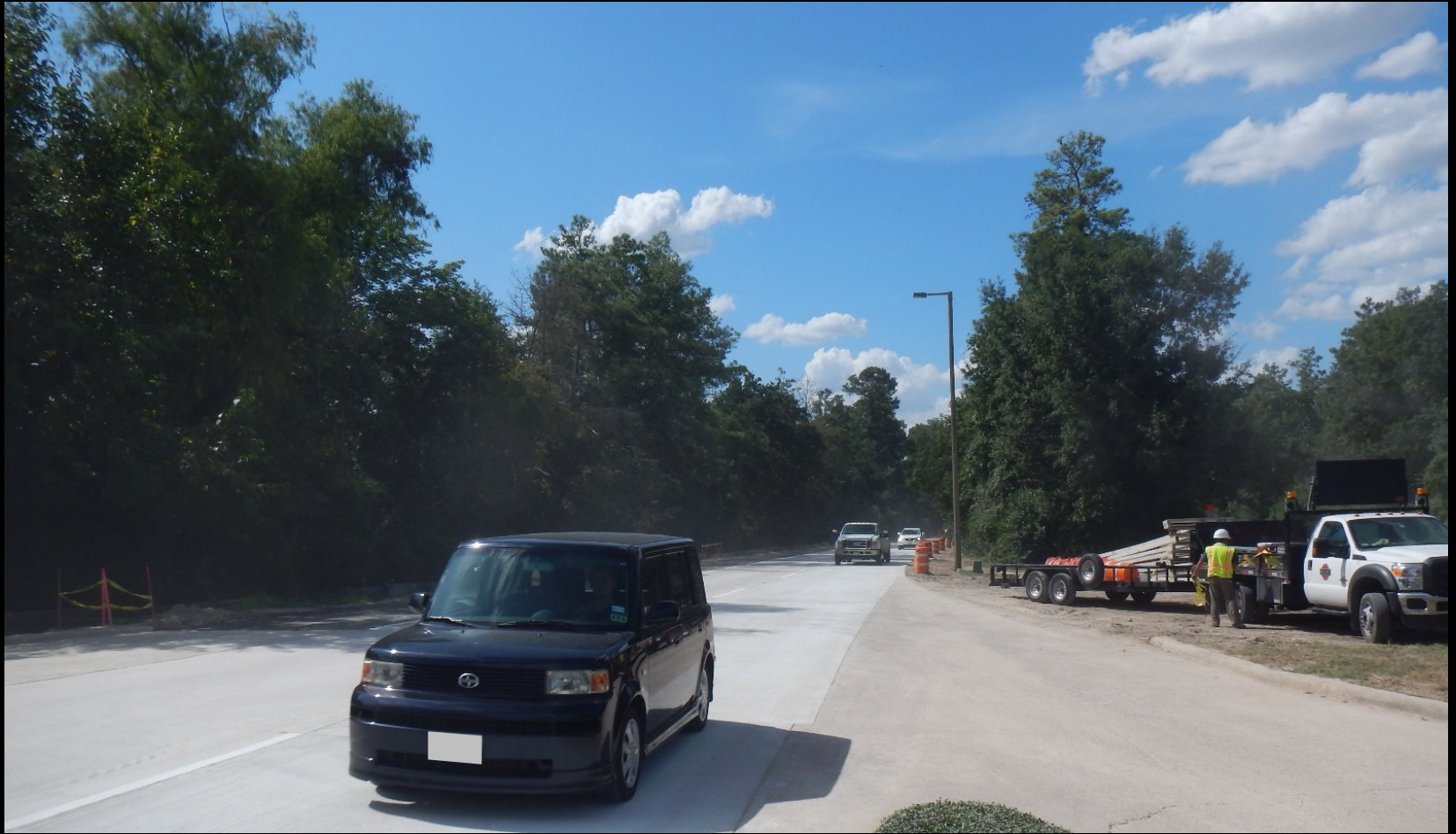
Traffic restoration at Grogans Mill Rd. and Millpark Dr.
