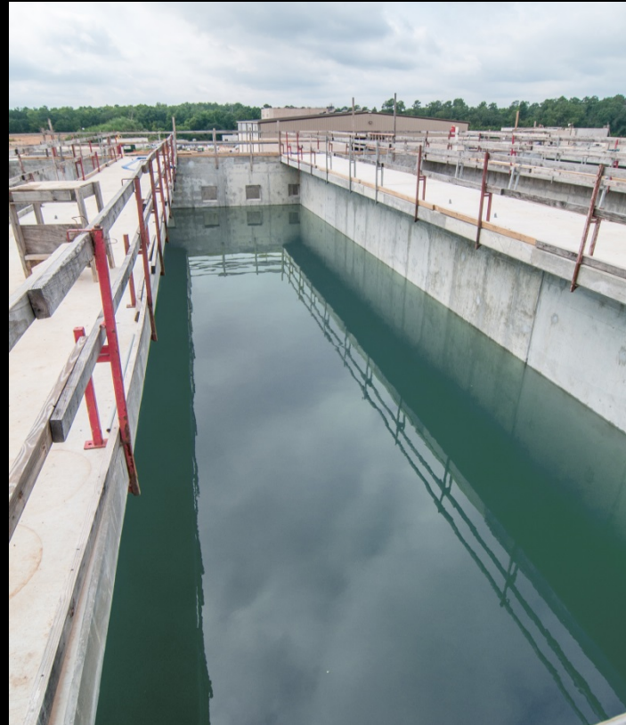
Pretreatment – Leak testing procedure
