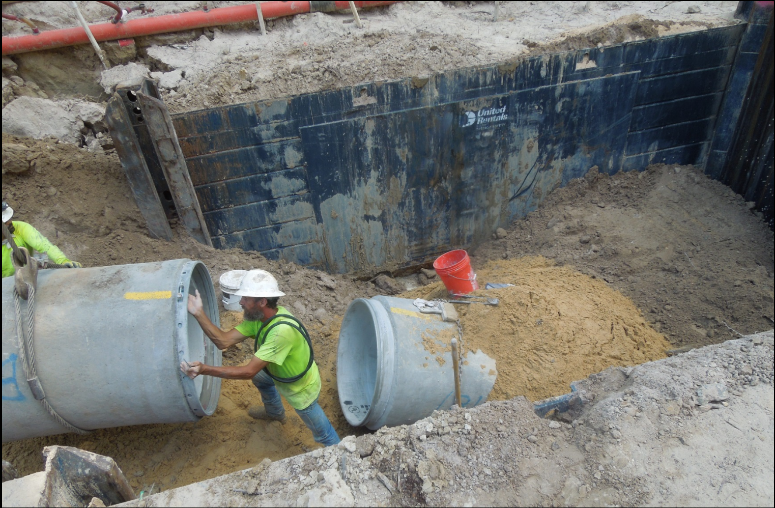
36-inch open cut pipe installation along Entergy easement
