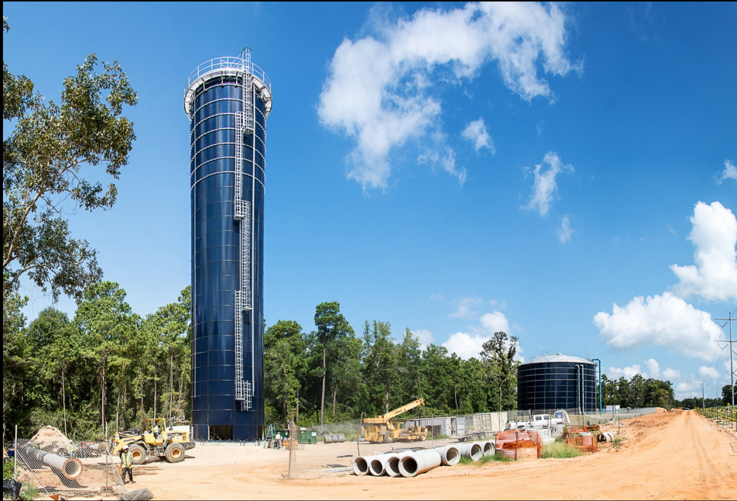
Standpipe tank installation – 120 feet tall and 25 feet in diameter
