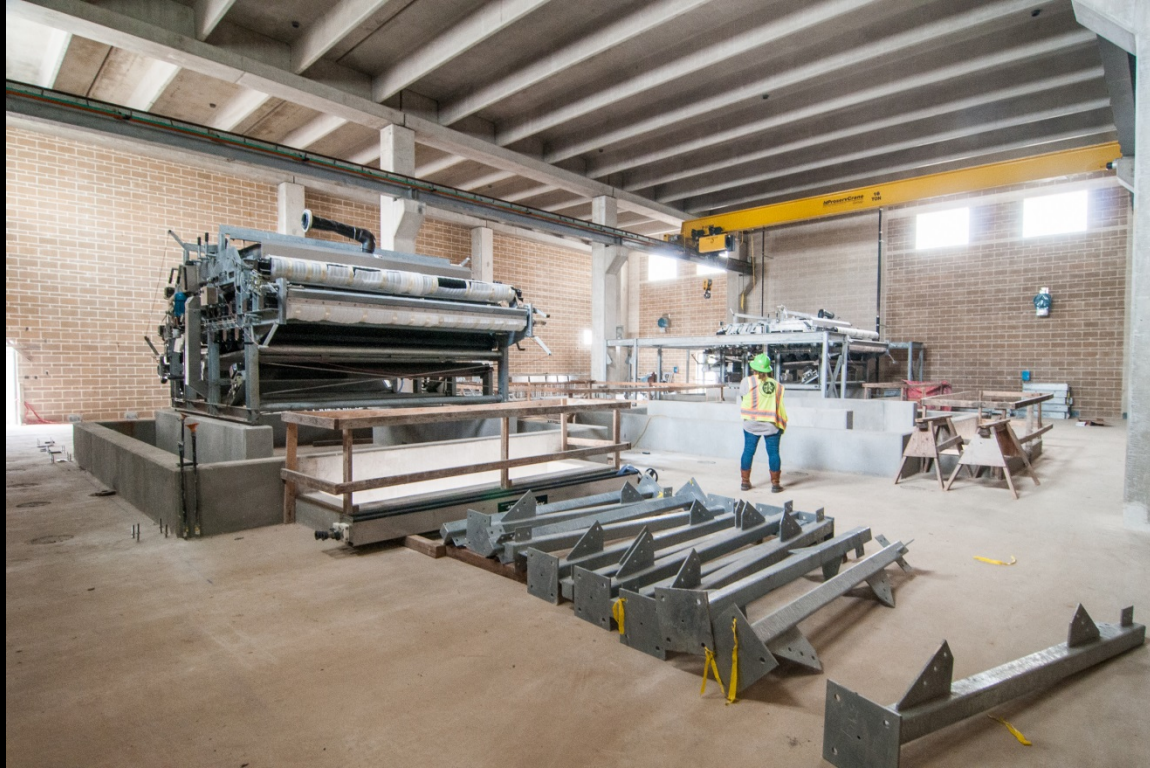
Dewatering Building – Belt filter press installation
