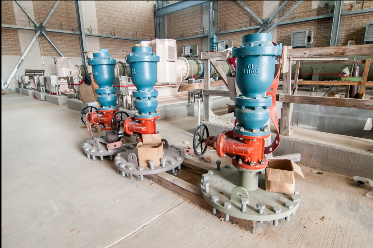
Raw Water Intake & Pump Station – Pressure reducing valve assemblies
