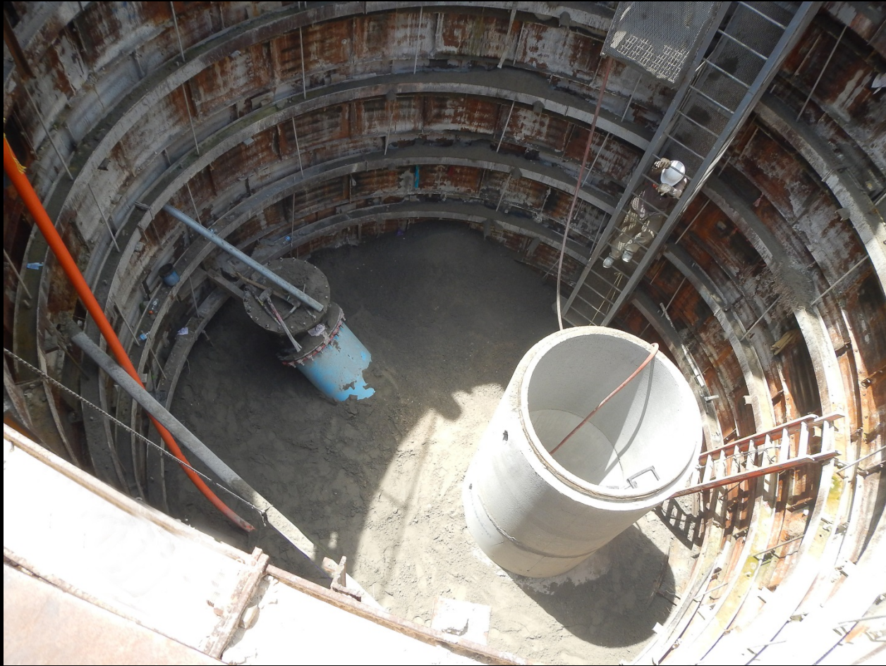
Backfilling of bore pit for Woodlands Waterway crossing
