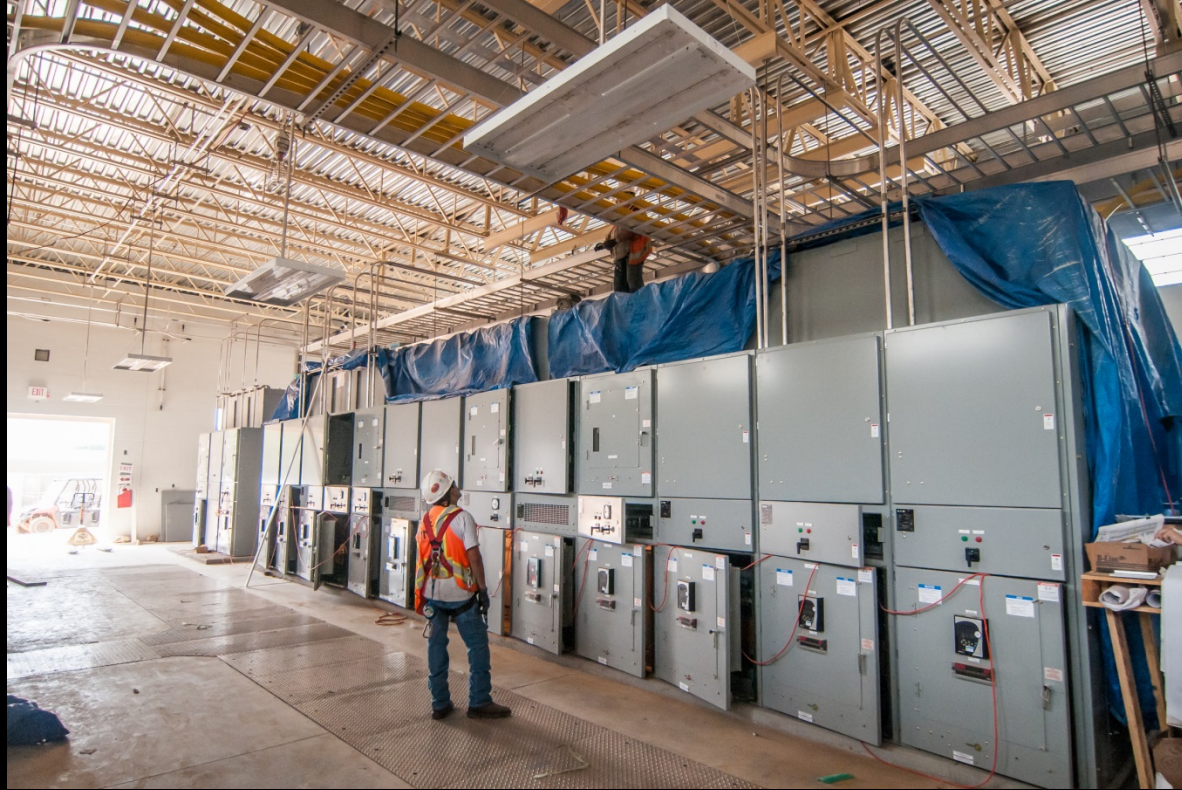
High Service Pump Station – Electrical gear installation
