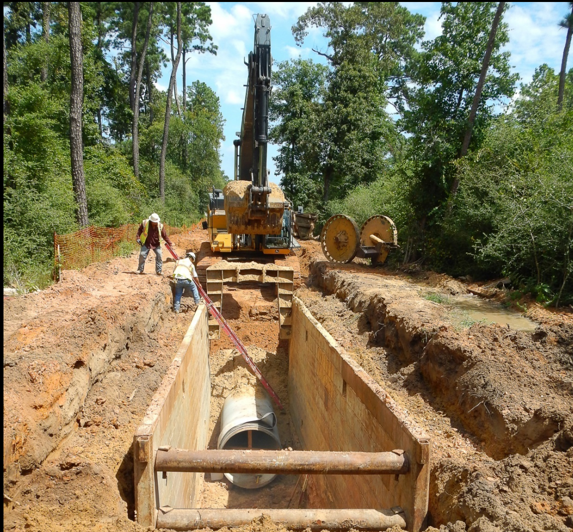
54-inch pipe installation along Sendera Ranch Road
