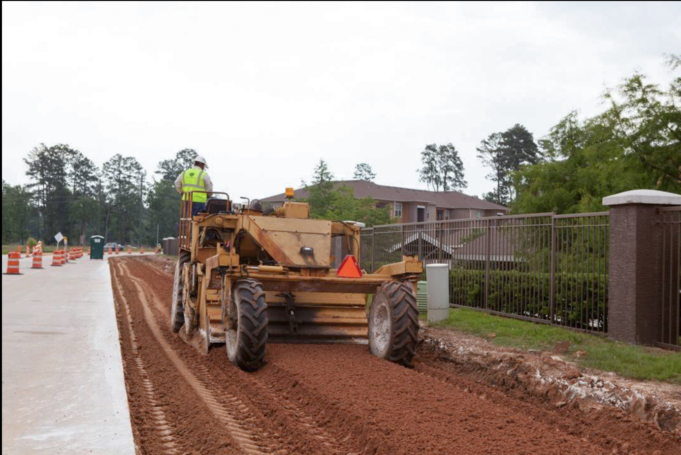
Pavement subgrade stabilization along Research Forest Drive
