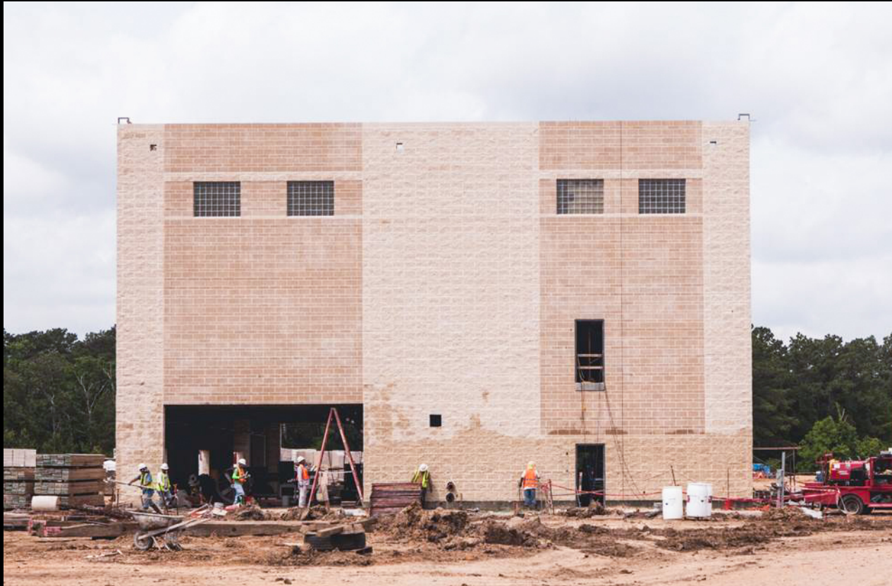
Dewatering Building – Masonry installation
