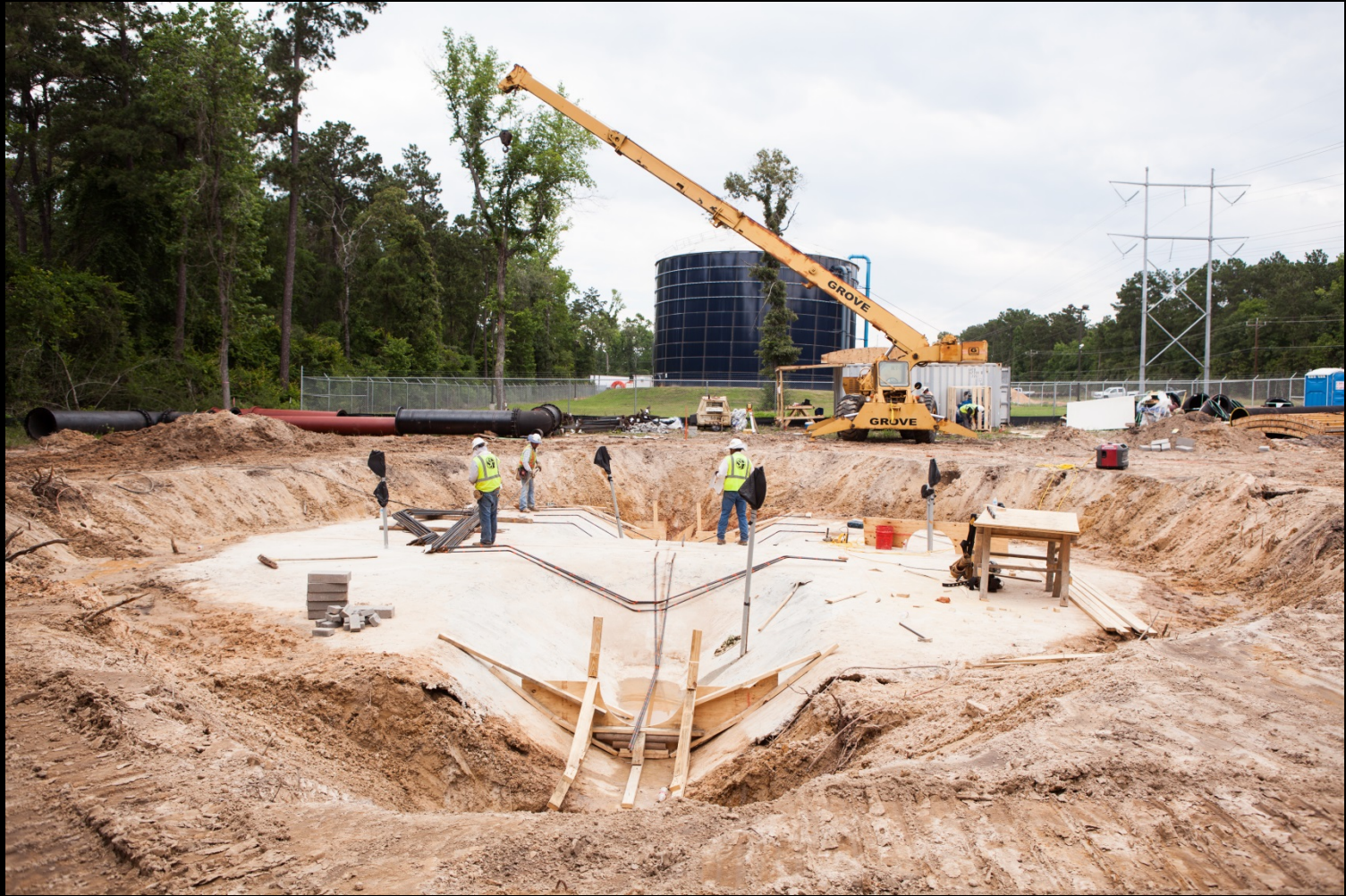
Reinforced steel and formwork installation
