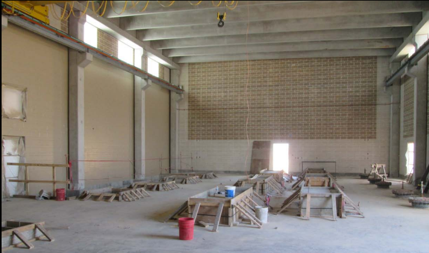
Membrane Building – Previous progress photograph
