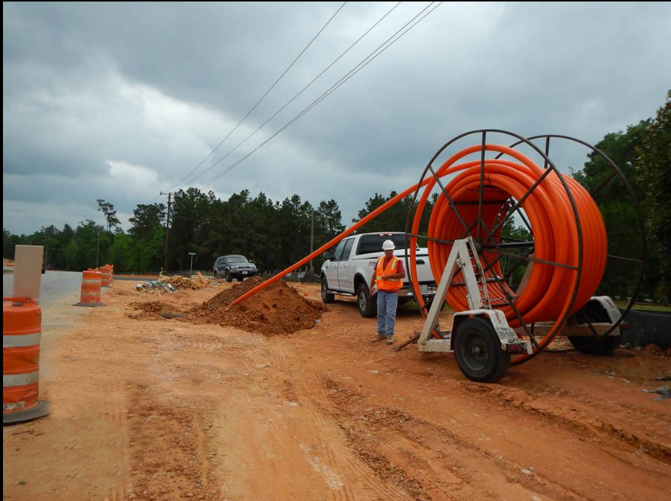
Fiber optic conduit installation along Fish Creek Thoroughfare
