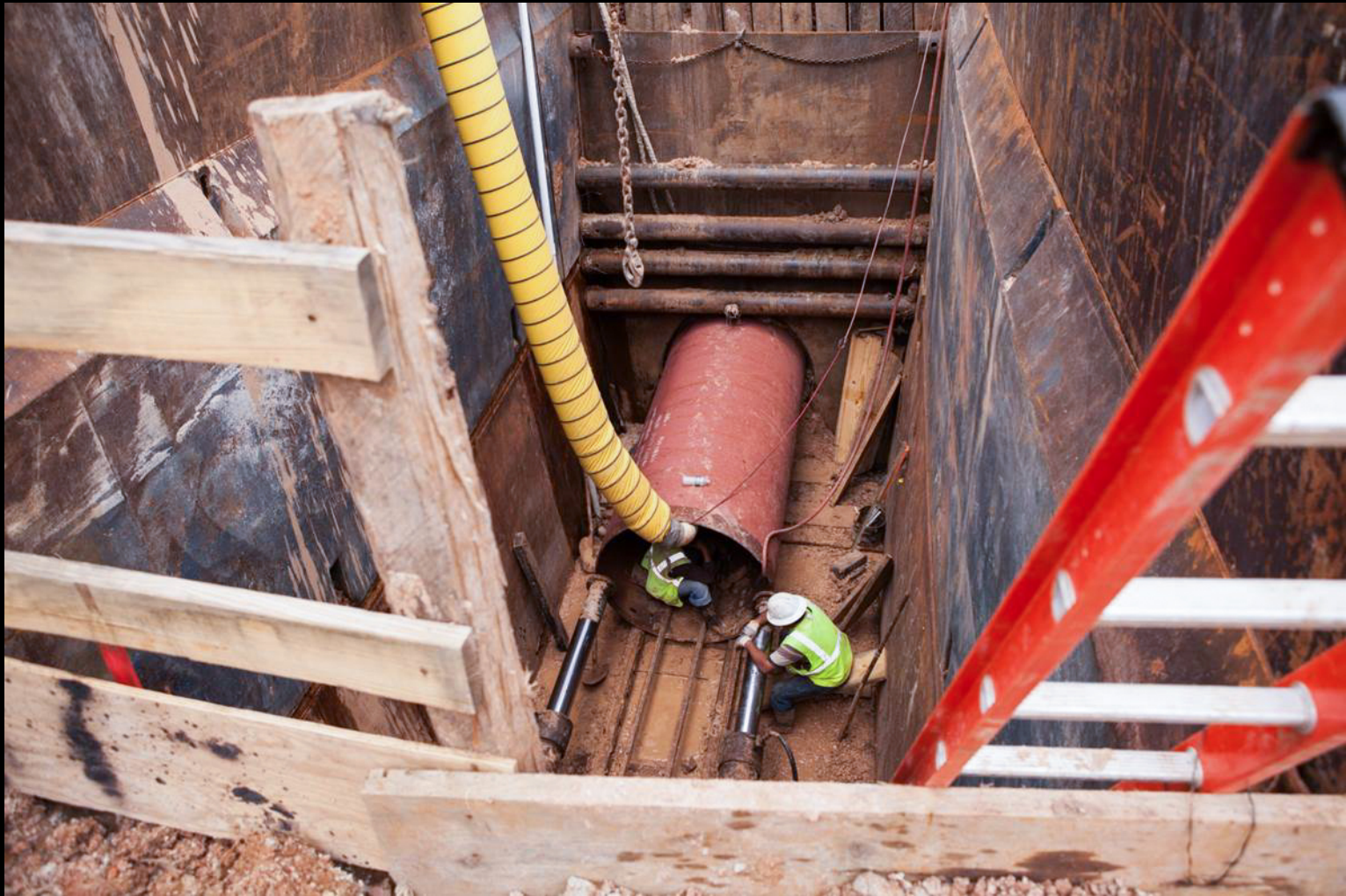
48-inch steel casing installation along Entergy easement
