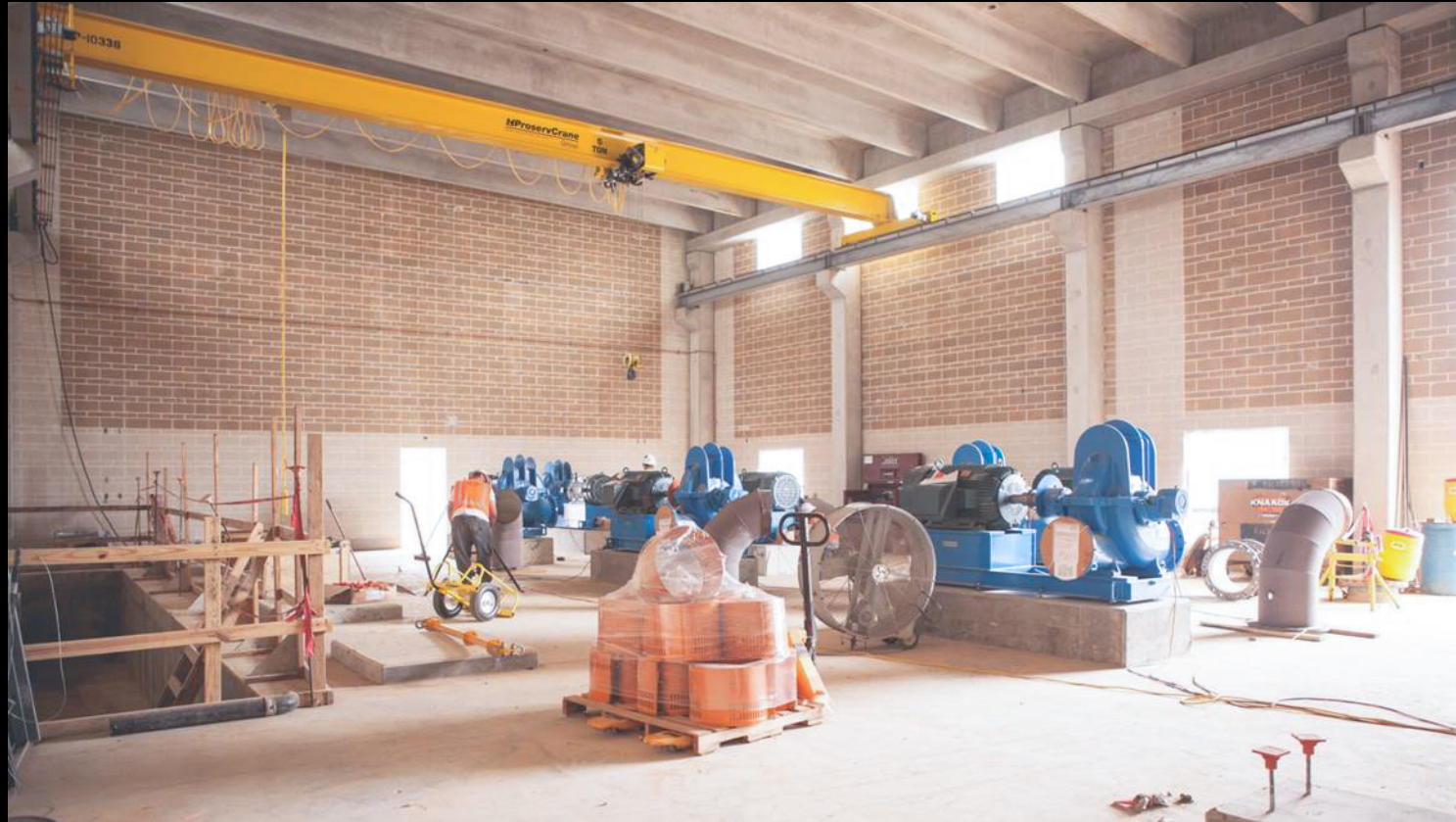
Membrane Building – Installation of membrane feed pumps
