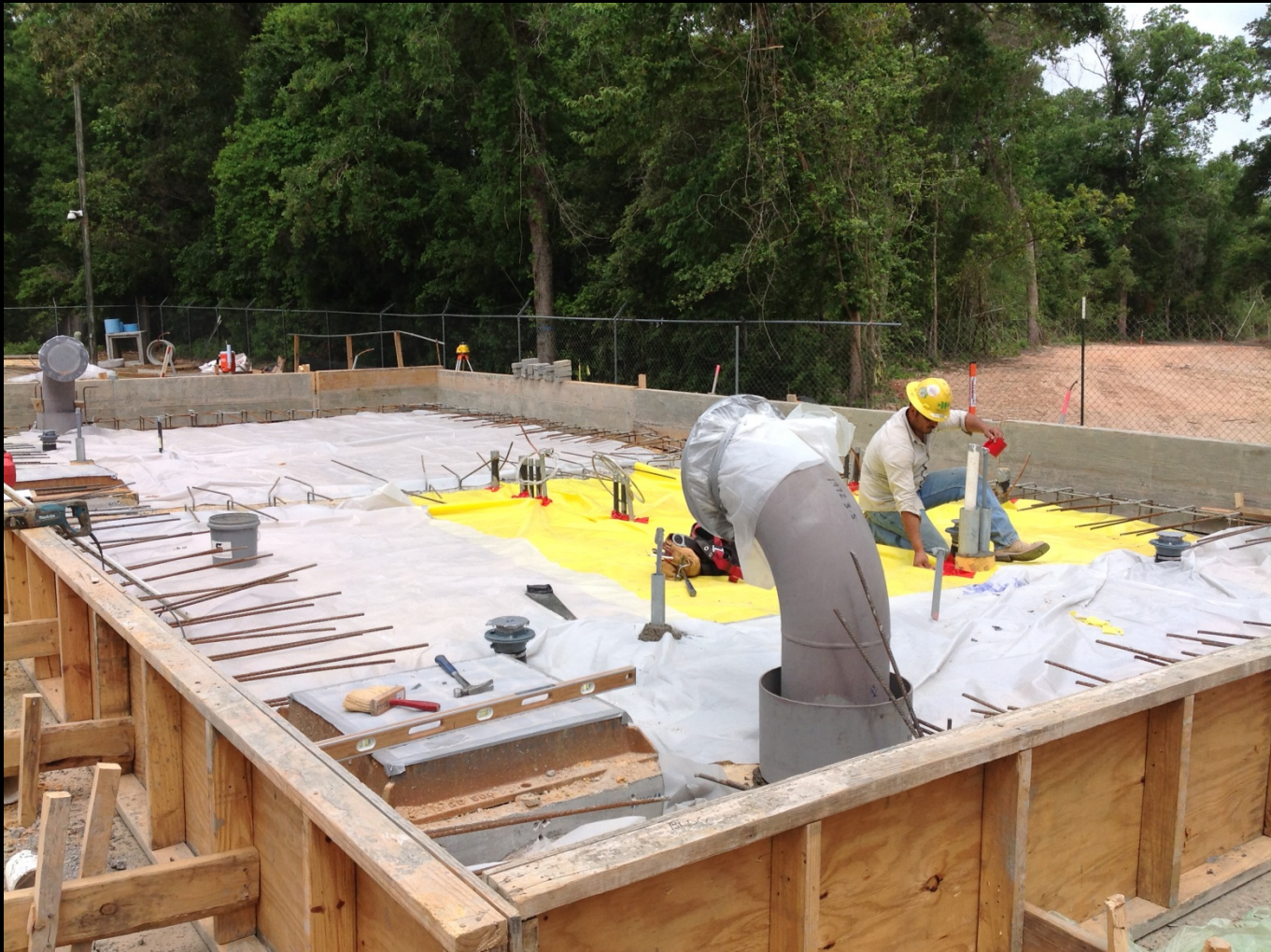
Flow Control Pressure Slab installation at Conroe Water Plant No. 14
