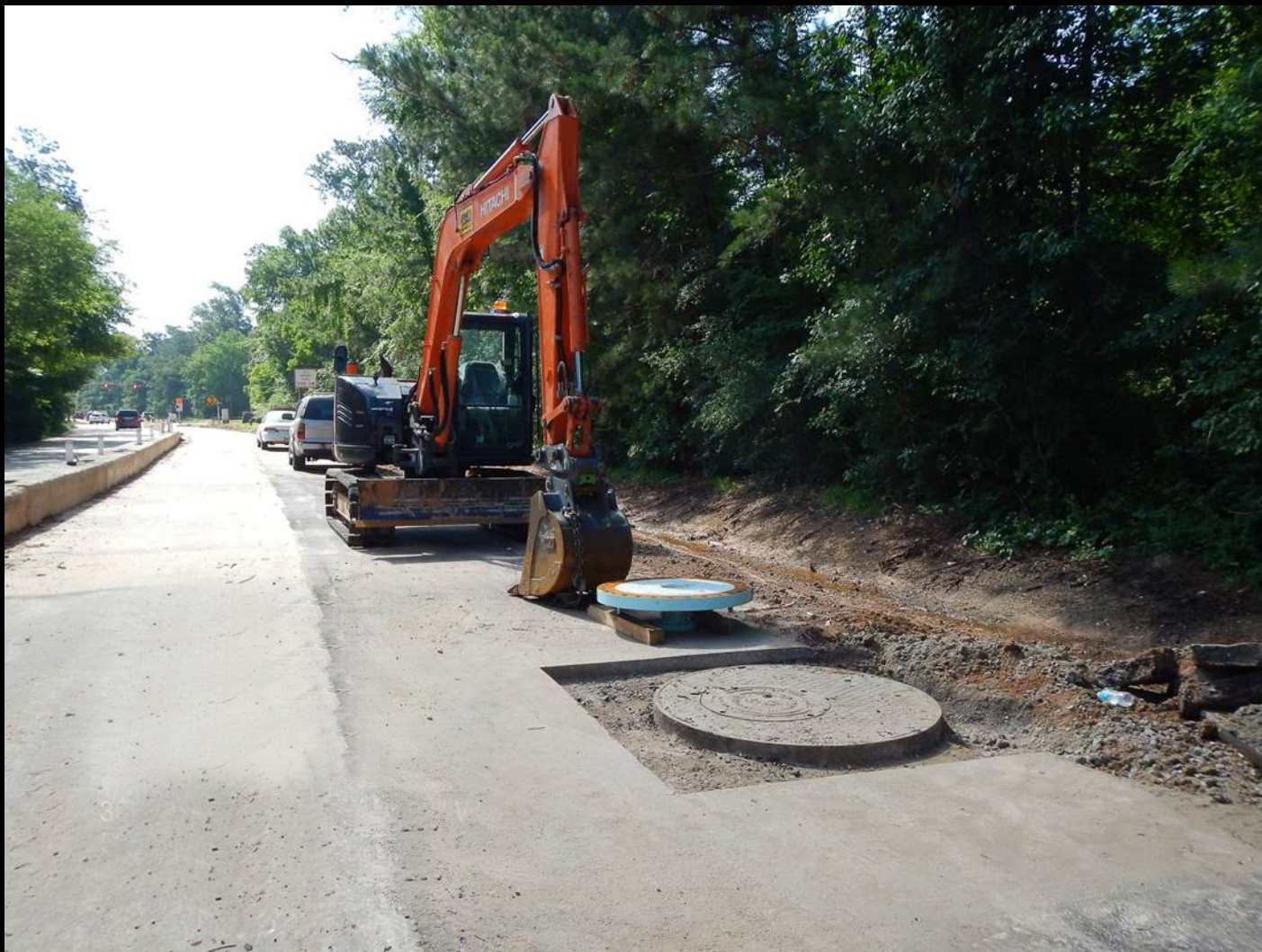
Manhole installation along Research Forest Drive
