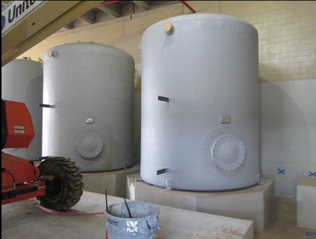
Chemical Building – Installation of sodium hypochlorite tanks
