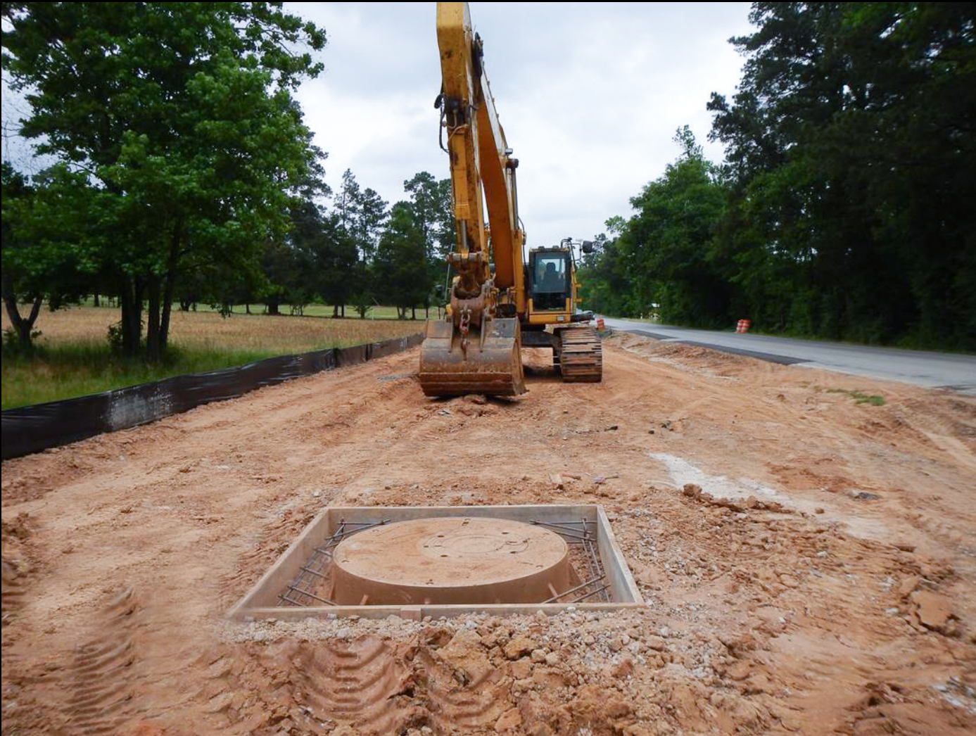
Manhole installation - McCaleb Road
