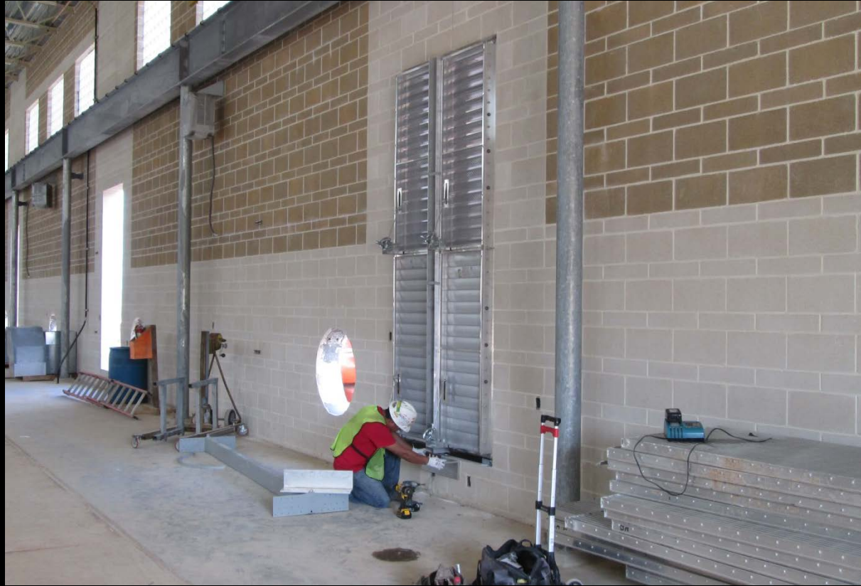
High Service Pump Station - Previous progress photograph
