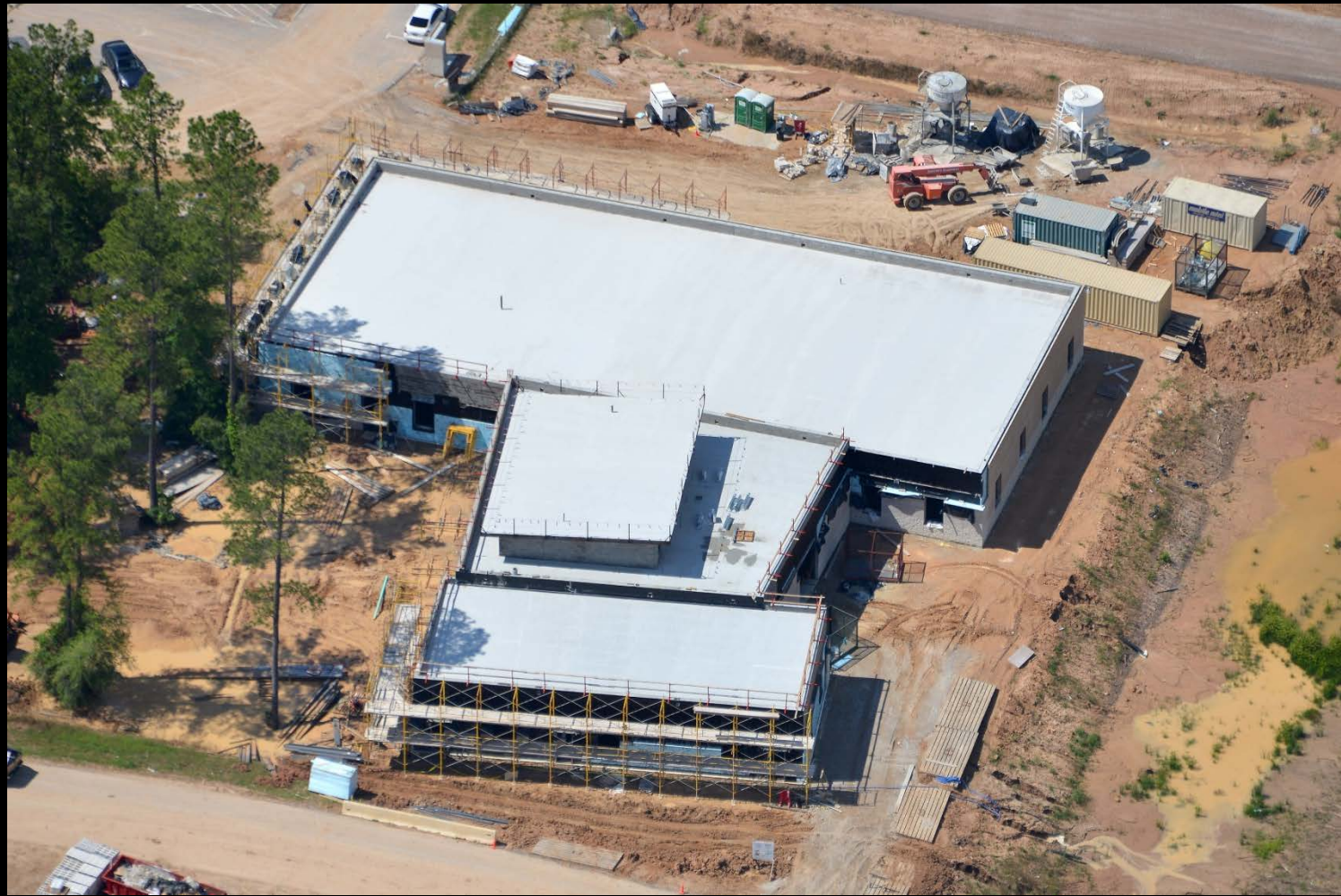
Operations Building – Completion of structural systems
