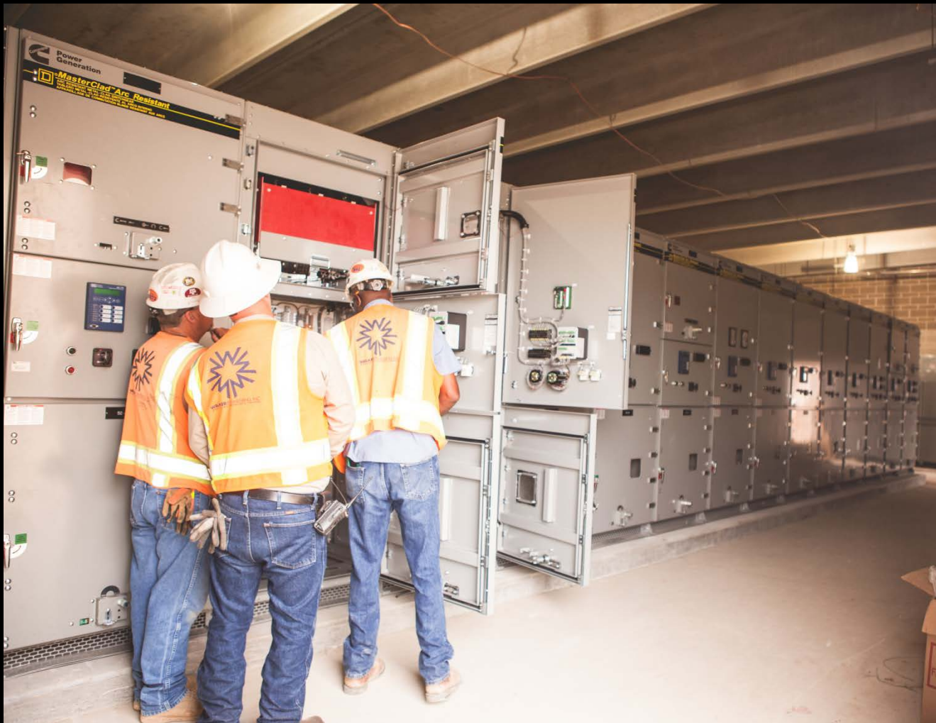
Electrical Facilities – Main electrical switchgear installation
