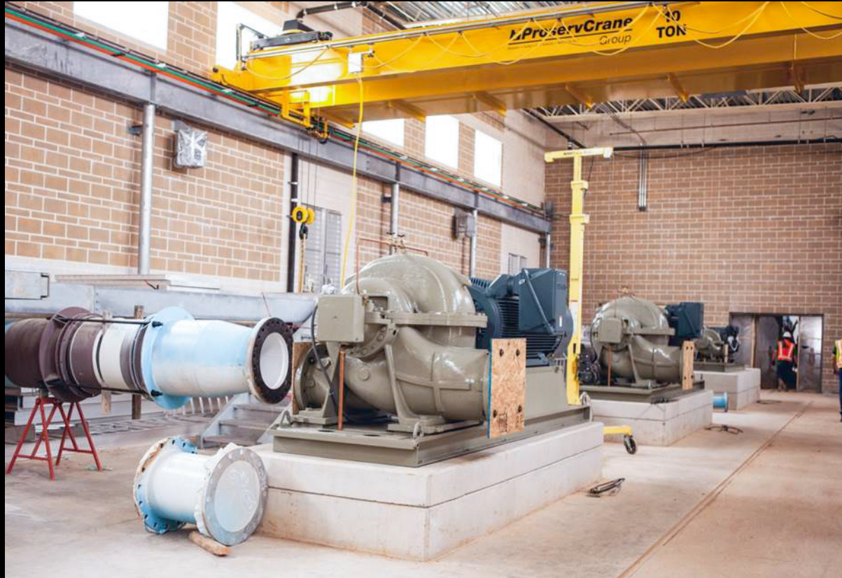
High Service Pump Station – Installation of pumps
