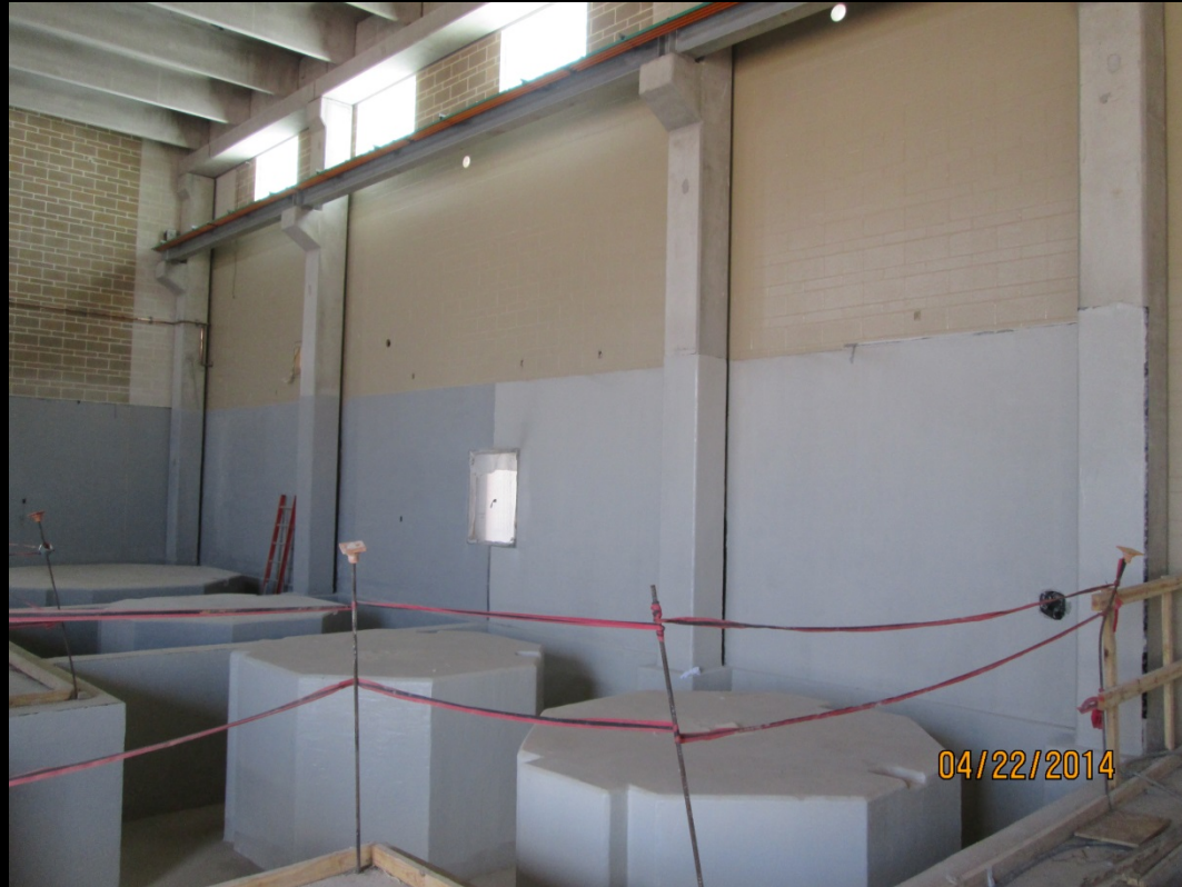
Chemical Building – Previous progress photograph
