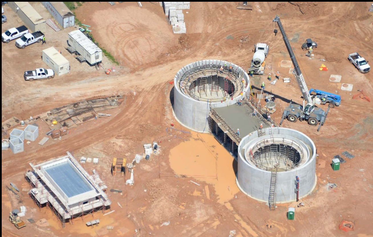
Sludge Thickeners – Pump room concrete roof installation
