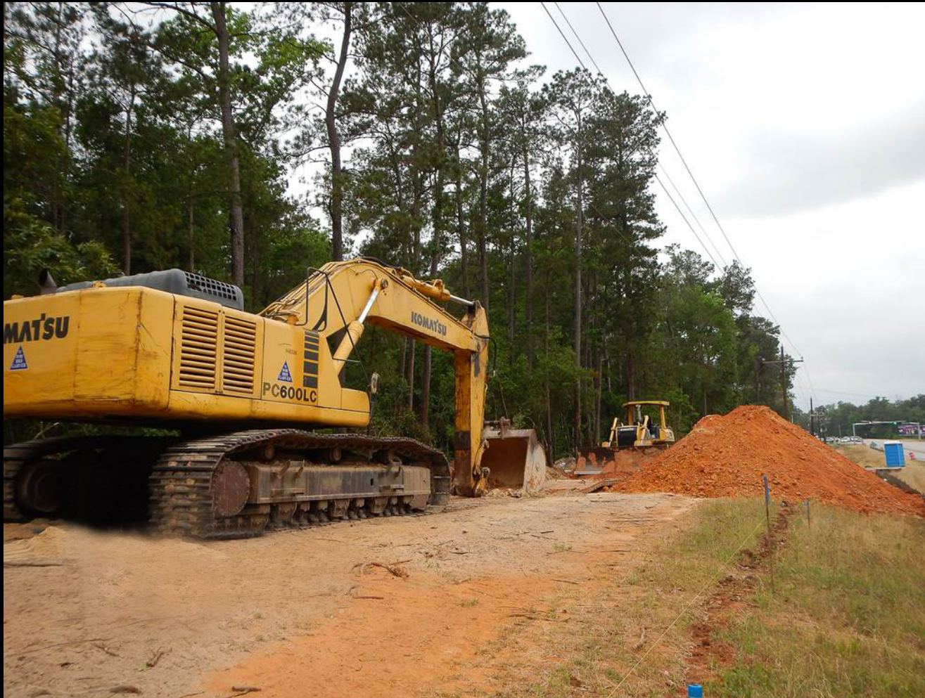
24-inch pipe installation along FM 830
