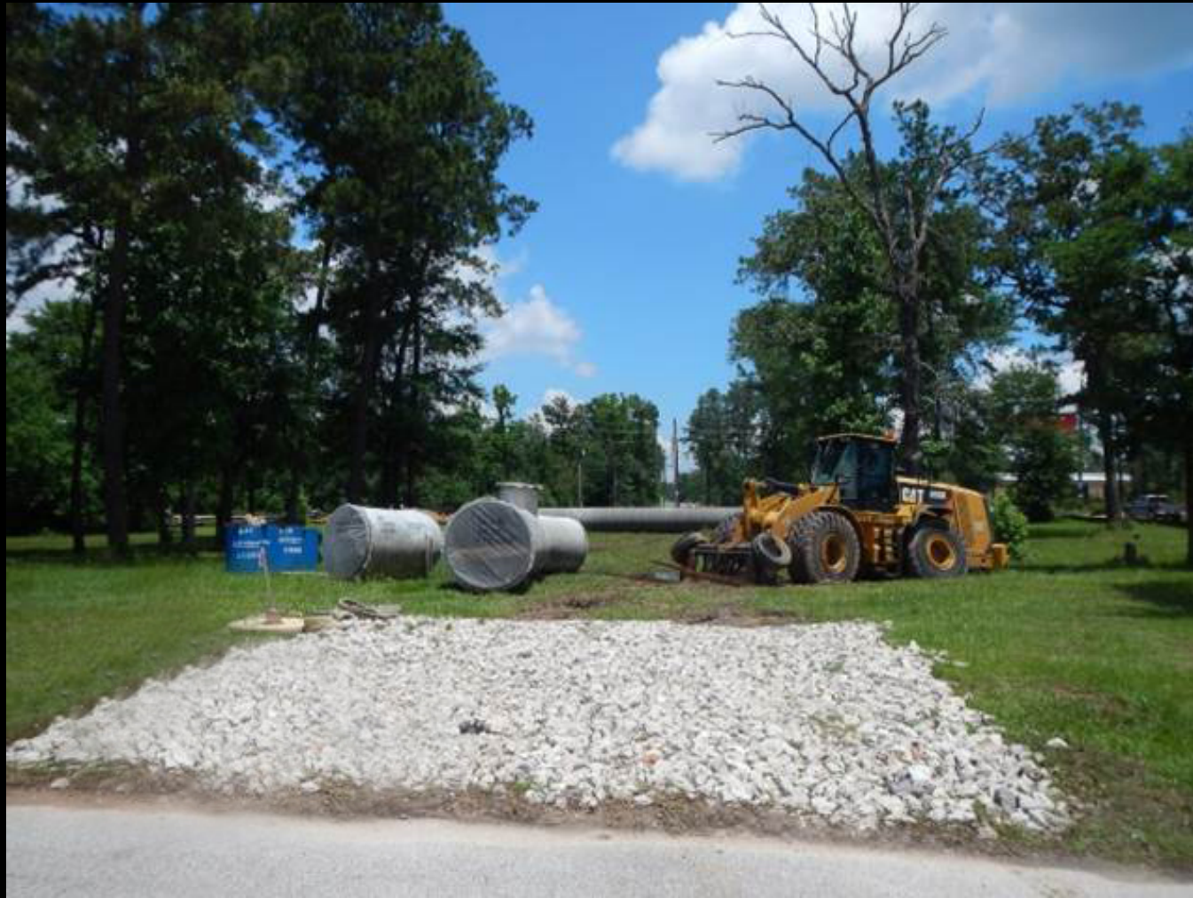
54-inch pipe installation along Sendera Ranch Road
