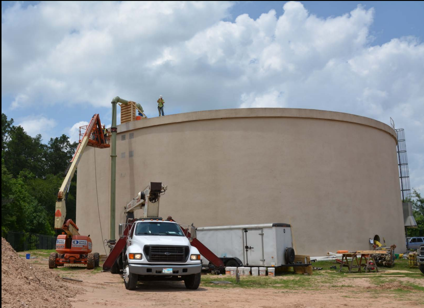
Riser pipe installation at Woodlands Water Plant No. 5
