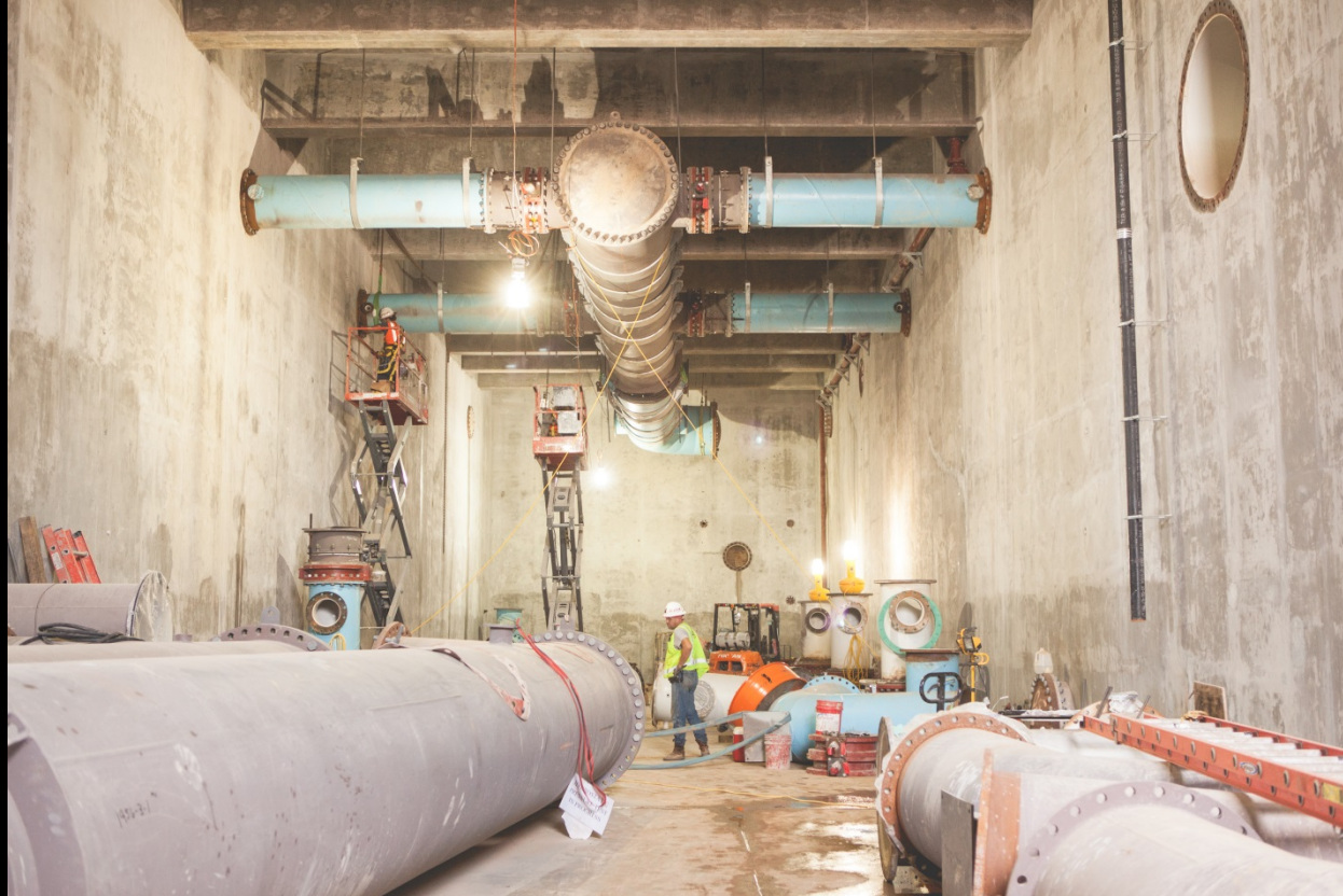
Granulated Activated Carbon Contactors – Pipe gallery installation
