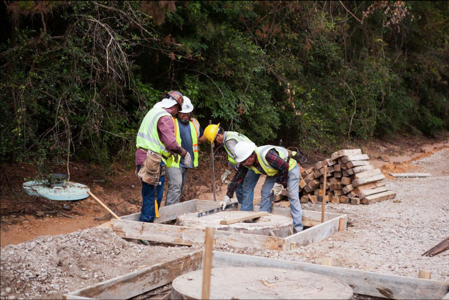
Manhole installation along Research Forest Drive
