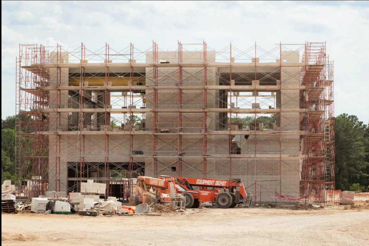
Dewatering Building – Previous progress photograph
