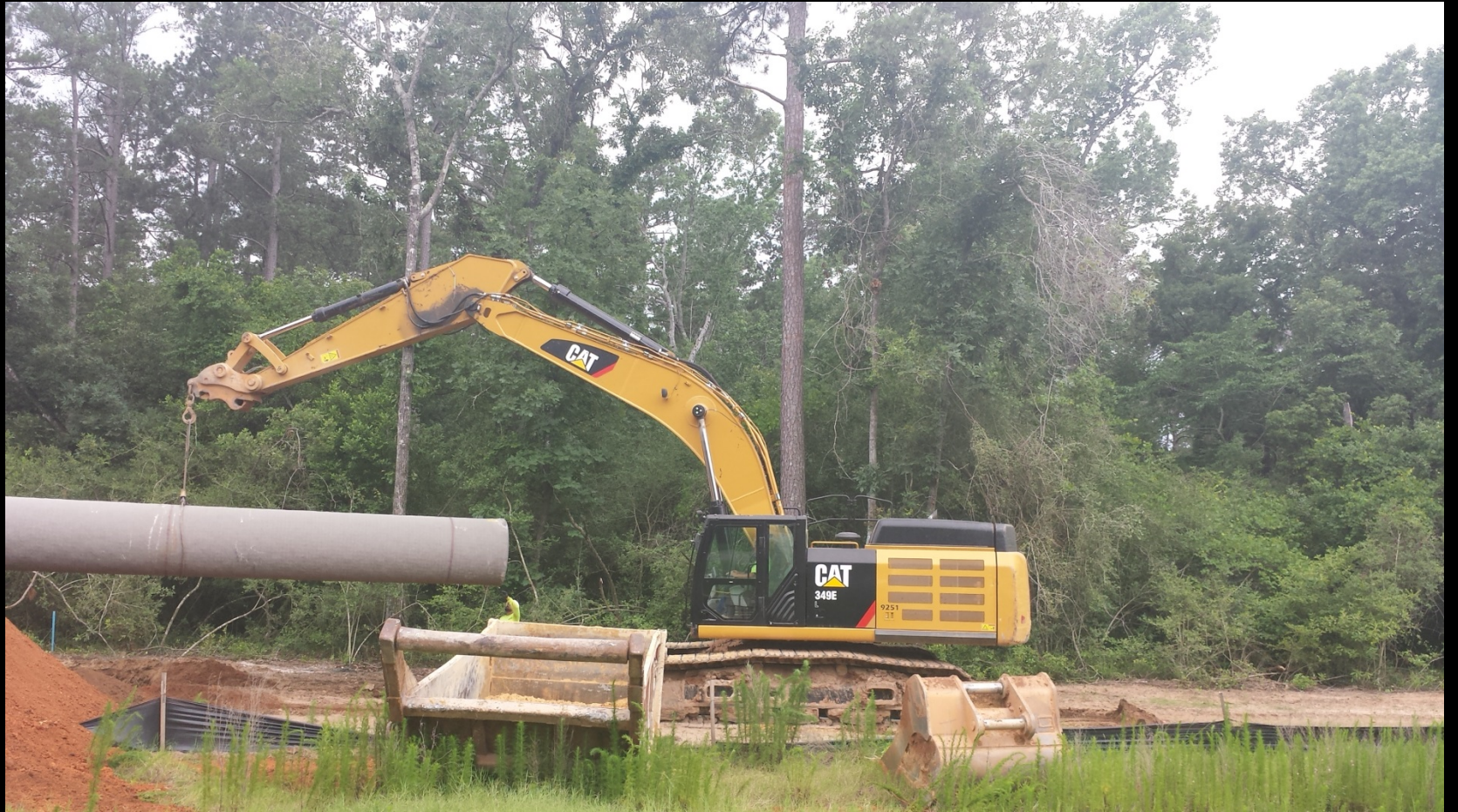
42-inch pipe installation along GRP Access Road
