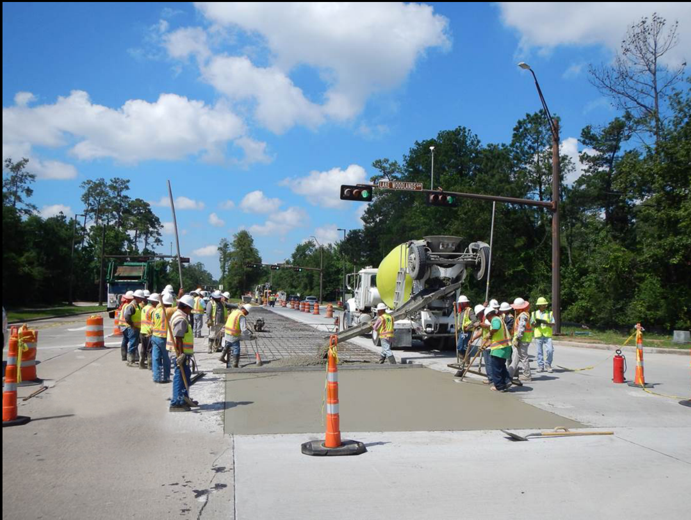
Concrete placement along Grogans Mill Road
