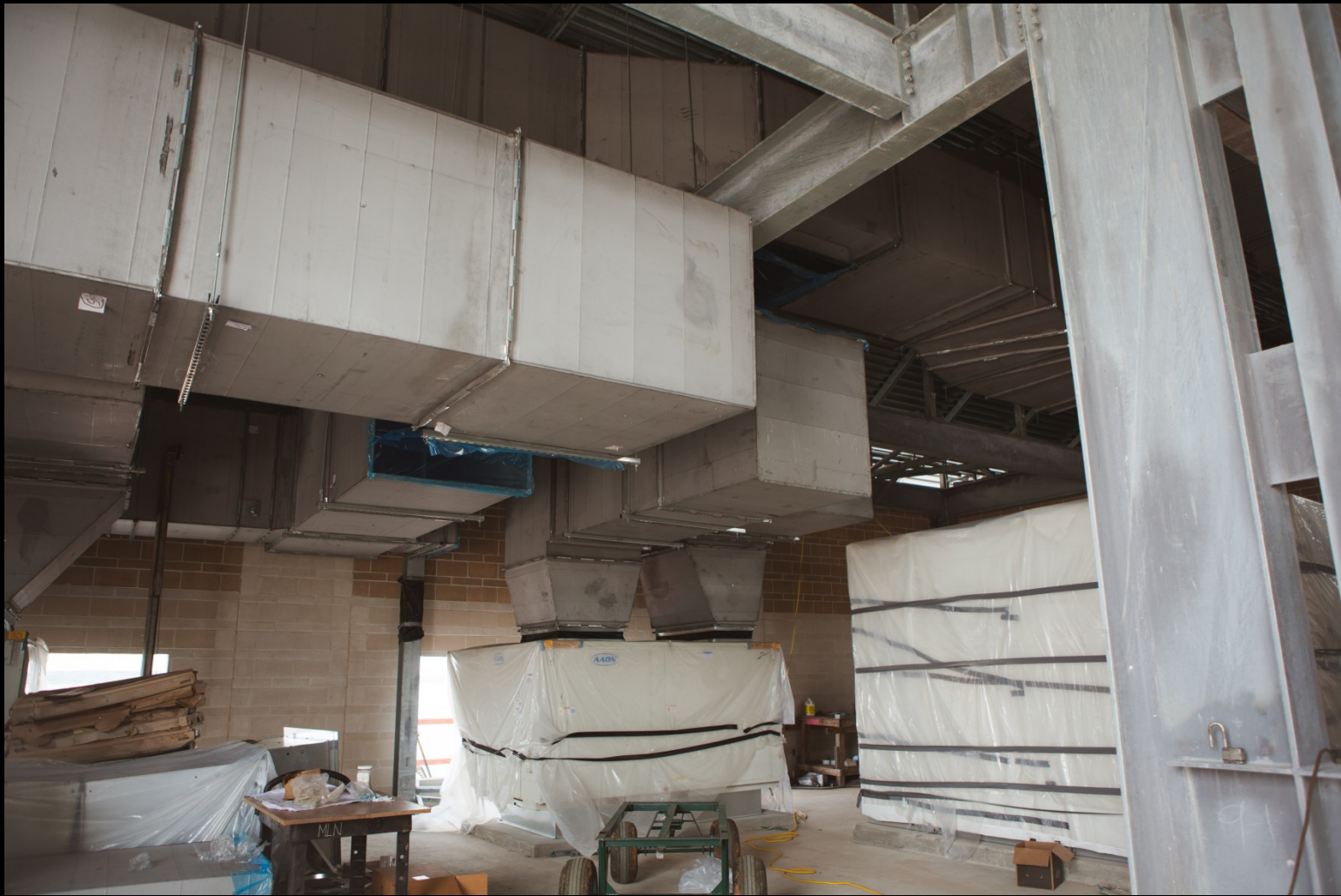
Raw Water Intake & Pump Station – HVAC installation
