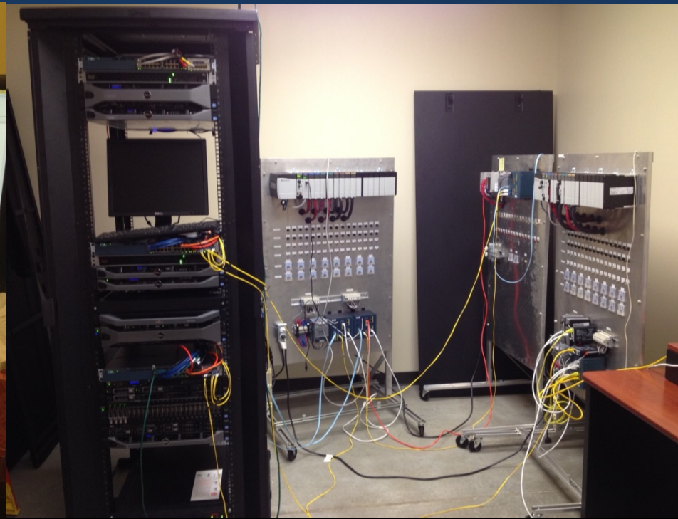
Development System Server Rack & PLCs
