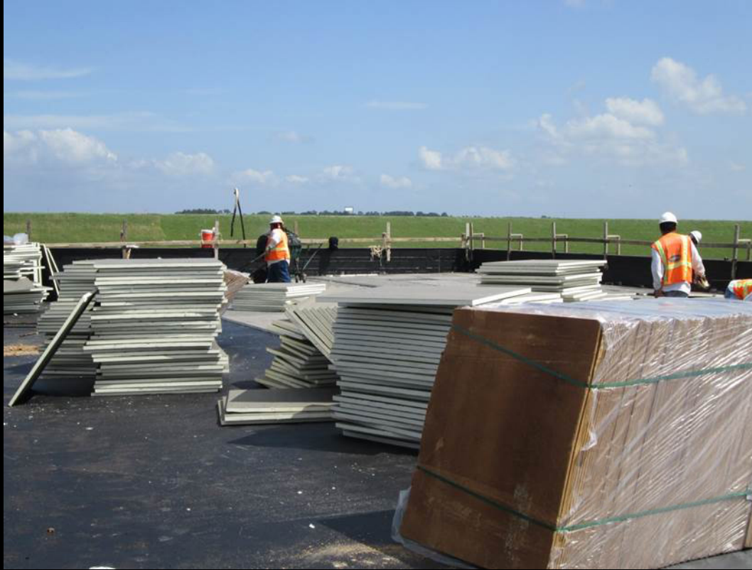
Blower Building – Roofing installation
