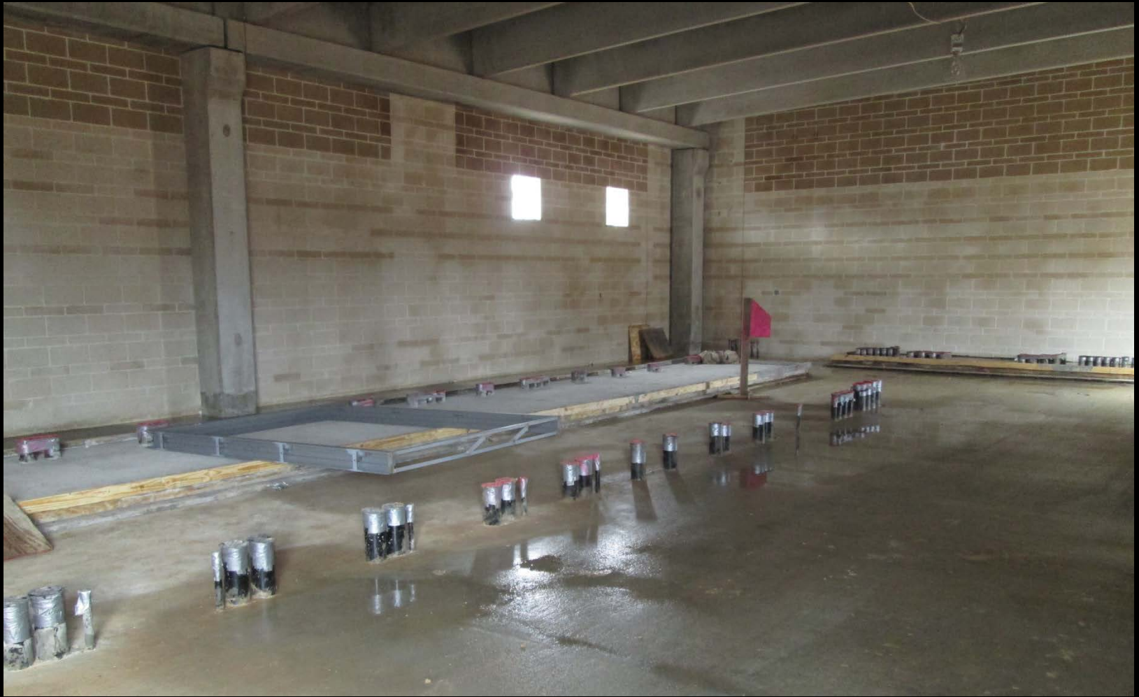
Electrical Facilities – Previous progress photograph
