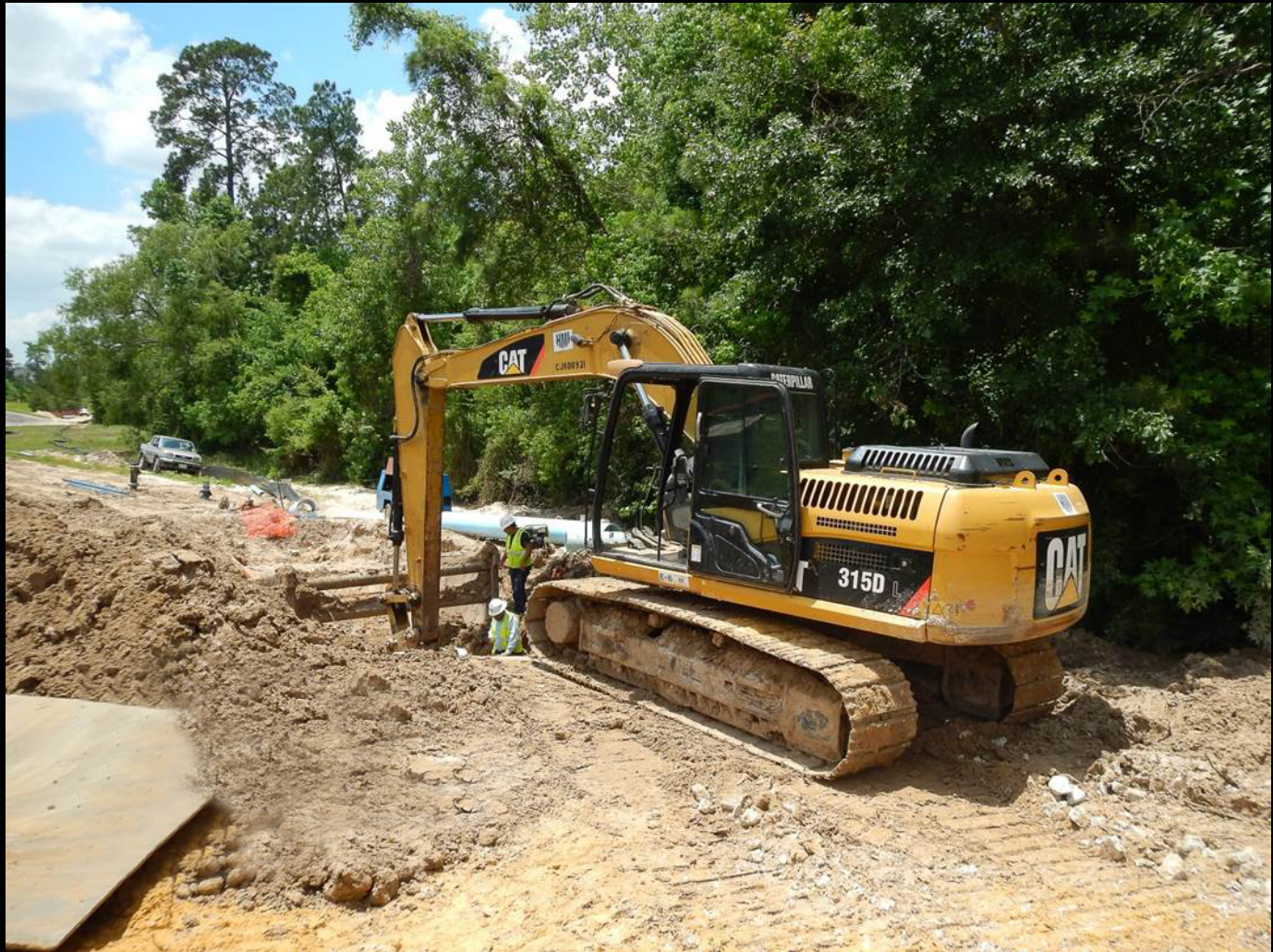
24-inch pipe and fiber optic conduit installation on Gosling
