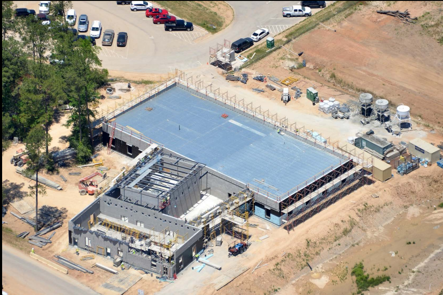
Operations Building – Previous progress photograph
