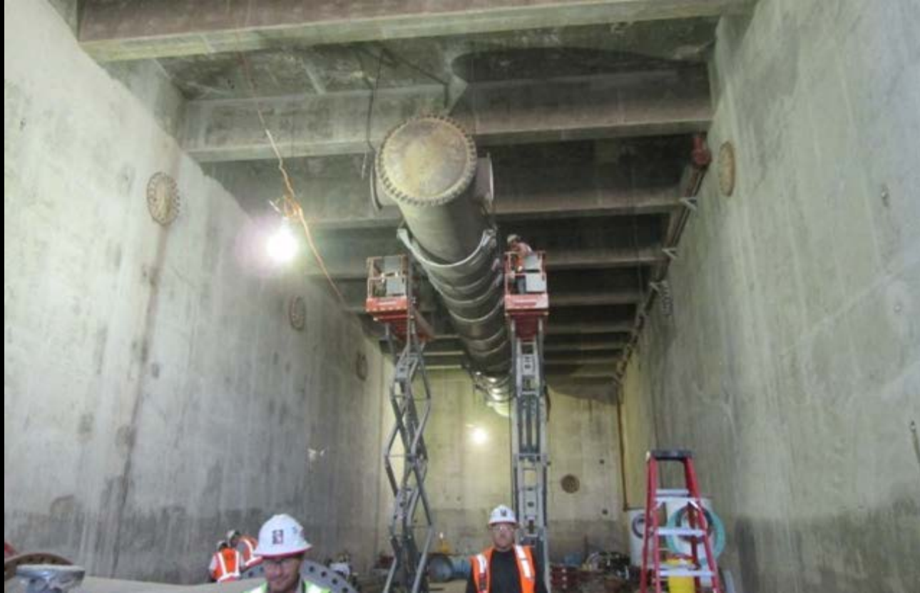
Granulated Activated Carbon Contactors – Previous progress photograph
