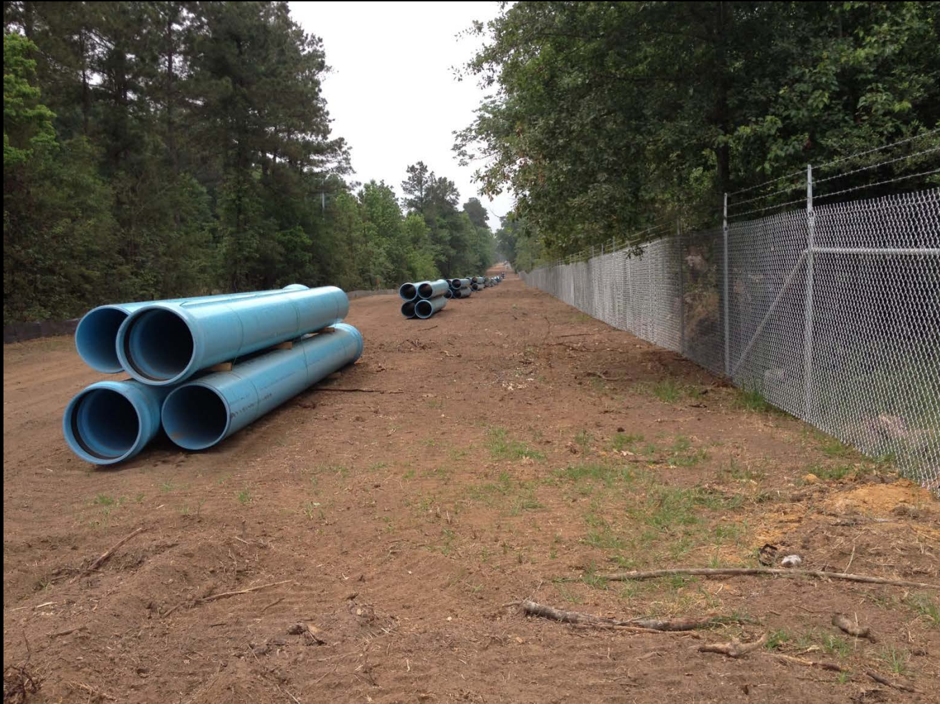
Staging of pipe materials along Girl Scout property
