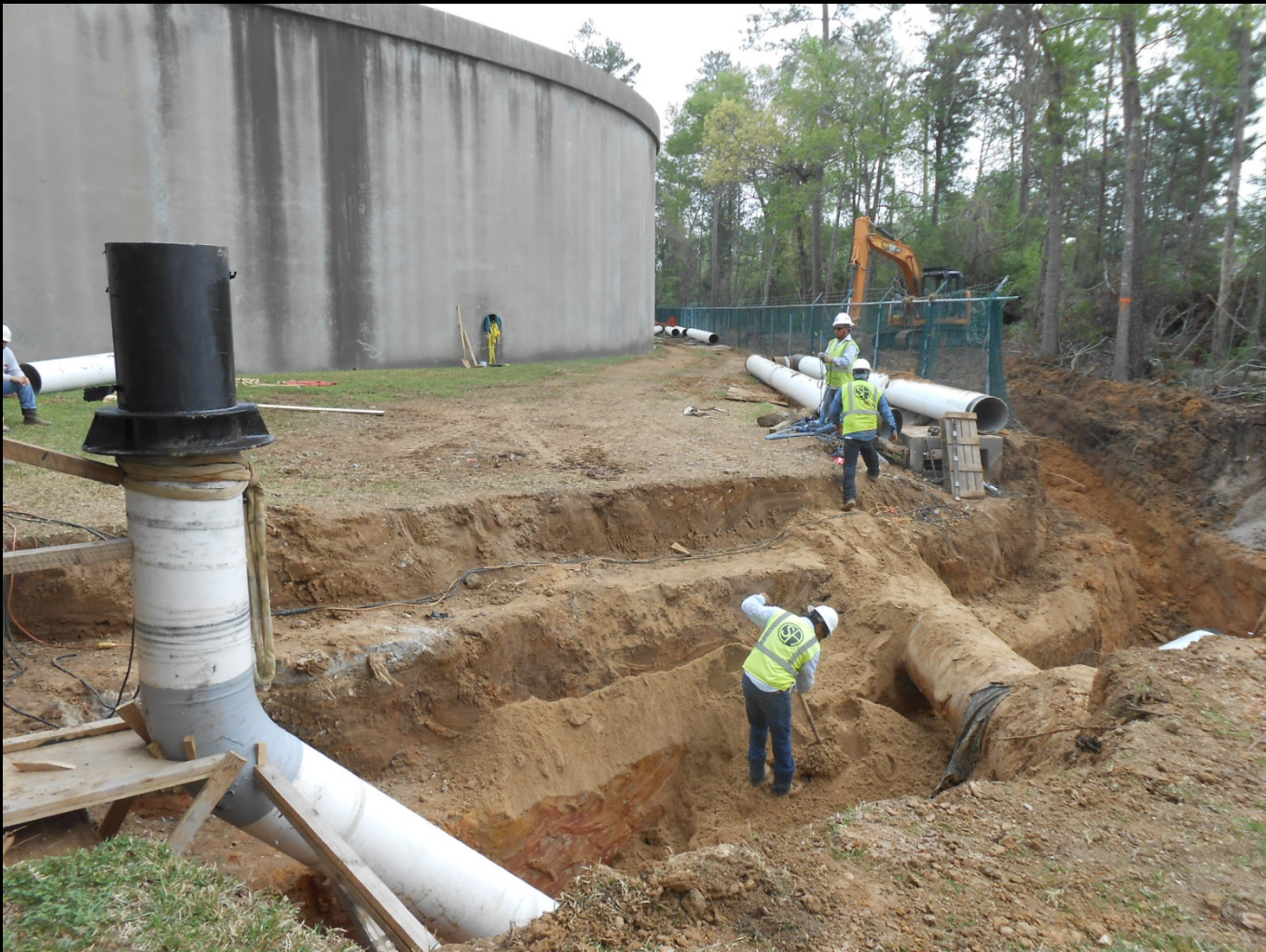
20-inch ground storage tank connection at SJRA Water Plant No. 2
