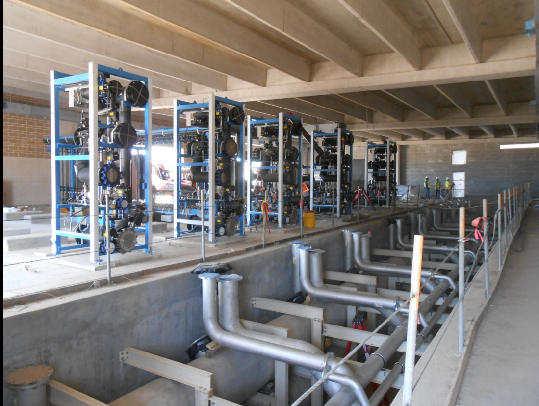
Membrane Building – Installation of membrane equipment racks and piping
