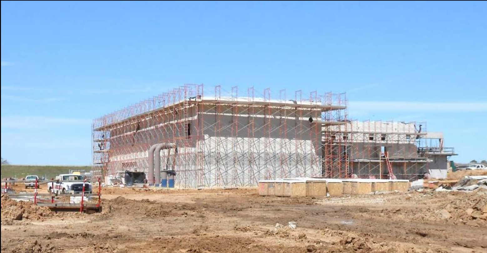
Granulated Activated Carbon Contactors – Previous progress photograph
