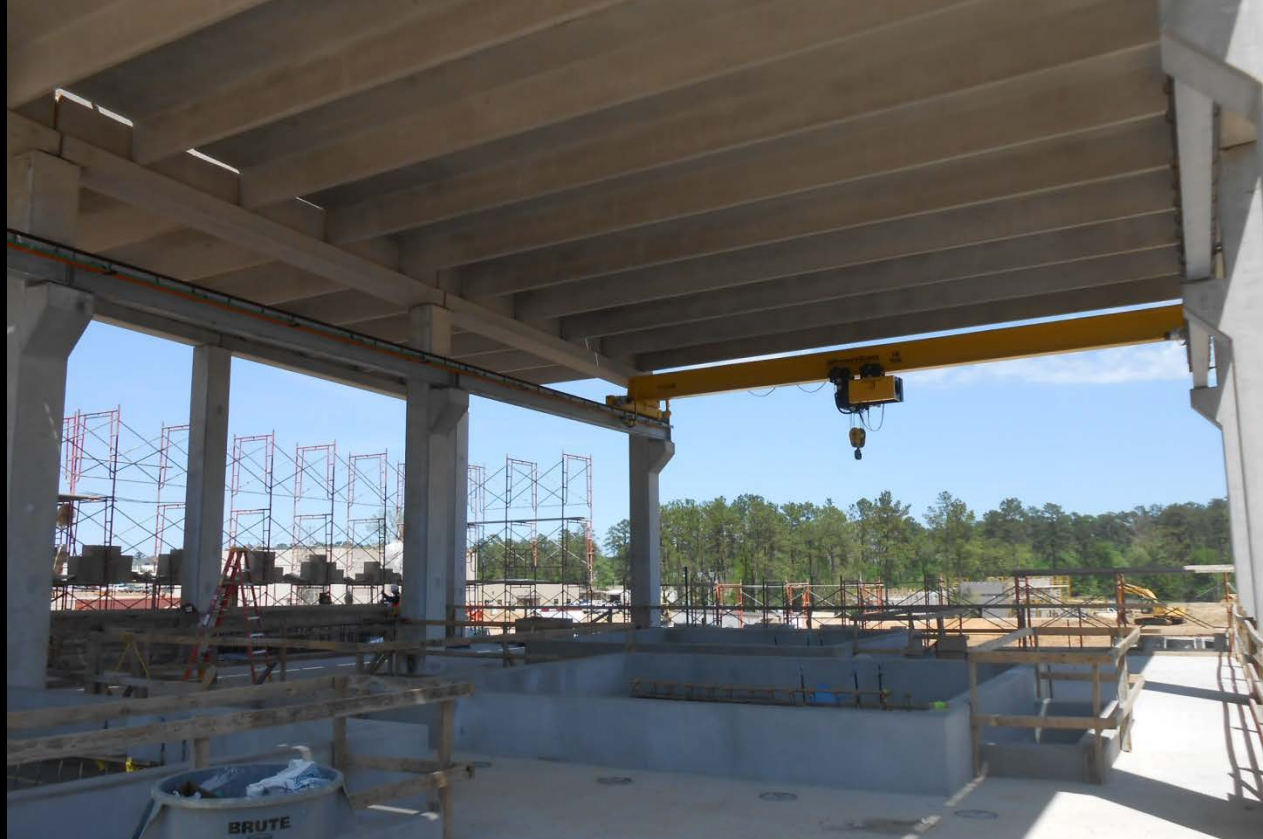
Dewatering Building – Second floor masonry installation
