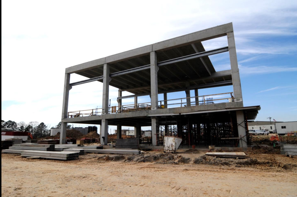
Dewatering Building – Previous progress photograph
