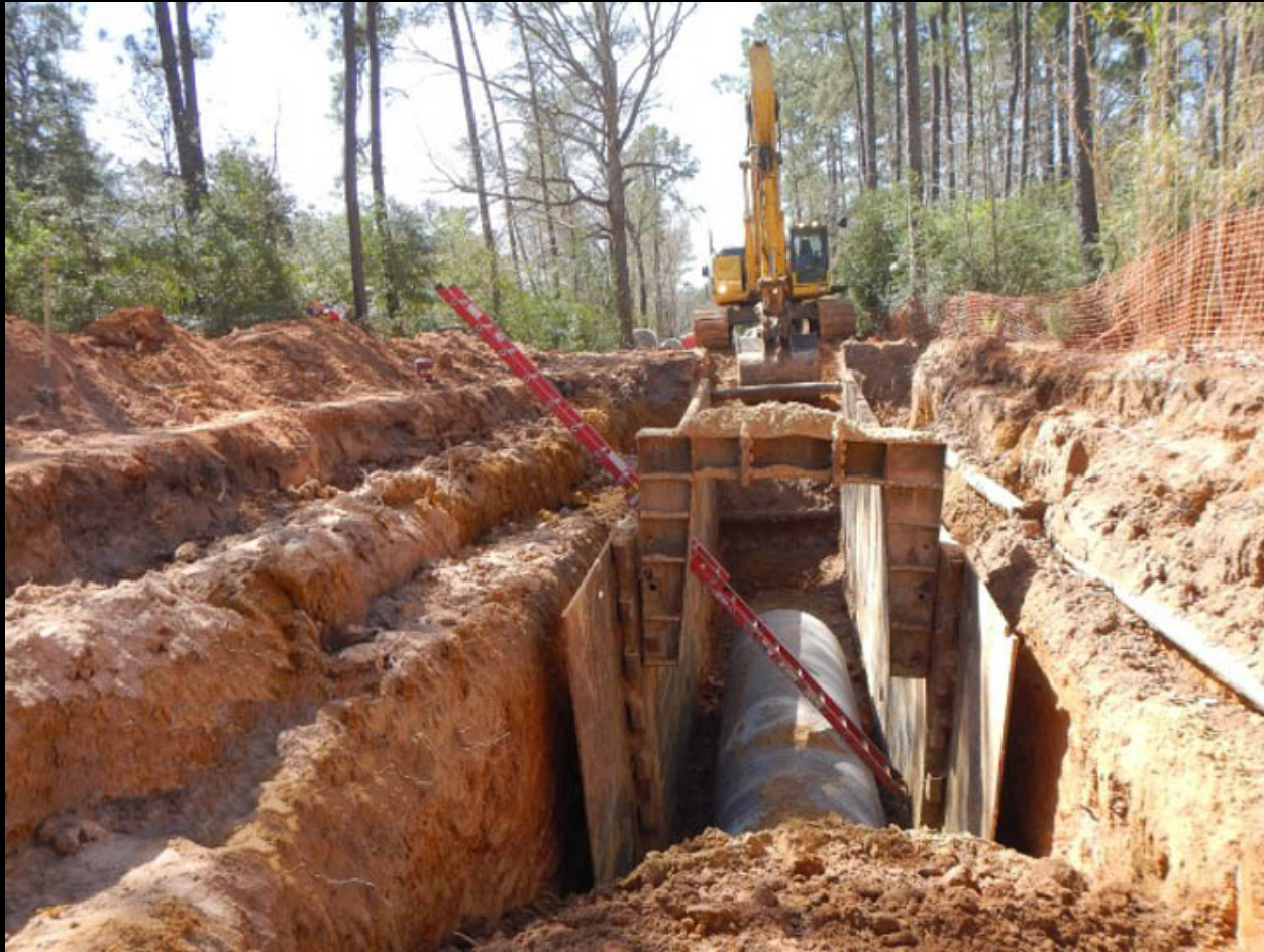
54-inch pipe installation along Sendera Ranch Road
