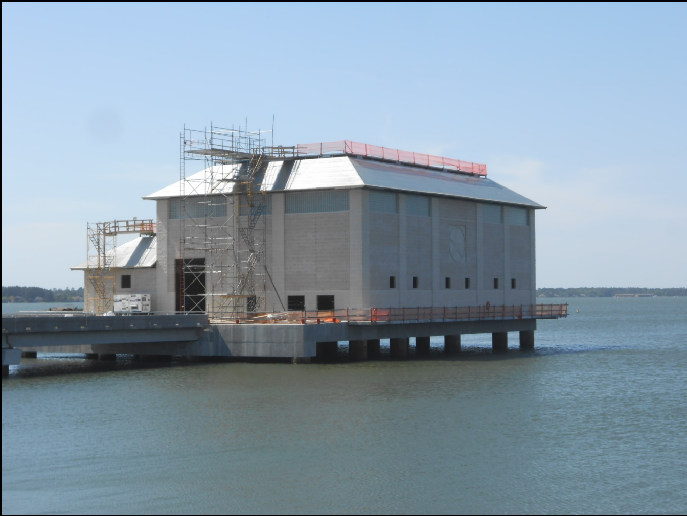
Raw Water Intake & Pump Station - Roof deck installation
