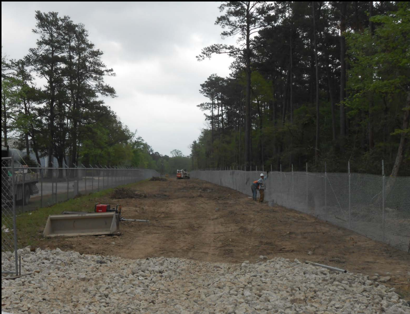
Security fence installation along Silver Springs Road at Girl Scout property
