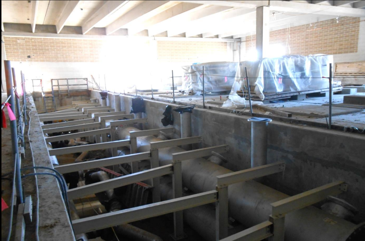
Membrane Building – Previous progress photograph
