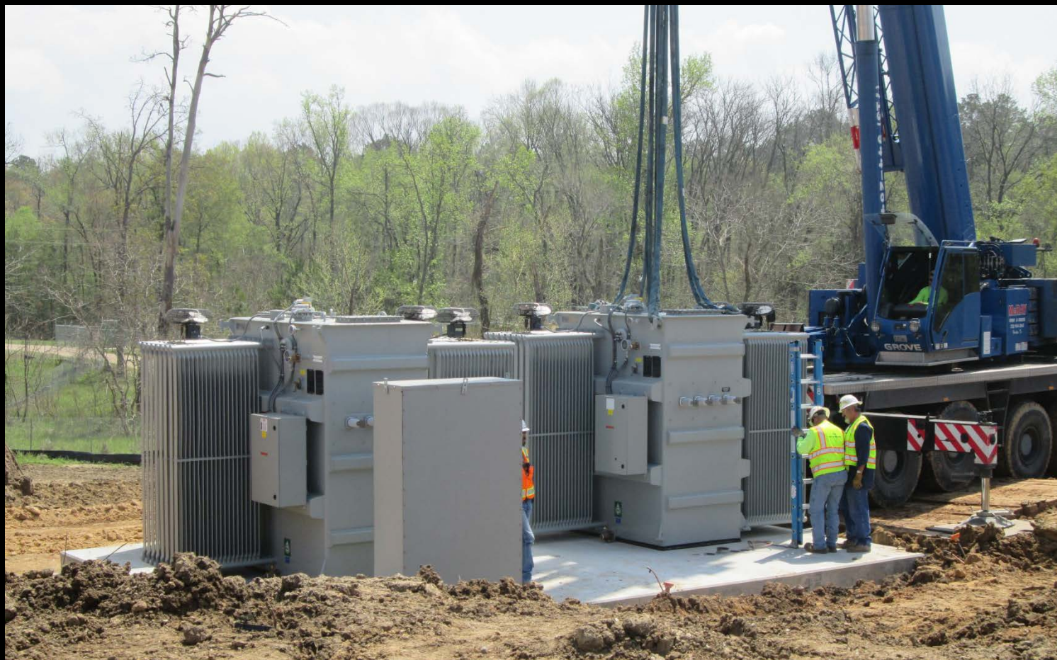
Electrical Facilities - Main transformer installation in progress
