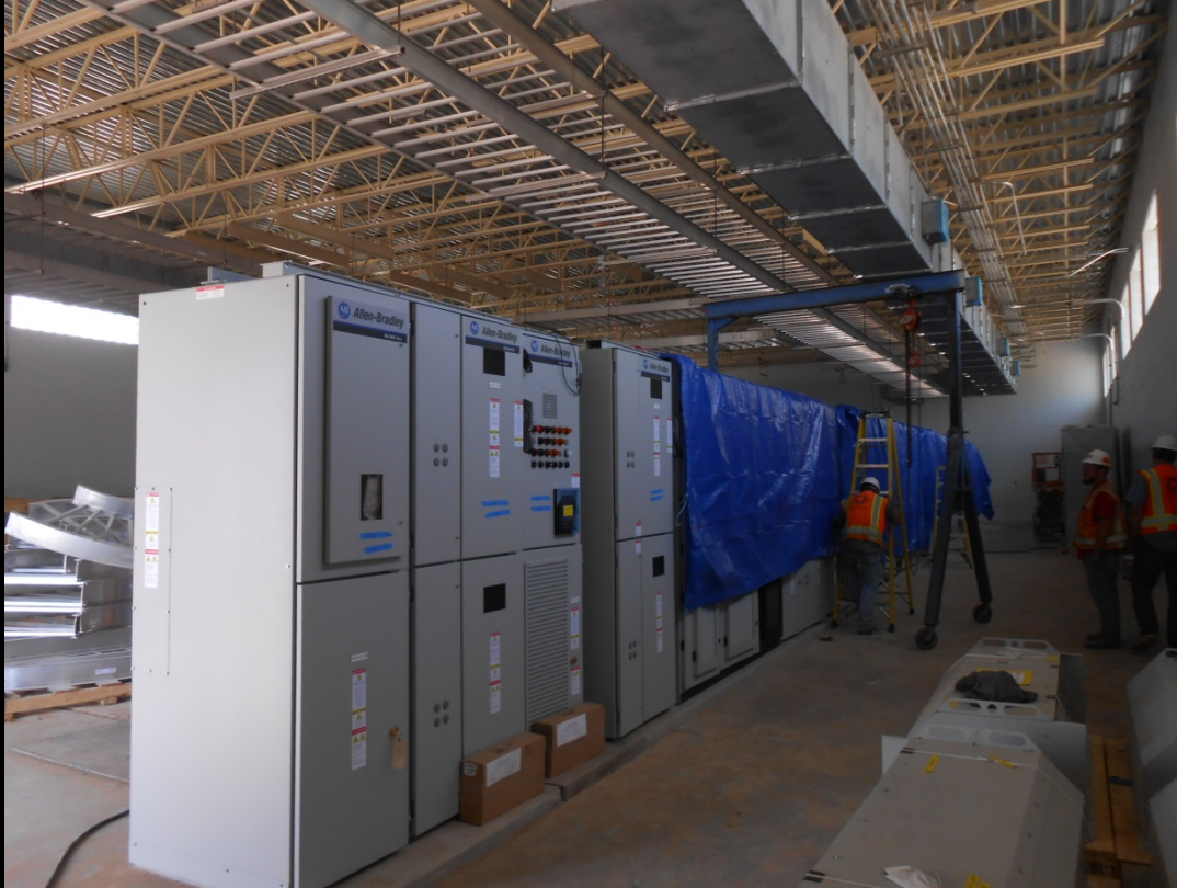
High Service Pump Station – Installation of electrical equipment
