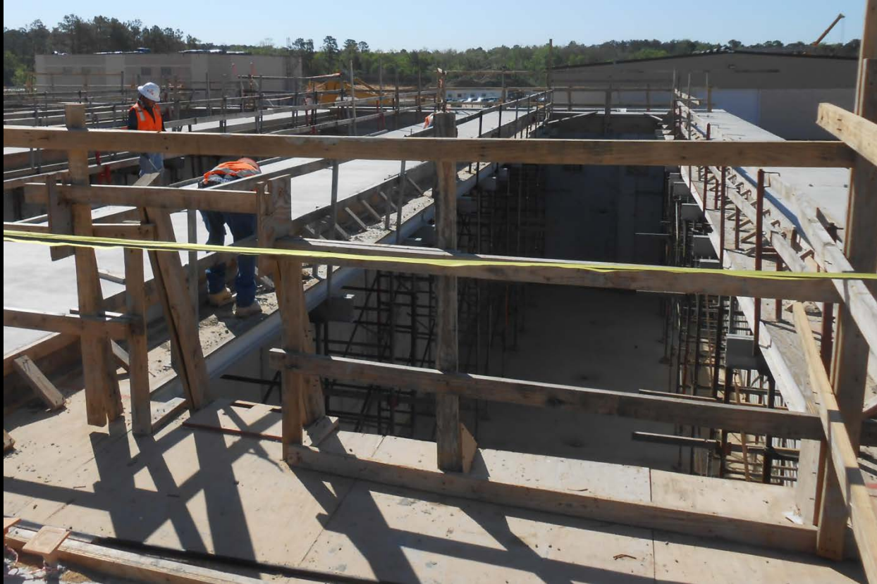
Pretreatment Facility - Access walkway installation
