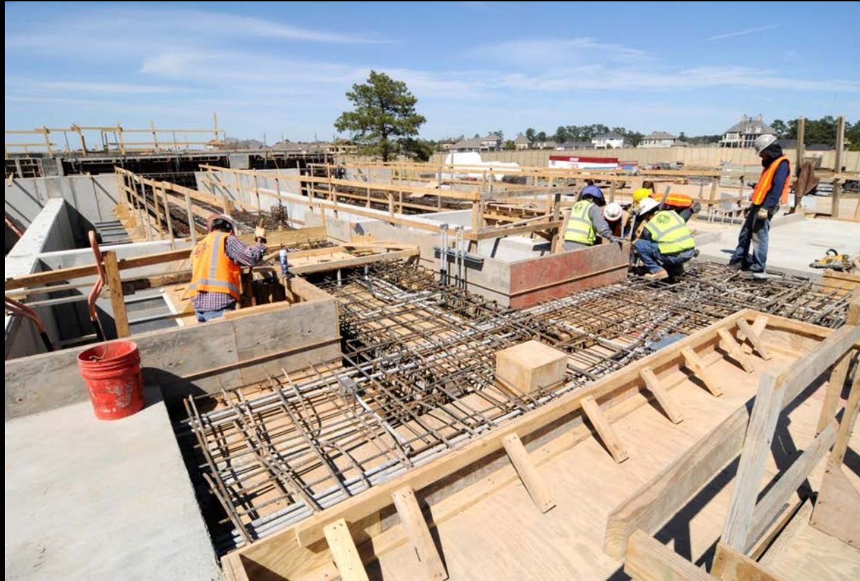
Pretreatment Facility – Previous progress photograph
