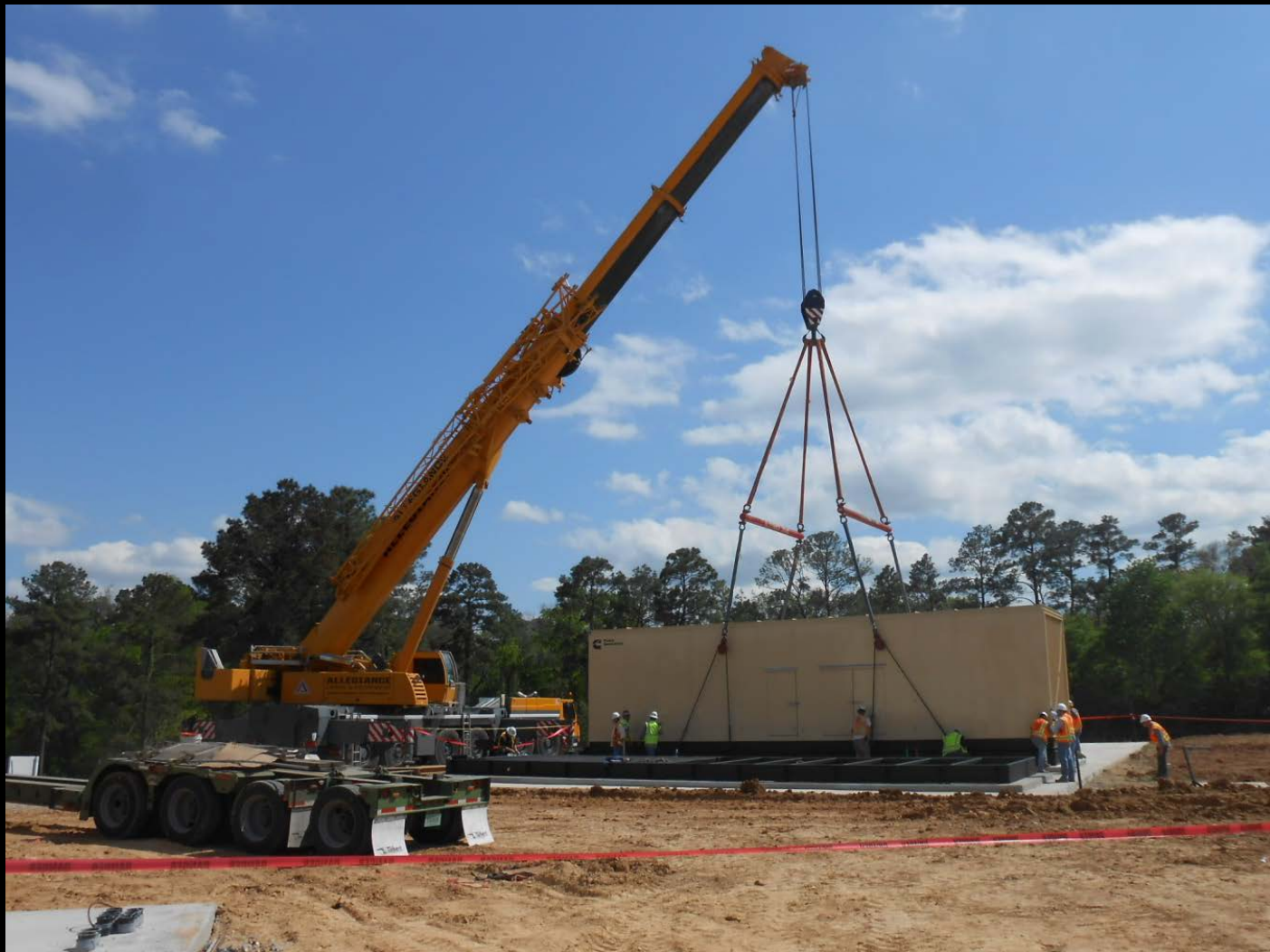
Electrical Facilities - Backup Generator installation
