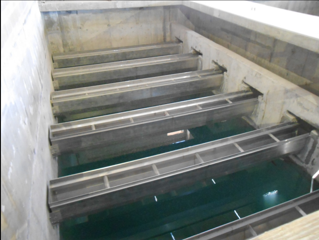
Granulated Activated Carbon Contactors – Leak testing contact basins
