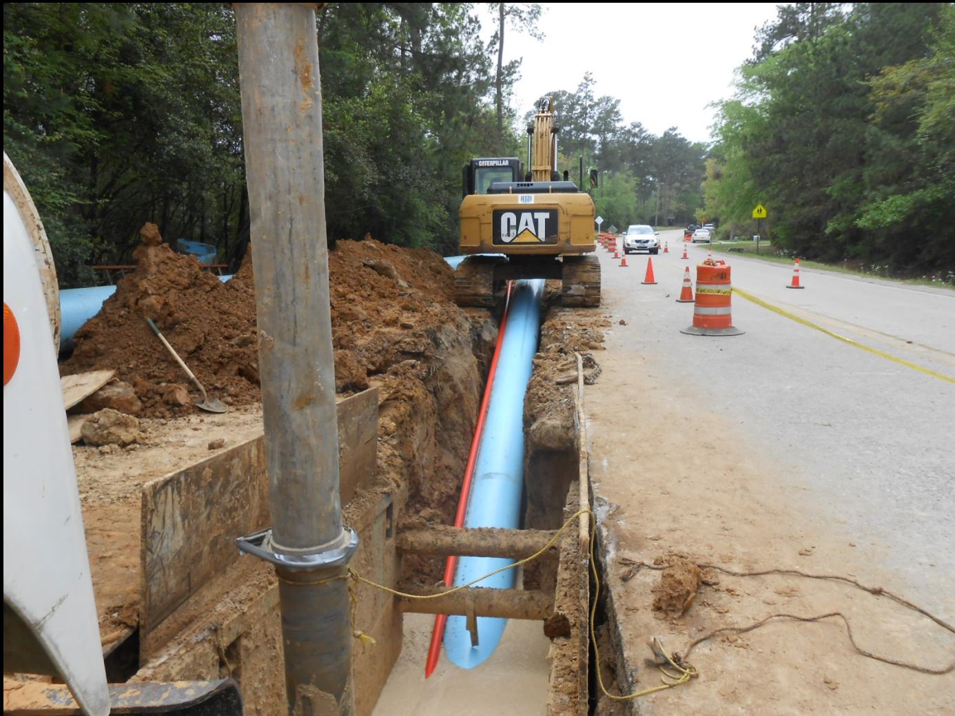
24-inch pipe and fiber optic conduit installation at Shadowbend Place
