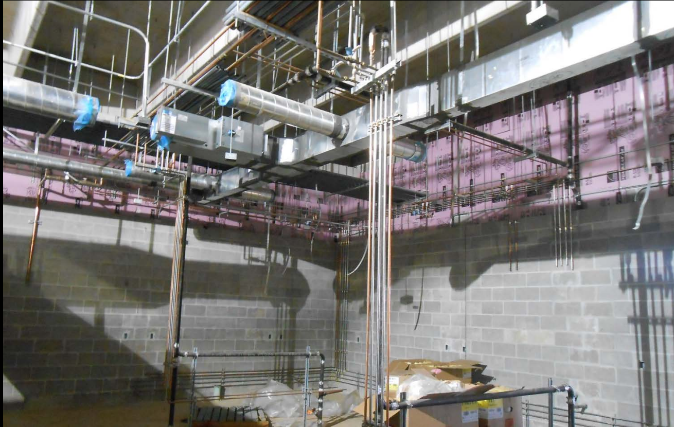
Membrane Building – Mechanical and Plumbing rough-in
