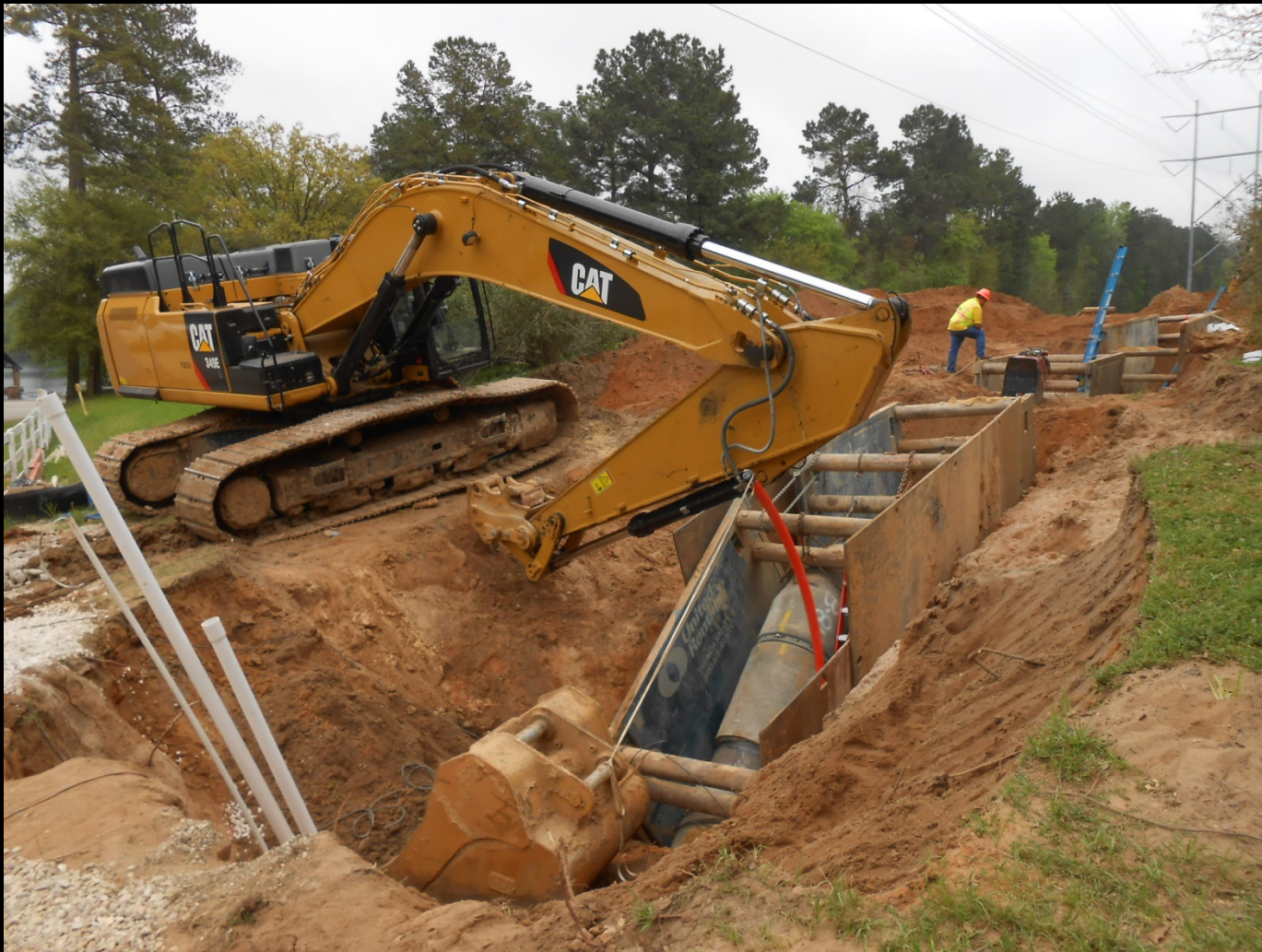
Pipe installation along Entergy easement and Wayne Bennett Court
