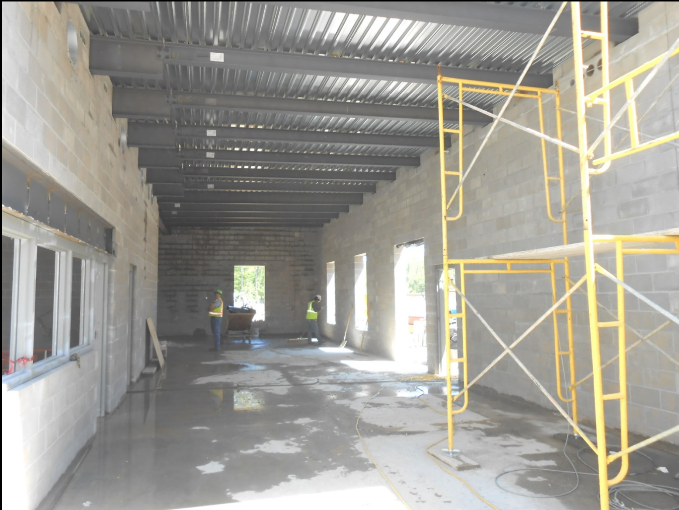
Operations Building - Masonry and structural steel installations
