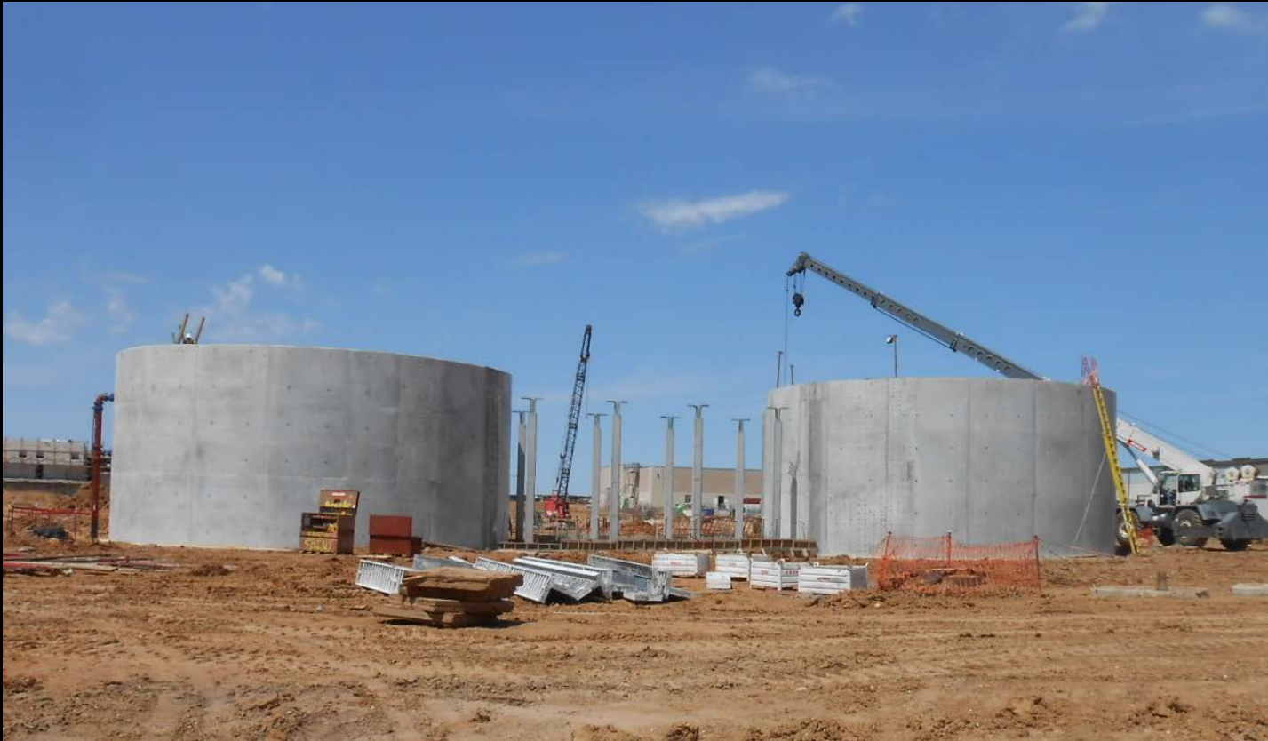
Sludge Thickeners – Concrete column installation
