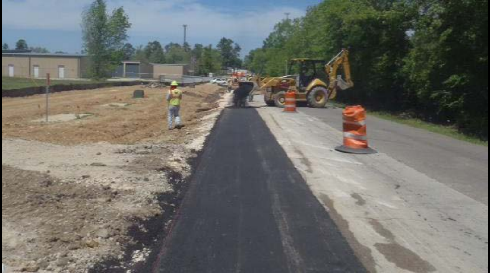
Asphalt pavement repairs along McCaleb Road
