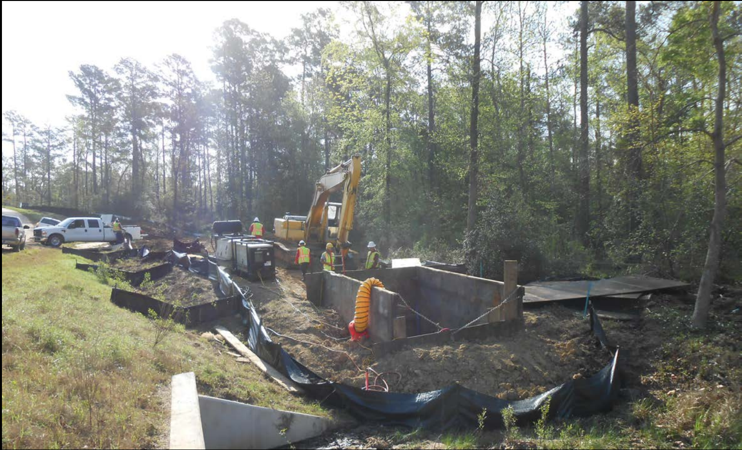
Tunnel installation at creek along GRP Access Road
