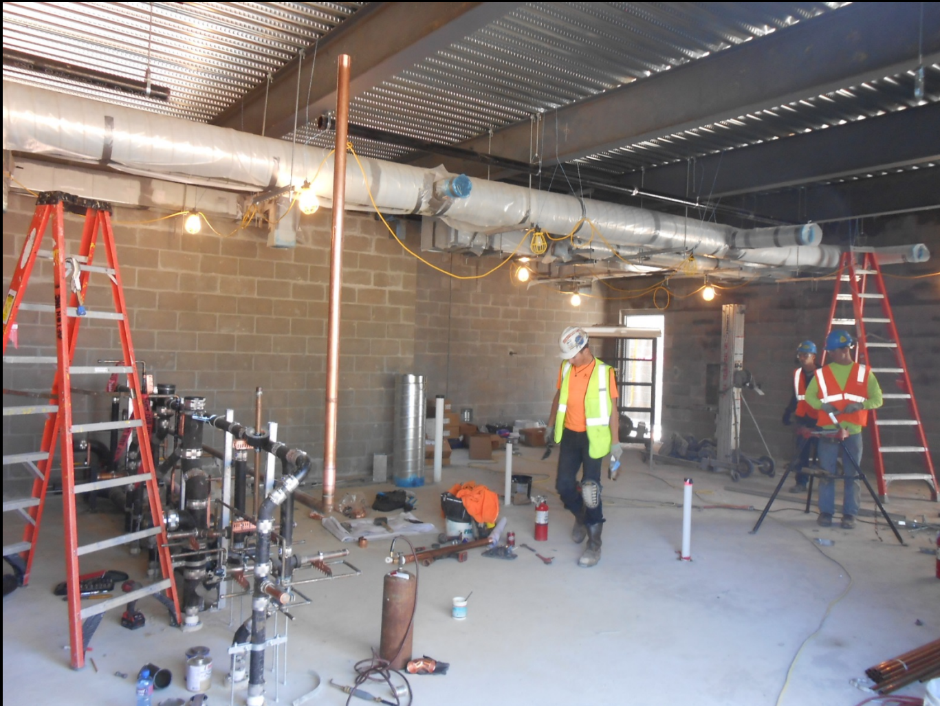
Operations Building - Mechanical and Plumbing rough-in
