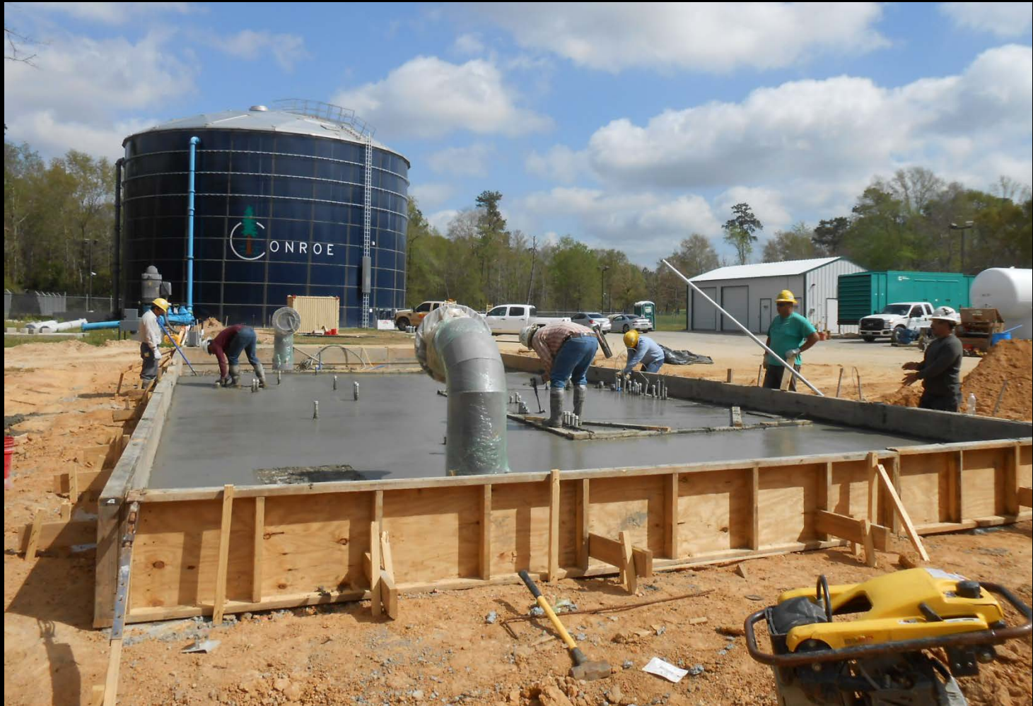
Flow and pressure control station slab installation at Conroe Water Plant No. 22
