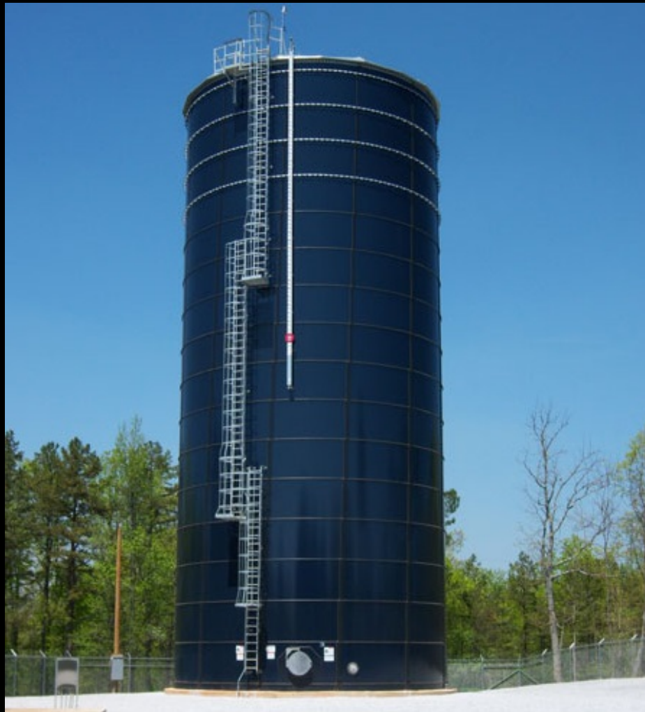
Example Standpipe - SJRA Standpipe currently under fabrication
