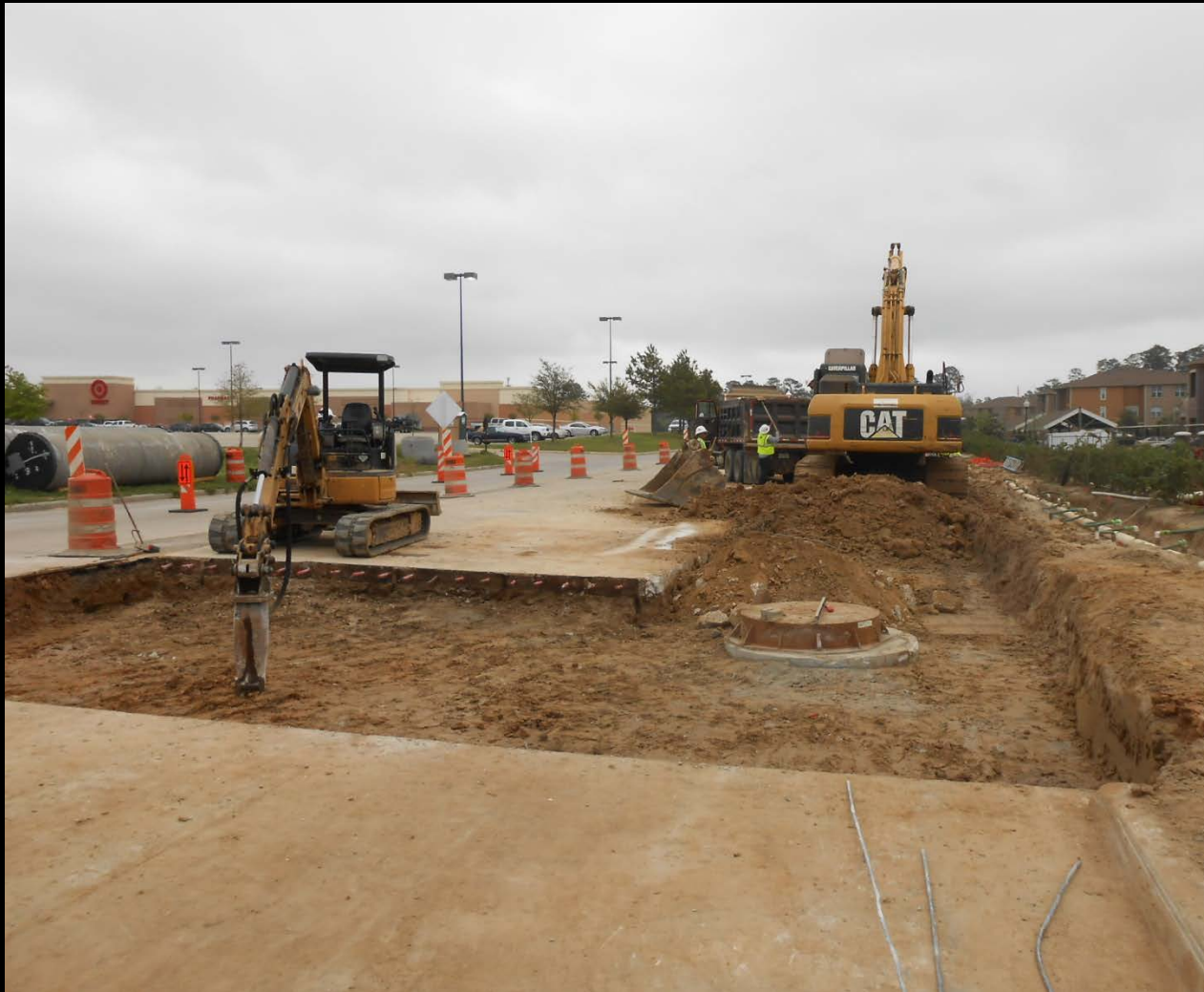
Concrete repairs along Research Forest Drive
