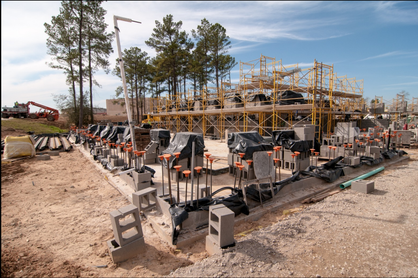
Operations Building – Previous progress photograph
