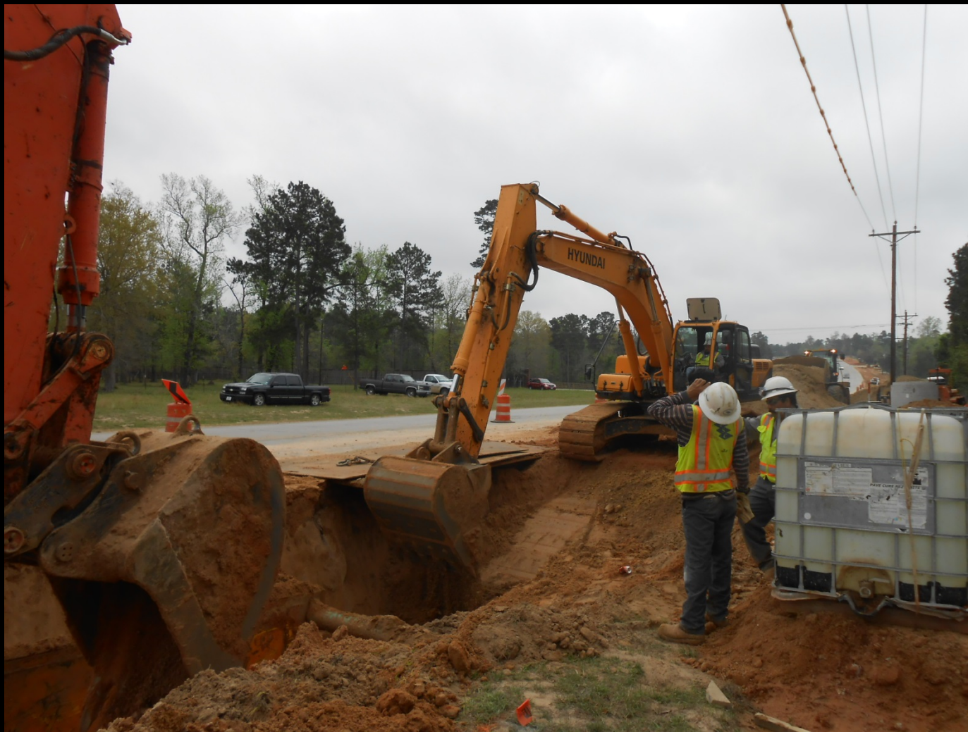
54-inch pipe installation along Fish Creek Thoroughfare
