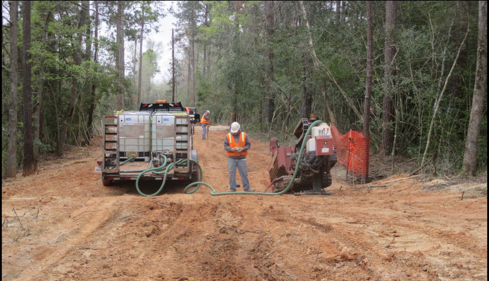
Horizontal directional drilling fiber optic conduit along Longmire Road
