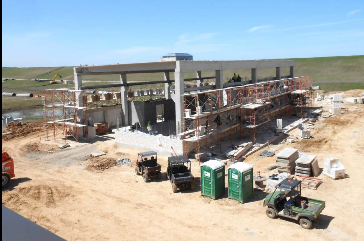
Blower Building – Previous progress photograph
