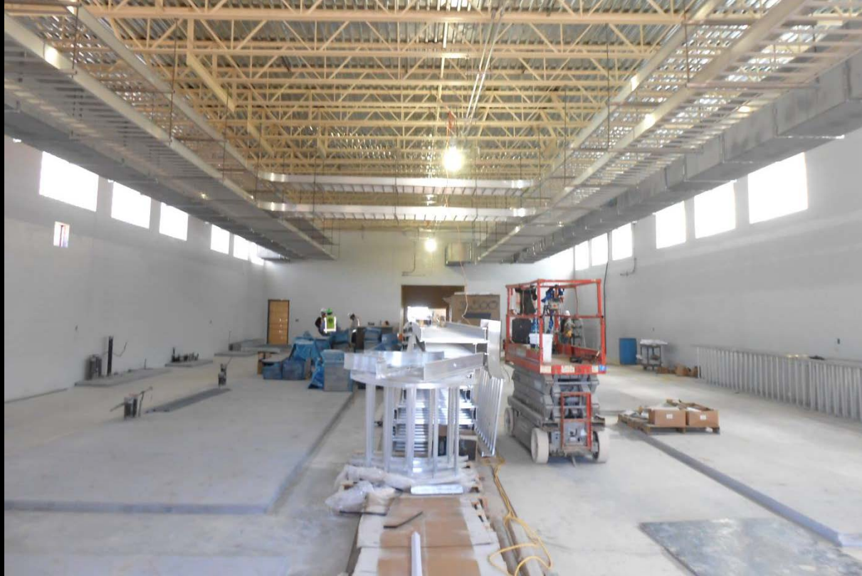
High Service Pump Station - Previous progress photograph
