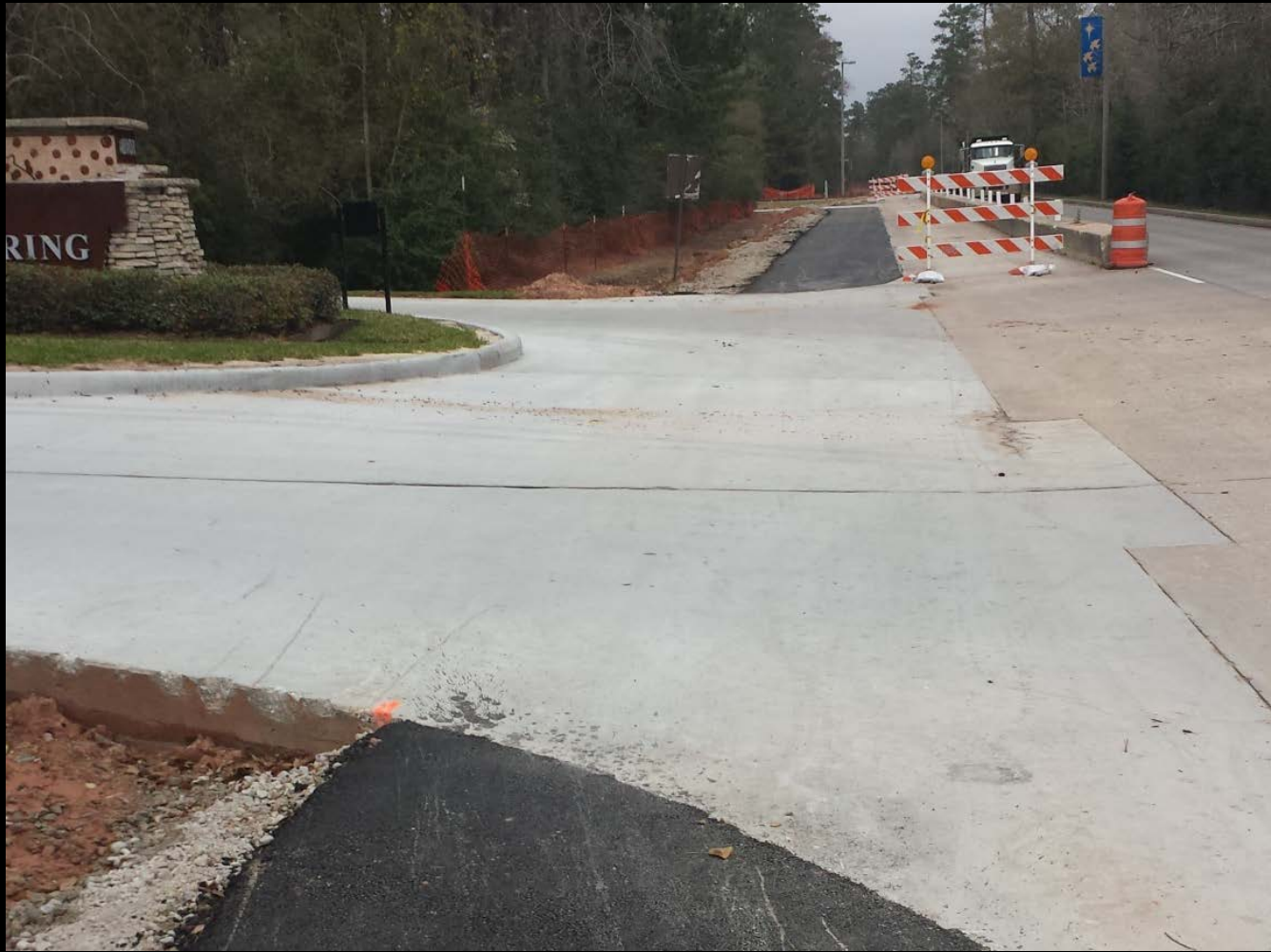
Asphalt shoulder repair along Research Forest Drive
