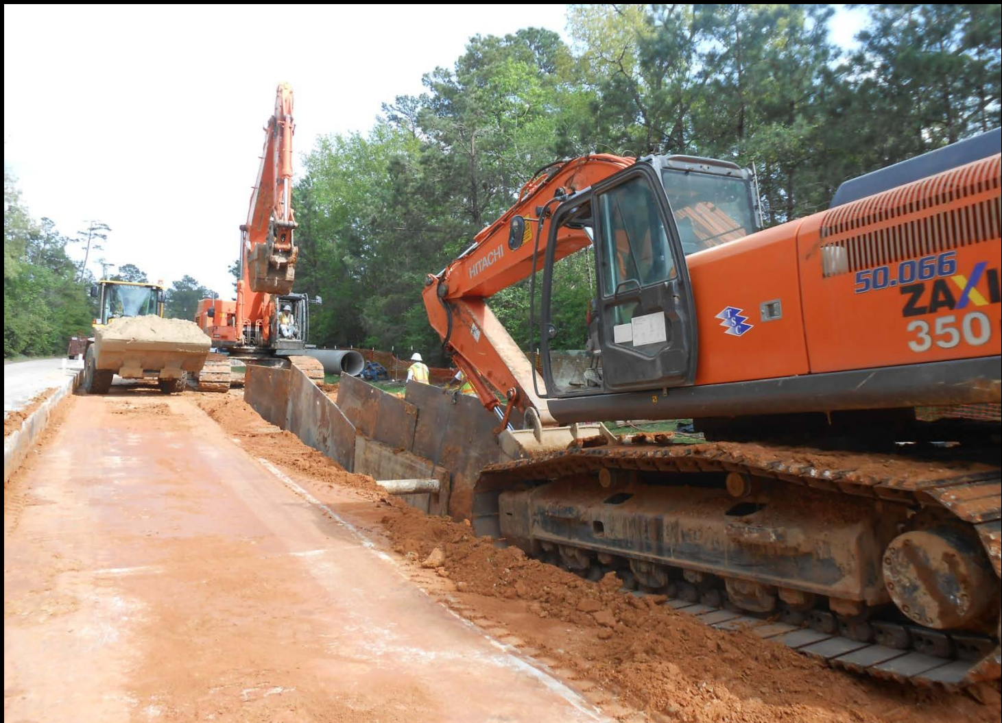
42-inch pipe installation along Research Forest Drive
