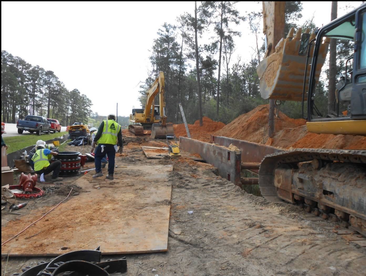
24-inch pipe and restrained joint installation along FM 830
