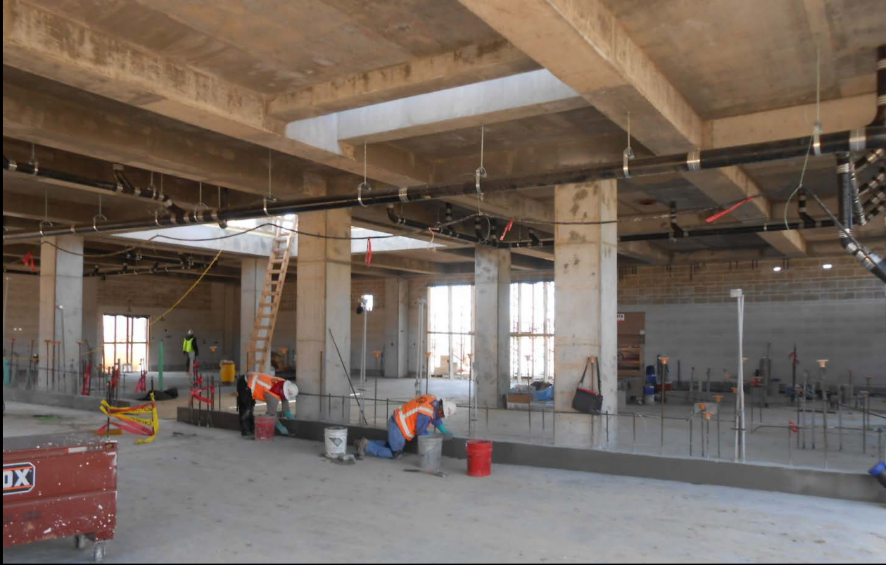
Dewatering Building – First floor mechanical installation
