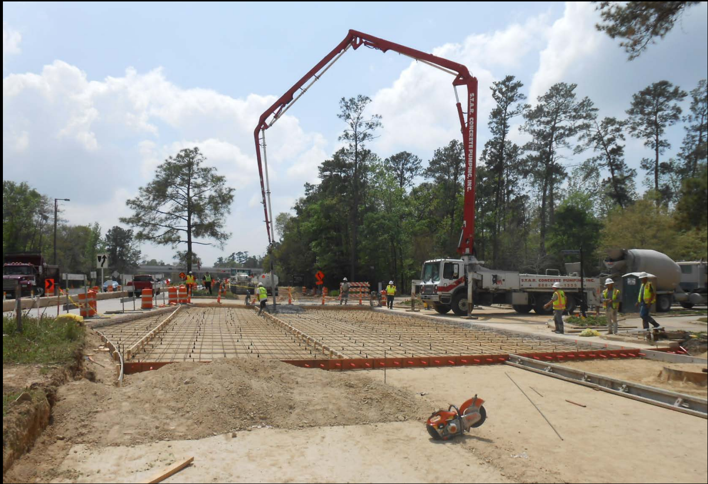
Concrete pavement installation at Grogan's Mill Road and East Shore Drive
