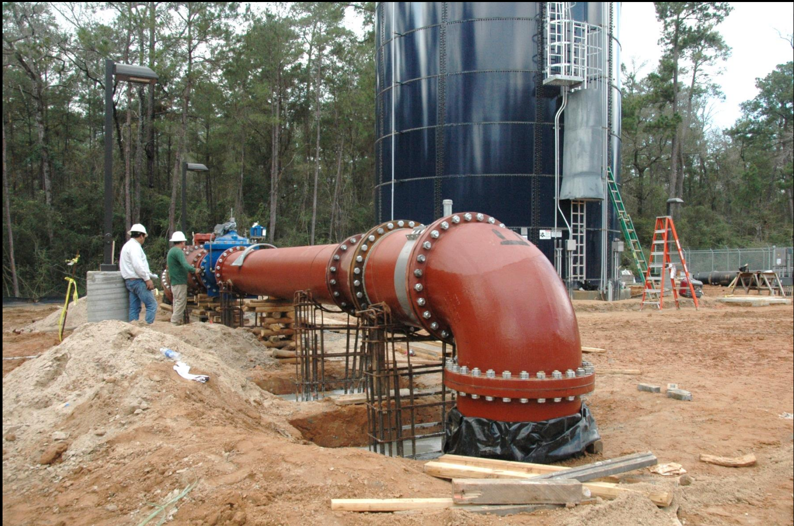
Above ground piping and pipe support installation
