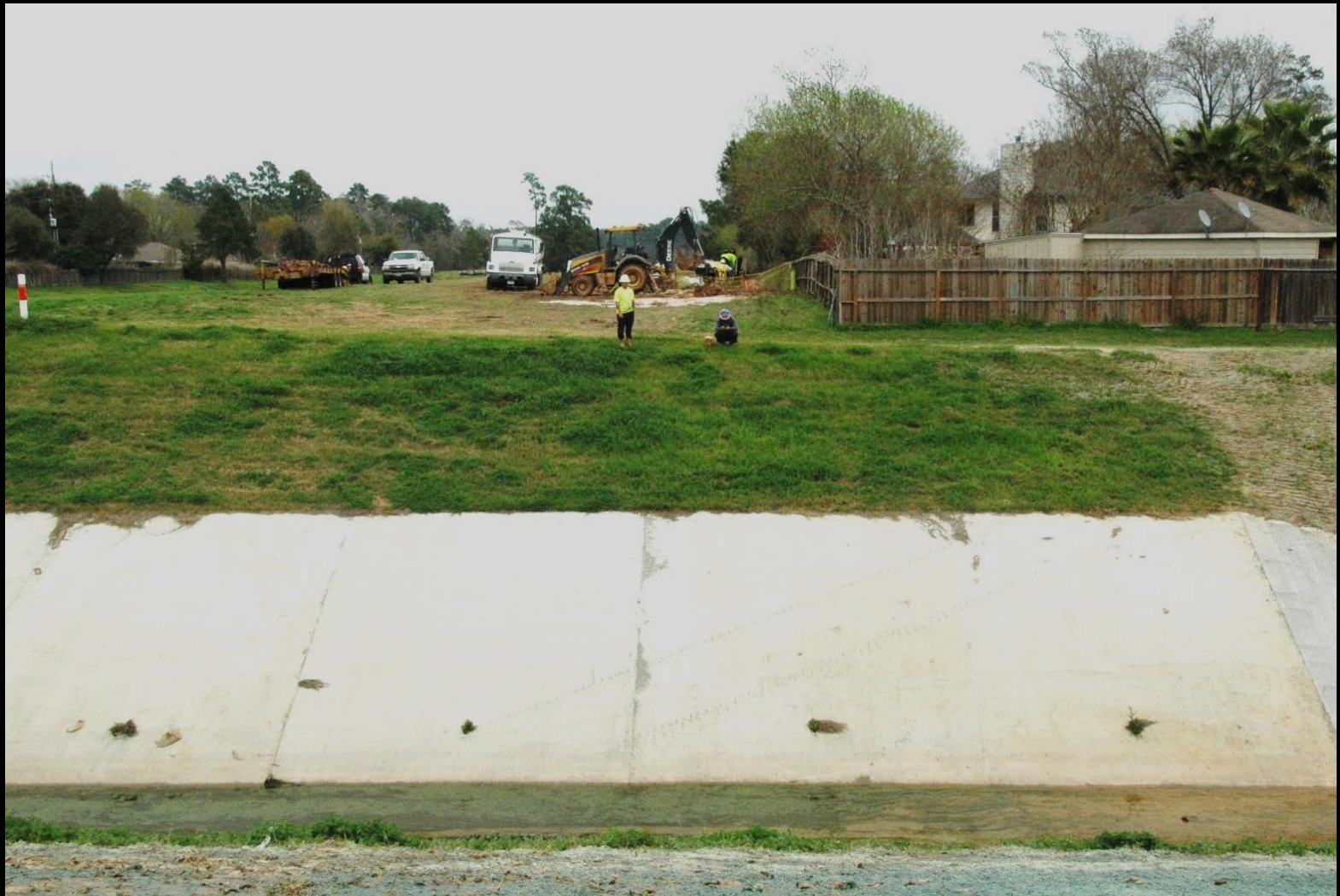
Tunnel operations for 20" HDPE pipe under drainage ditch
