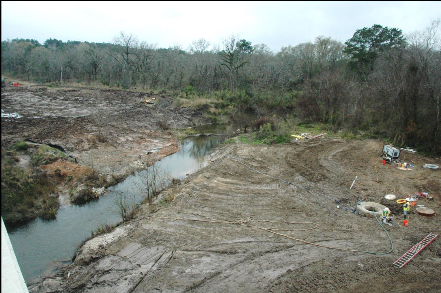
Site restoration at Lake Creek crossing
