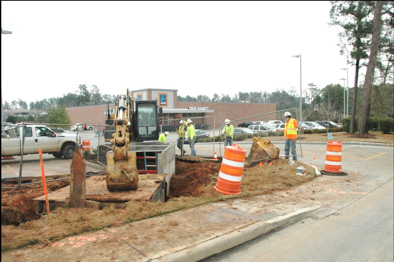
Tunneling operations at Longmire Road and Loop 336 North
