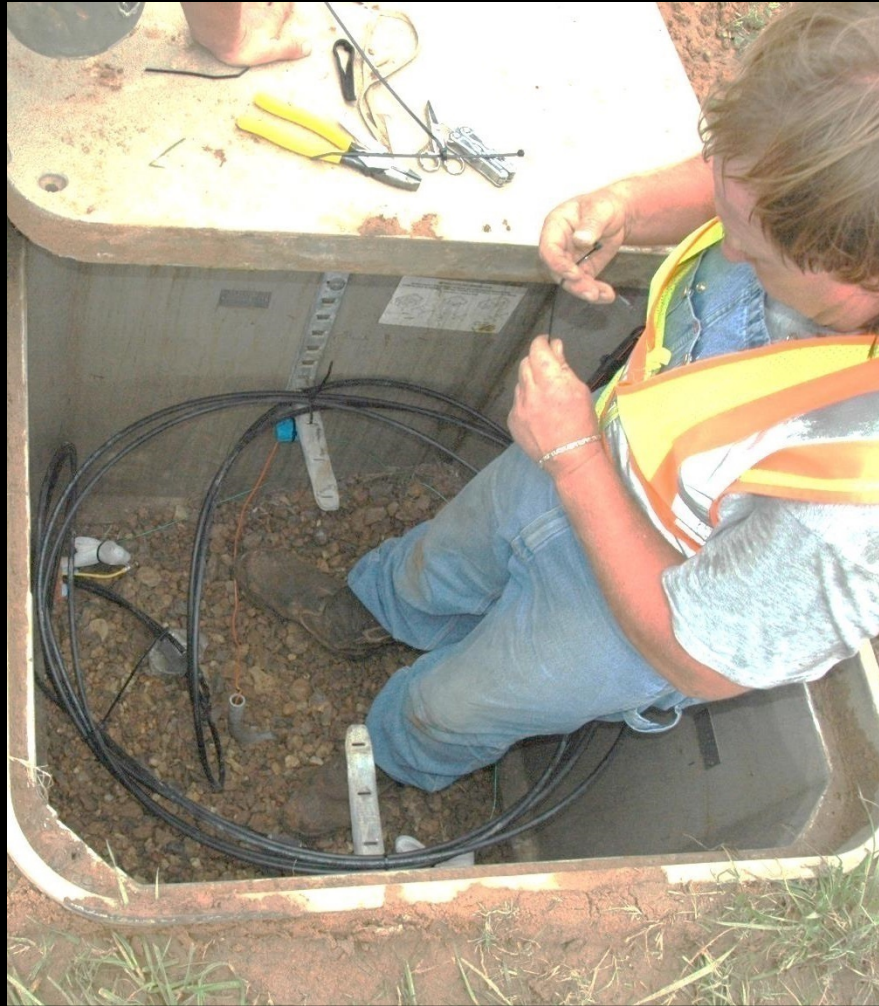
Fiber Optic termination and cable tagging at ground box
