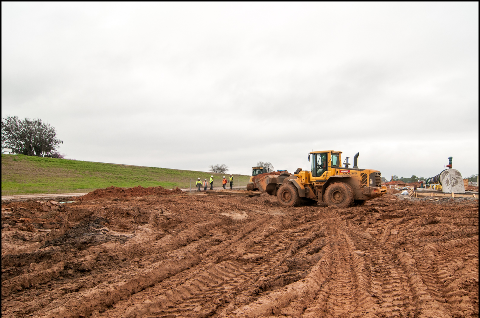
General Site – Recent heavy rainfall impact to construction site
