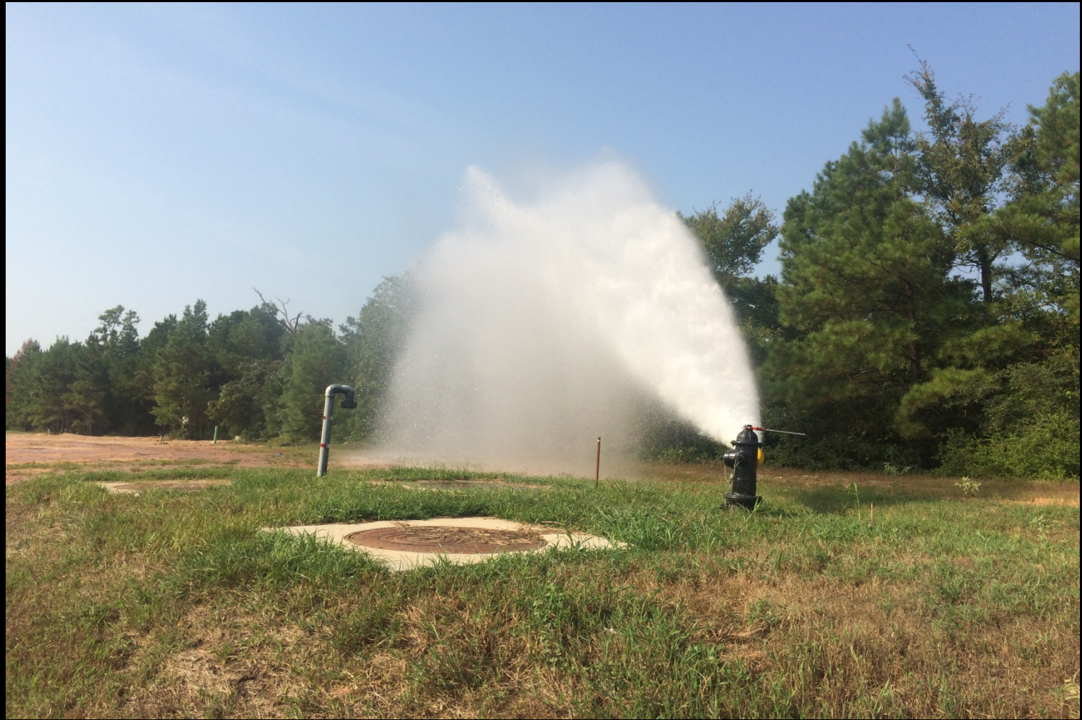
Transmission line flushing at the in-line flushing hydrant
