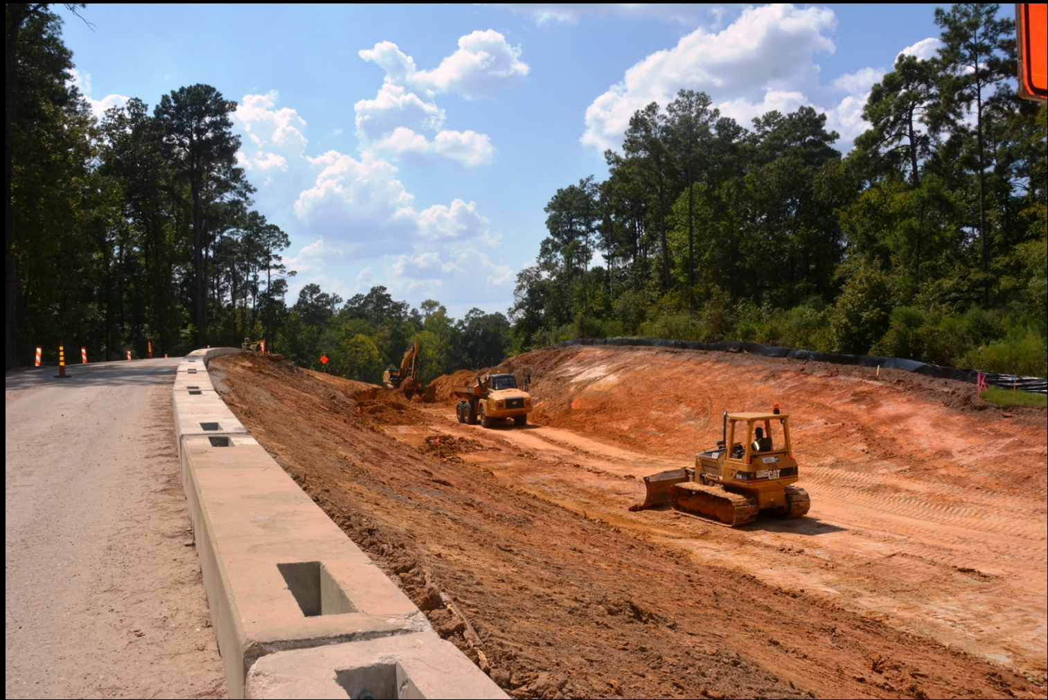
Access Road – Excavation and grading to final subgrade
