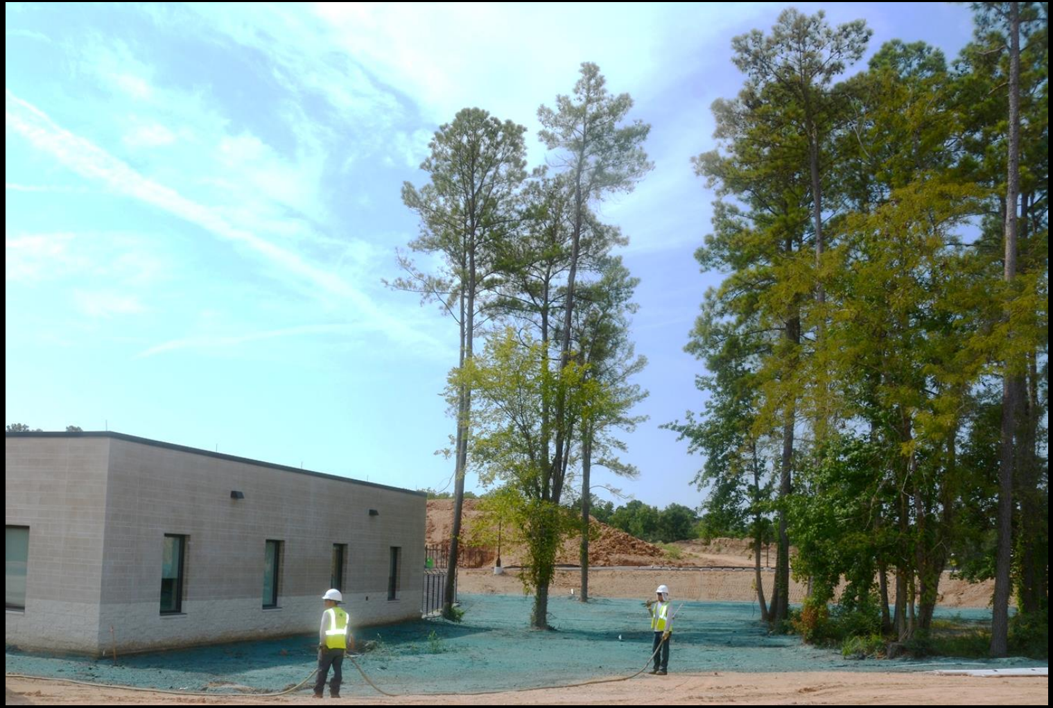
Operations Building- Hydromulching and clean up
