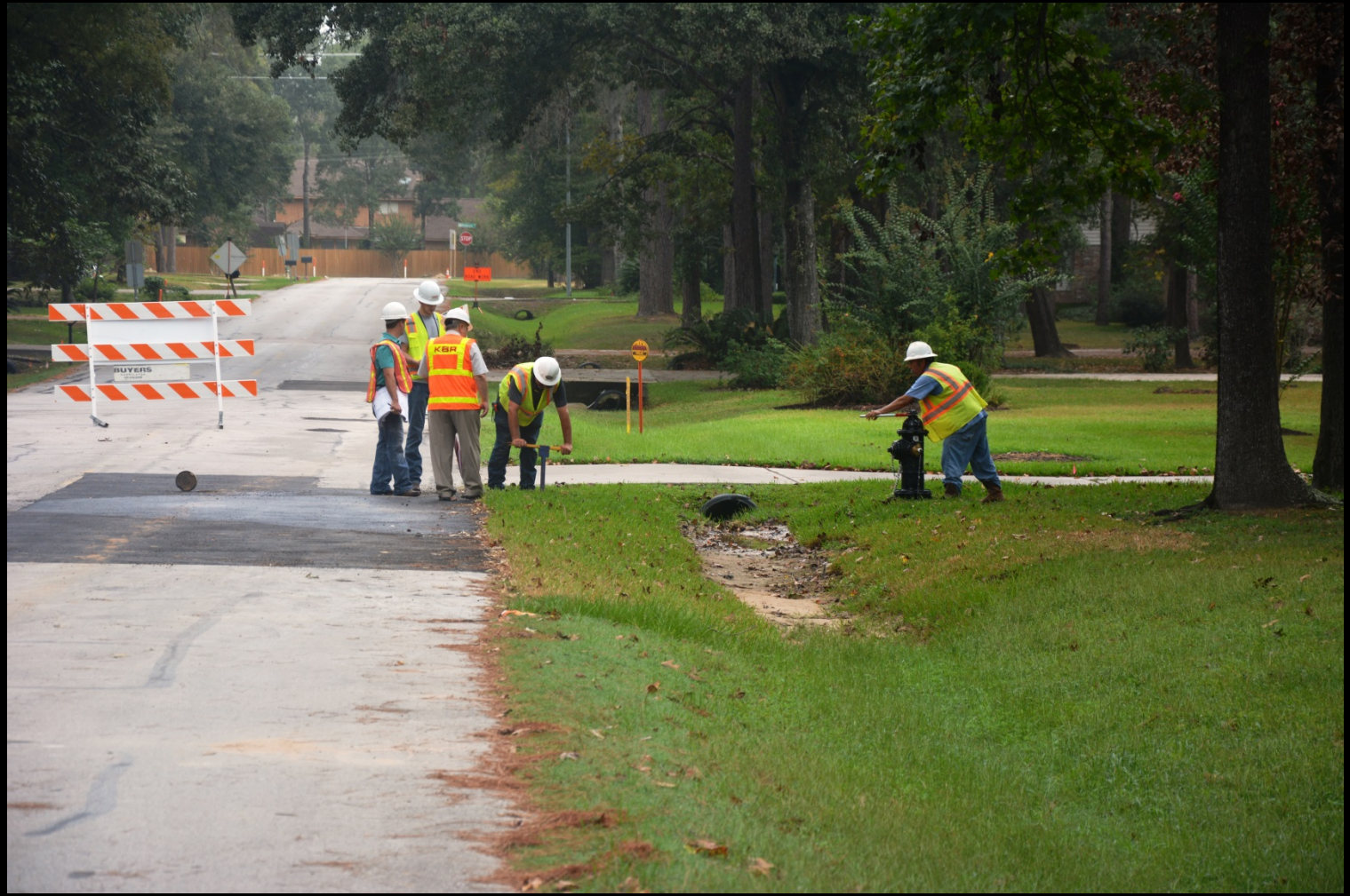
Transmission Line W3D – Completion of site restoration
