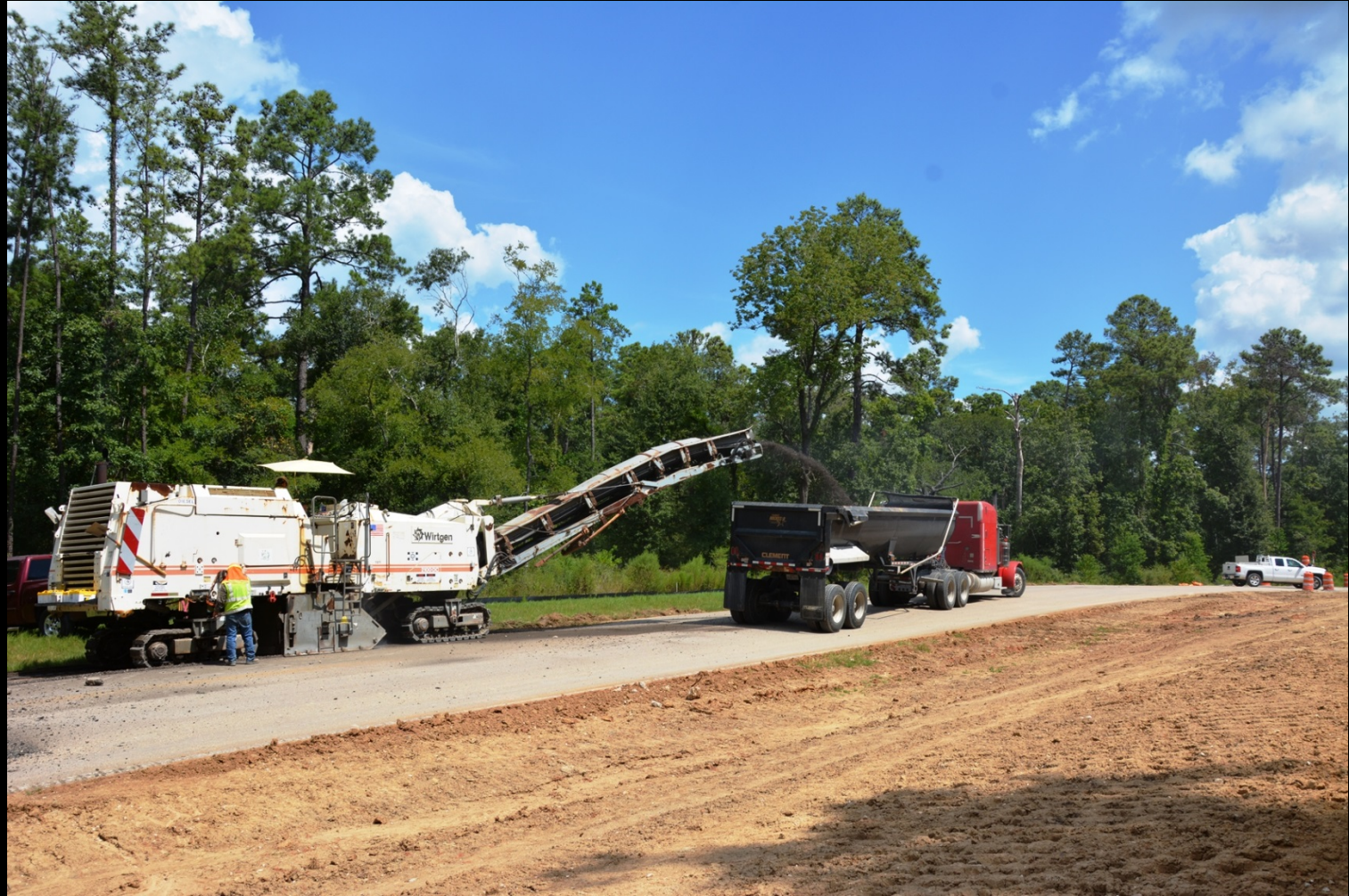
Access Road – Milling of asphalt for the permanent access road
