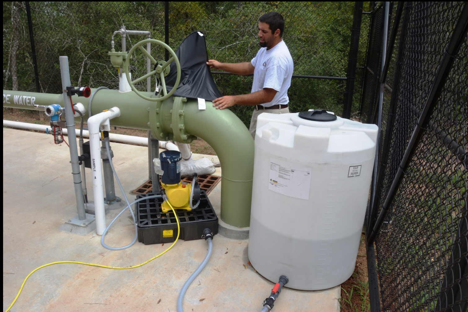
Transmission line dechlorination at the Water Receiving Facilities
