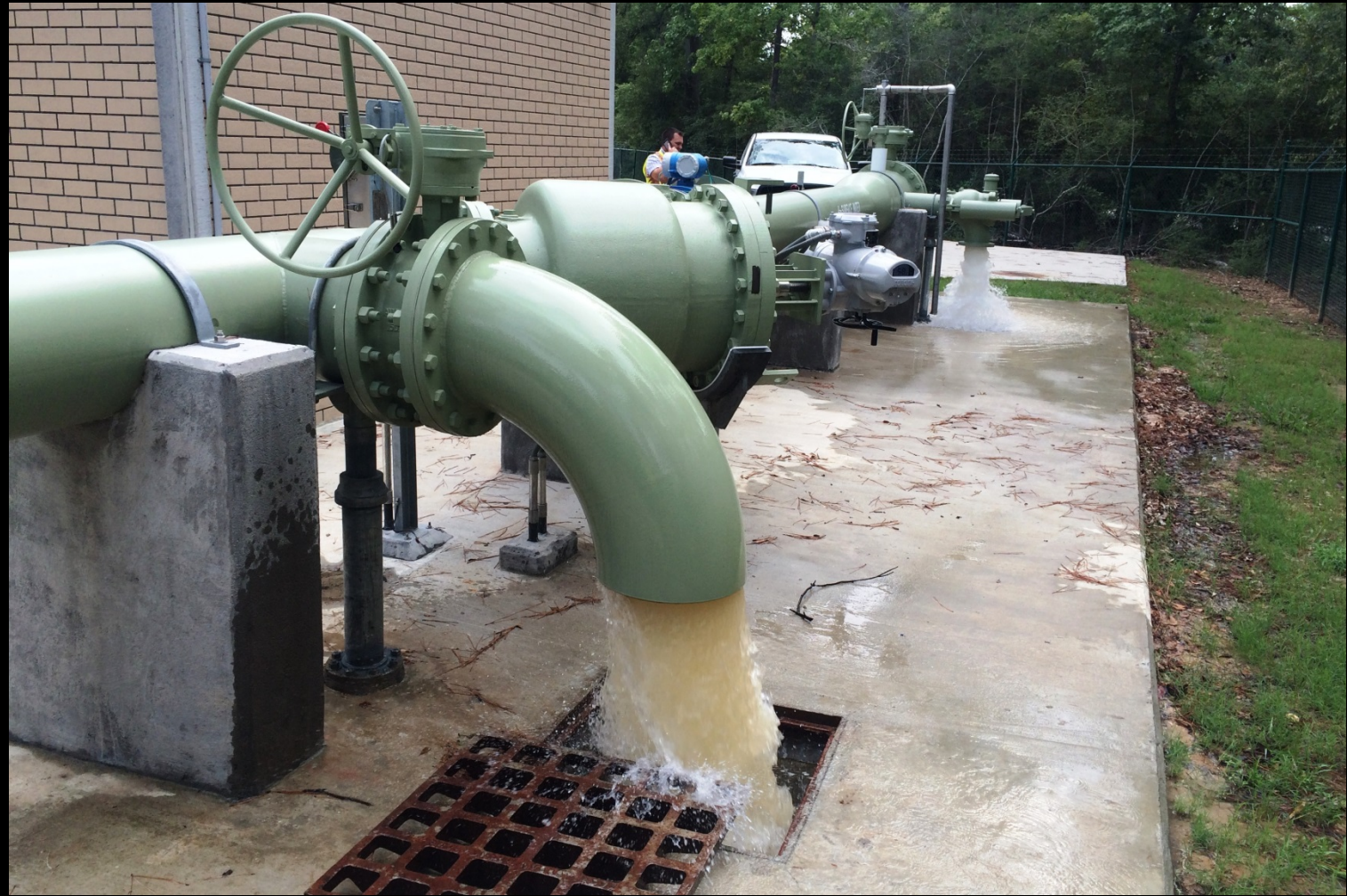
Transmission line flushing at the Water Receiving Facilities
