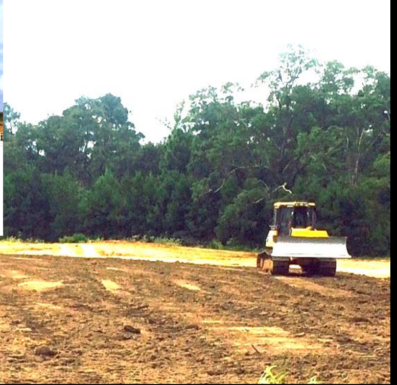
General Site-Grading and clean up
