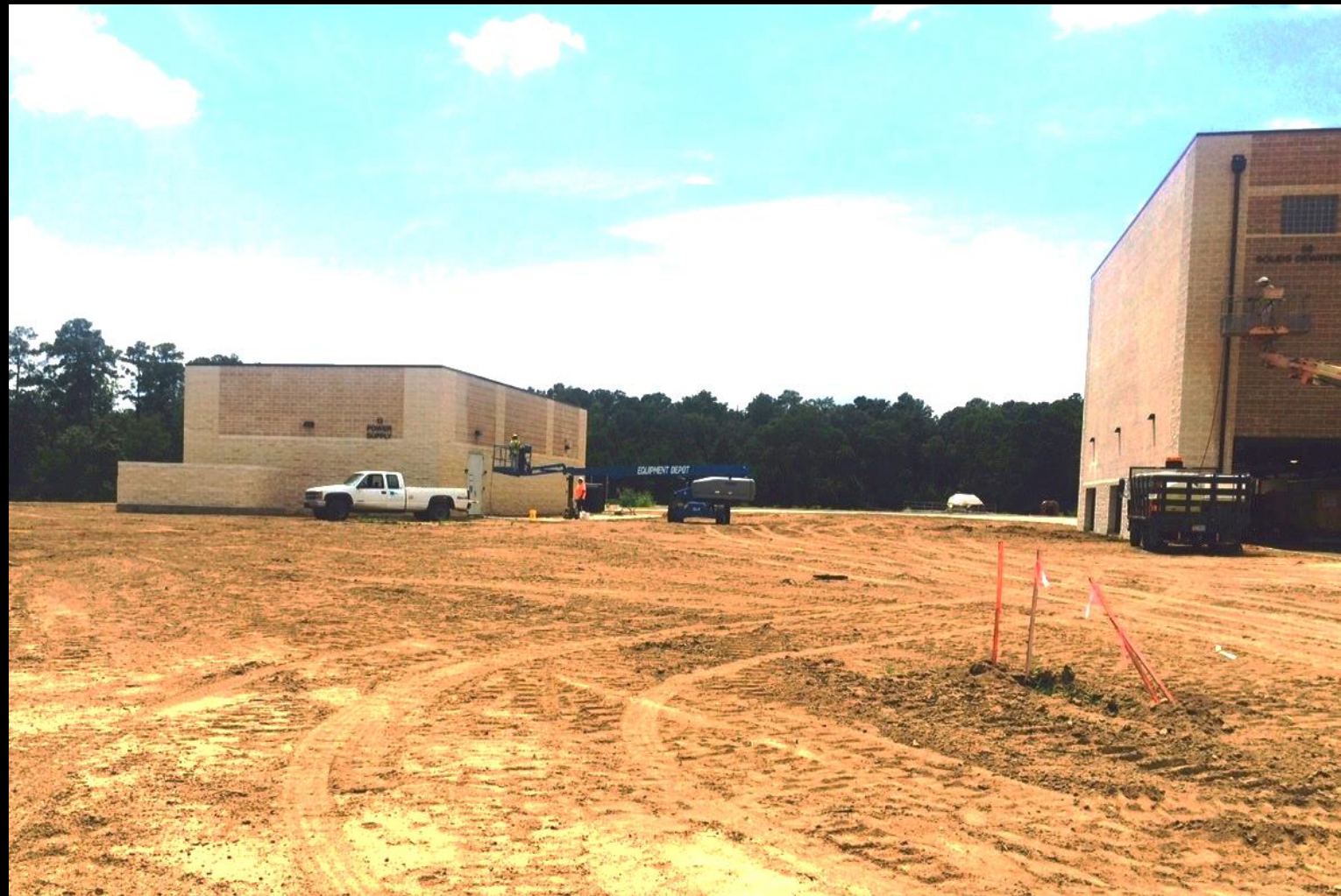
General Site- Site clean up, power washing and sealing of exterior masonry
