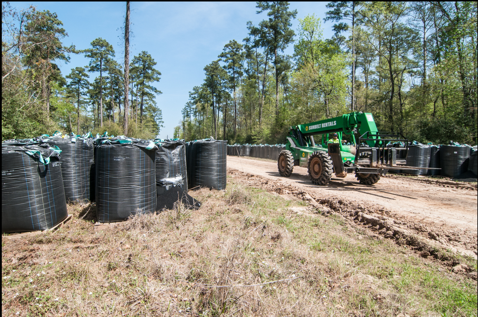
Granulated Activated Carbon – Delivery and storage of 880 tons of GAC
