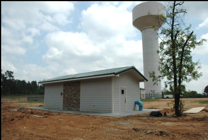
Mid-South Water Receiving Facility
