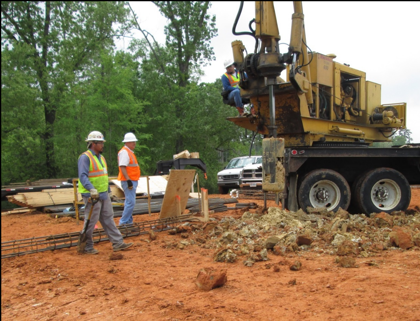
Maintenance Building – Installation of drilled shafts
