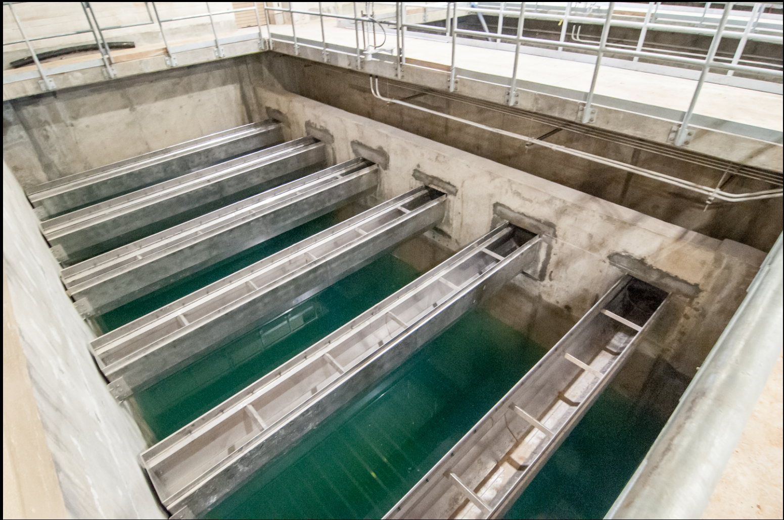
Granulated Activated Carbon Building – Underdrain testing during backwash cycle
