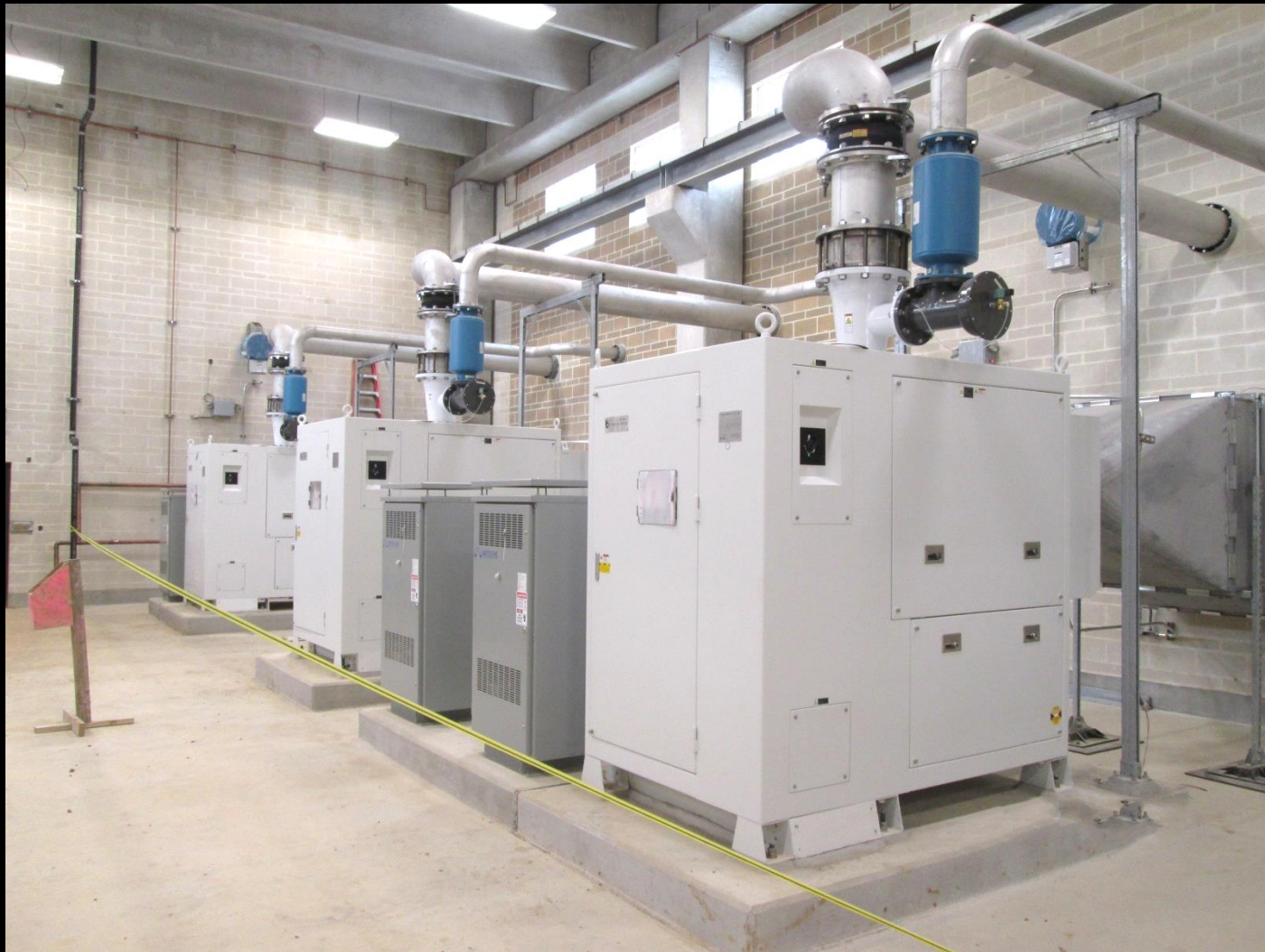
Blower Building – Neuros turbo blowers and piping
