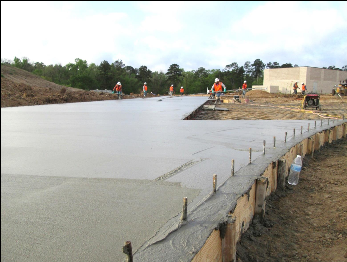
General Site – Roadway installation from main entrance to the Power Supply Building
