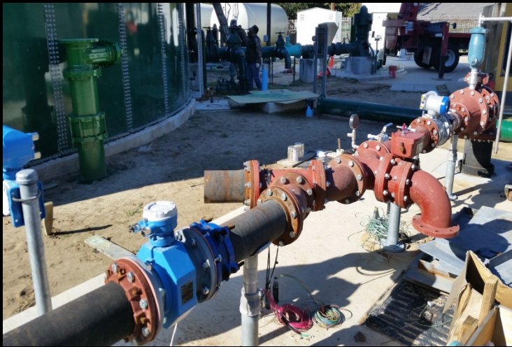
Rayford Road Water Receiving Facility
