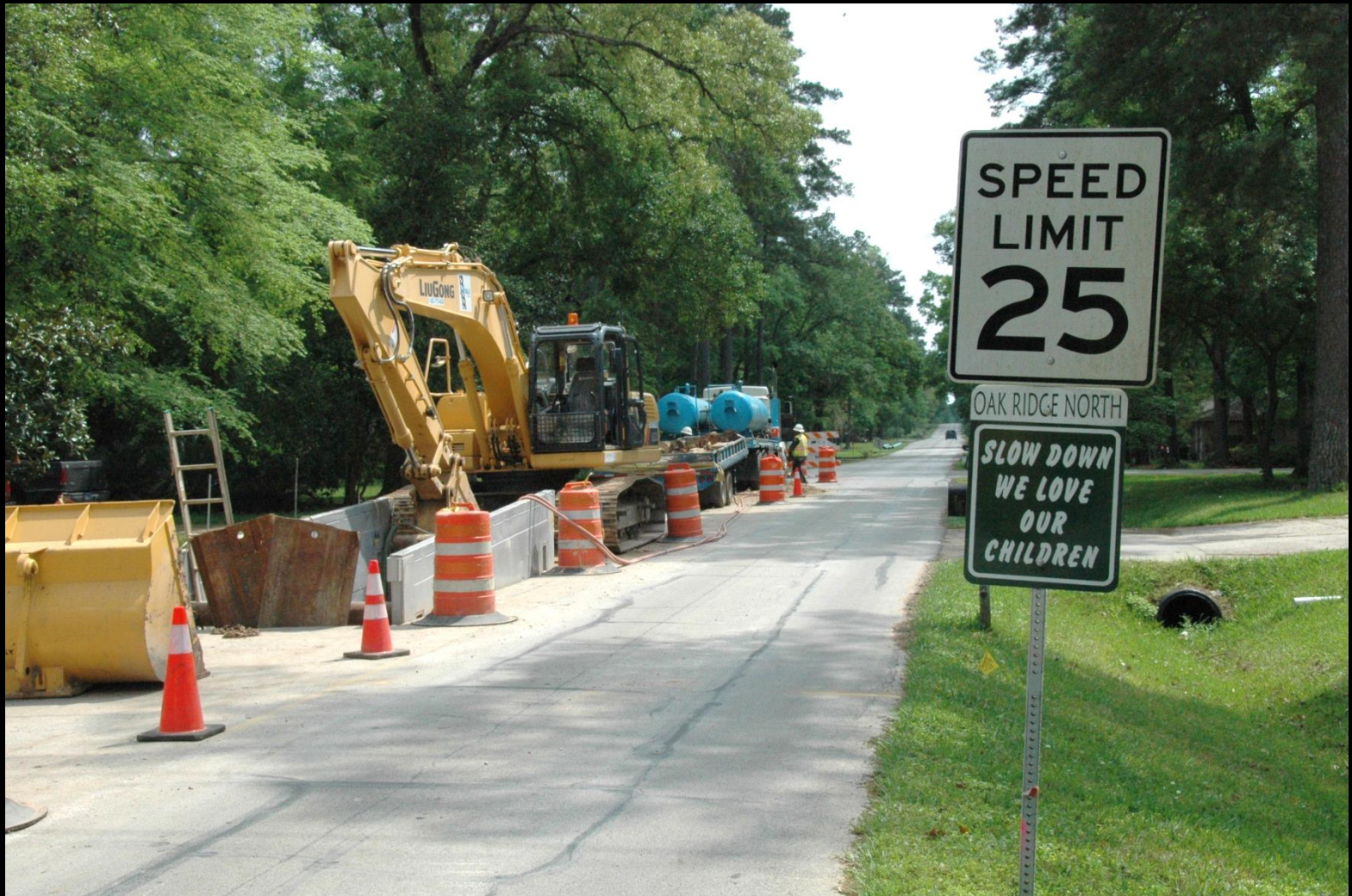
16-inch pipe trenchless bore pit installation along Maplewood Dr.
