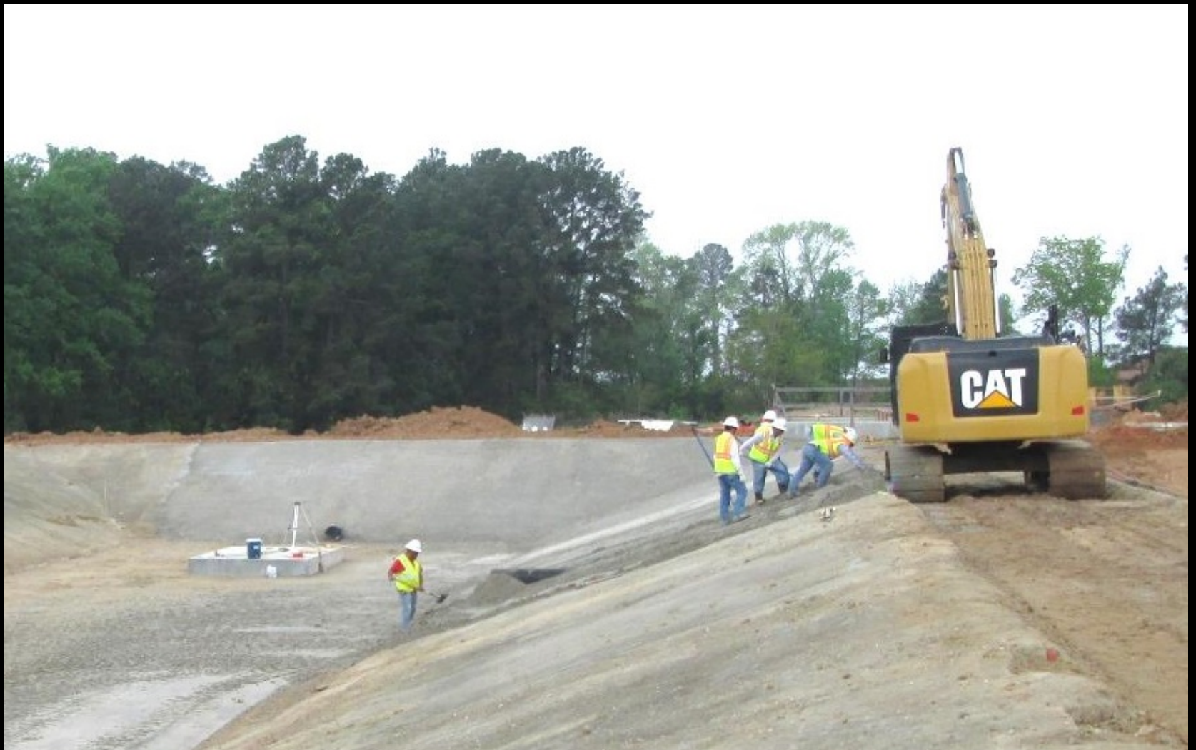
Process Water Recovery – Soil cement lining installation
