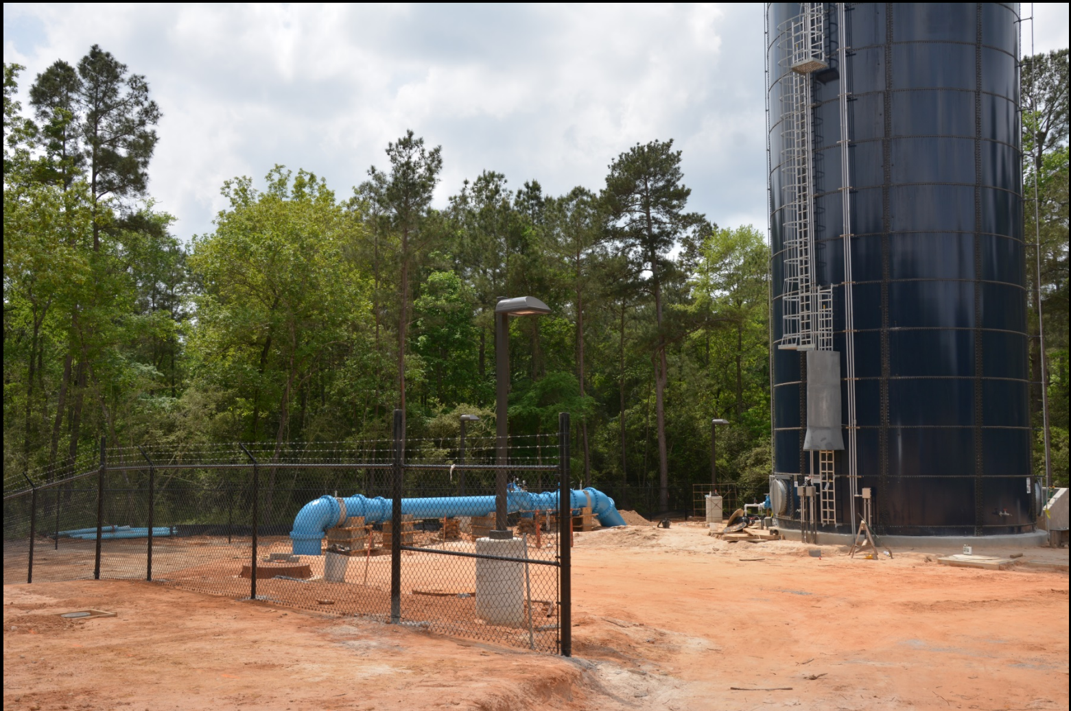
Final grading, aboveground pipe coating, and fencing complete.
