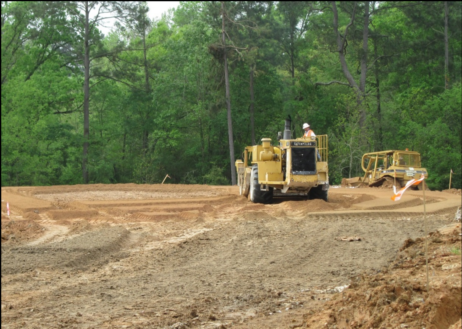
General Site – Stabilization of pavement subgrade
