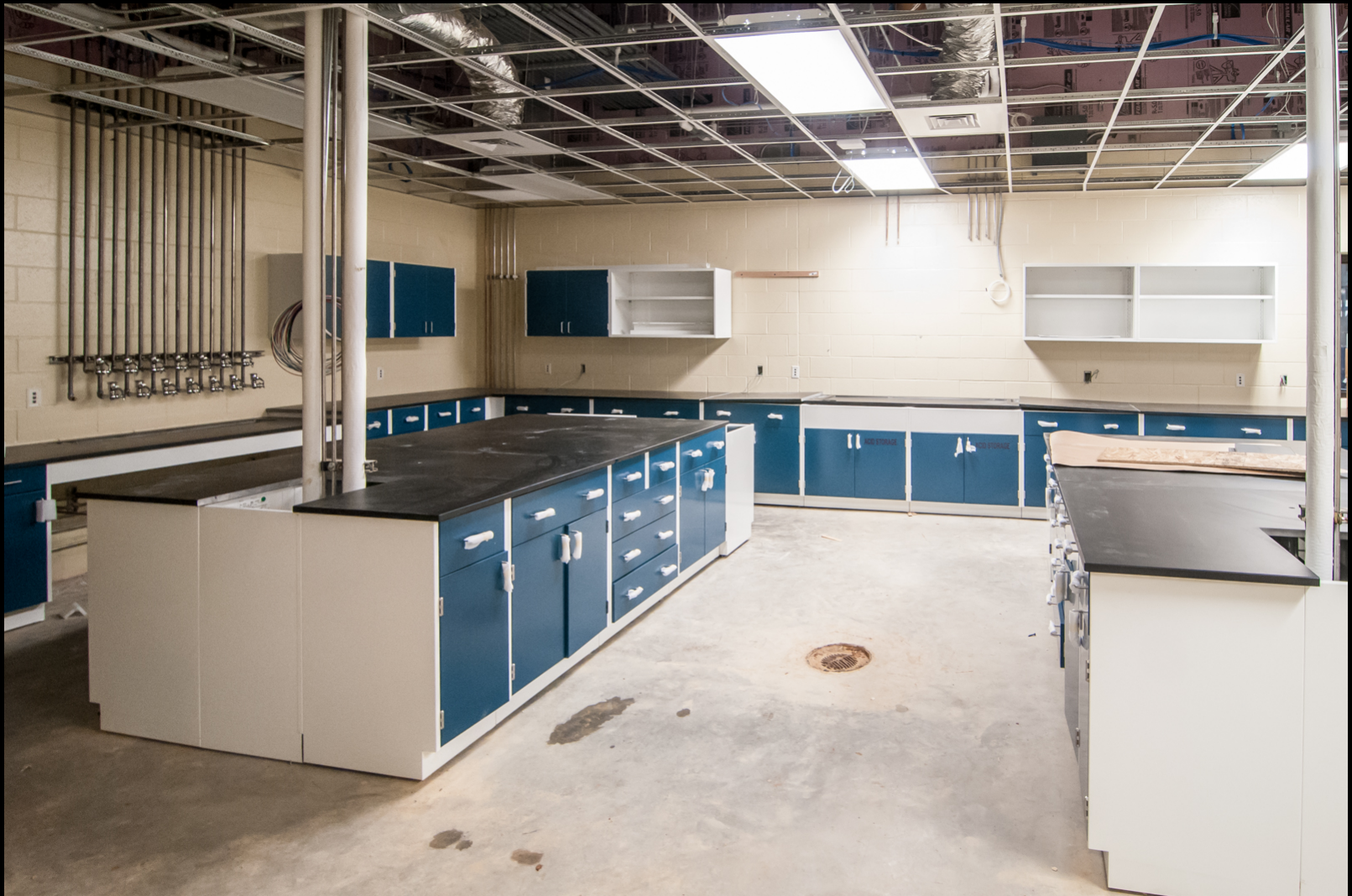
Membrane Building – Lab millwork installation
