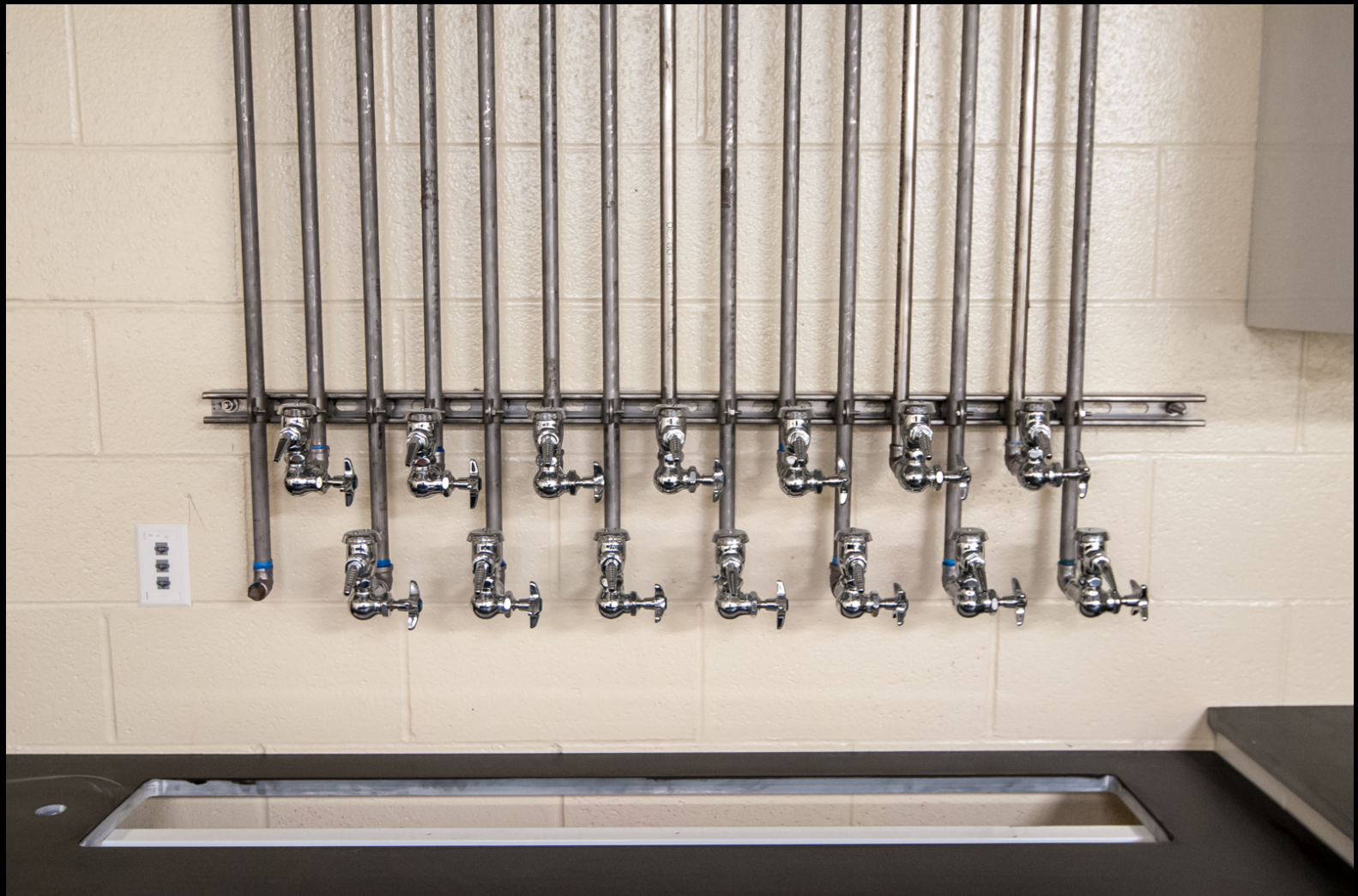
Membrane Building – Installation of process water sample faucets
