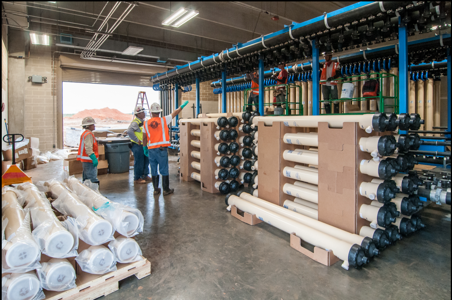
Membrane Building – Installation of membrane cartridges
