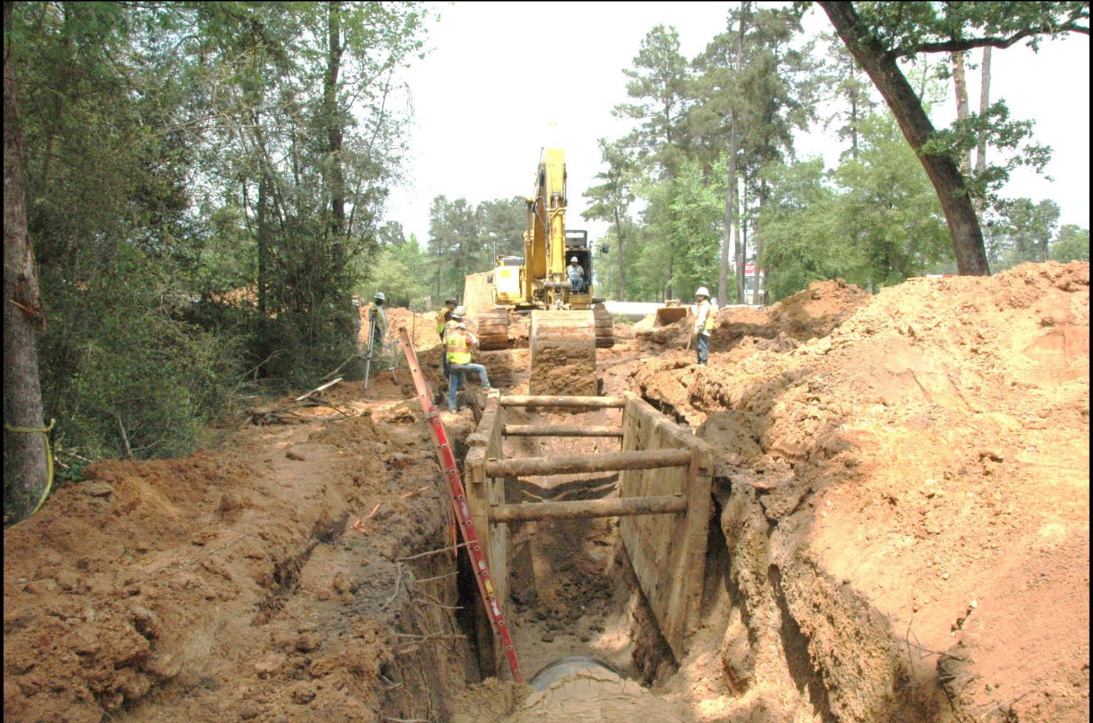
54-inch open cut installation along Sendera Ranch Dr.
