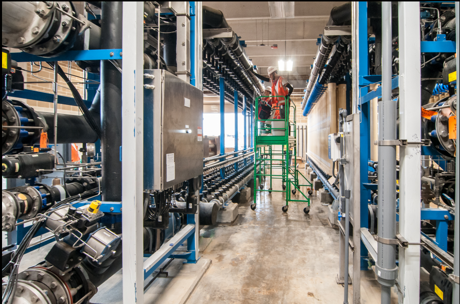
Membrane Building – Installation of membrane cartridges
