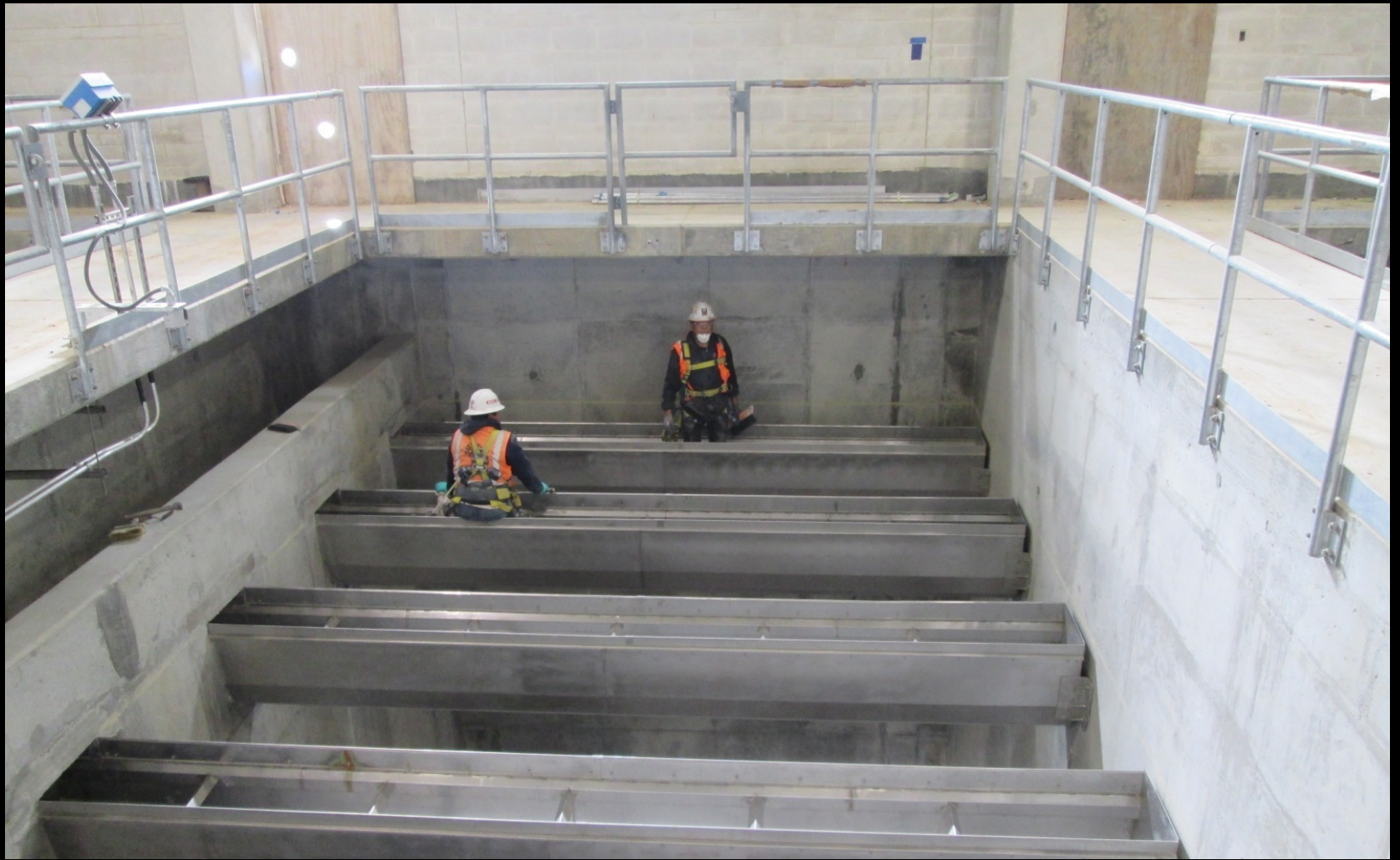
Granulated Activated Carbon Building – Cleaning of contactor trough and basin
