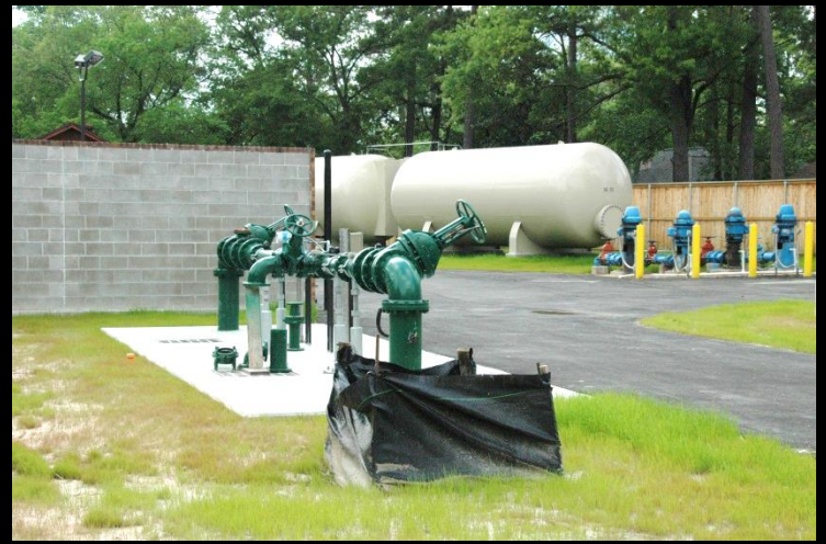
Oak Ridge North Water Receiving Facility
