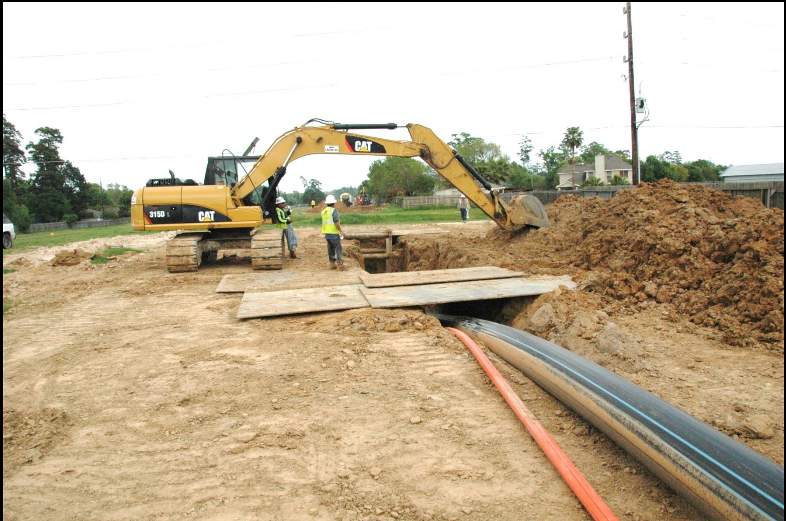
12-inch pipe and 3-inch conduit being installed under MCDD No. 6 drainage ditch
