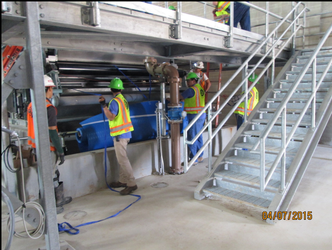
Dewatering Building – Operations Staff installing belts during equipment training
