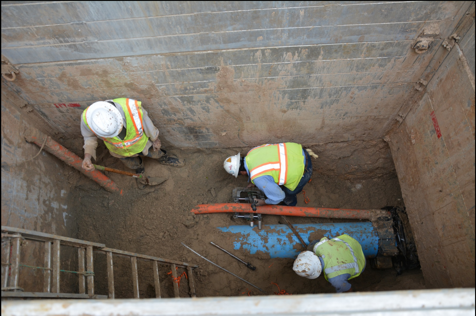
Fusion of fiber conduit adjacent waterline
