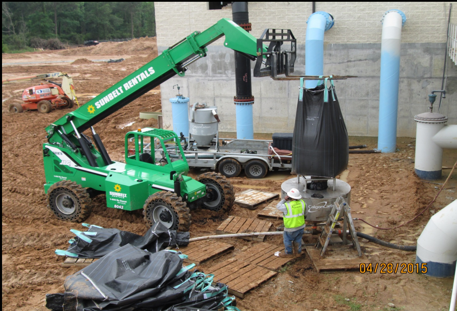
Granulated Activated Carbon Building – Eductor system installation of GAC media
