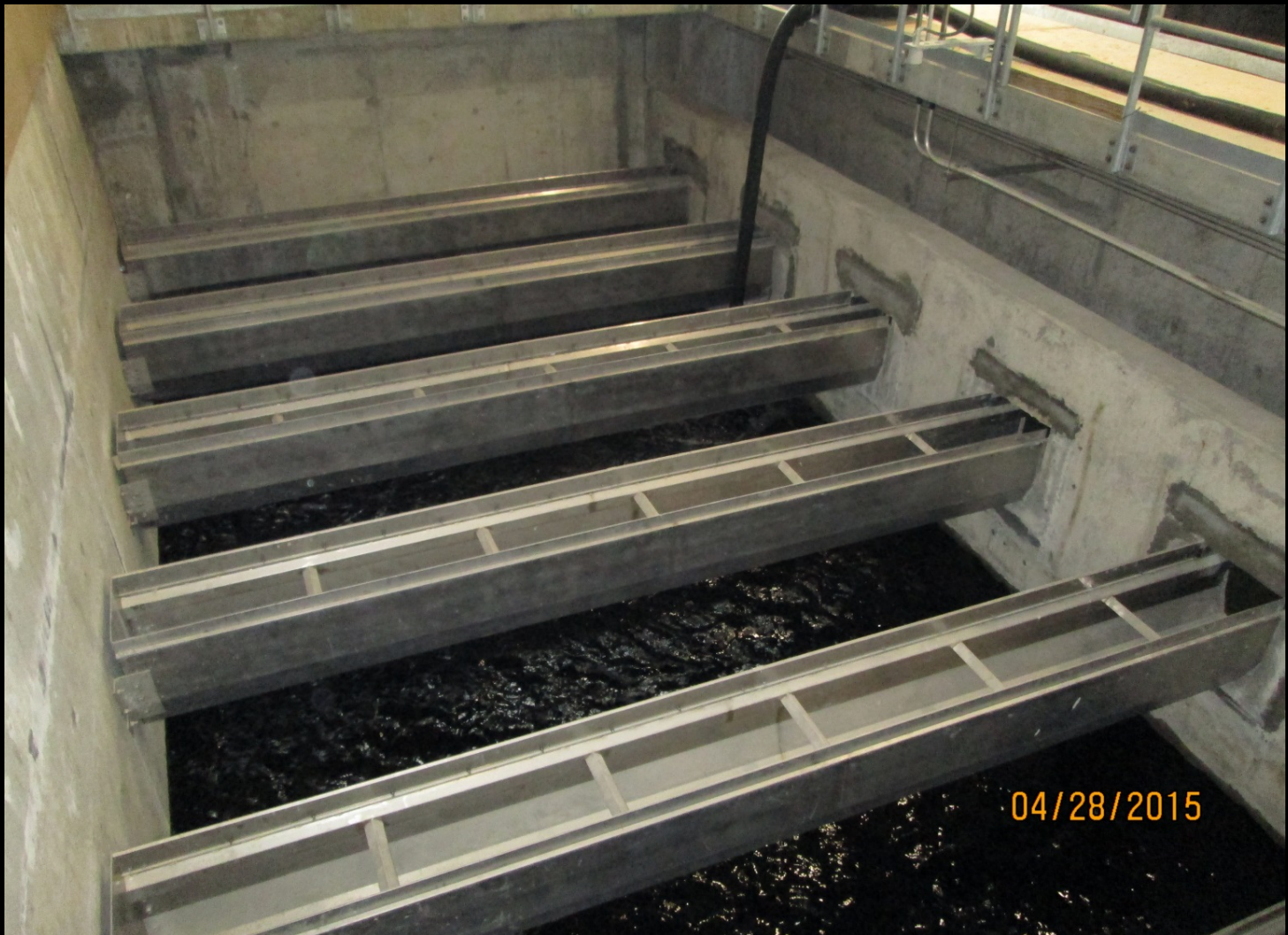
Granulated Activated Carbon Building – Installation of GAC material into contractor basin
