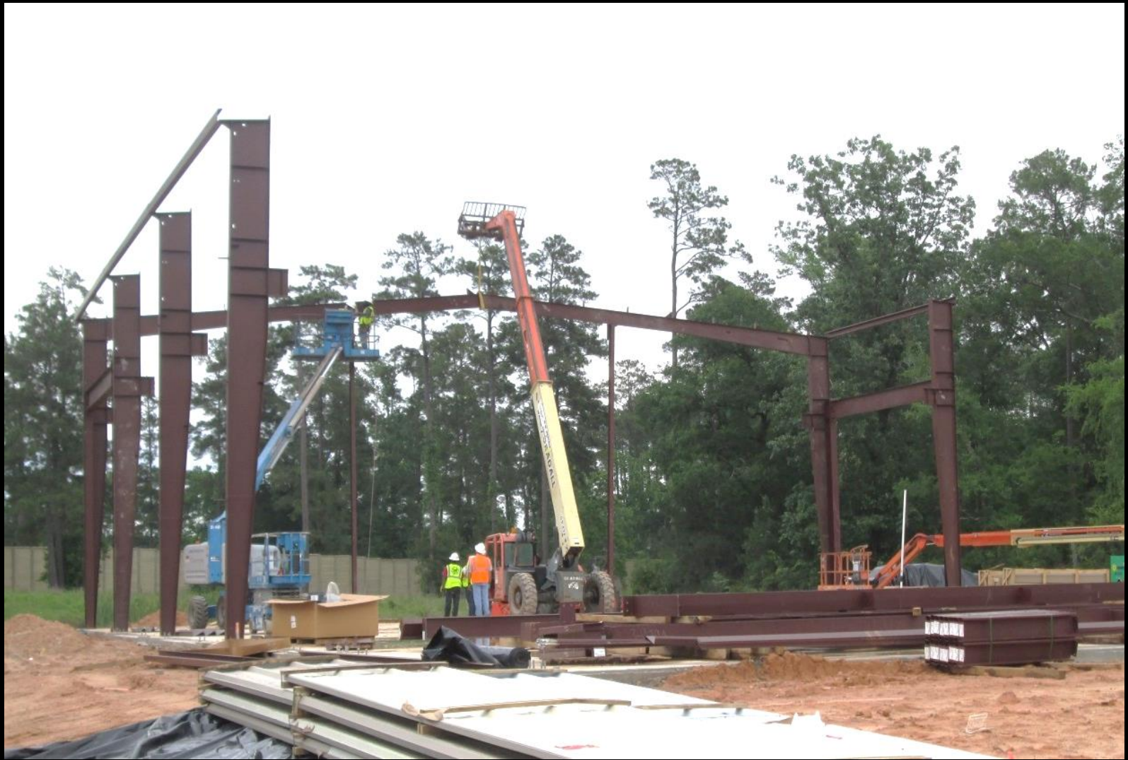
Maintenance Building – Erection of structural steel framing system
