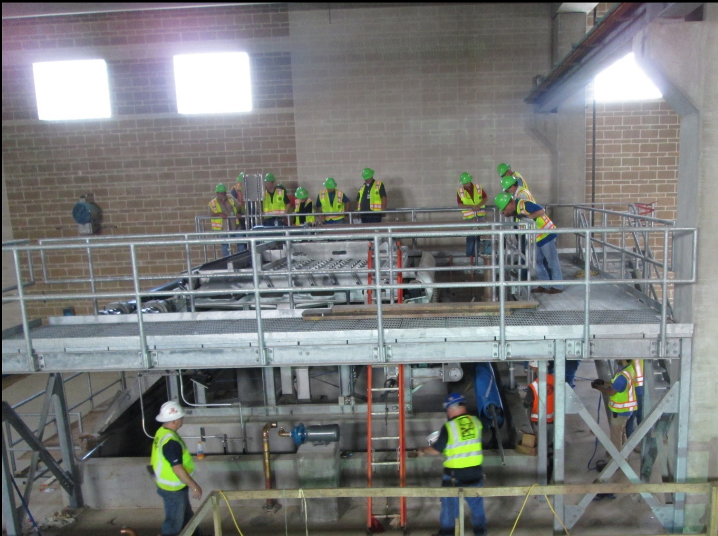
Dewatering Building – Belt Filter Press training for Operations Staff
