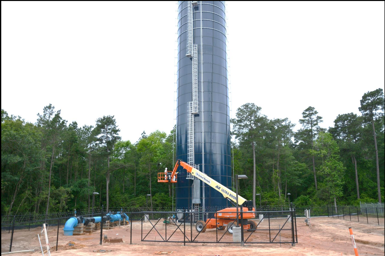
Exterior cleaning of the Standpipe
