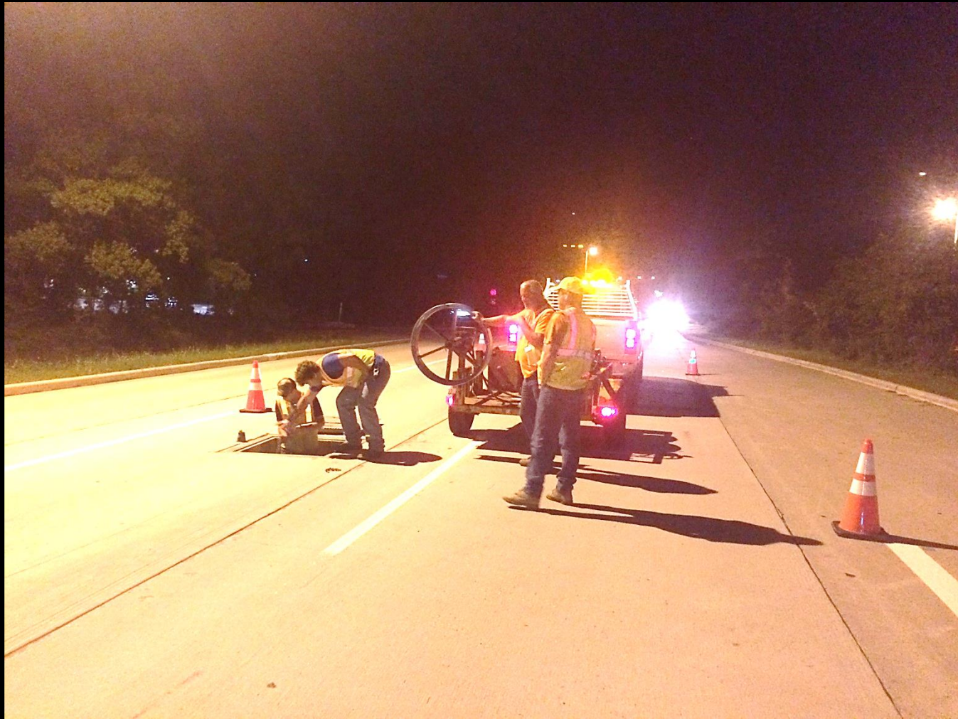
Night time installation of fiber optic cable along Research Forest Drive
