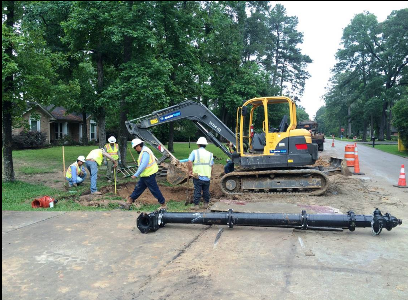
Installation of flushing hydrant adjacent to 16-inch waterline along Maplewood Drive
