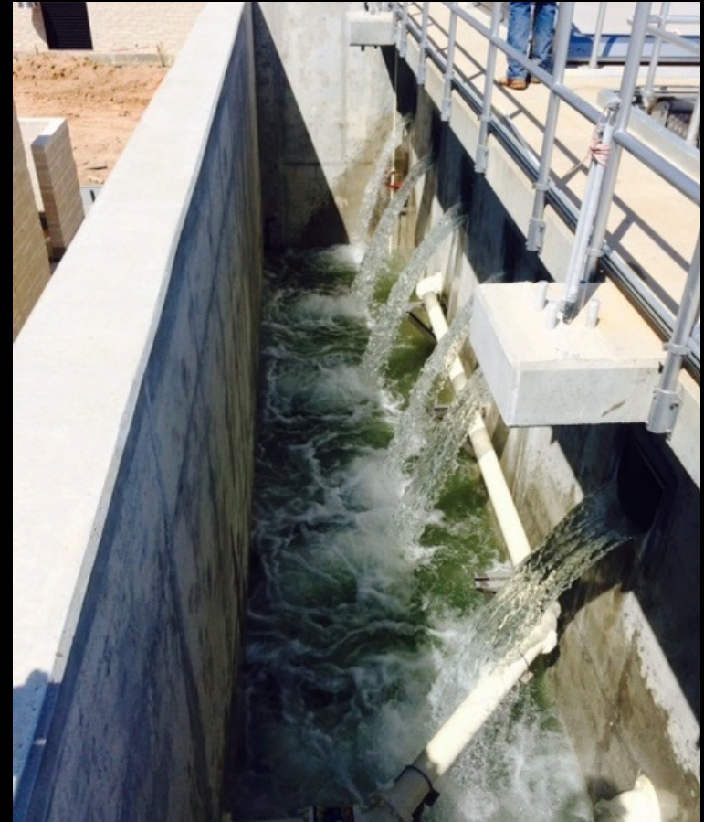
Pretreatment Facility – Raw water flowing through the Pretreatment Basin
