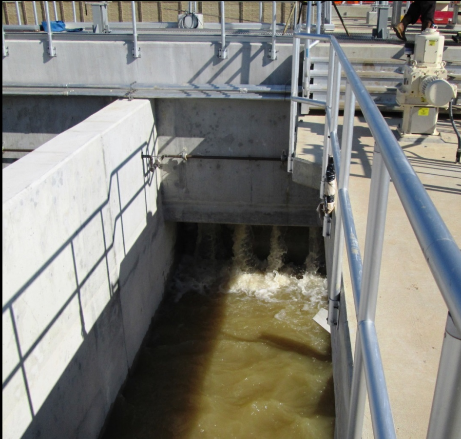
Pretreatment Facility – Raw water flowing through the Pretreatment Basin
