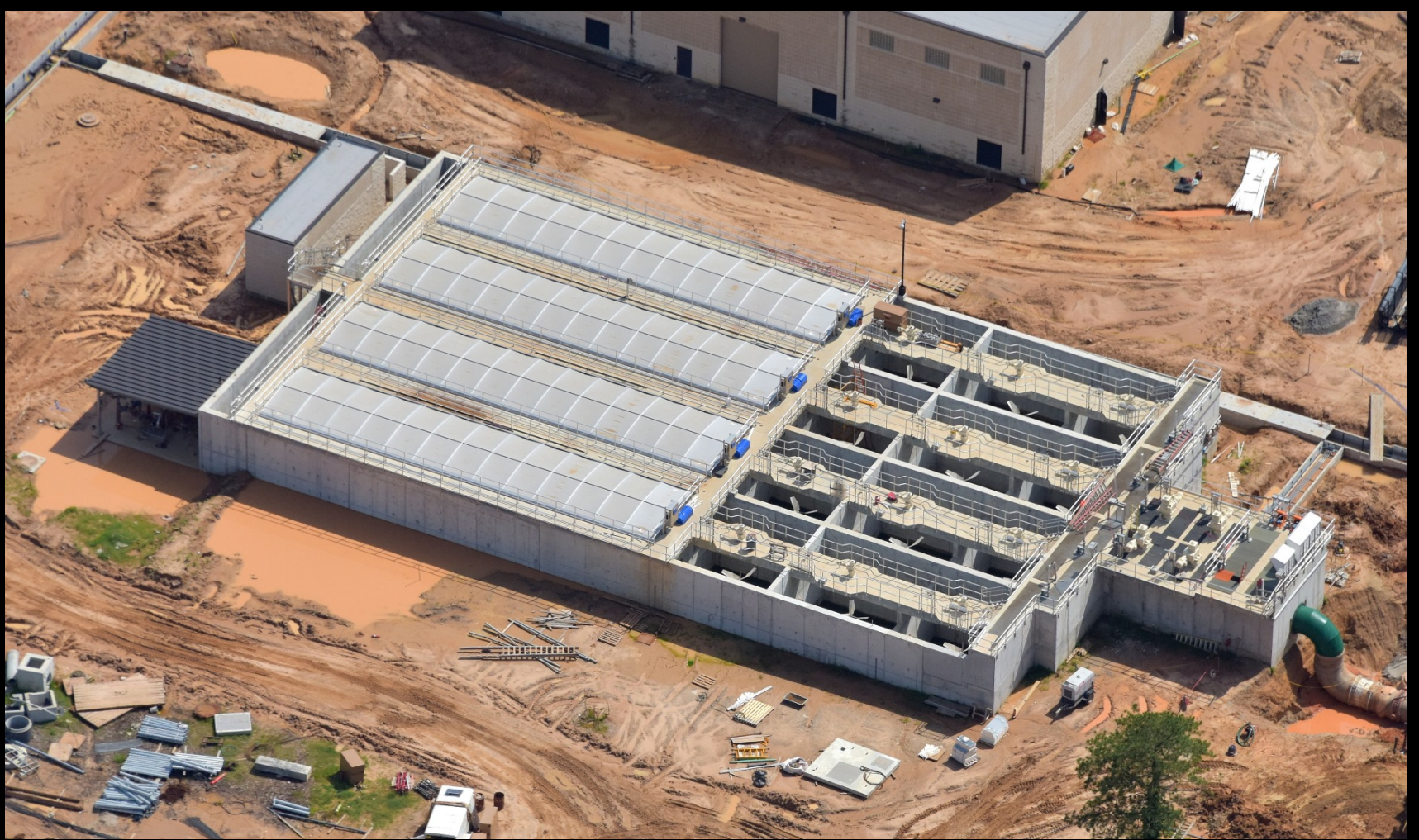
Pretreatment Facility – Covers installed over the suspended solids plate settlers
