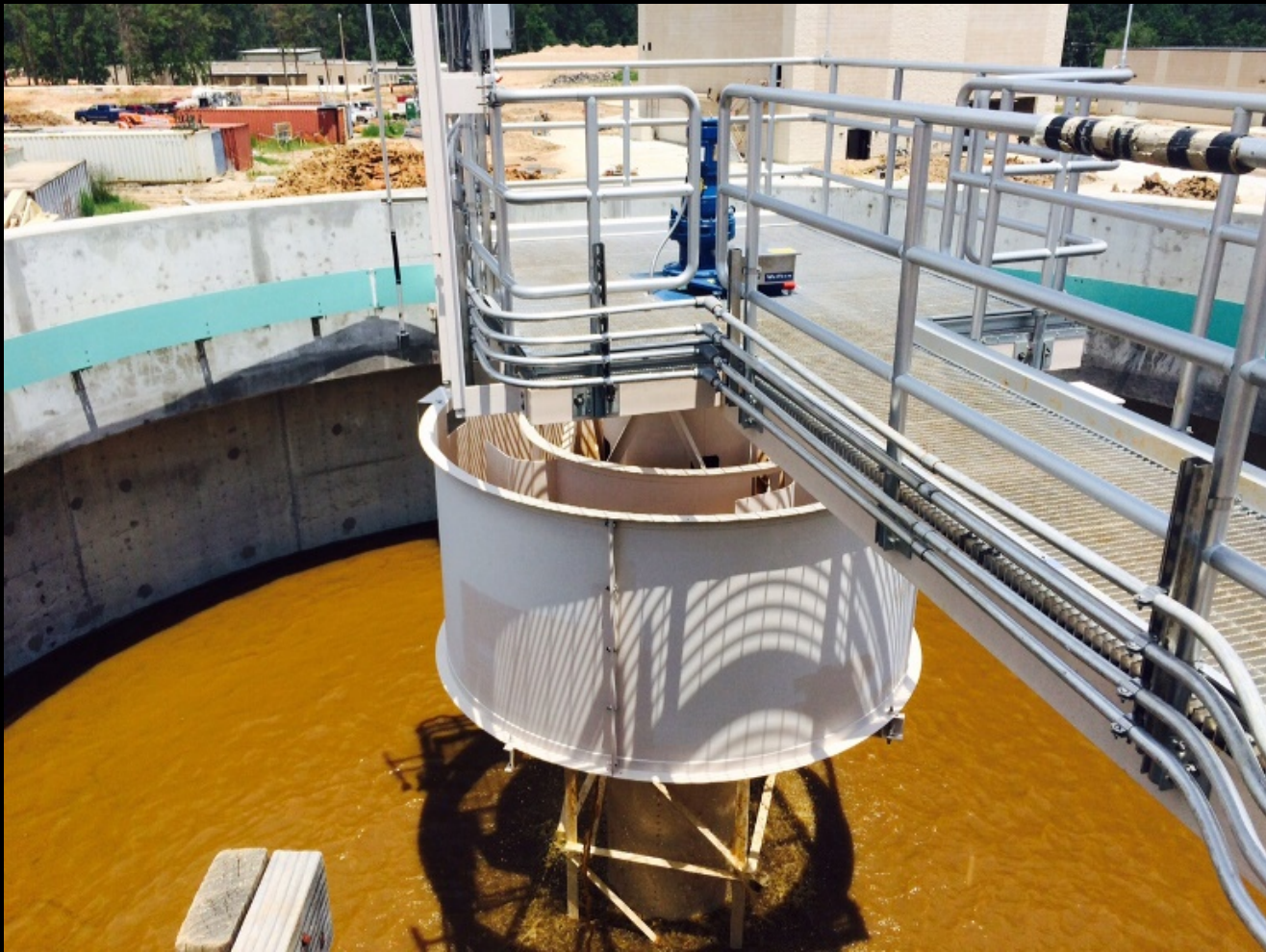
Sludge Thickeners – Solids received from the Pretreatment Facility for sludge formation
