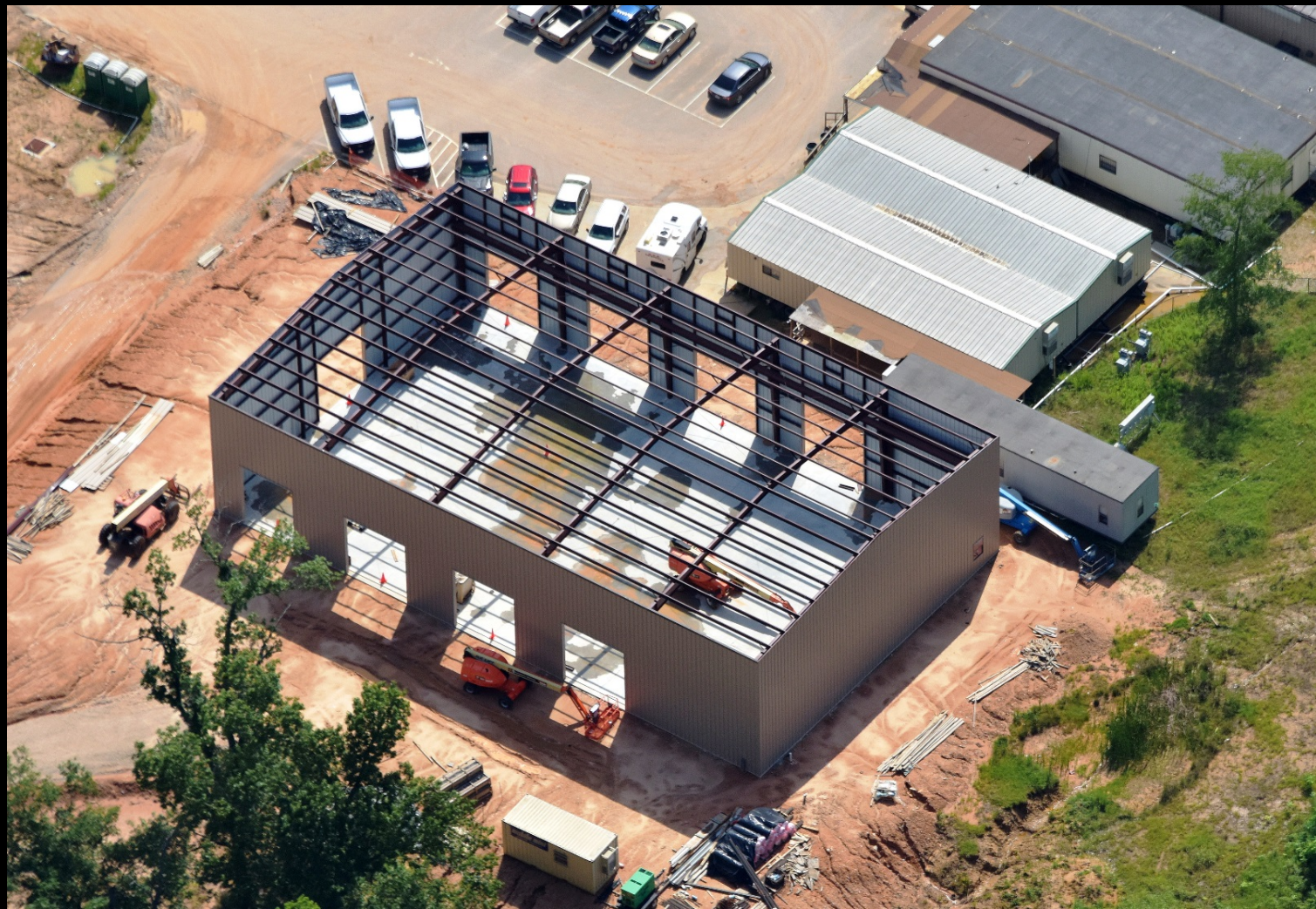
Maintenance Building – Installation of exterior metal wall panels
