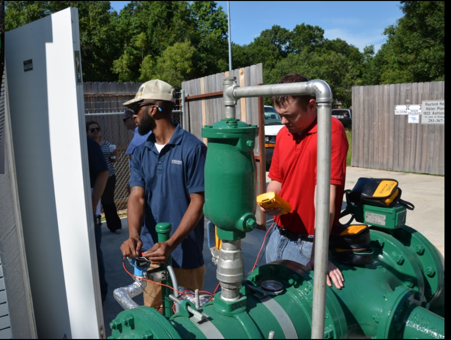
System Improvements - SCADA PLC communication check-out at Rayford Rd. MUD's Water Plant No. 2
