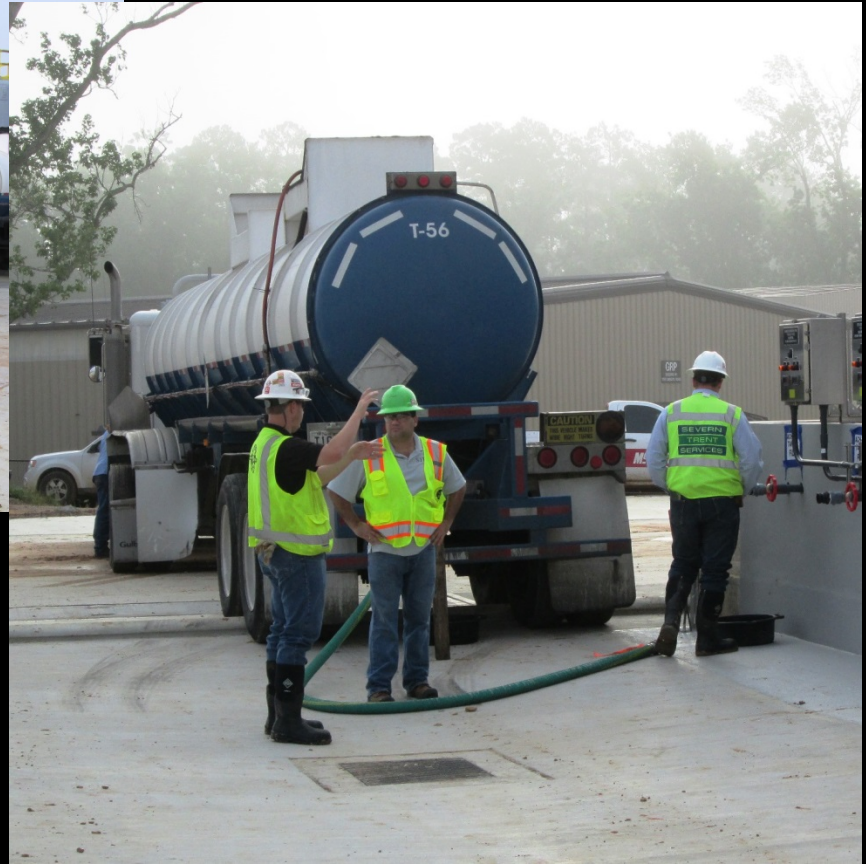
Chemical System— The first chemical delivery (Aluminum Chlorohydrate)
