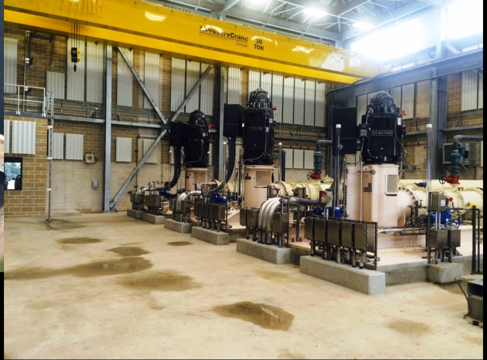
Raw Water Intake – Aerial and final cleaning in progress
