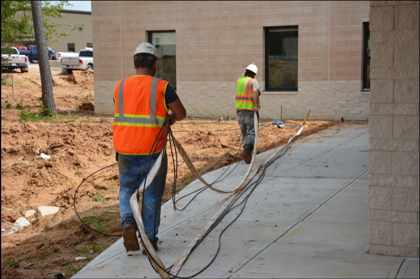
Layout of fiber optic cable prior to installation into the GRP Operations Building
