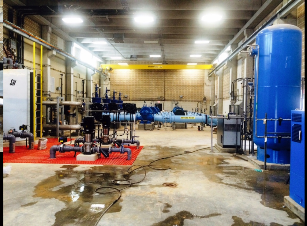
Membrane Building – Final cleaning of pump room in progress
