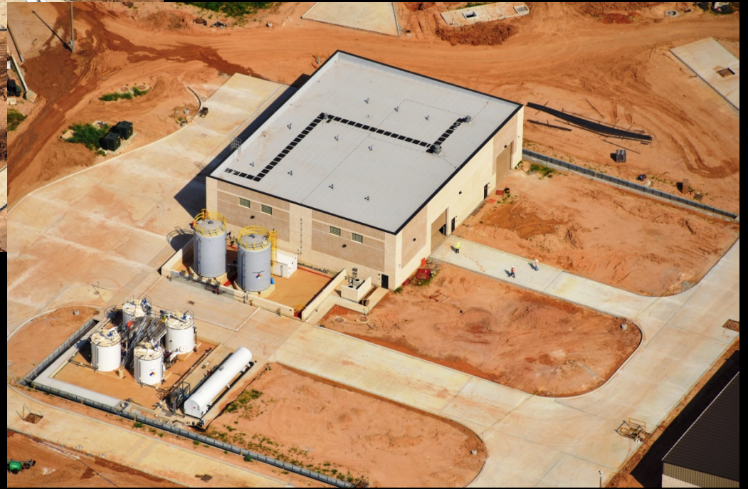
Sitework – Paving and final grading of the project site
