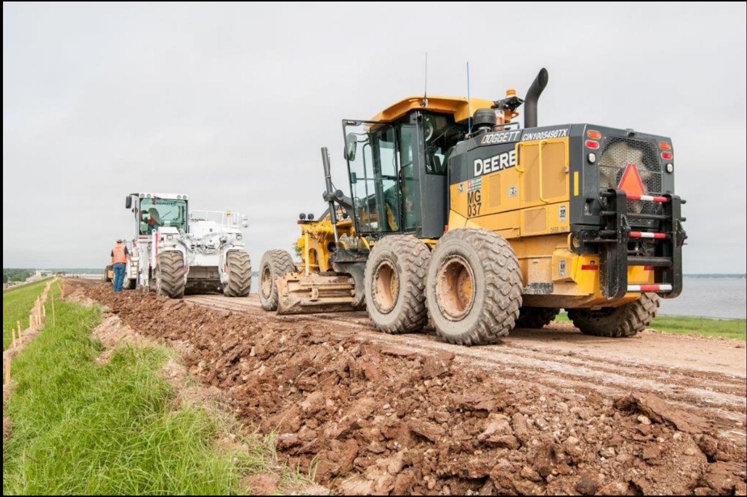
Sitework – Reconstruction of the Dam road
