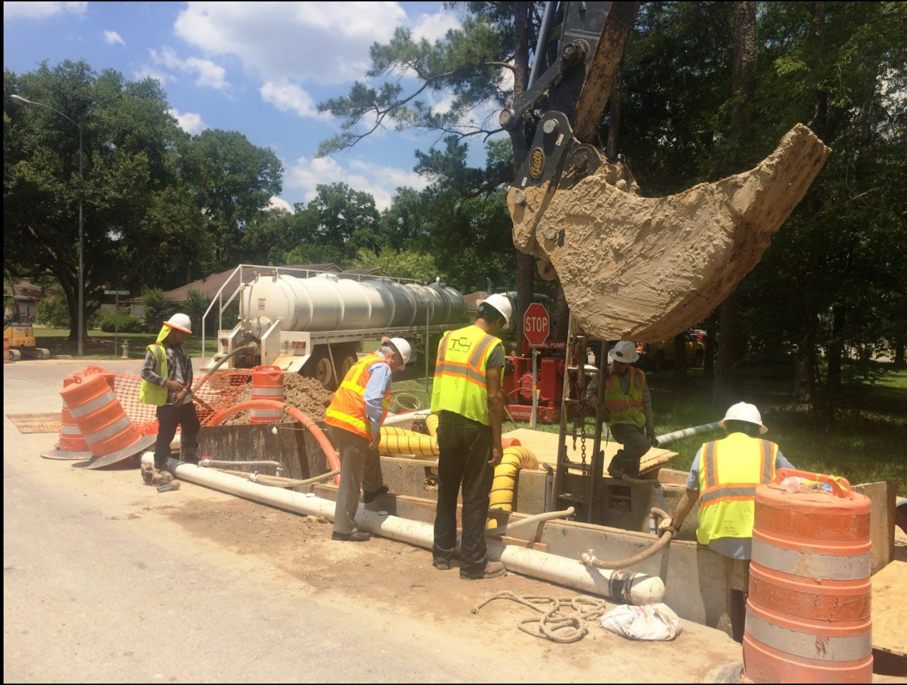
Auger pit for installation of 30" steel casing under high pressure gas lines
