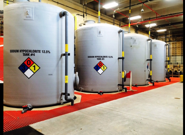
Chemical Building – Final cleaning in progress
