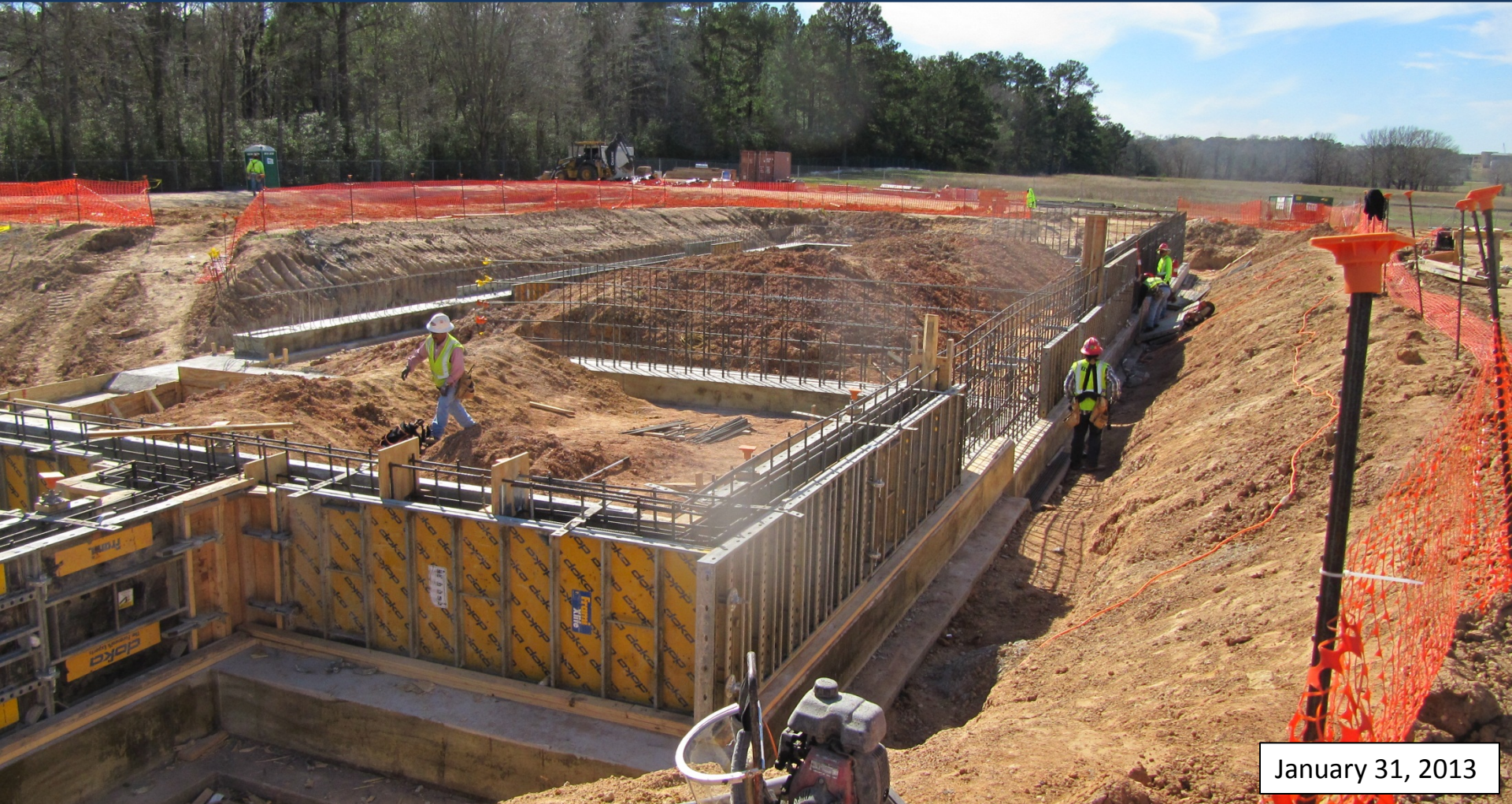
Foundation stem wall (grade beams) installation
