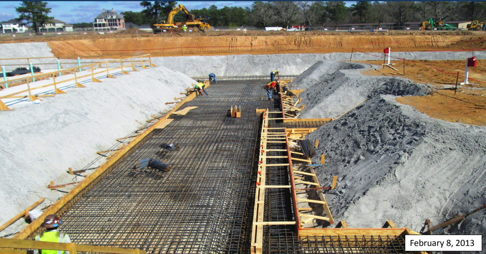
Lower trench drain foundation for the Membrane Building
