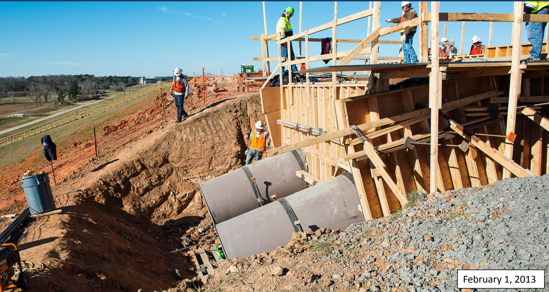
Dual 48” Raw Water piping installation thru the crest of the Dam
