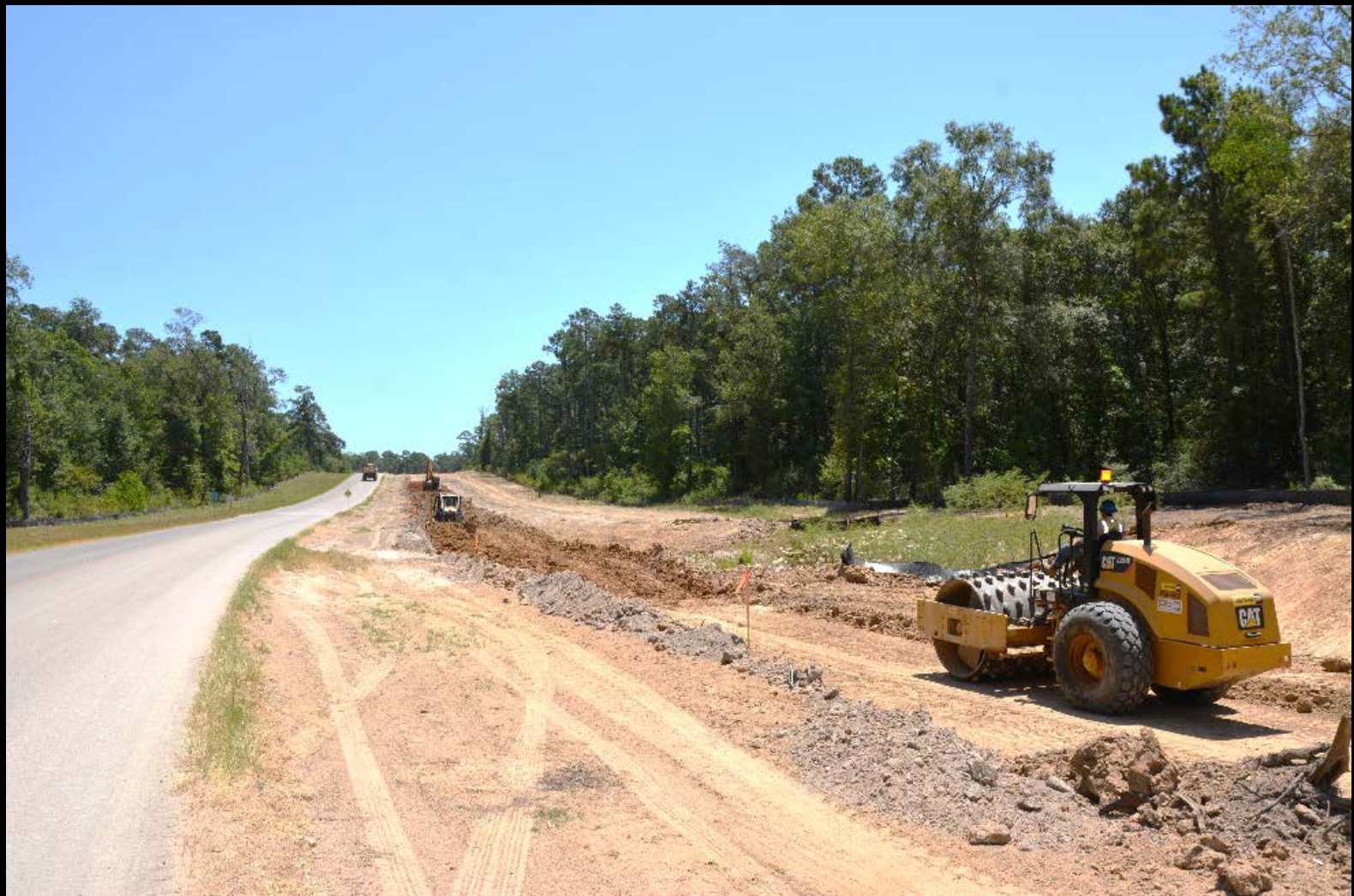
Access Road – Subgrade preparation for eastbound boulevard section
