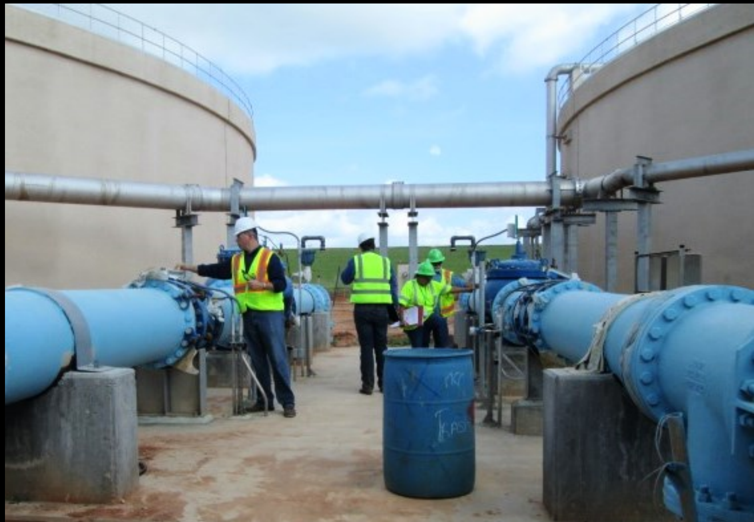
Punchlist inspection with SJRA Staff and Engineers of Record
