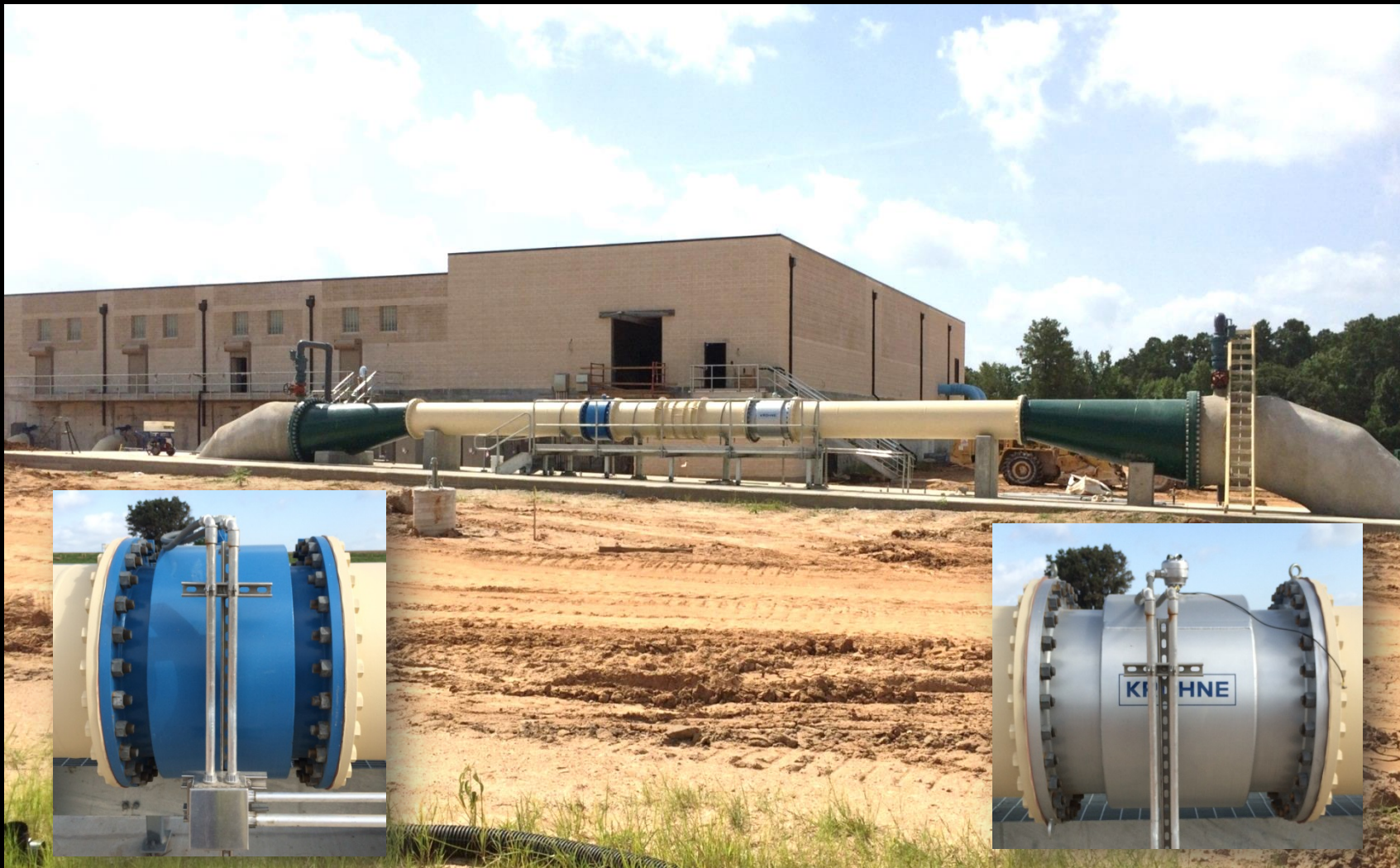
Flow meters ranging from 54-inch to 3/8-inch
