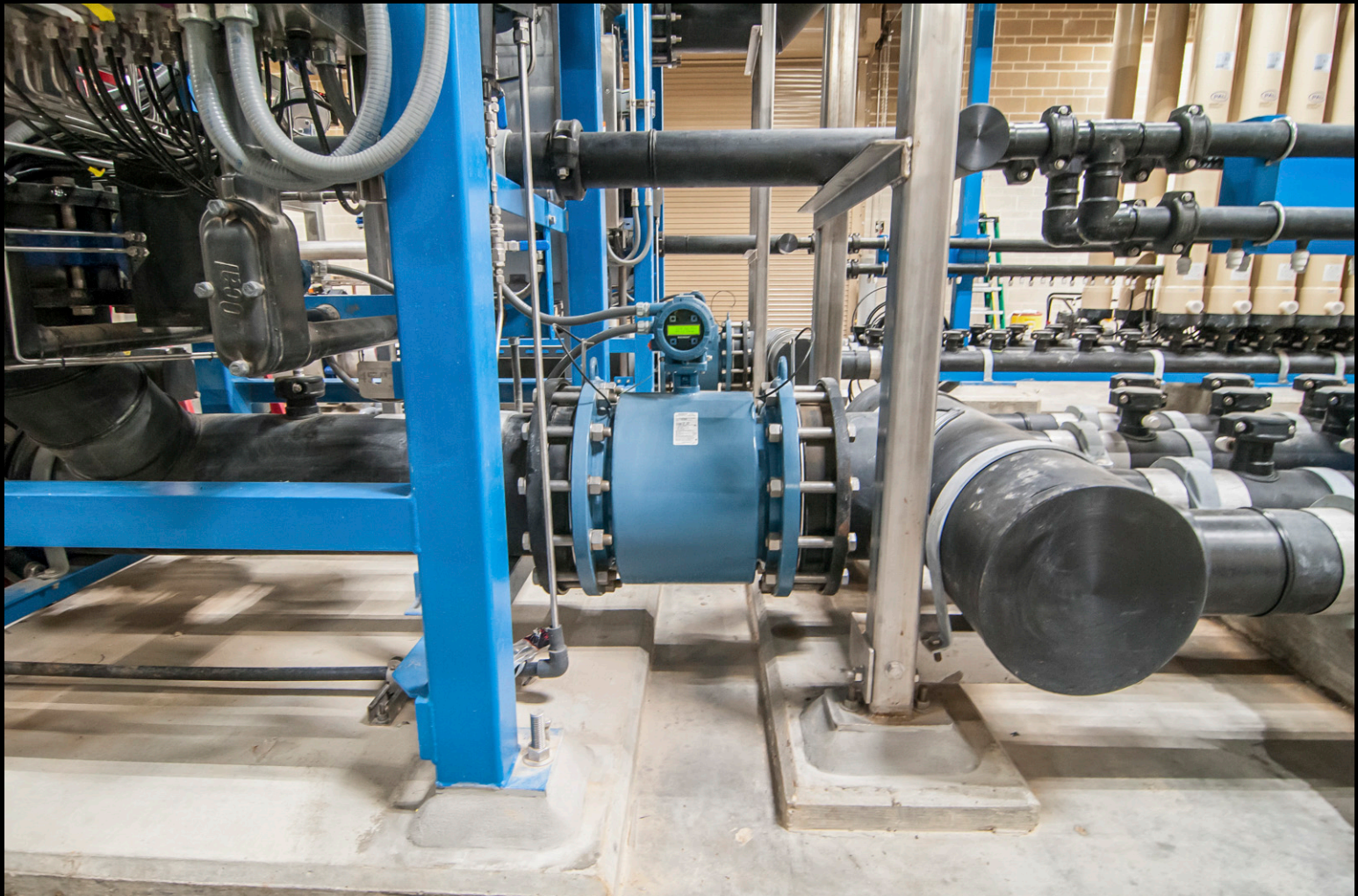
Flow meters on the membrane system
