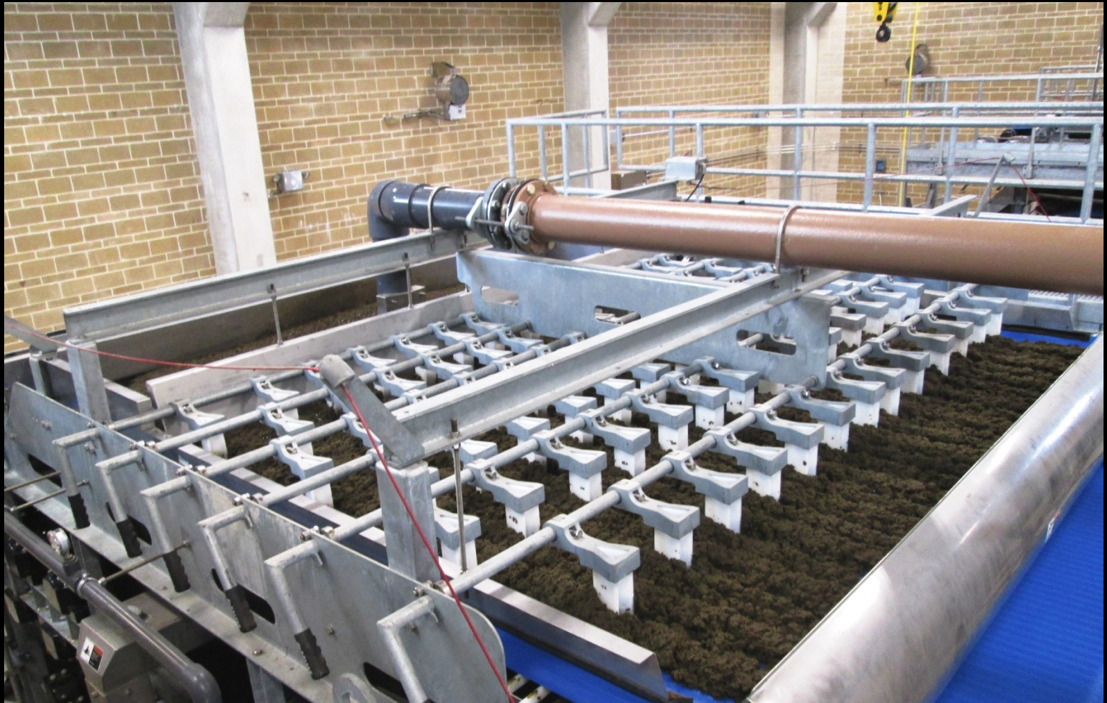
Solids dewatering system in operation
