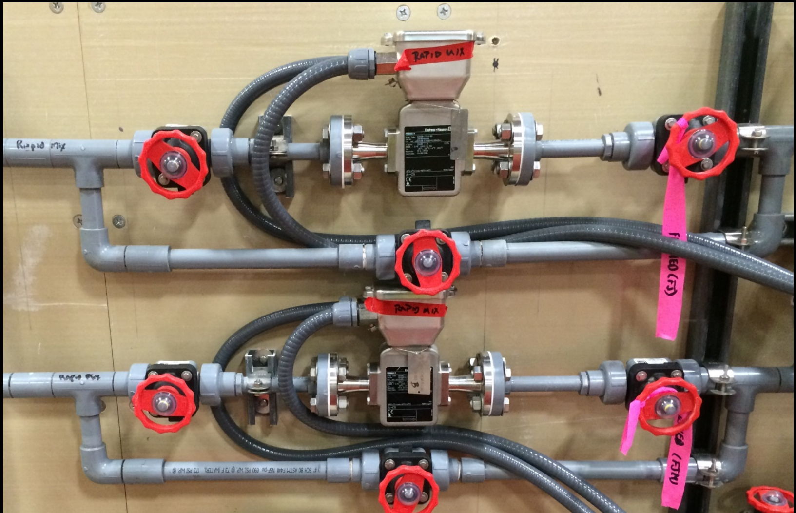
Flow meters for chemical supply system
