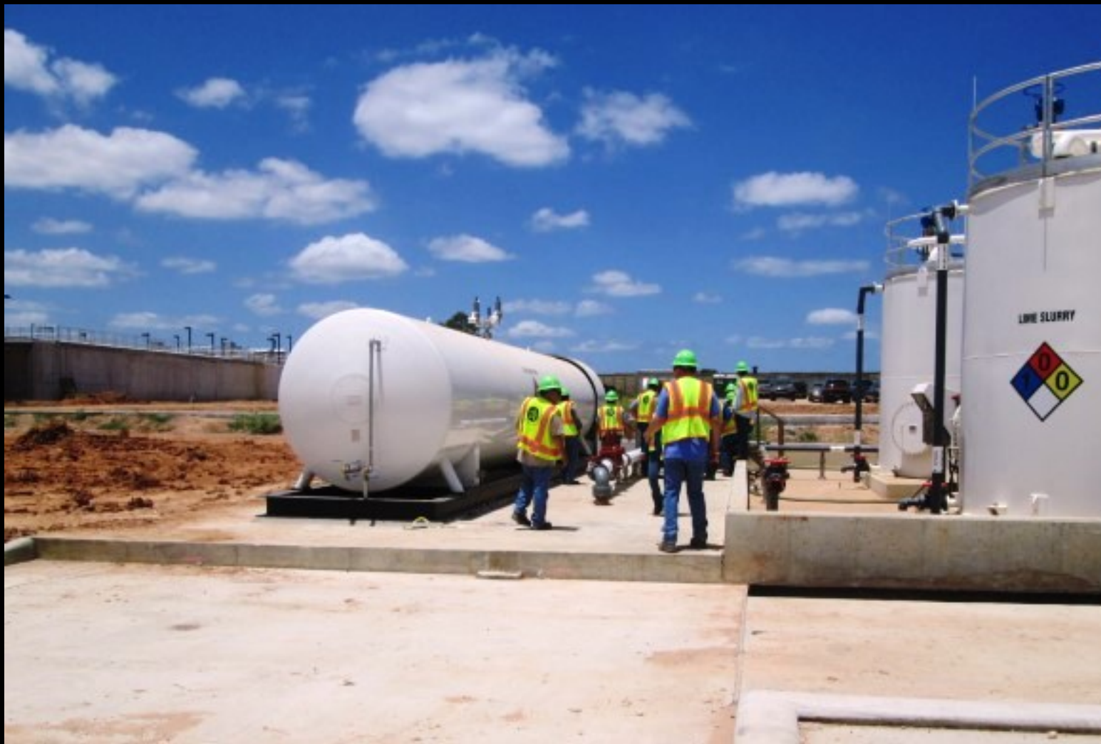
Carbon dioxide (CO 2 ) system training for Operations Staff
