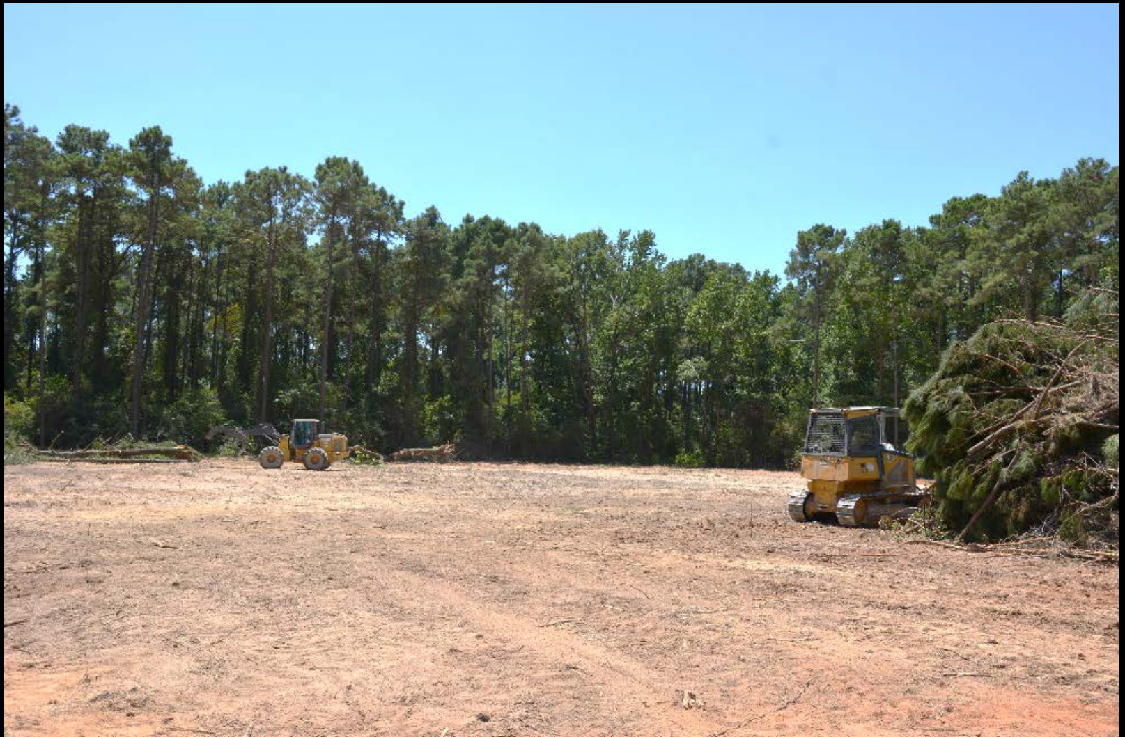
Access Road – Detention pond clearing and grubbing
