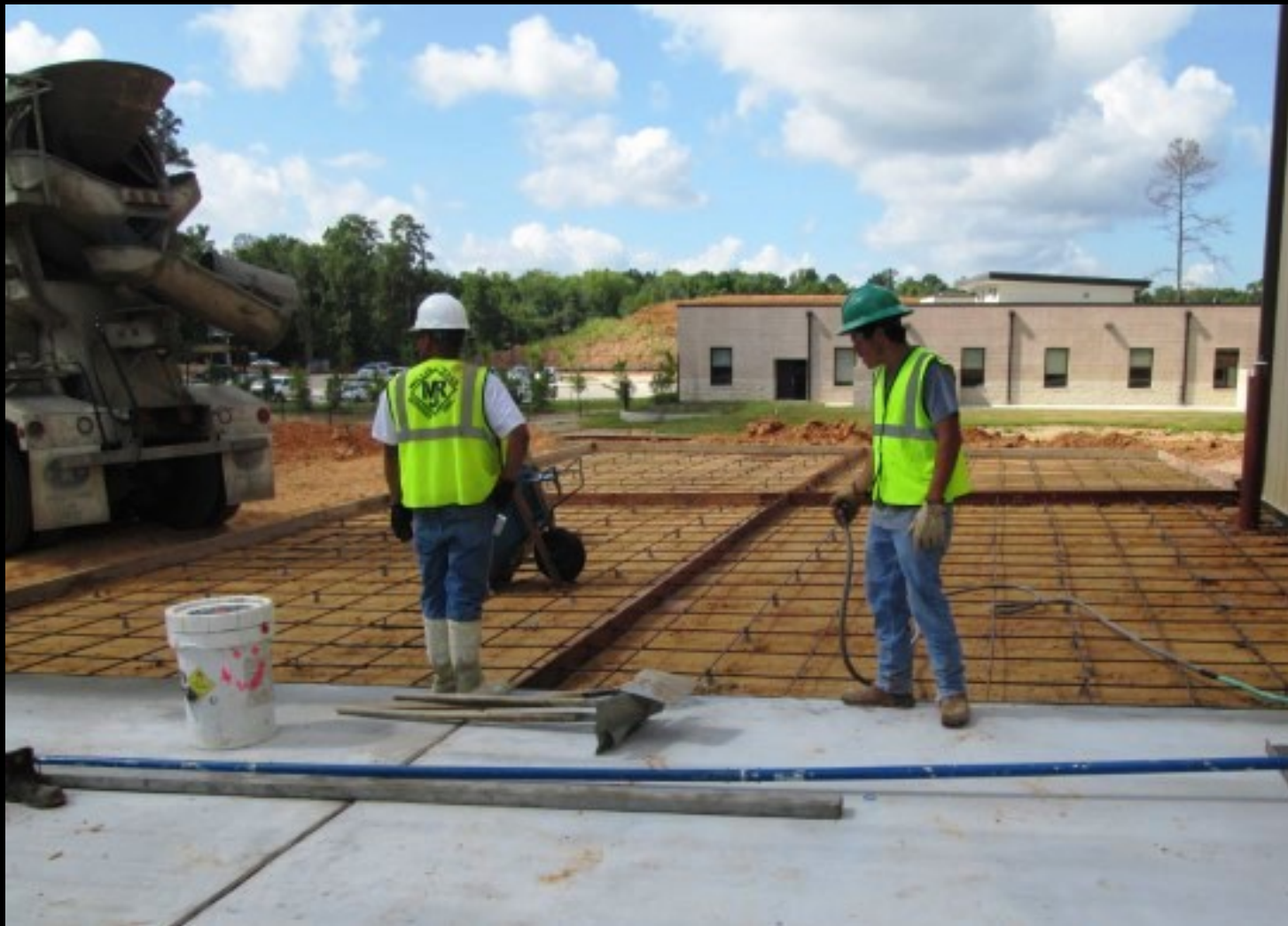
Continued concrete paving throughout the site
