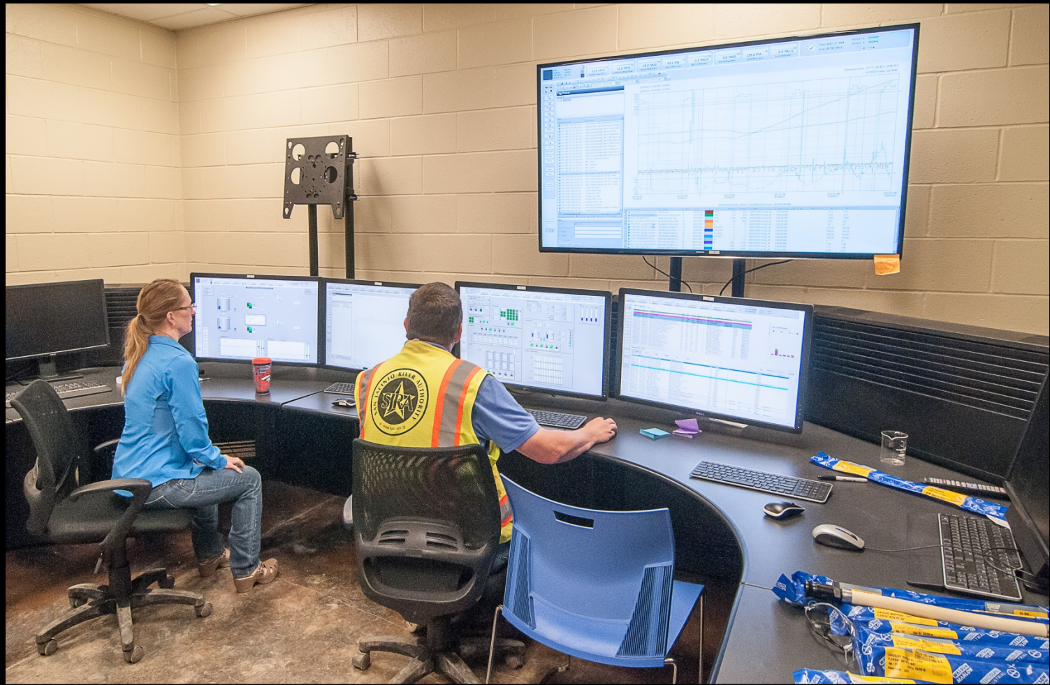
Membrane Building Control Room
