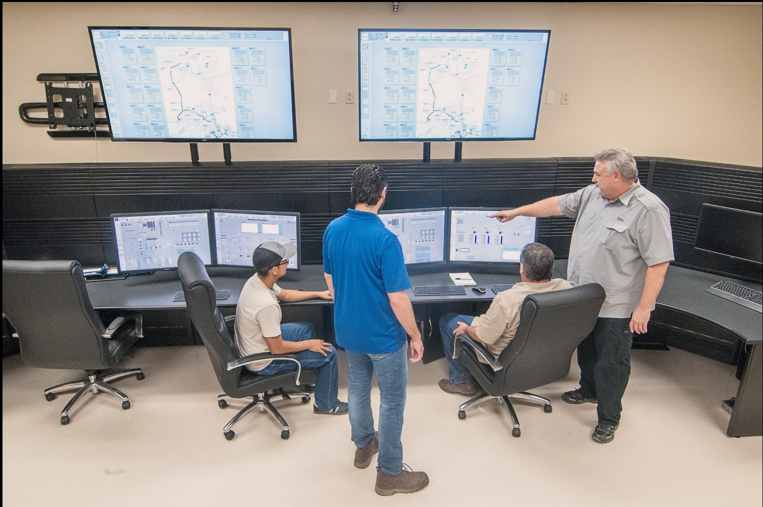
Operations Building Control Room
