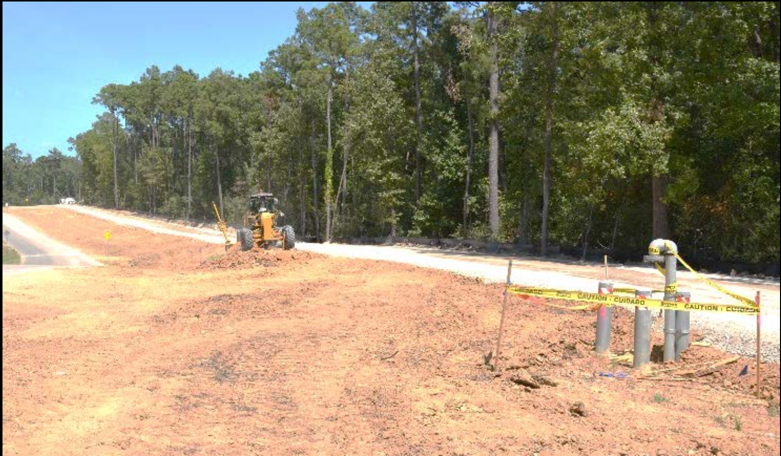
Access Road –Temporary bypass roadway installation
