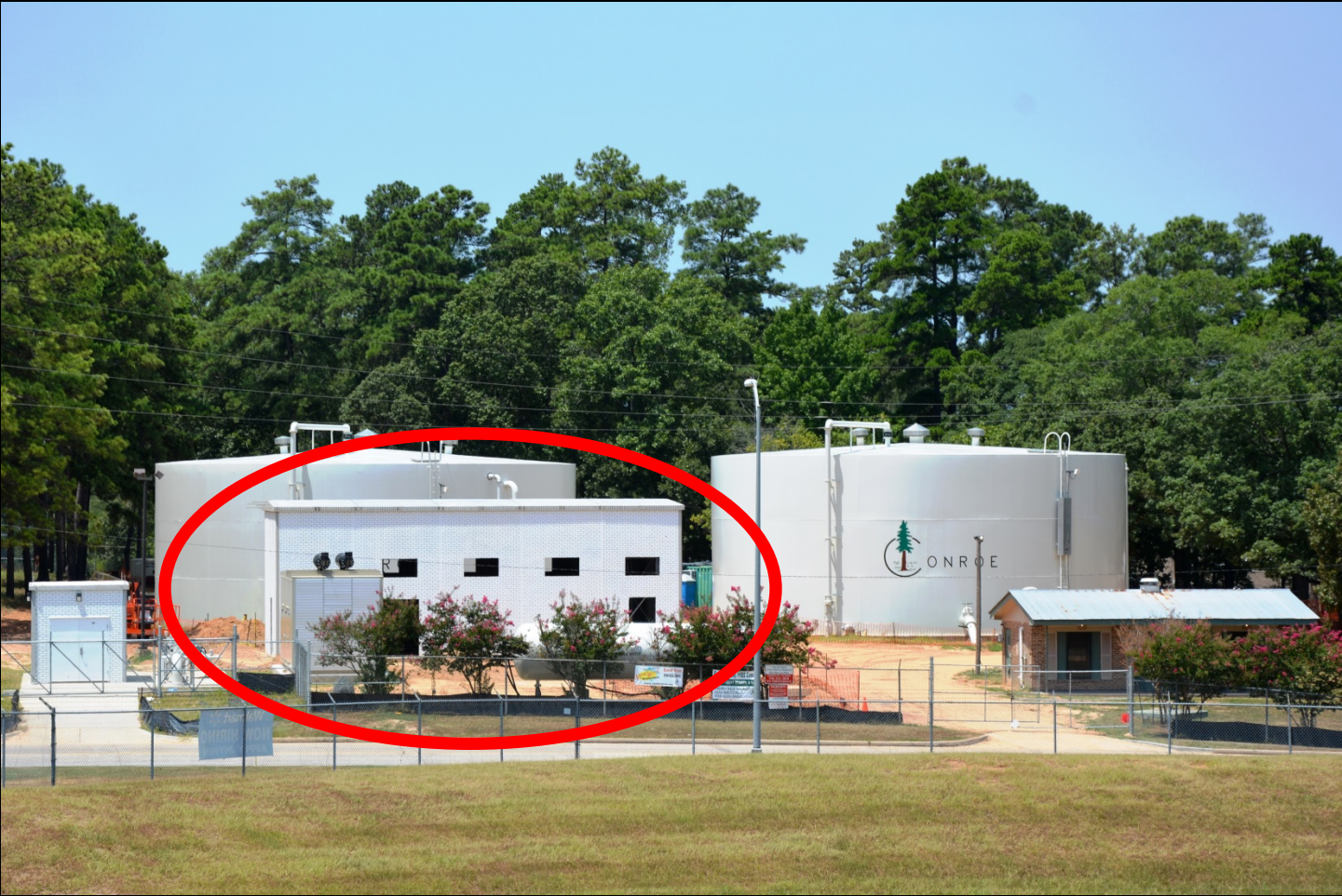
New pump building and generator at Conroe Water Plant No. 6
