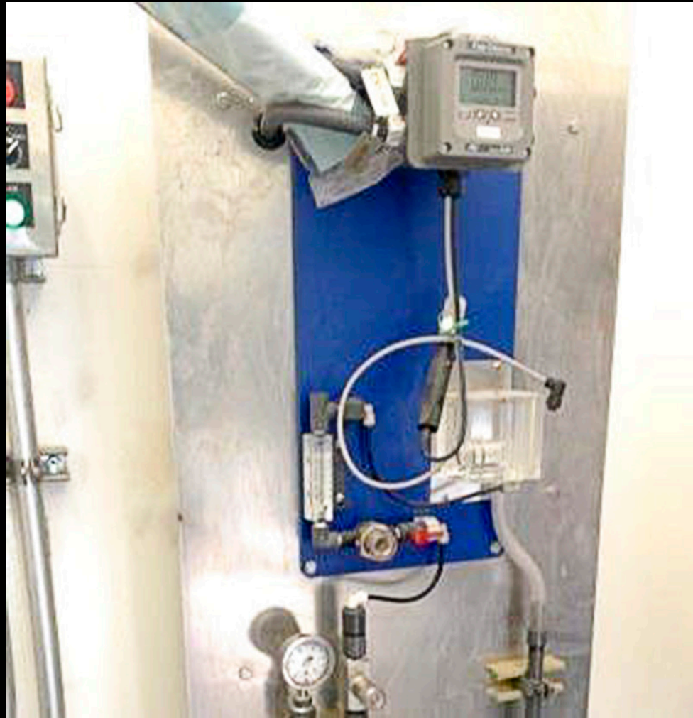
Water Receiving Facility chlorine analyzer
