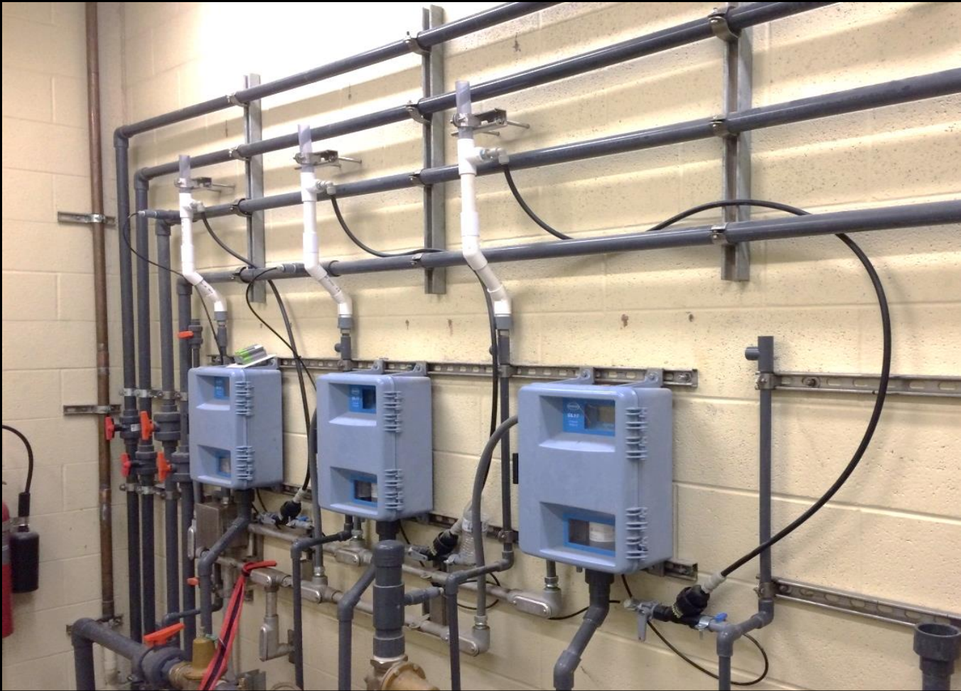
Surface Water Treatment Plant chlorine analyzers
