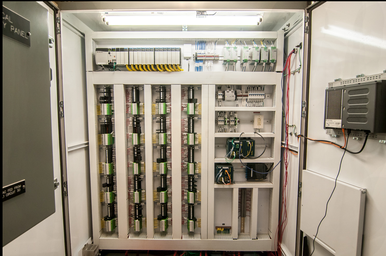
Programmable Logic Controller (PLC) panel - Programmed by SJRA
