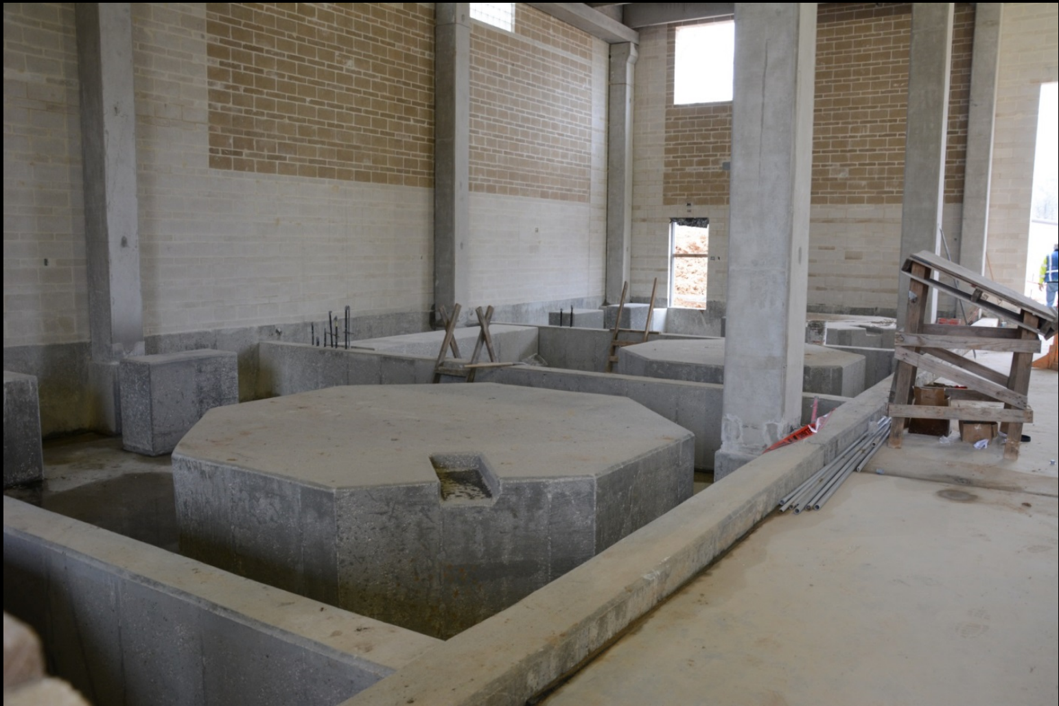
Previous progress photograph
