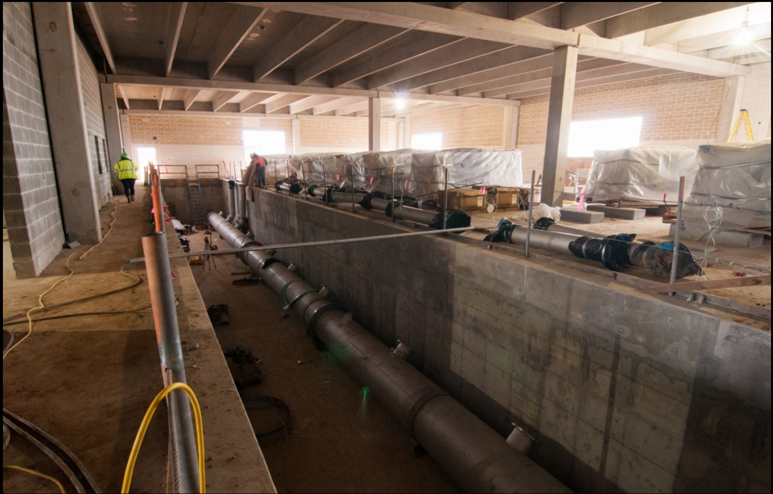
Membrane Building – Previous progress photograph
