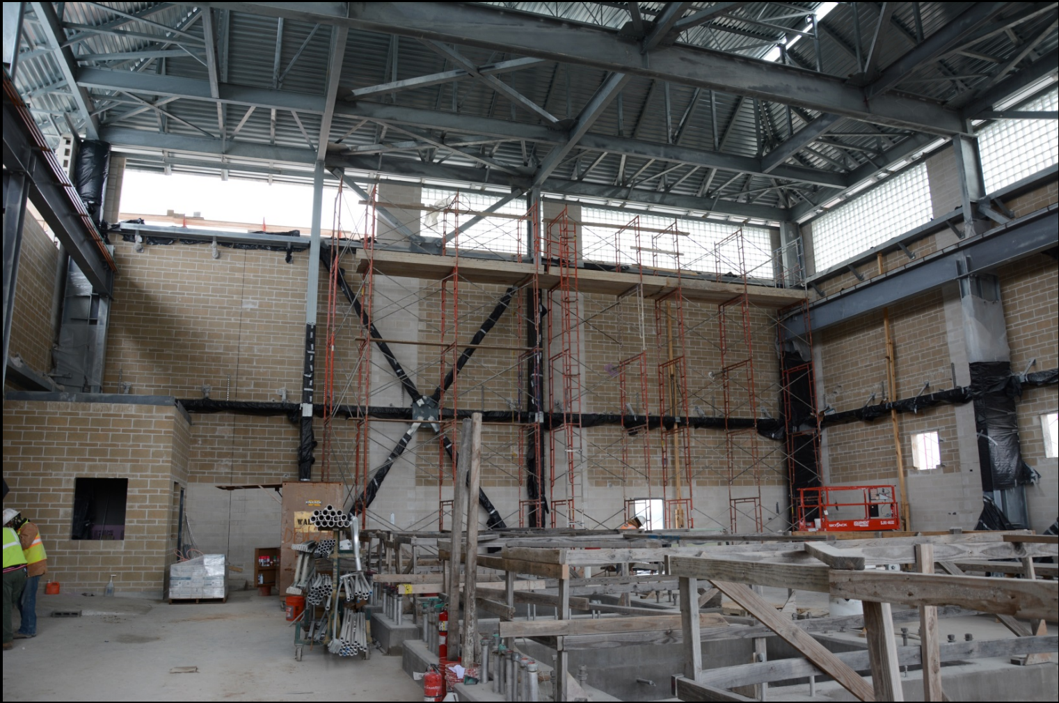
Previous progress photograph
