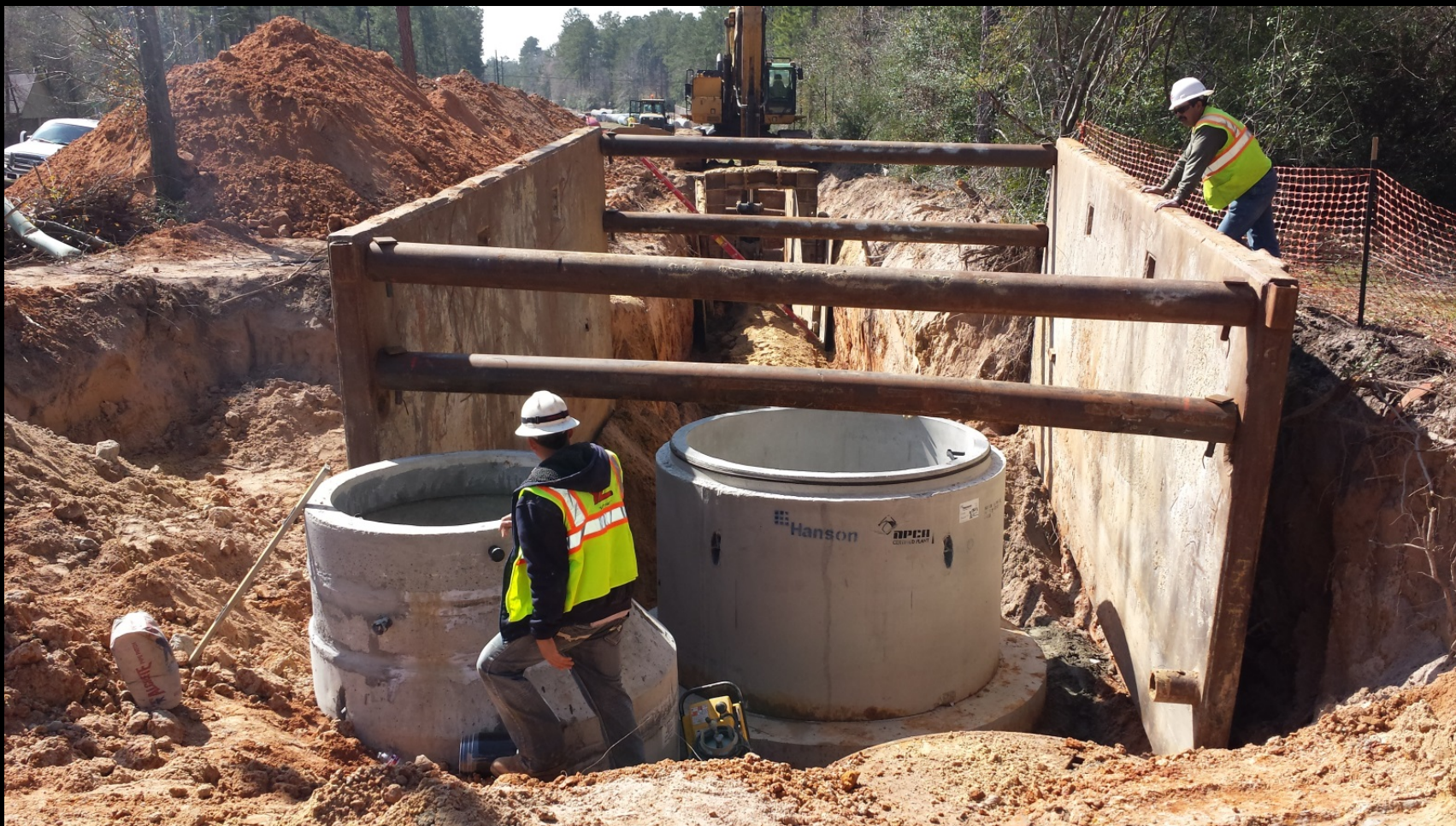
Manhole installation along Sendera Ranch Road
