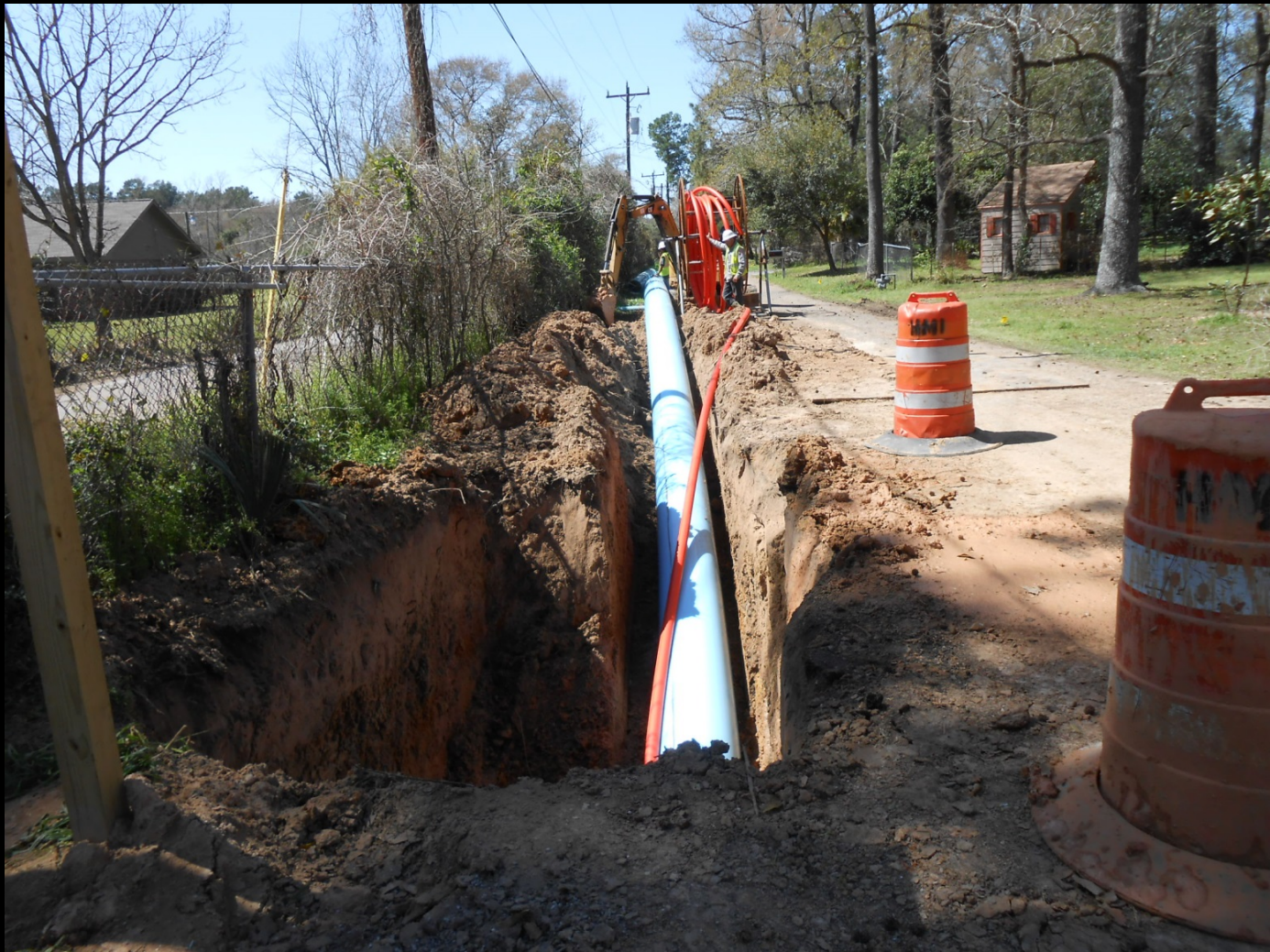
Pipe and Fiber Optic Conduit Installation at Sun Perch Road and Catfish Lane
