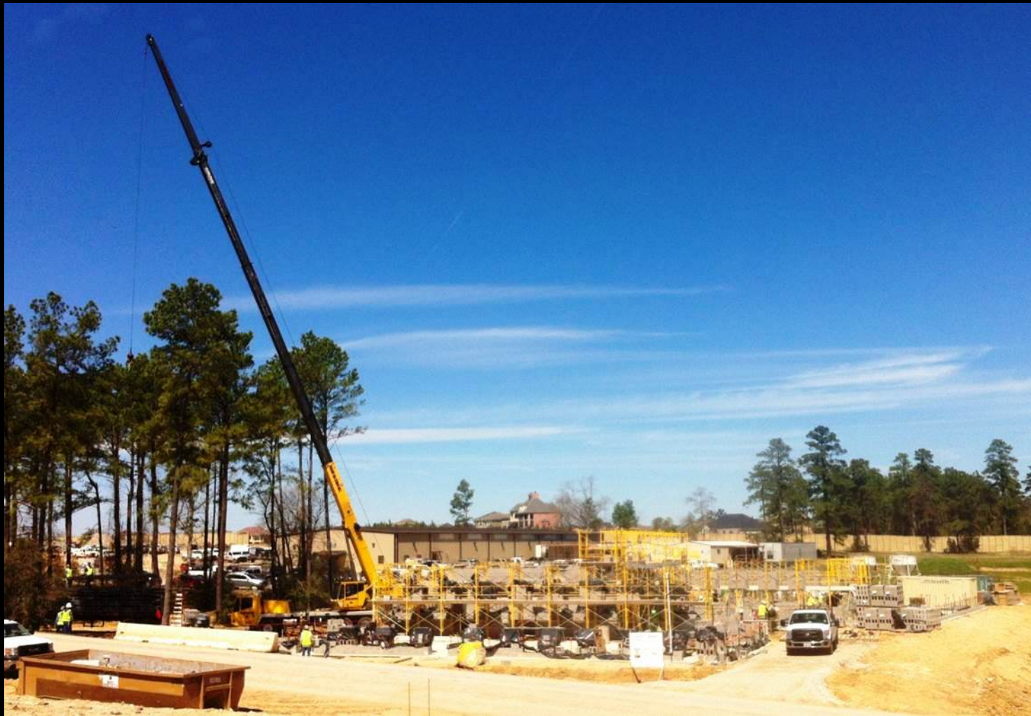
Masonry installation in progress
