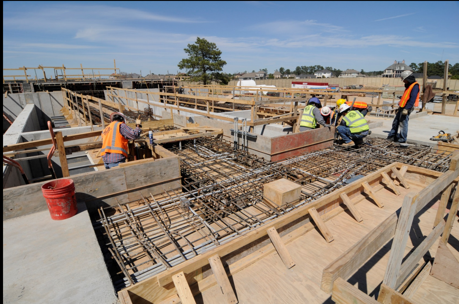
Pretreatment Facility - Access walk way installation
