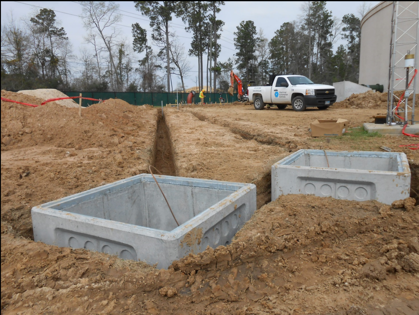
Electrical junction box installation and duct bank excavation at SJRA Water Plant No. 4
