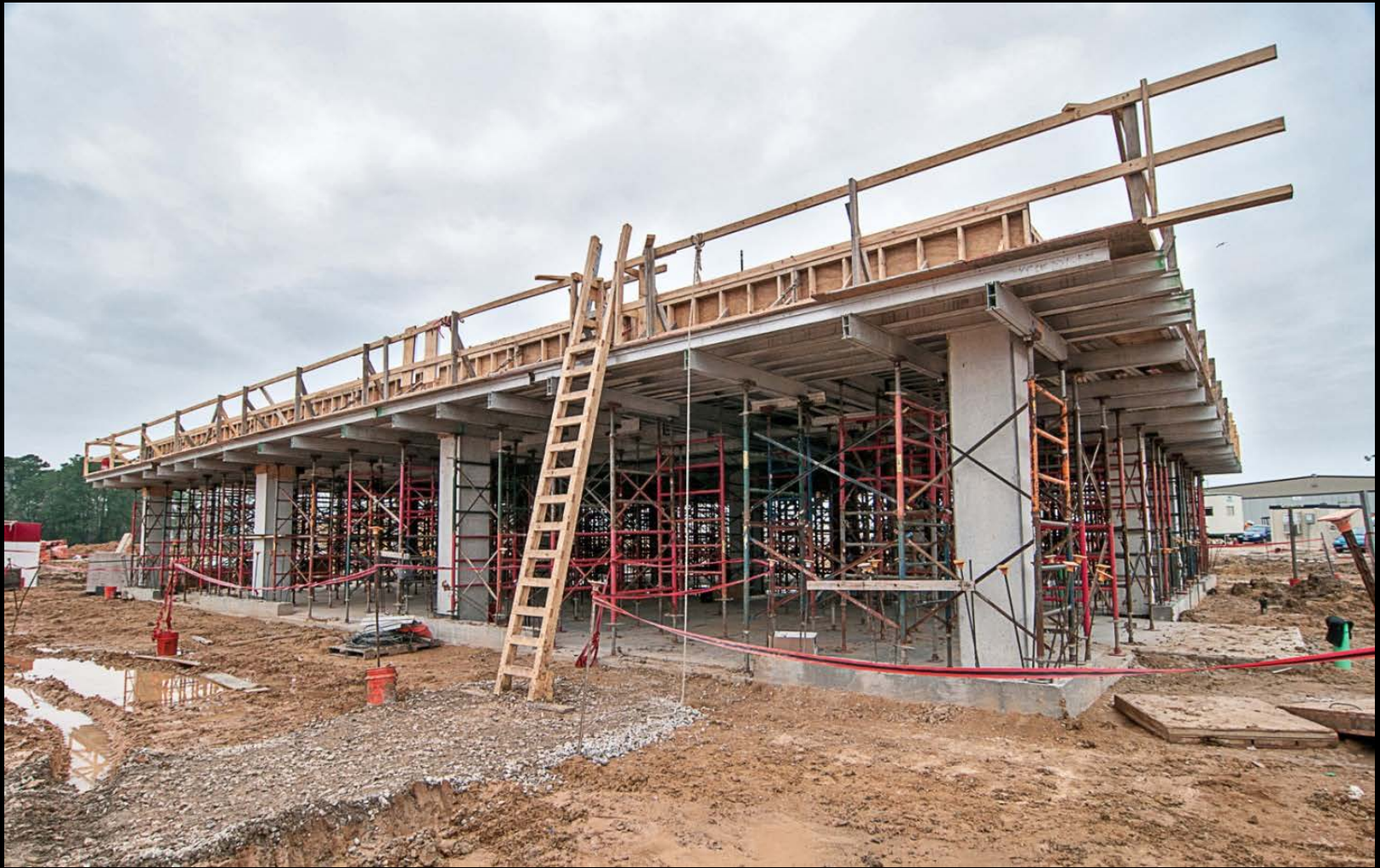
Dewatering Building – Previous progress photograph
