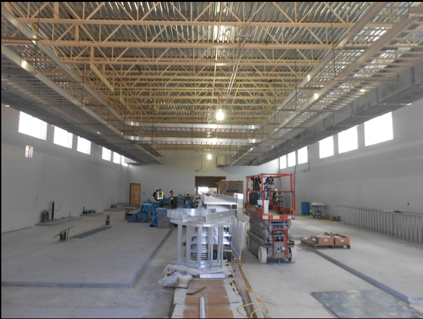
HSPS – Electrical room
