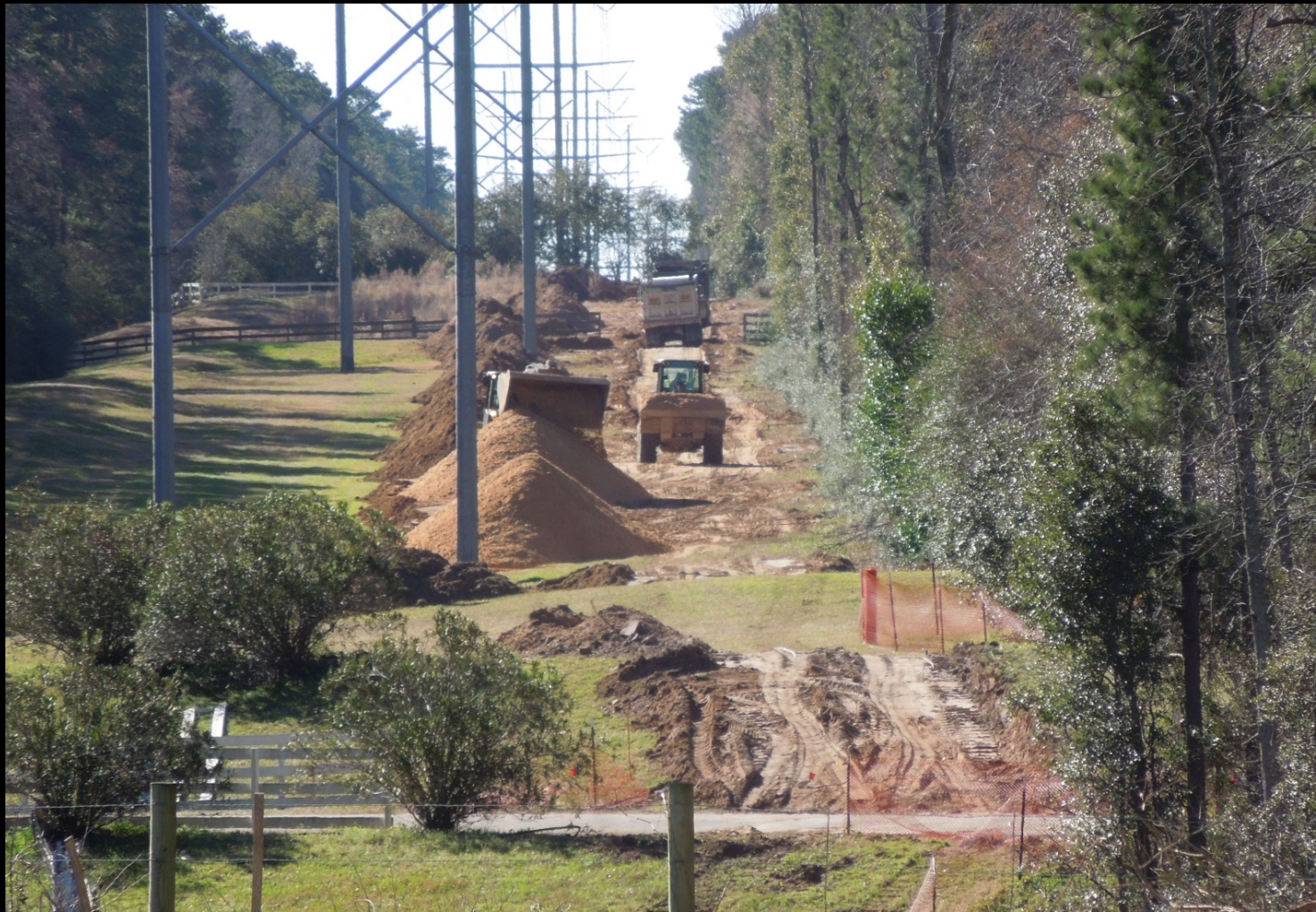
Pipe installation along Entergy easement
