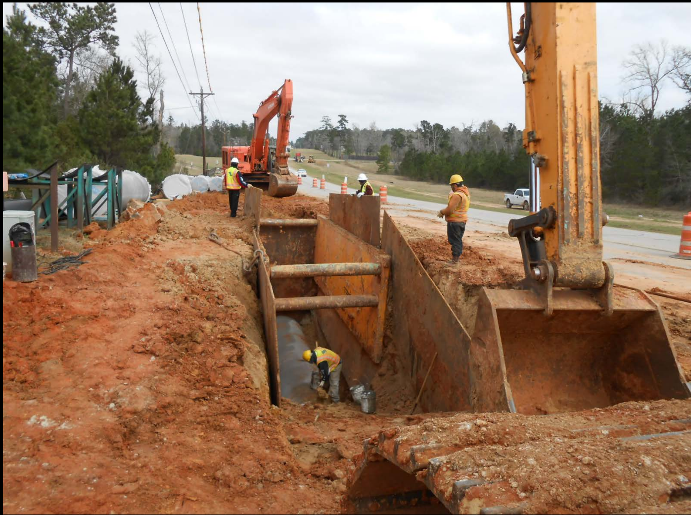
54 - inch pipe installation along Fish Creek Thoroughfare
