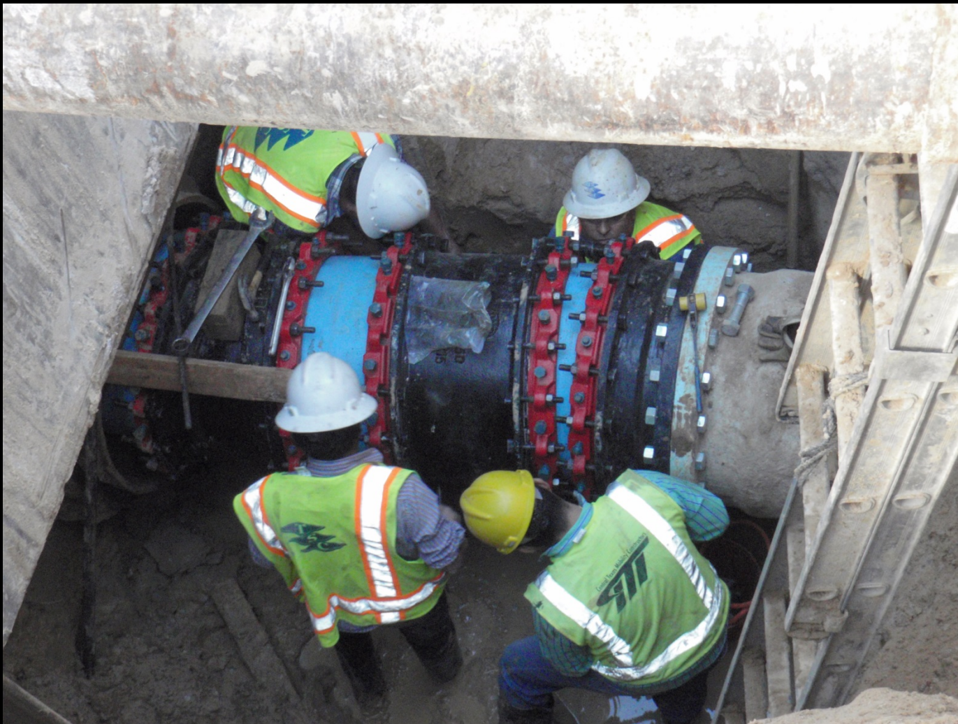
Restrained joint installation along Research Forest Drive
