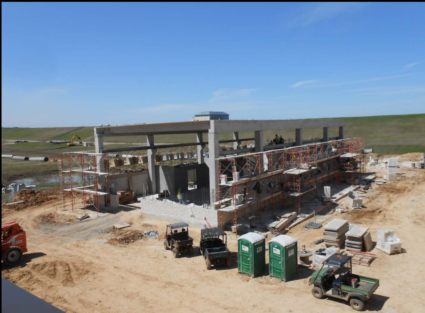
Blower Building – Masonry installation
