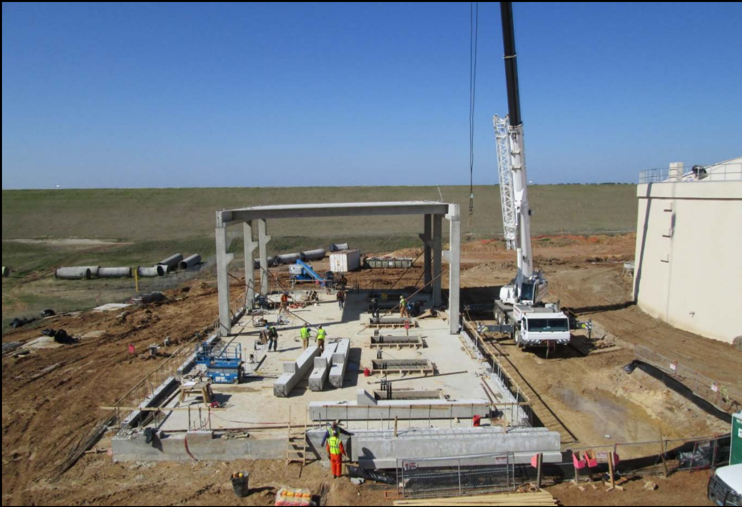
Blower Building – Previous progress photograph
