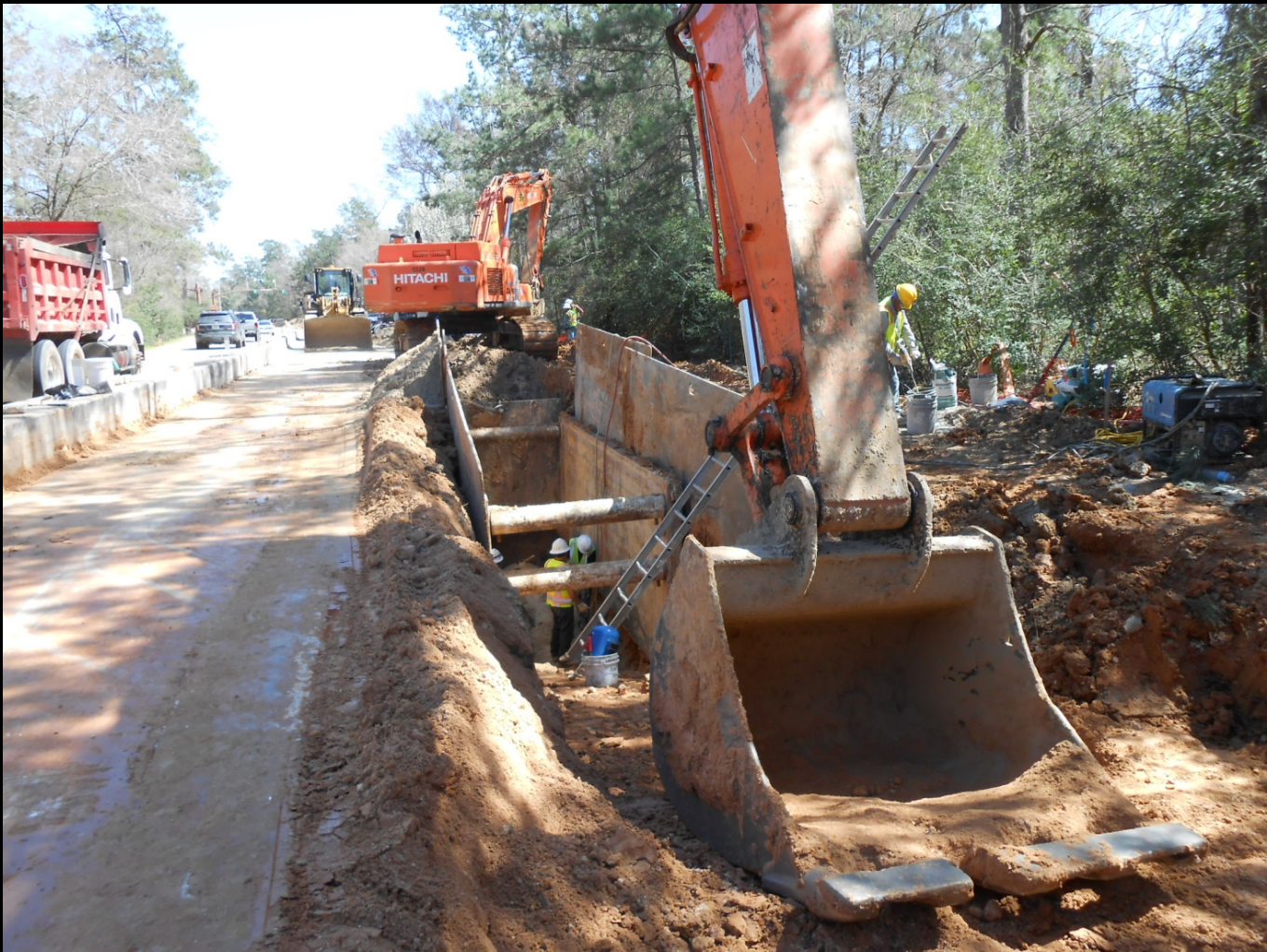
Open cut operation along Research Forest Drive
