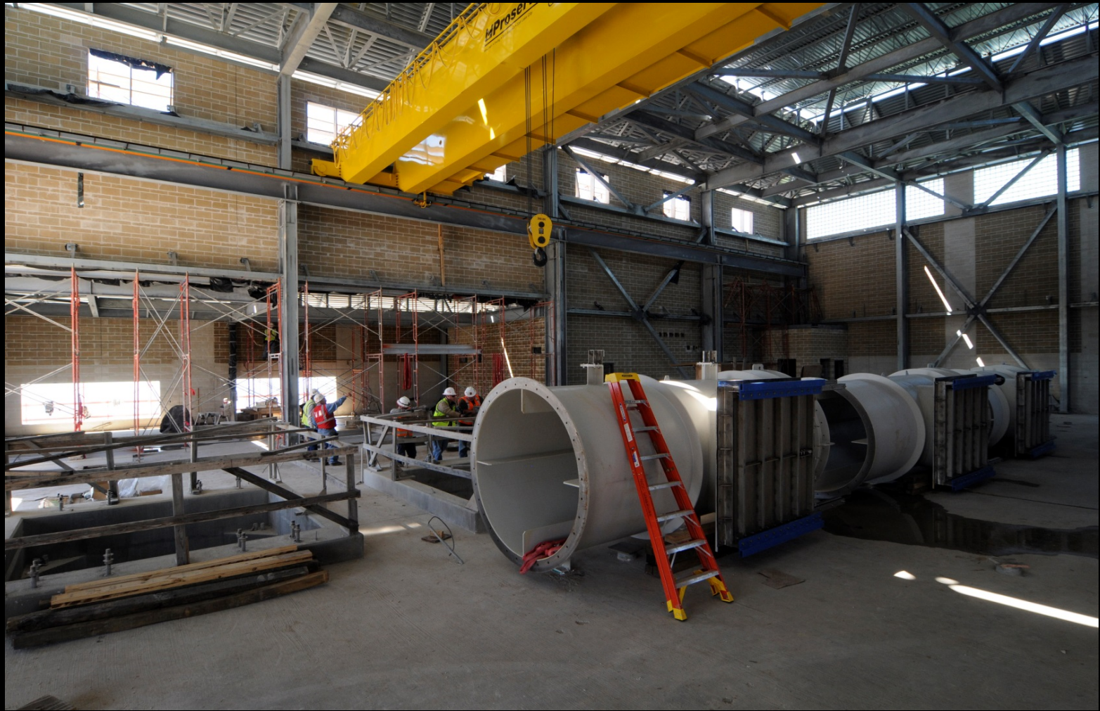
Interior view of masonry installation
