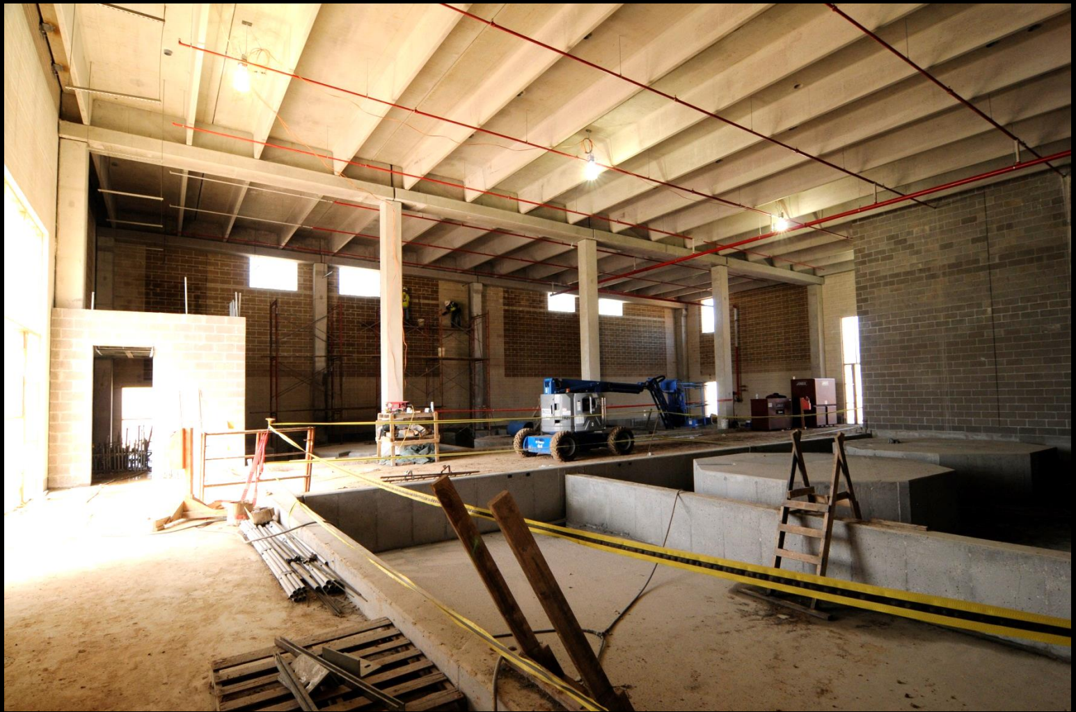
Interior view of fire suppression system
