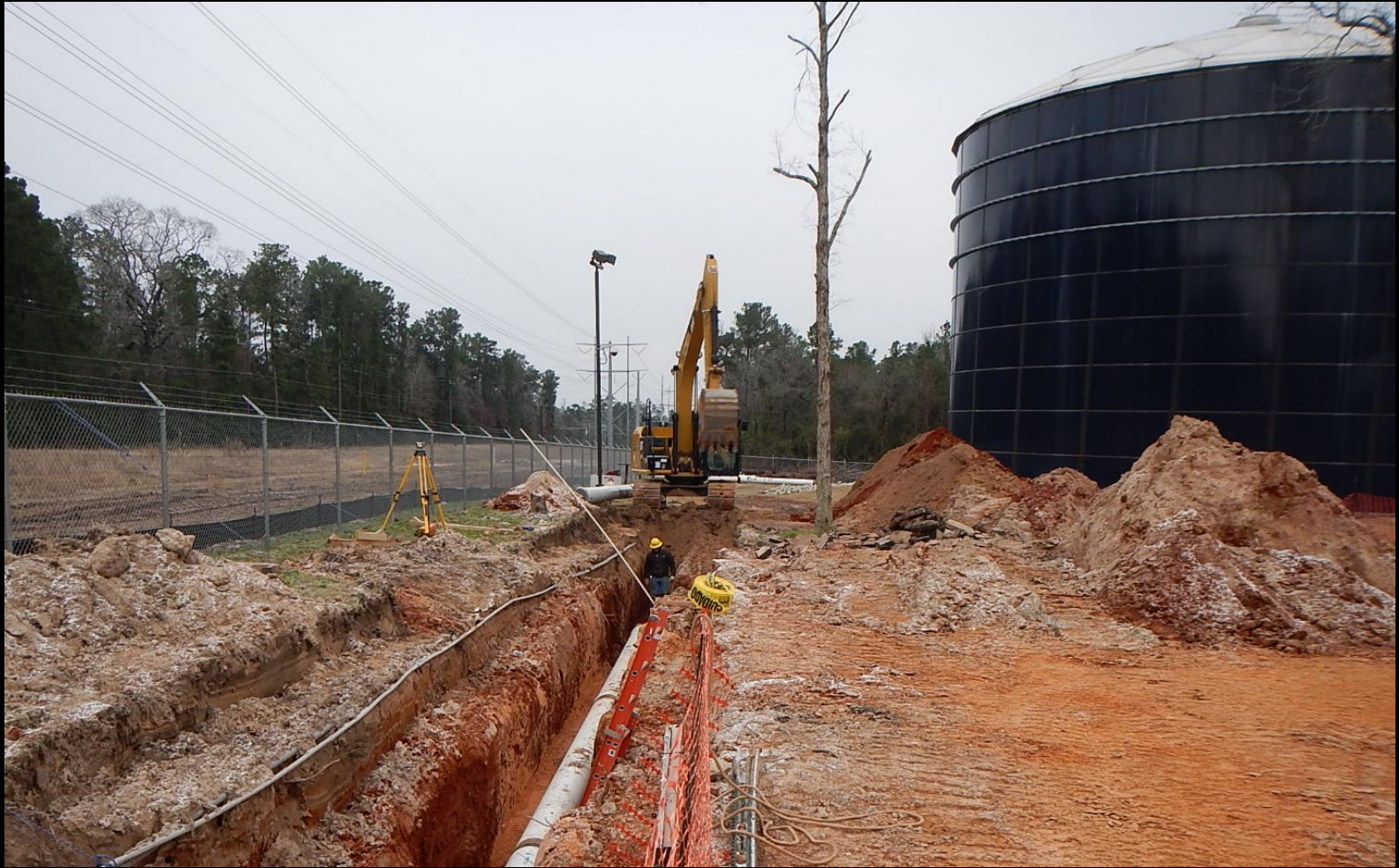
Yard piping installation at Conroe Water Plant No. 21
