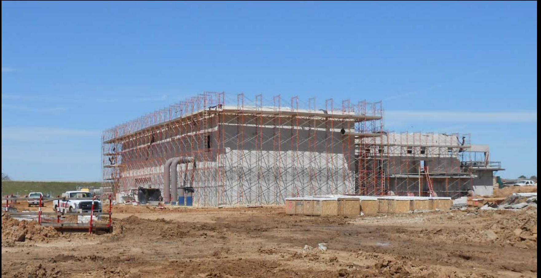
GAC – Exterior masonry installation
