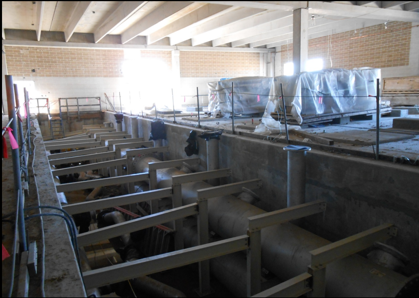
Membrane Building – Interior pipe trench
