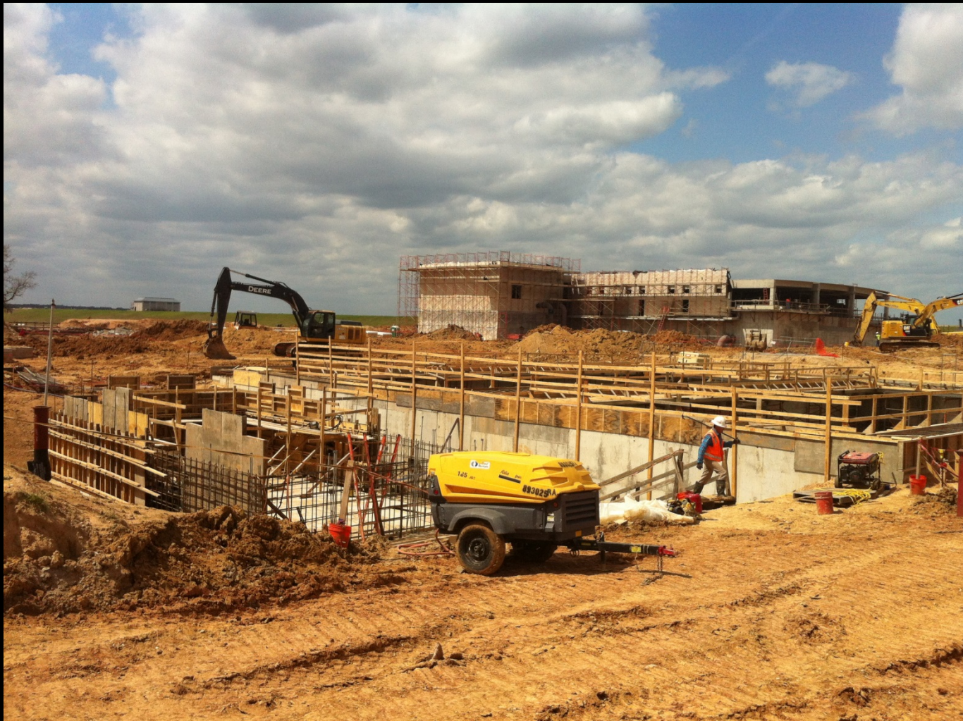
Backwash Equalization – Concrete Installation
