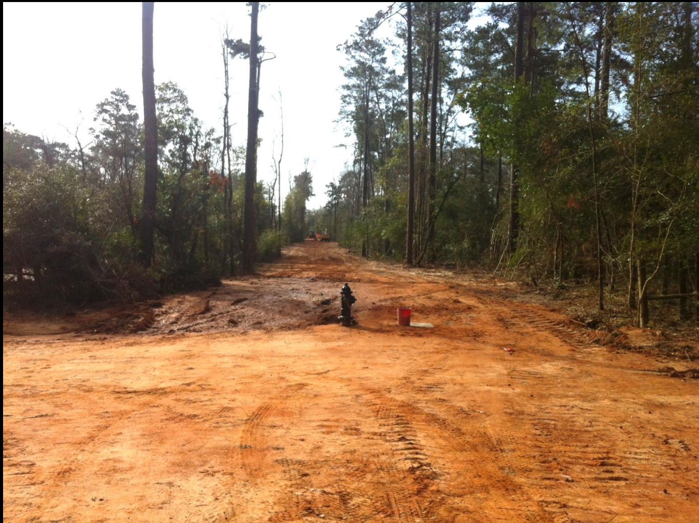
Site Restoration along Longmire Road
