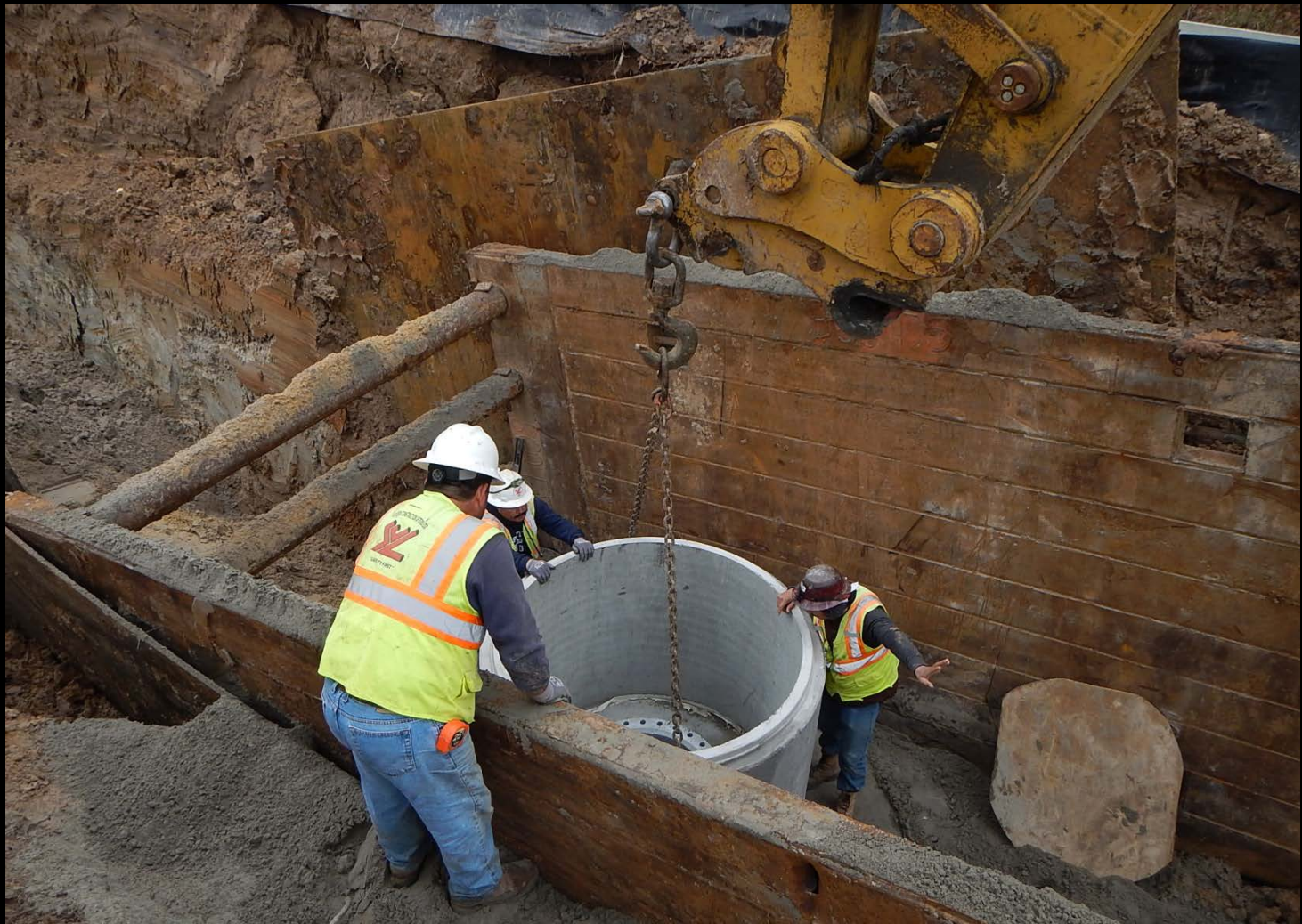
Manhole installation along McCaleb Road
