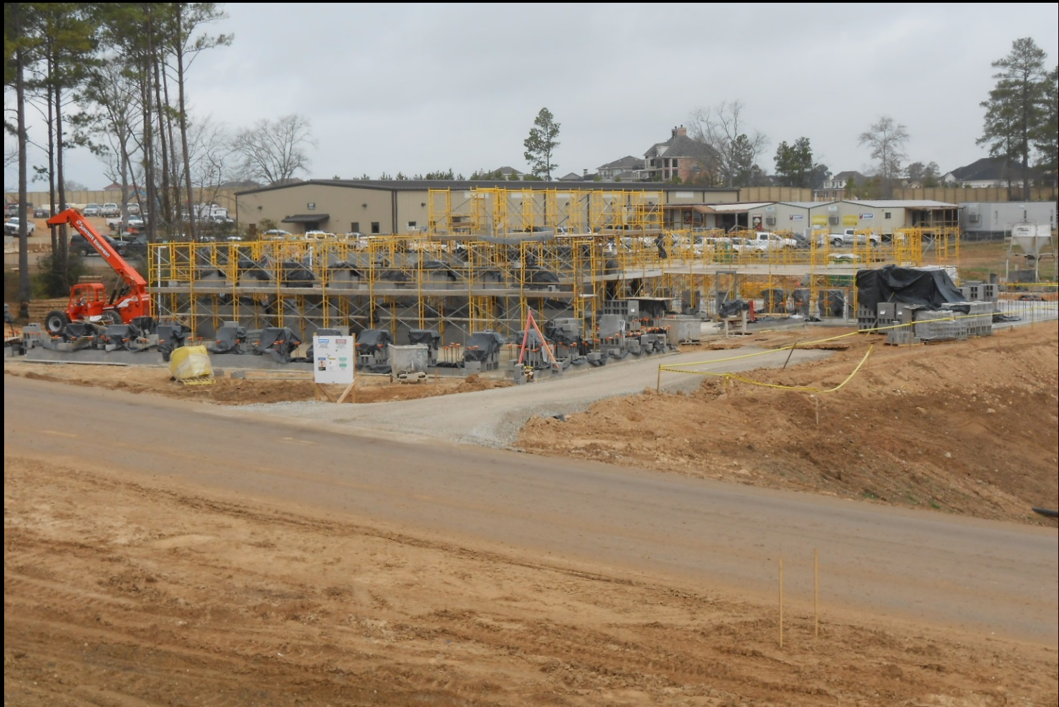
Previous progress photograph
