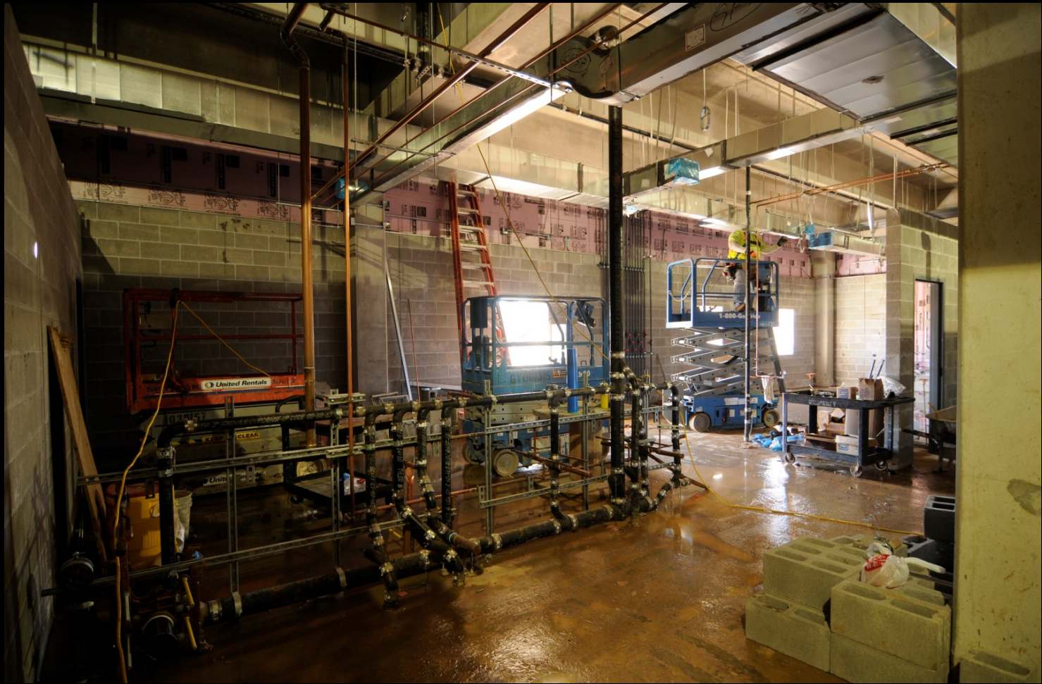
Membrane Building – Mechanical and Plumbing rough-in
