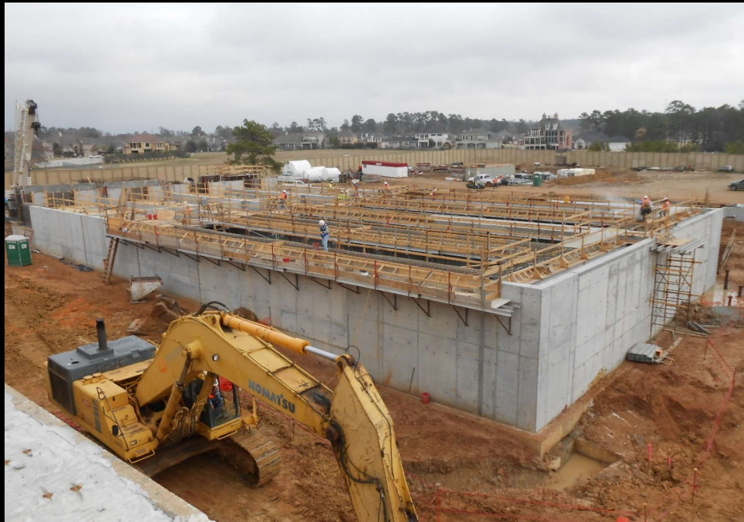
Pretreatment Facility– Previous progress photograph
