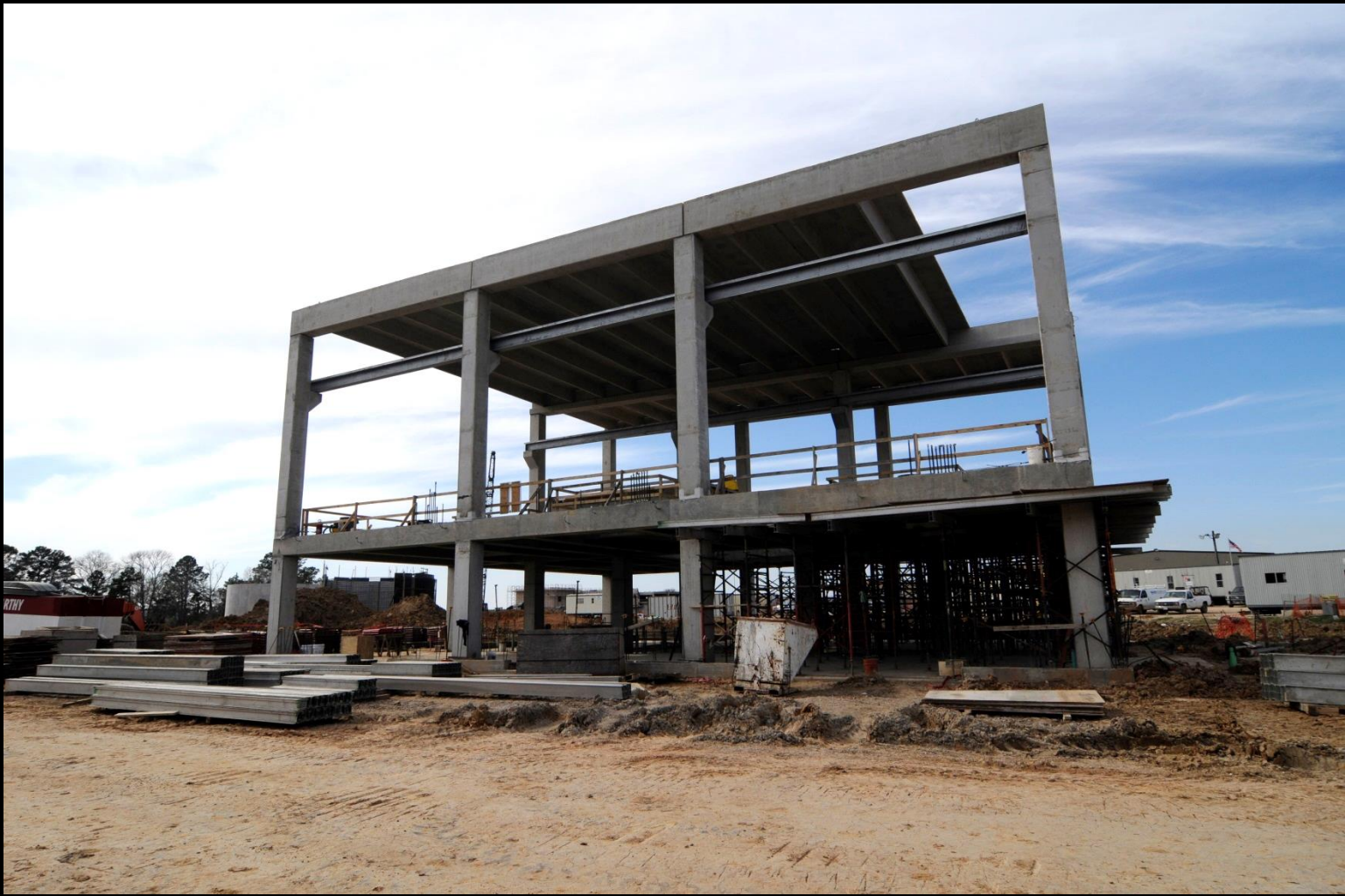
Dewatering Building – Second floor deck installation
