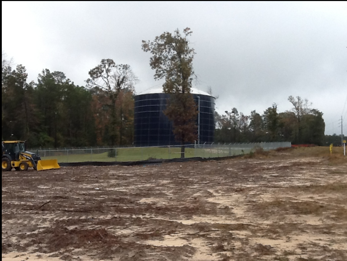
Cleared Standpipe site adjacent to Conroe WP 21
