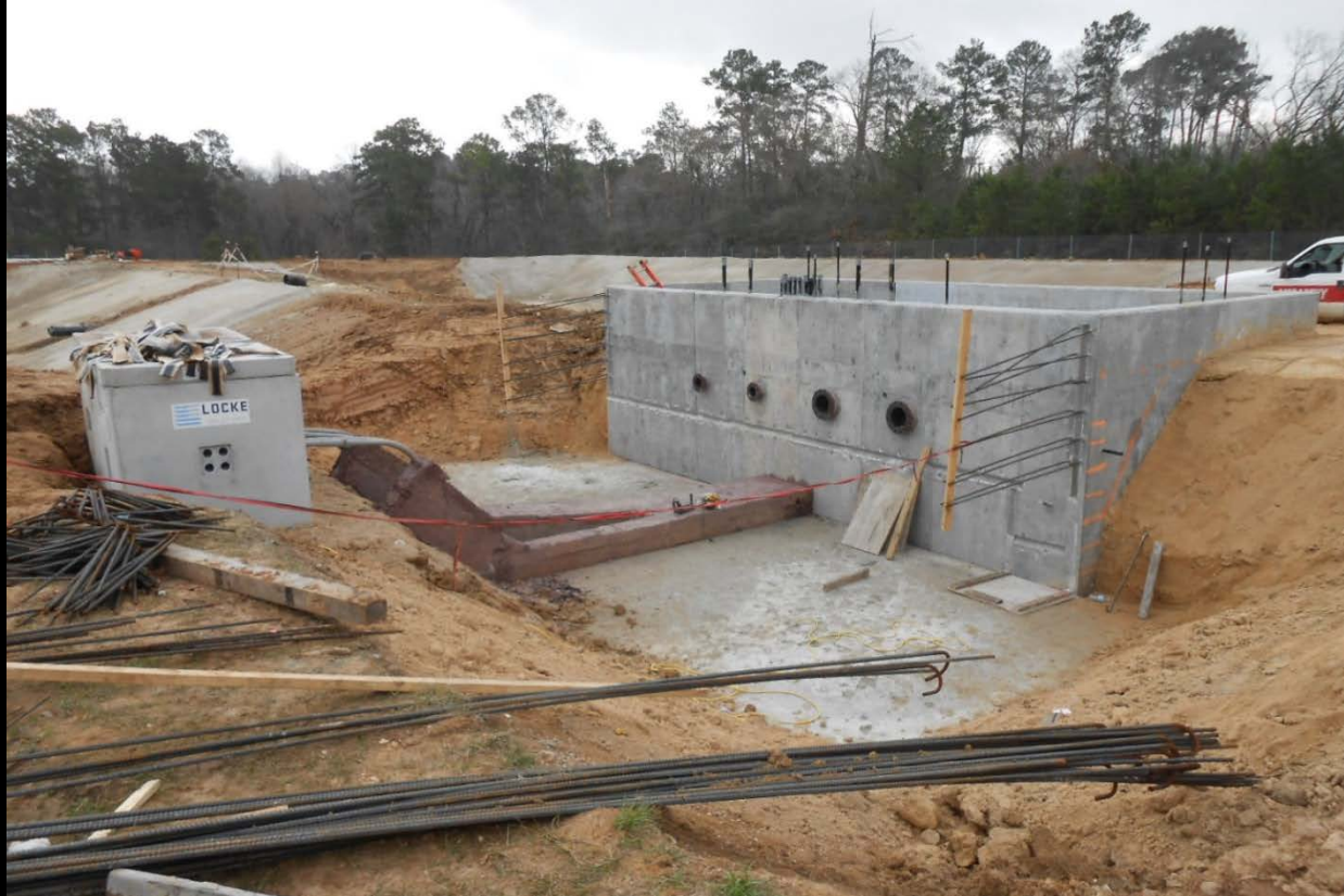
Water Recovery Basin Pump Station
