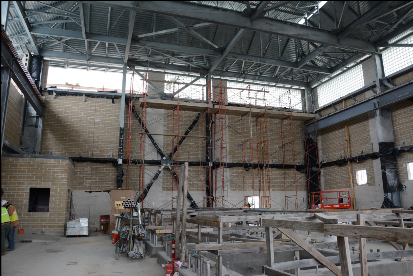
Interior view of masonry installation
