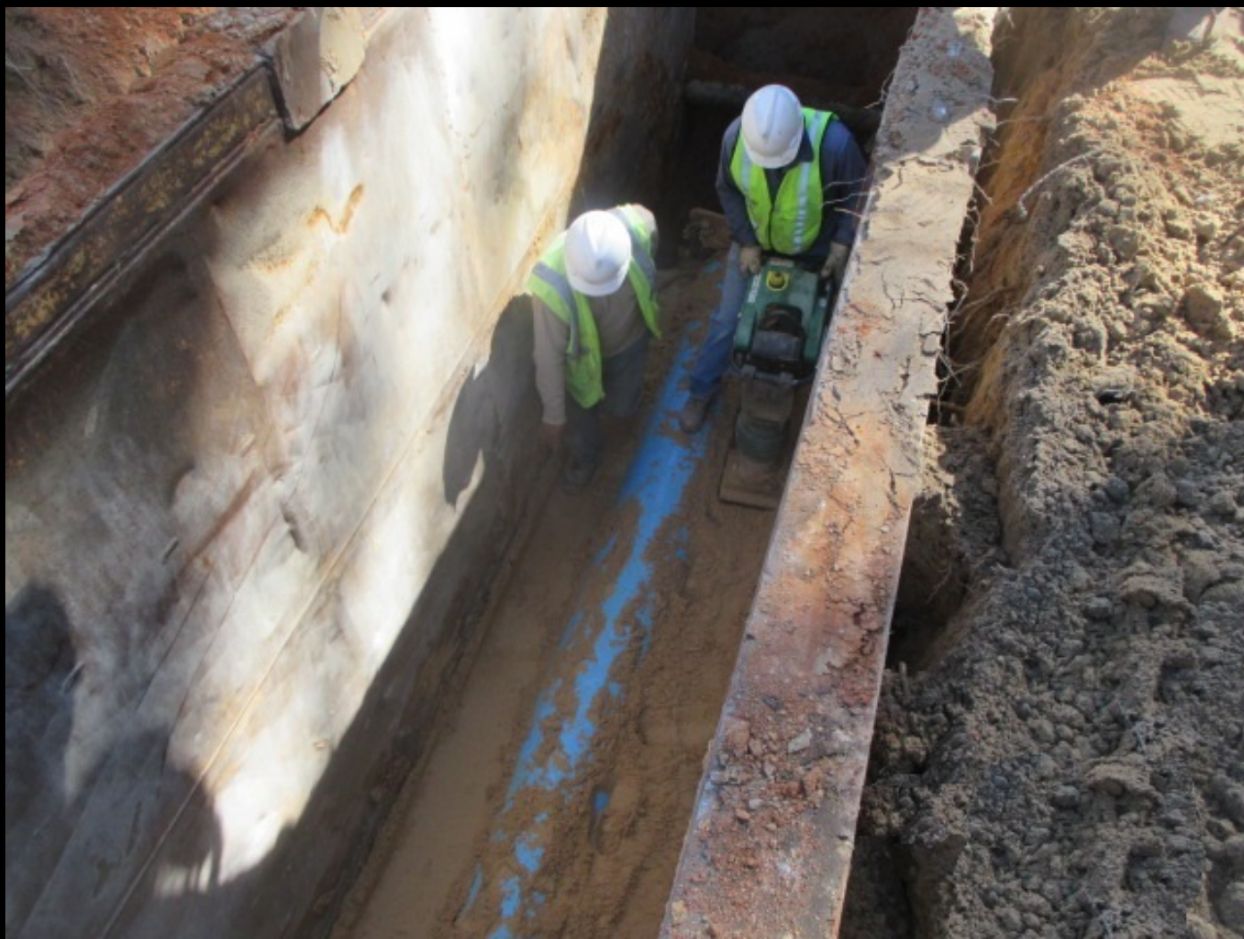
16 inch PVC pipe installation along Longmire Road
