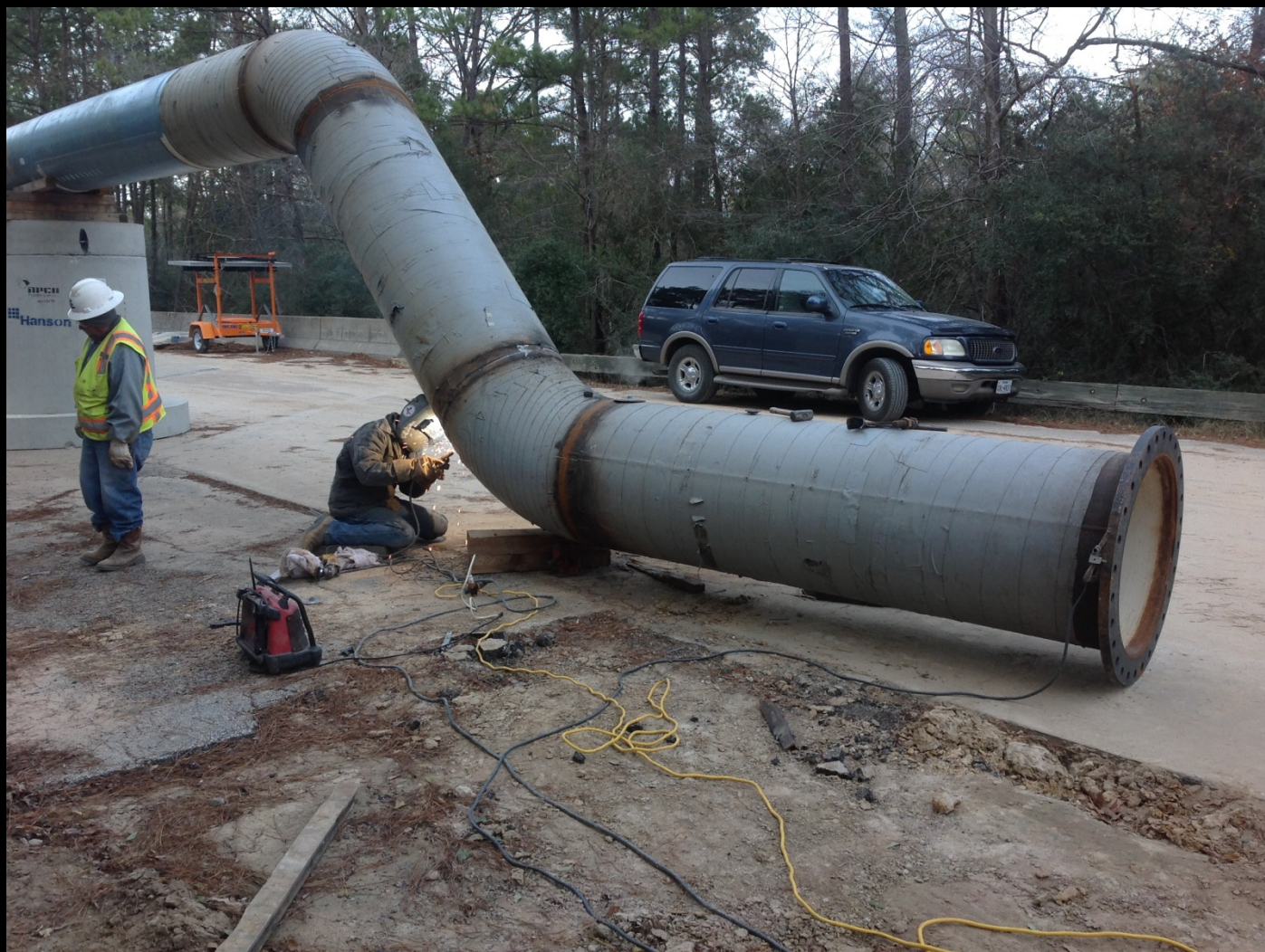
30 inch aerial pipe fabrication for Panther Branch crossing
