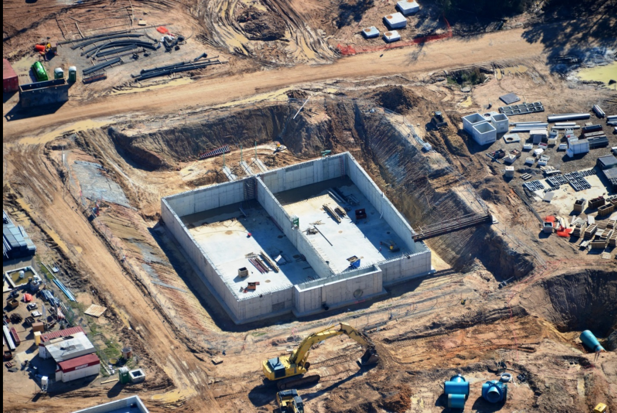
Previous progress photograph
