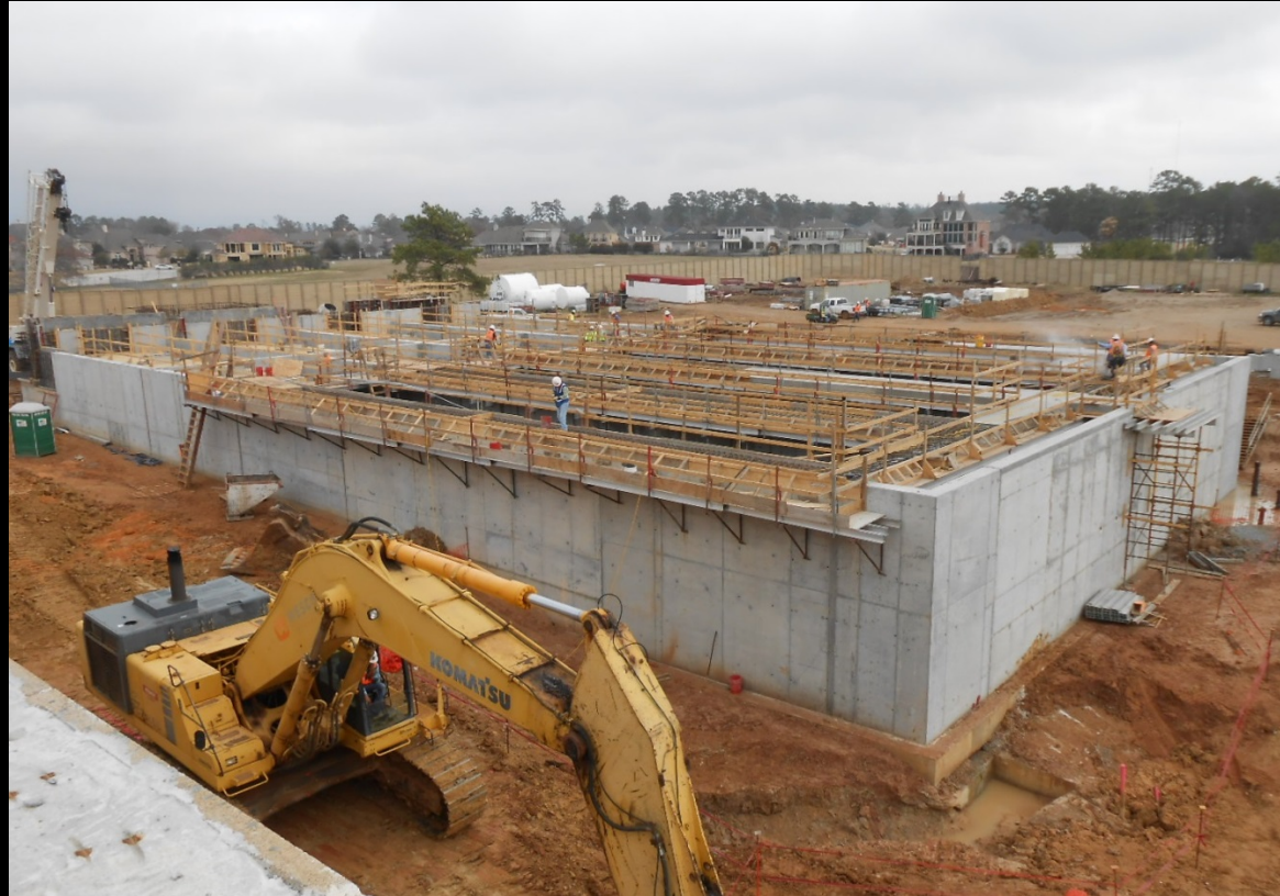
Pretreatment Facilities – Elevated walkway construction
