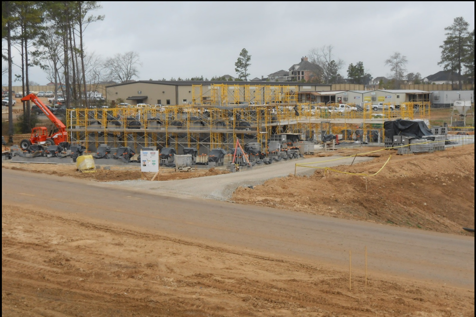
Masonry installation in progress
