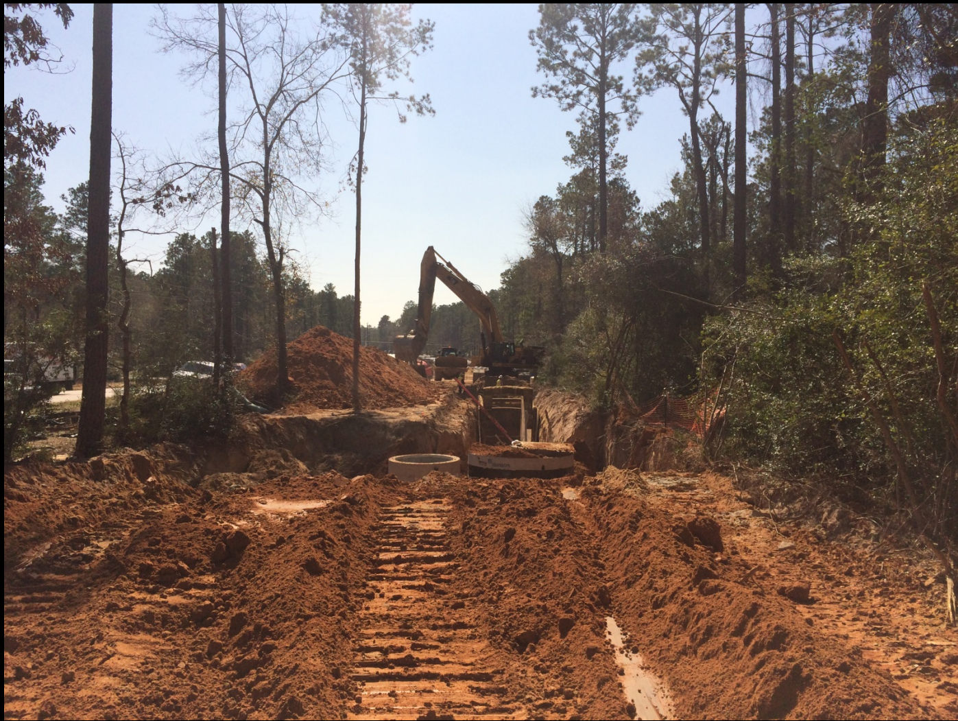
54 inch pipe installation along Fish Creek Thoroughfare
