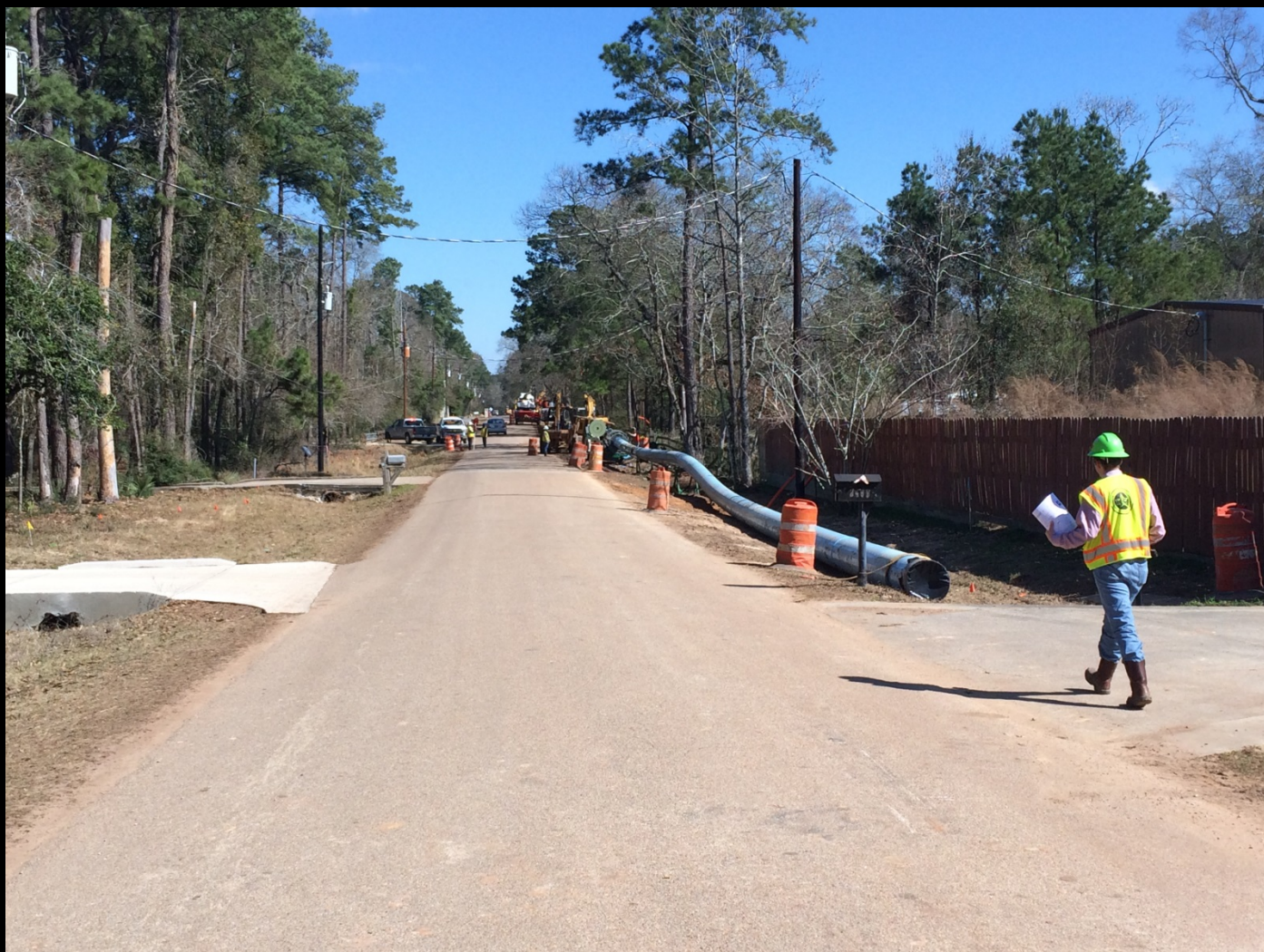
PVC pipe fusing operation along Southline Road
