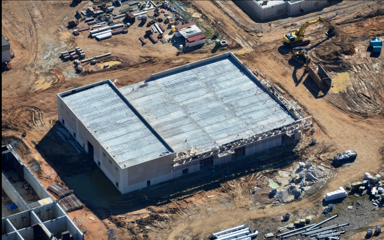
Membrane Building – Previous progress photograph
