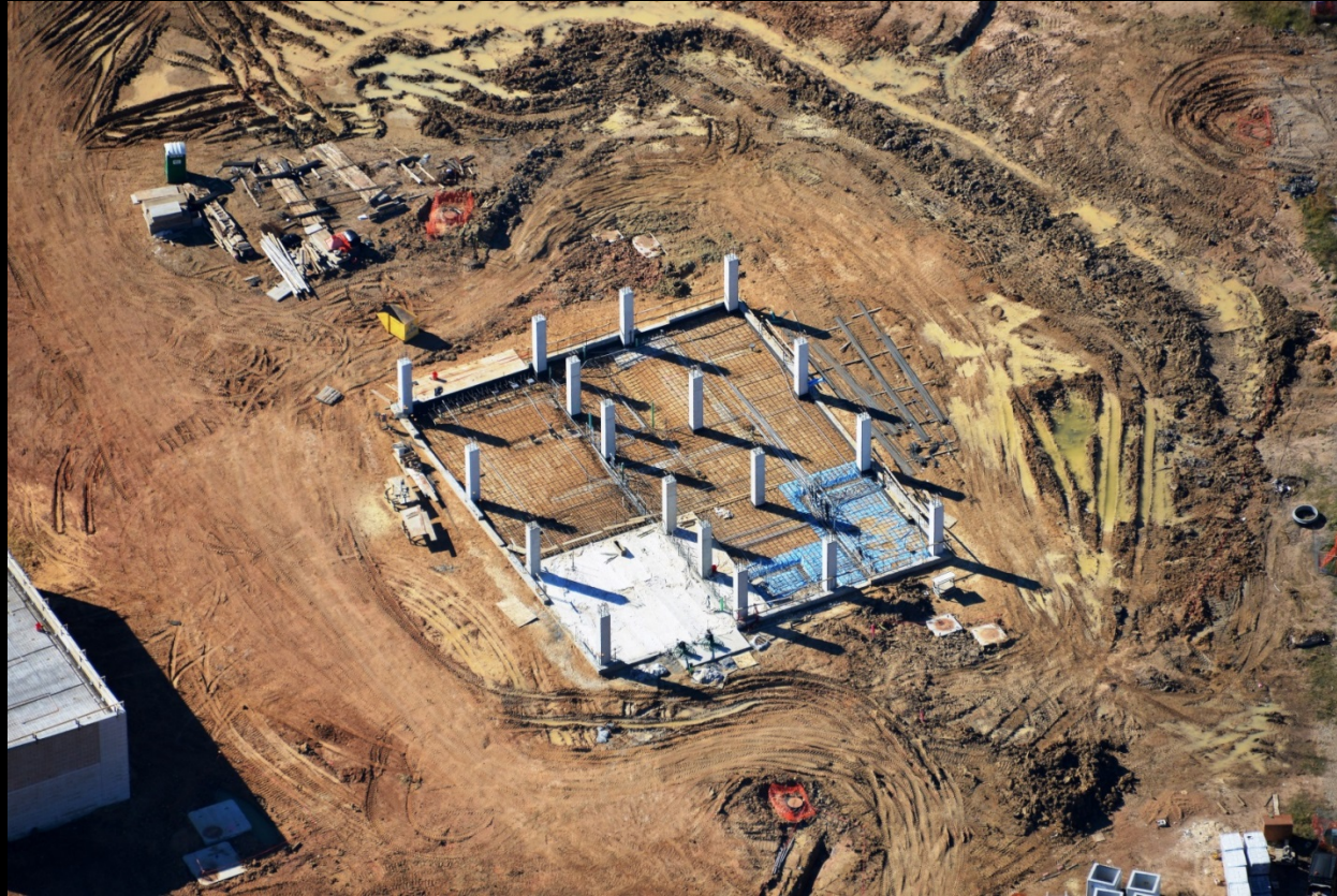
Dewatering Building – Previous progress photograph
