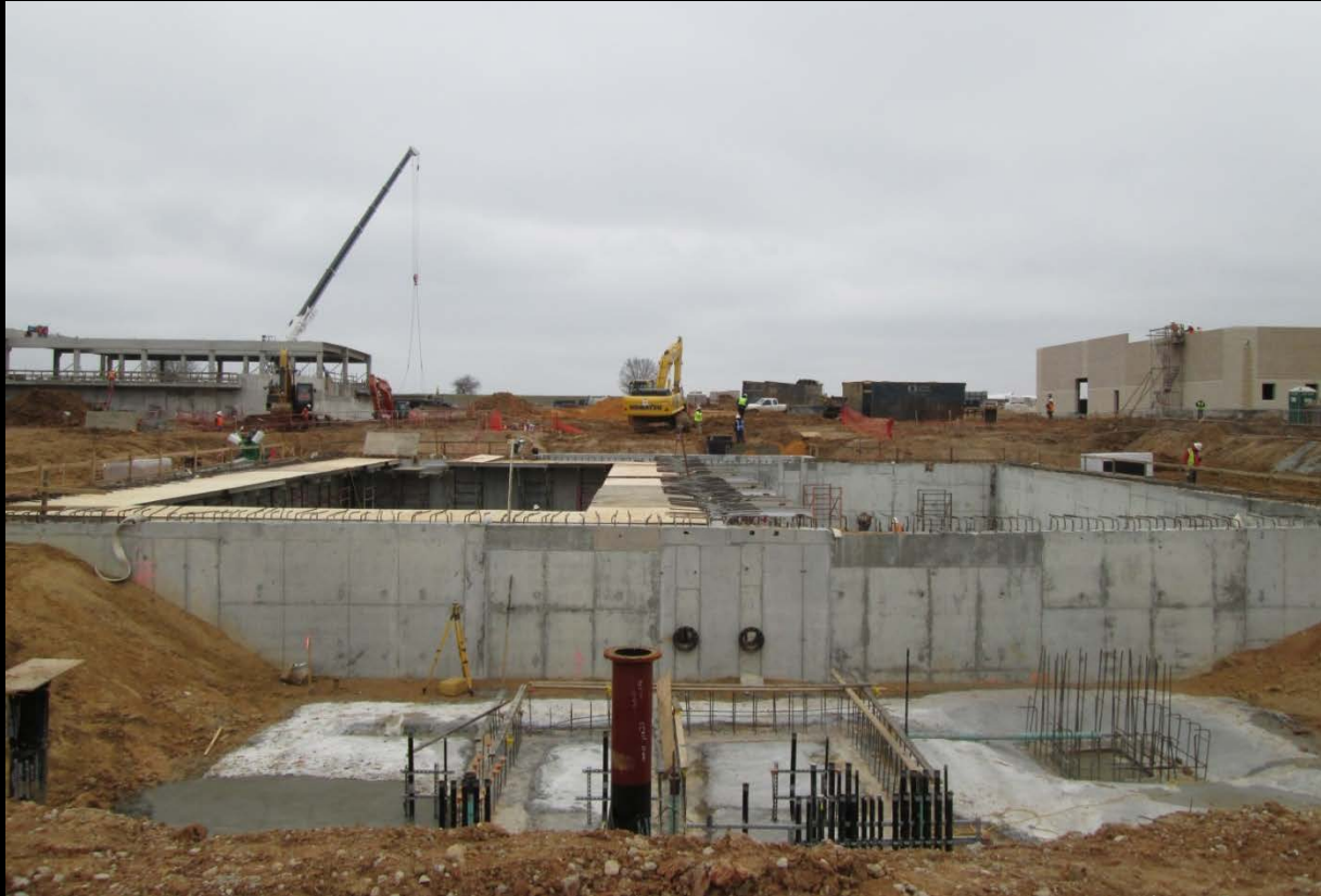
Backwash Equalization Pump Room Foundation
