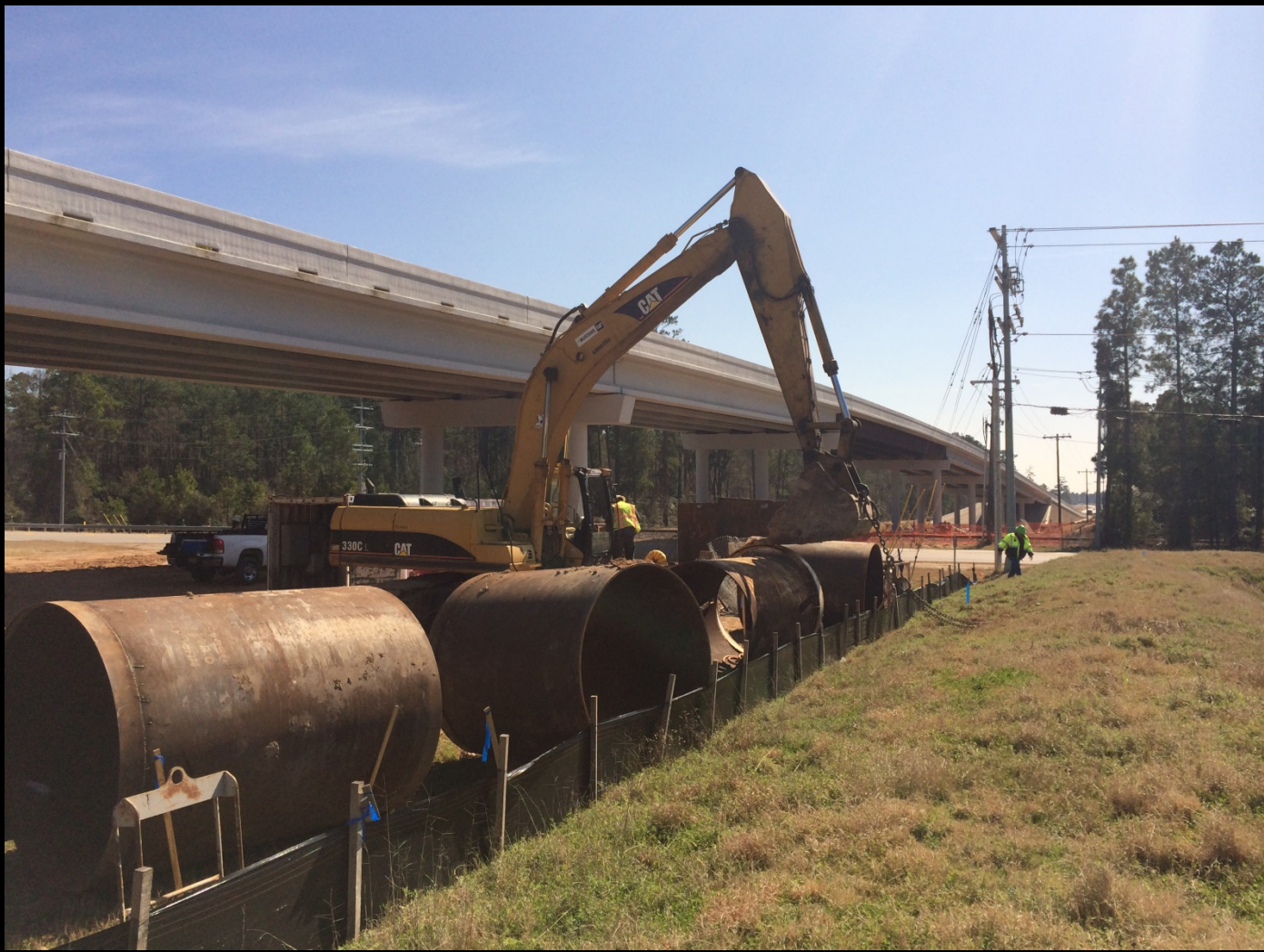
Tunnel operation for FM 2854 and BNSF Railroad crossing
