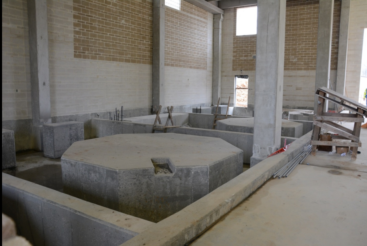
Interior view of chemical storage basin pedestals
