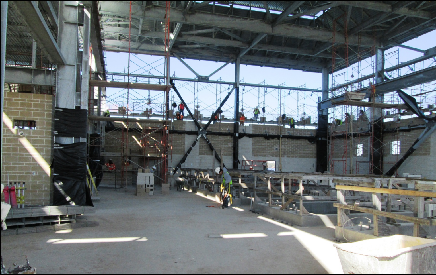
Previous progress photograph
