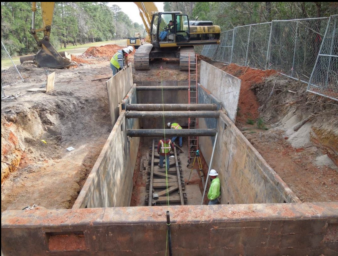
Tunnel operation for 16 inch pipe crossing Longmire Road
