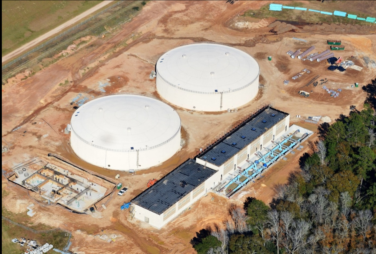
Previous progress photograph
