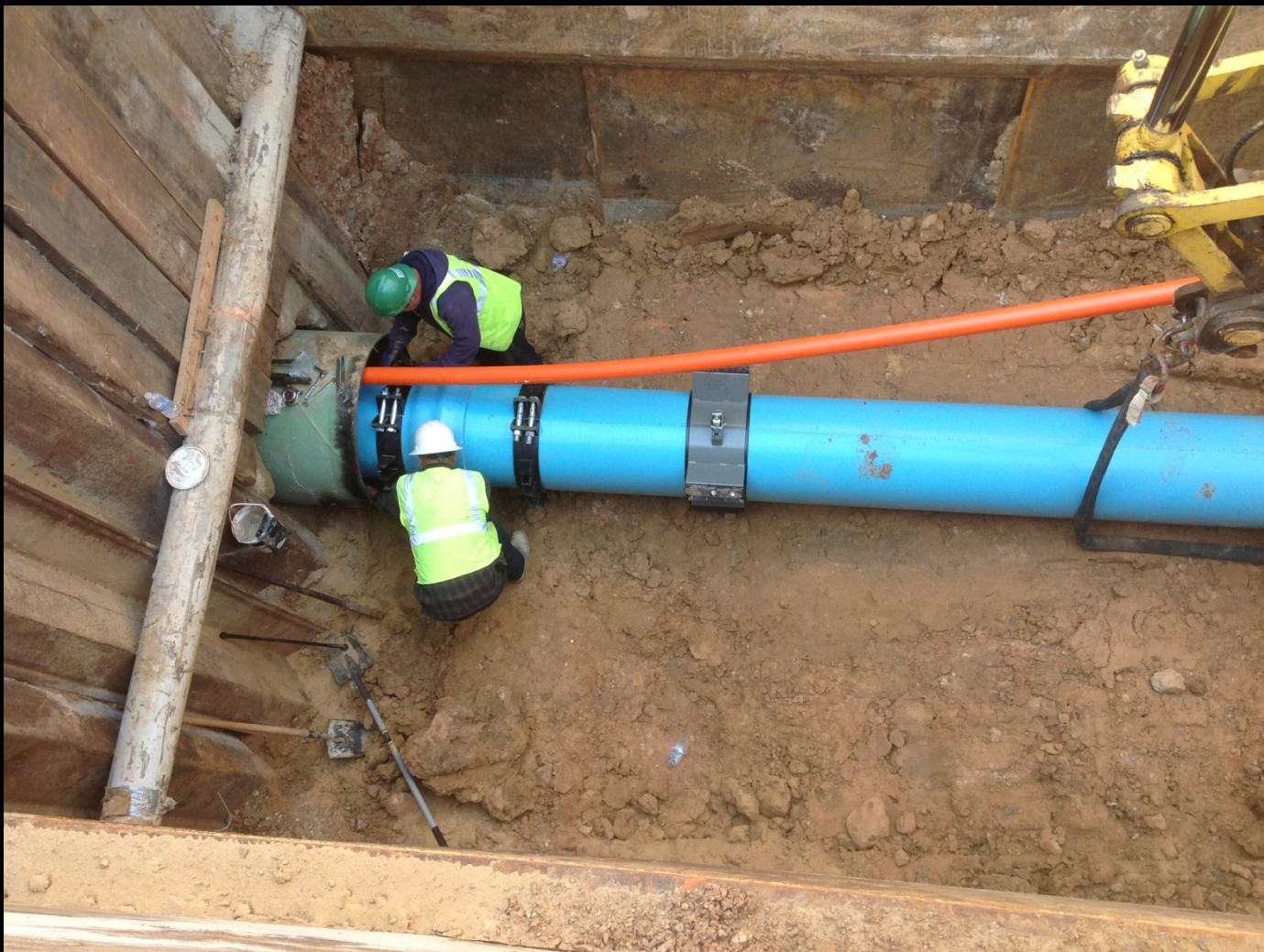
Fiber optic conduit installation at Tom Stinson Drive and Pollok Drive
