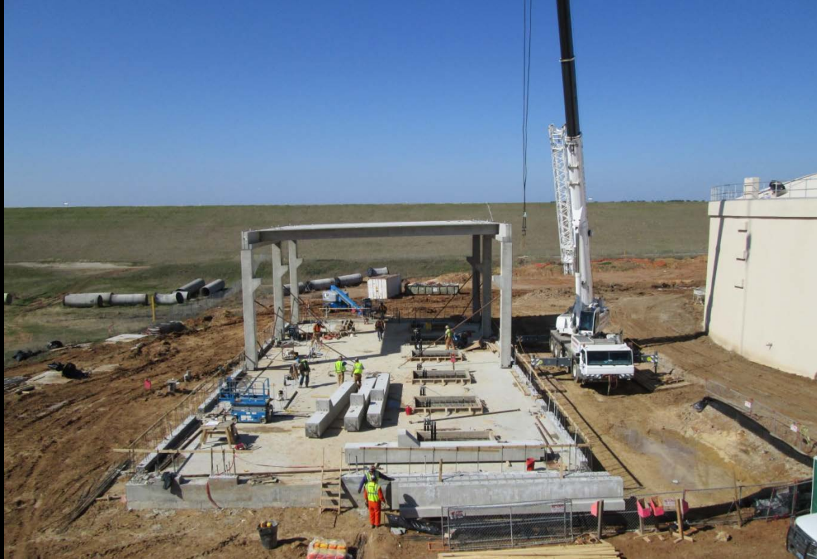
Blower Building – Precast structure installation
