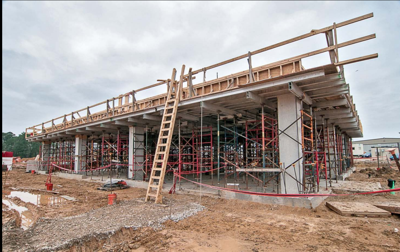
Dewatering Building – Second floor deck installation
