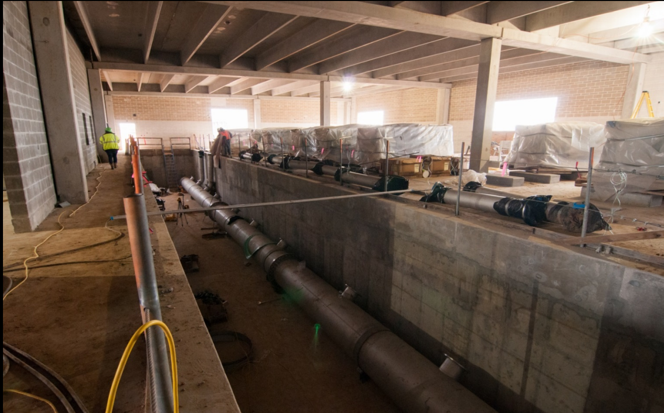
Membrane Building – Interior pipe trench
