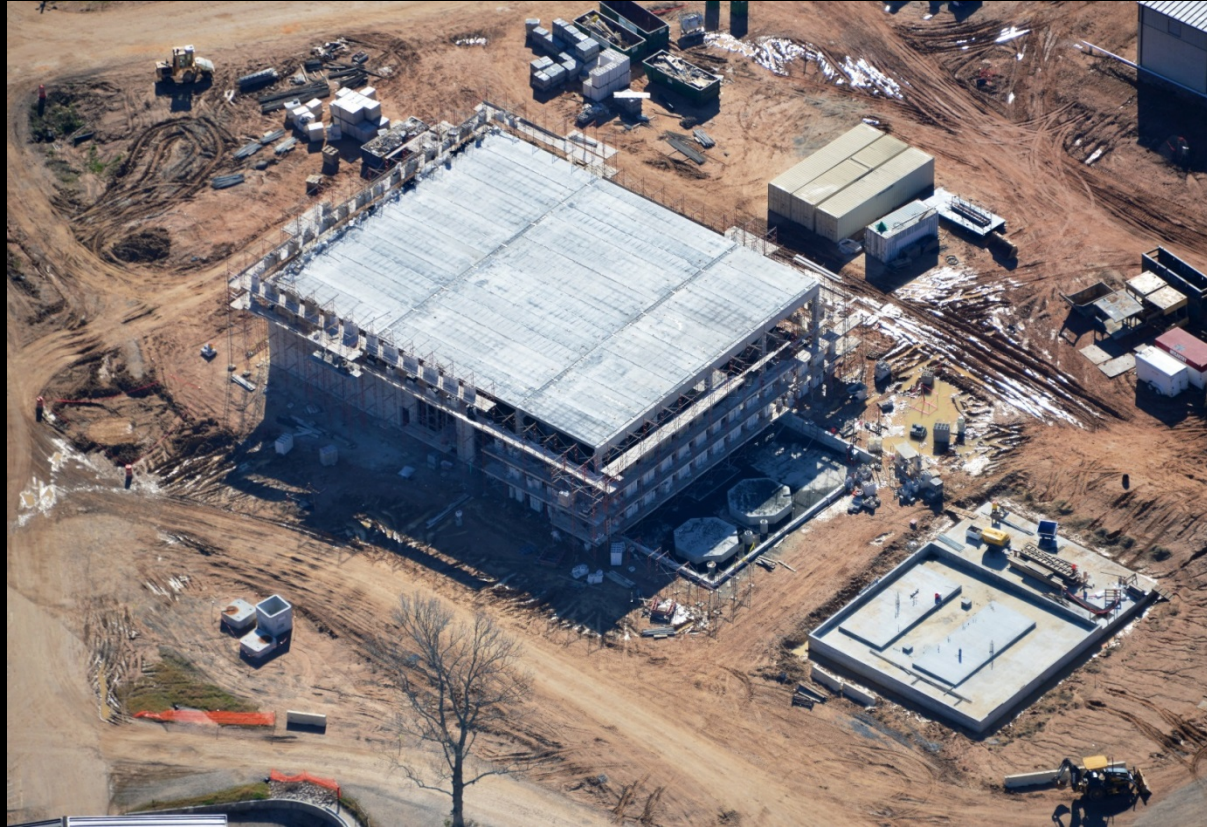
Previous progress photograph
