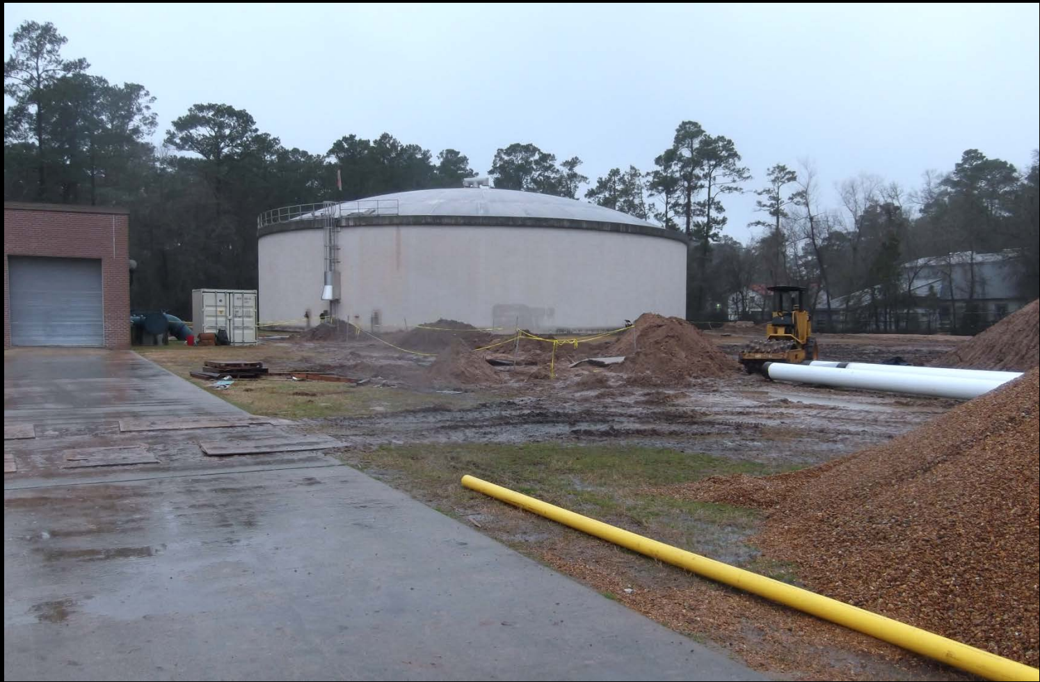
Yard piping installation at SJRA Water Plant No. 3
