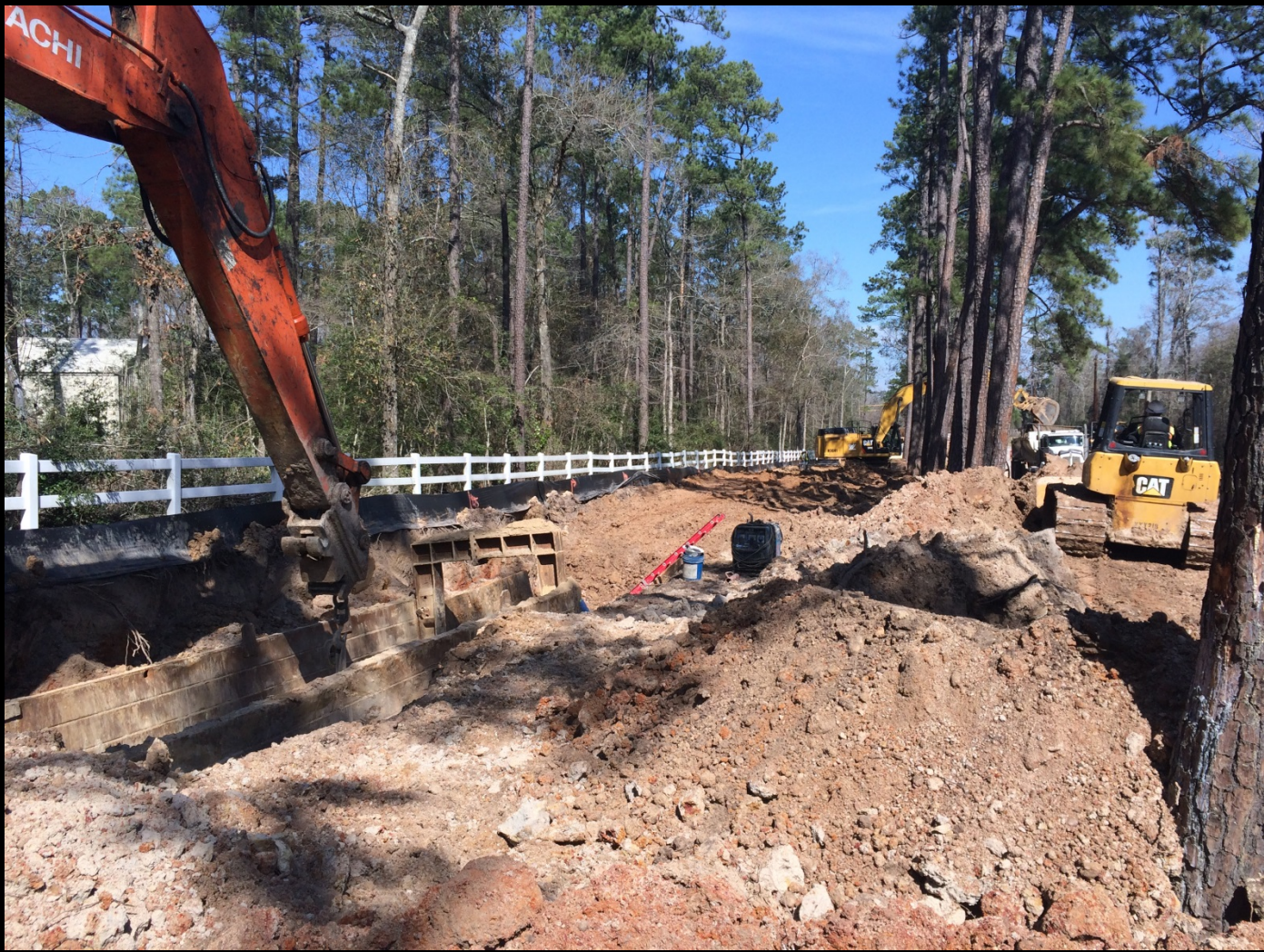
60 inch pipe installation along McCaleb Road
