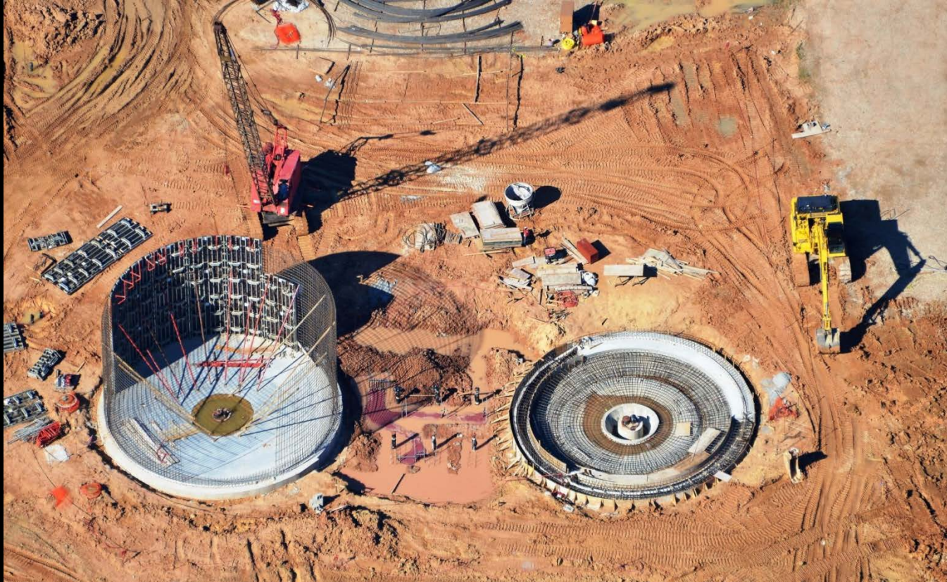
Thickeners – Previous progress photograph
