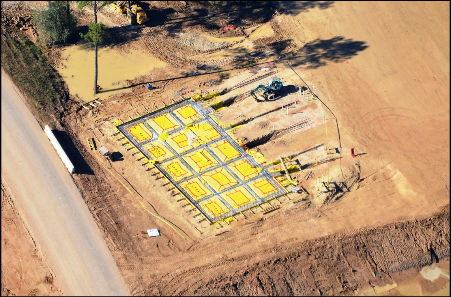
Previous progress photograph
