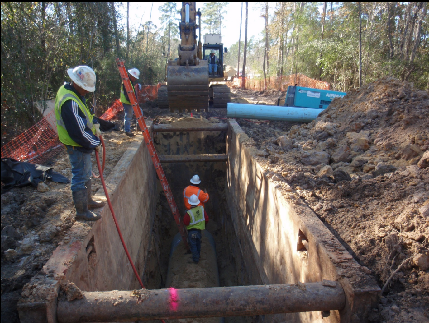
48 inch pipe installation along future Research Forest Drive
