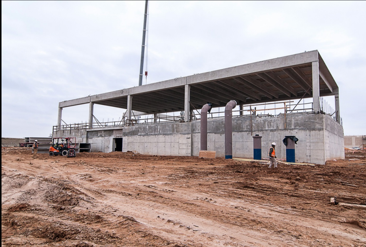
GAC – Exterior view from west
