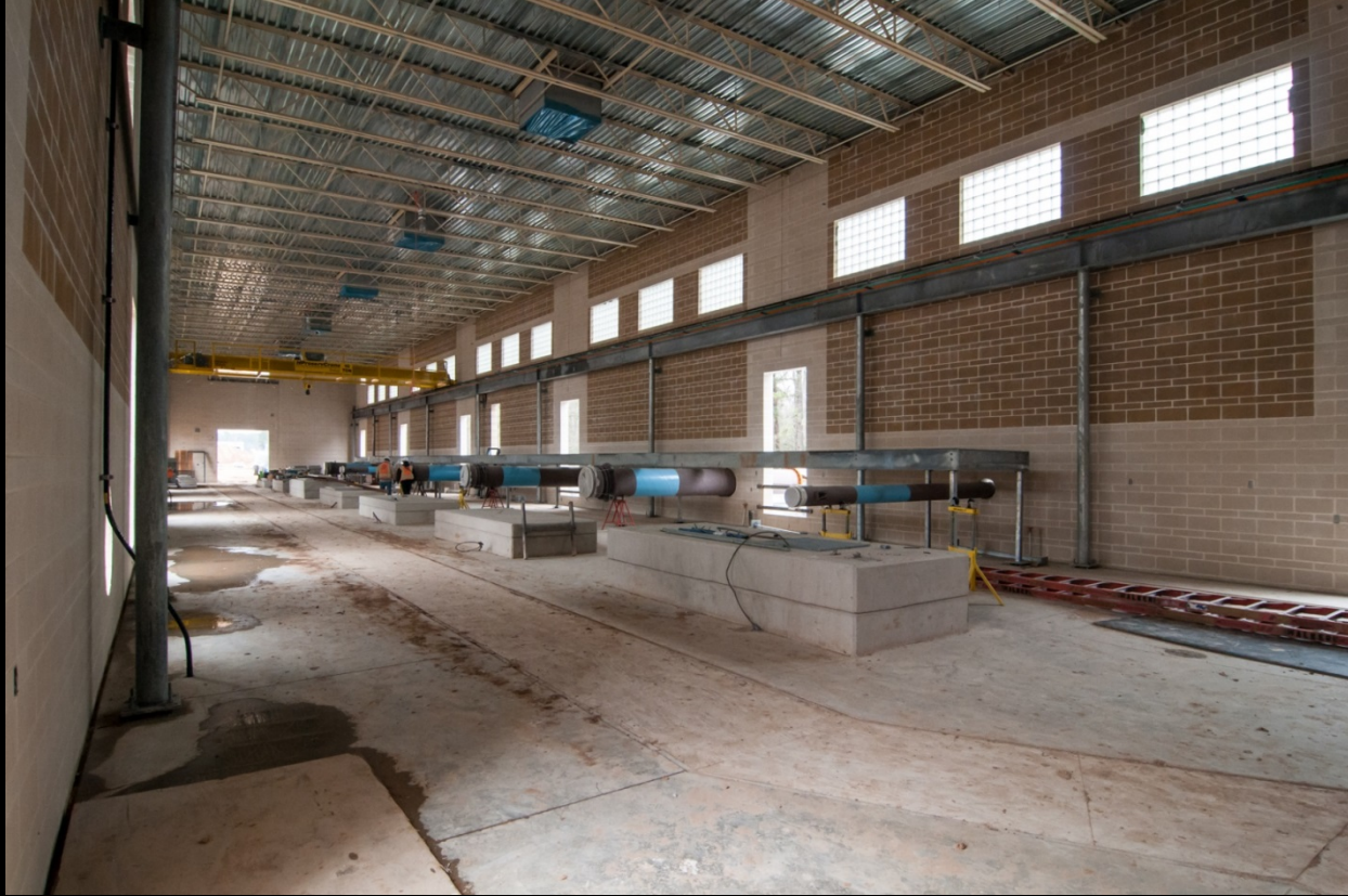
HSPS – Pump room
