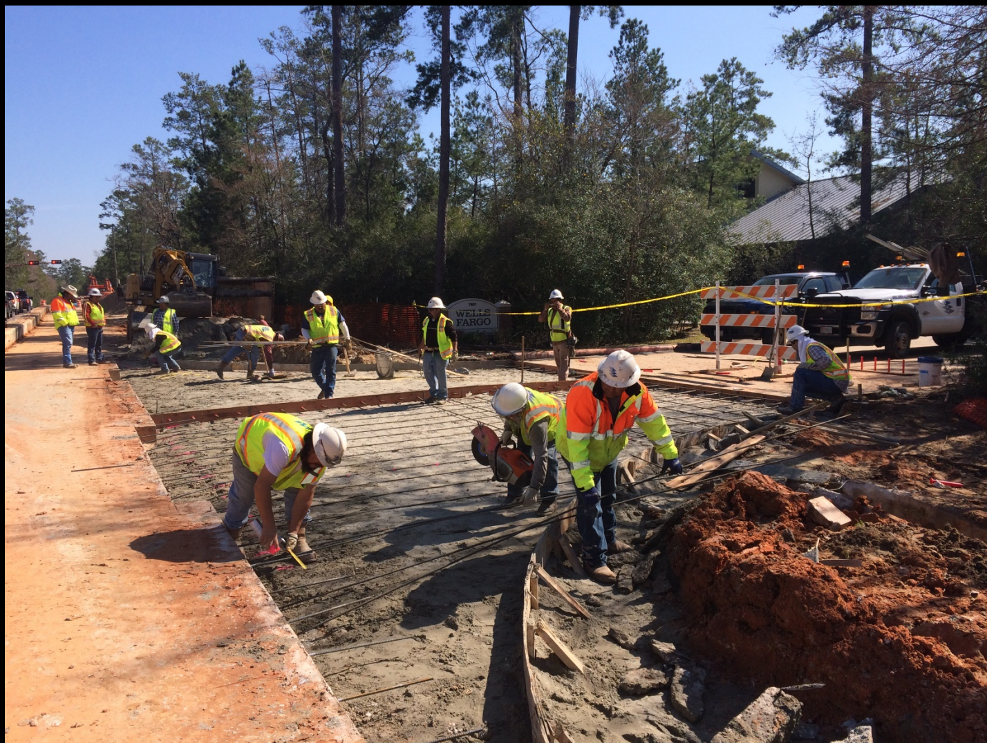
Concrete pavement replacement along Research Forest Drive near Kuykendahl Road
