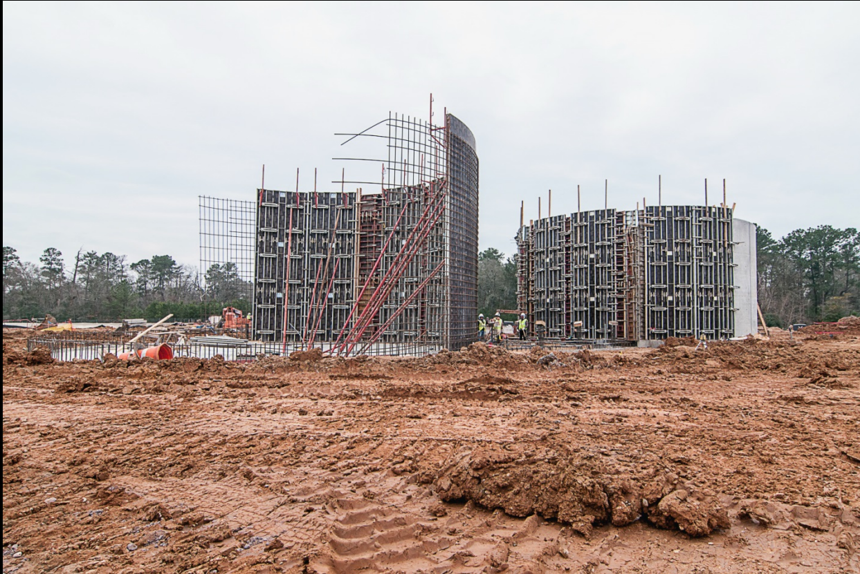
Thickeners – Wall construction
