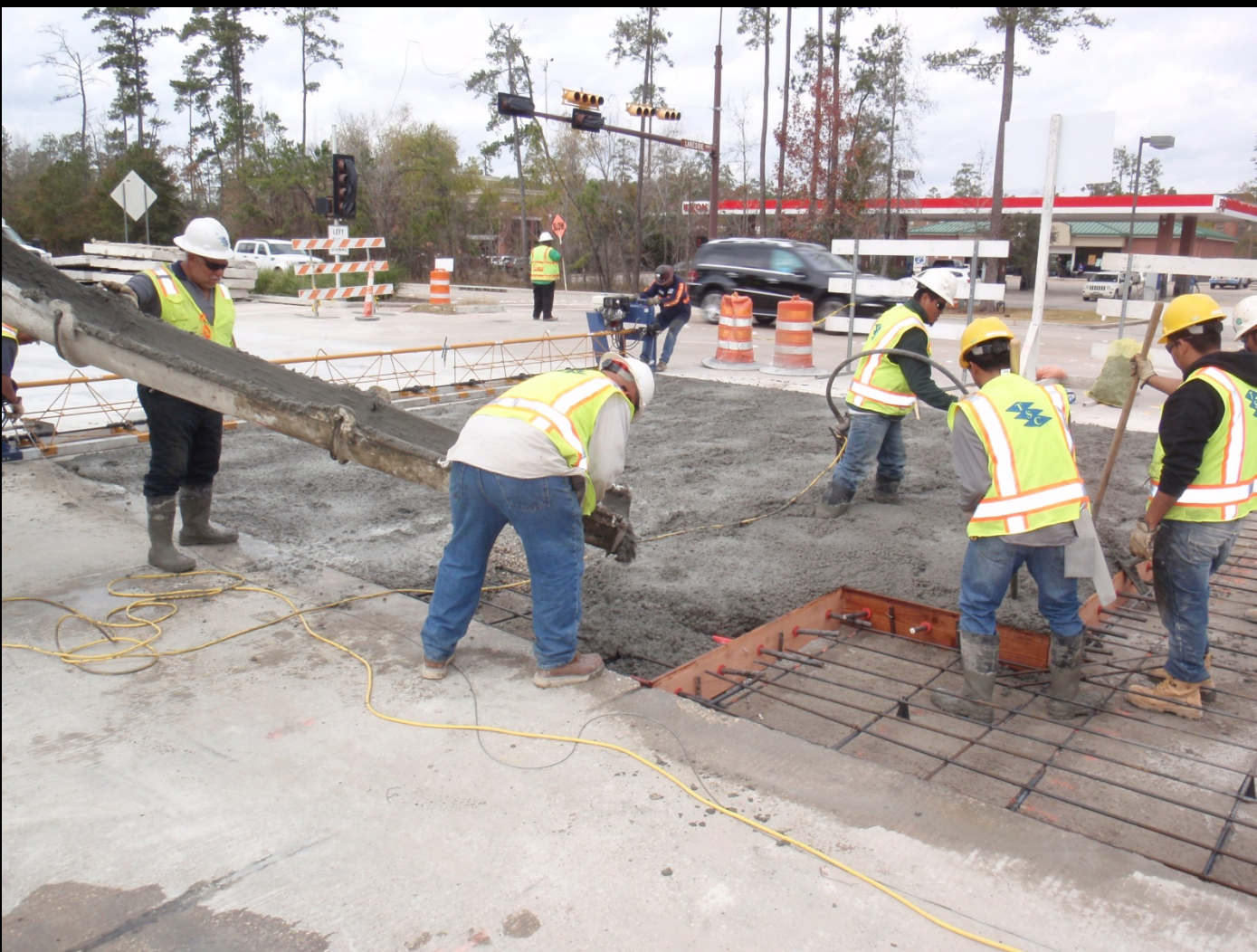
Concrete pavement placement at Research Forest Drive and Lakeside Boulevard
