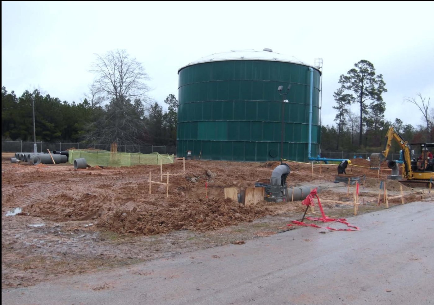
Yard piping installation at City of Conroe Water Plant No. 20
