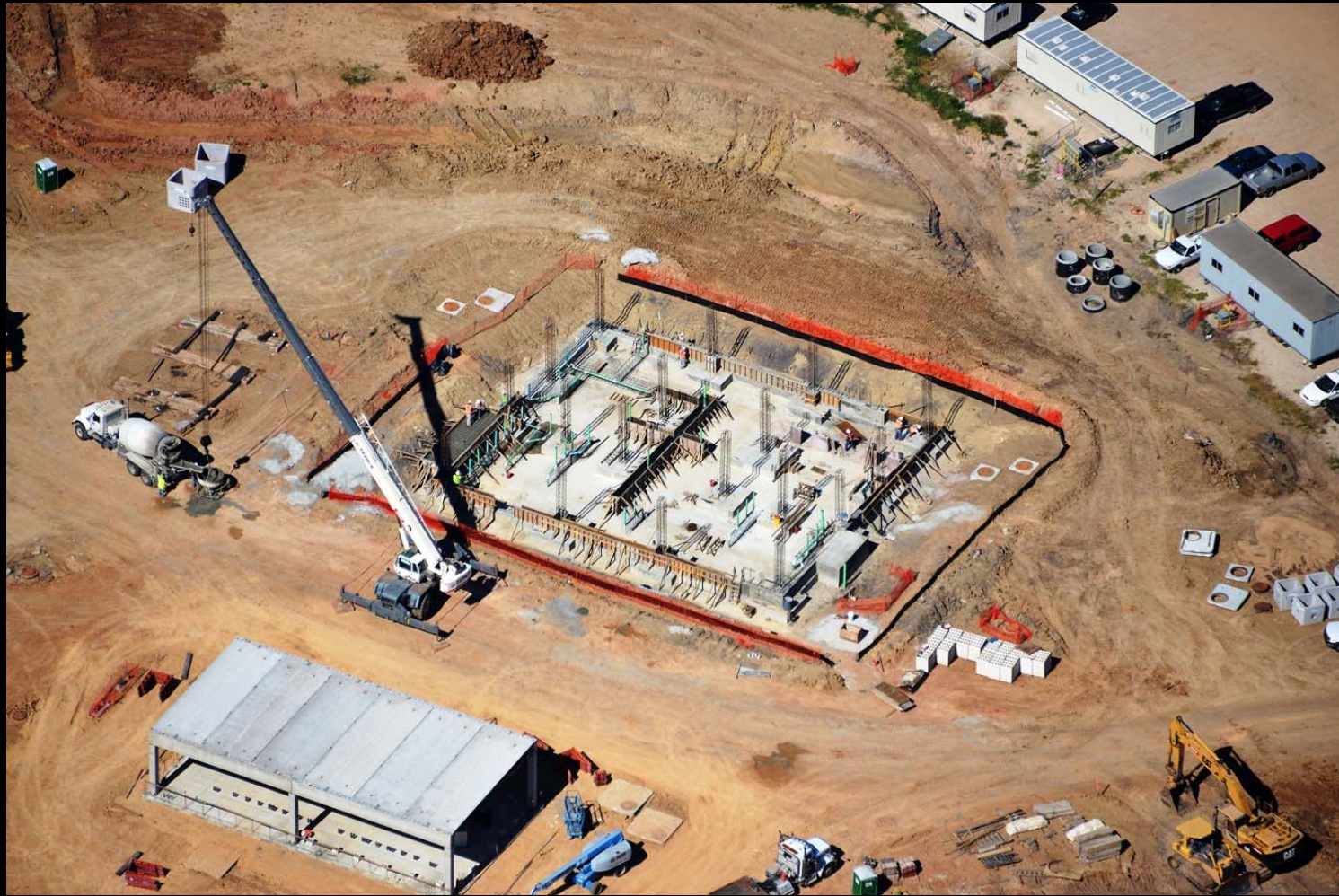
Aerial view of Dewatering Building foundation
