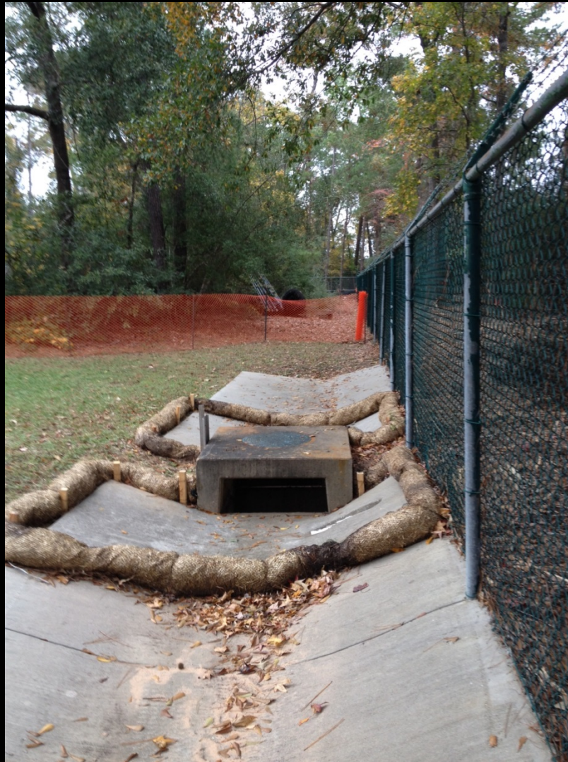
SWPPP measures installed at SJRA Water Plant #2
