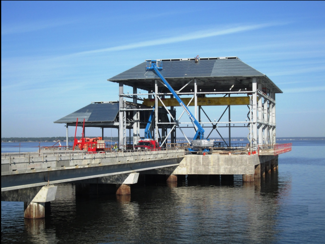
Completion of structural steel installation
