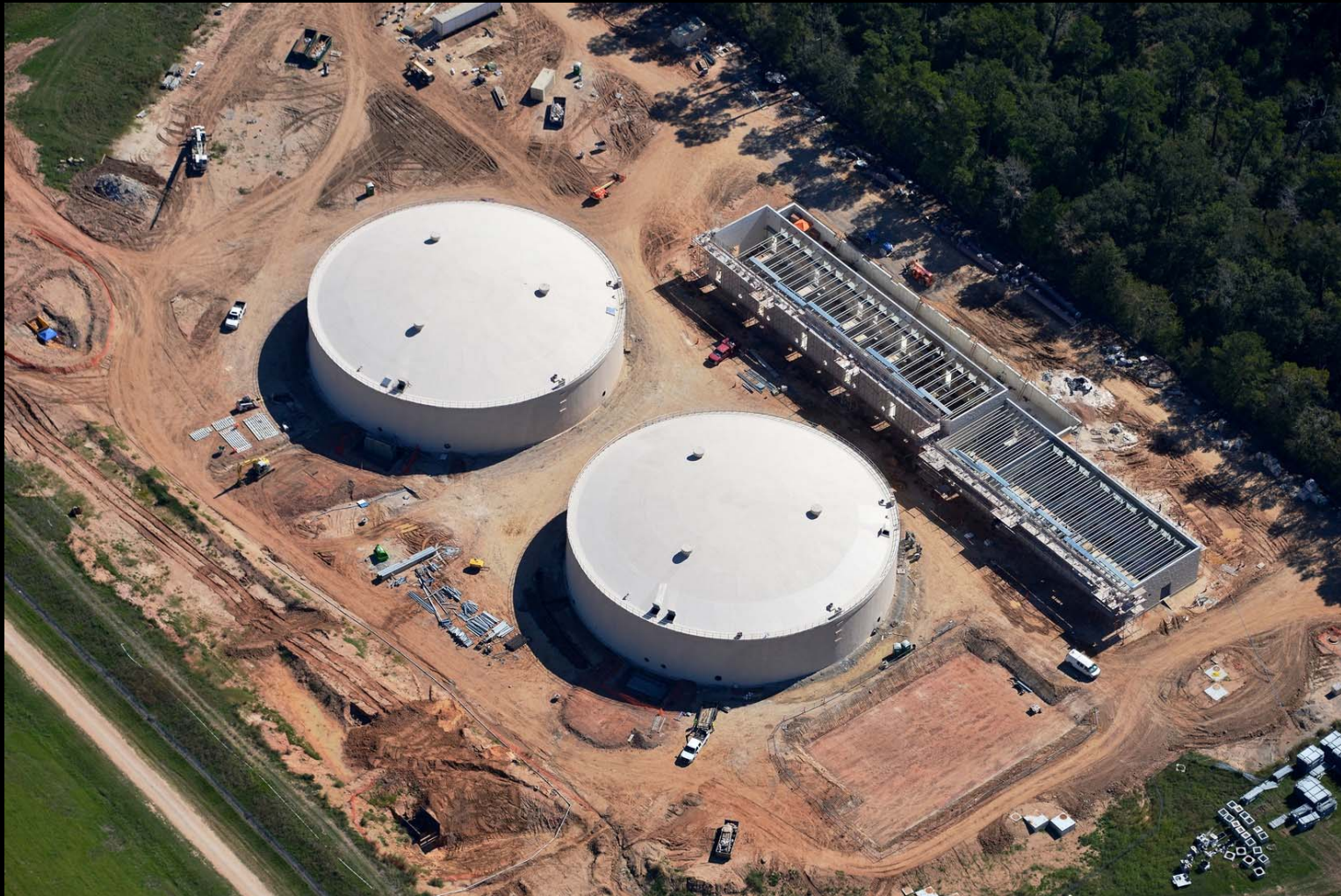
Aerial view of GST's, currently undergoing leak testing
