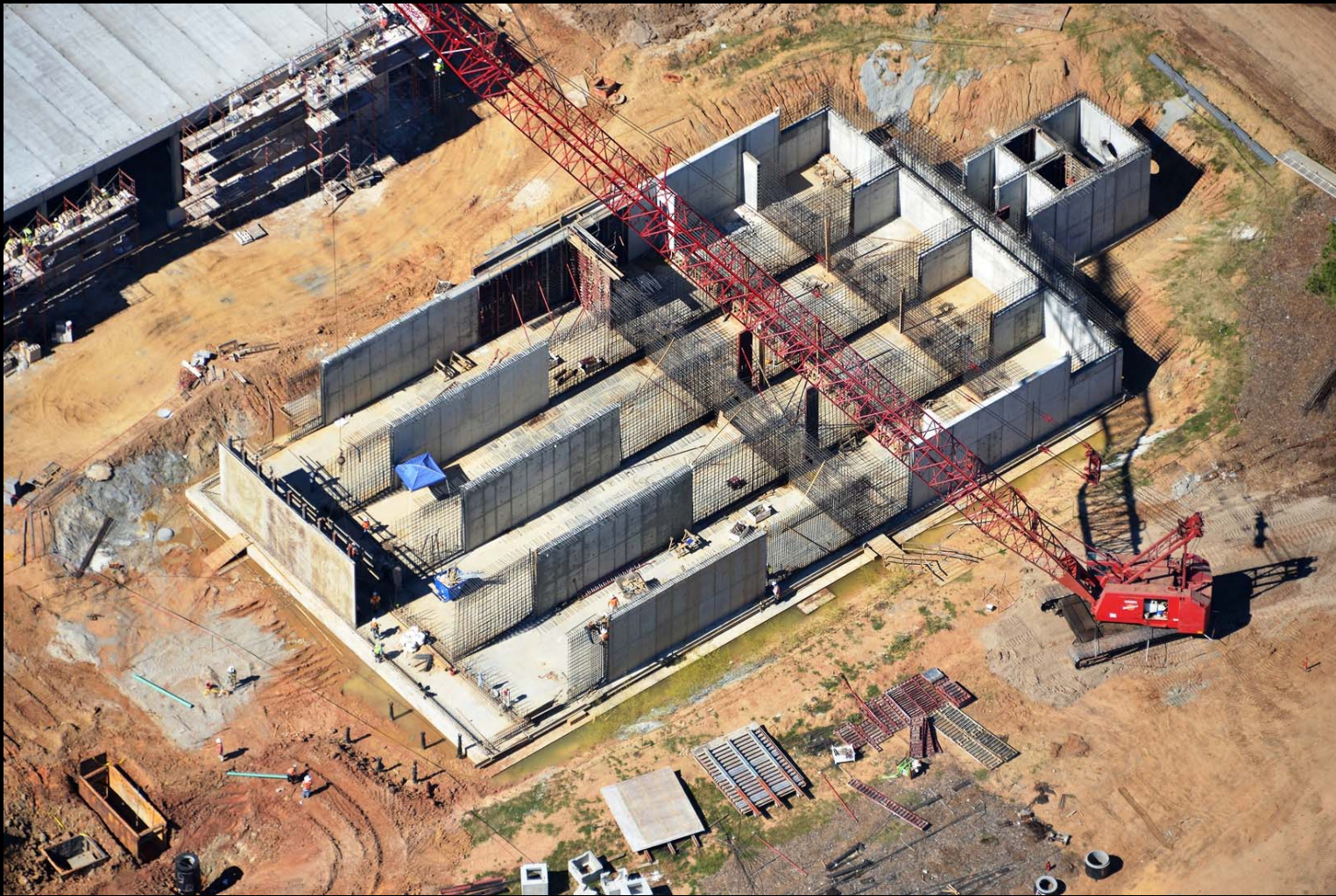
Aerial view of Pretreatment foundation installation
