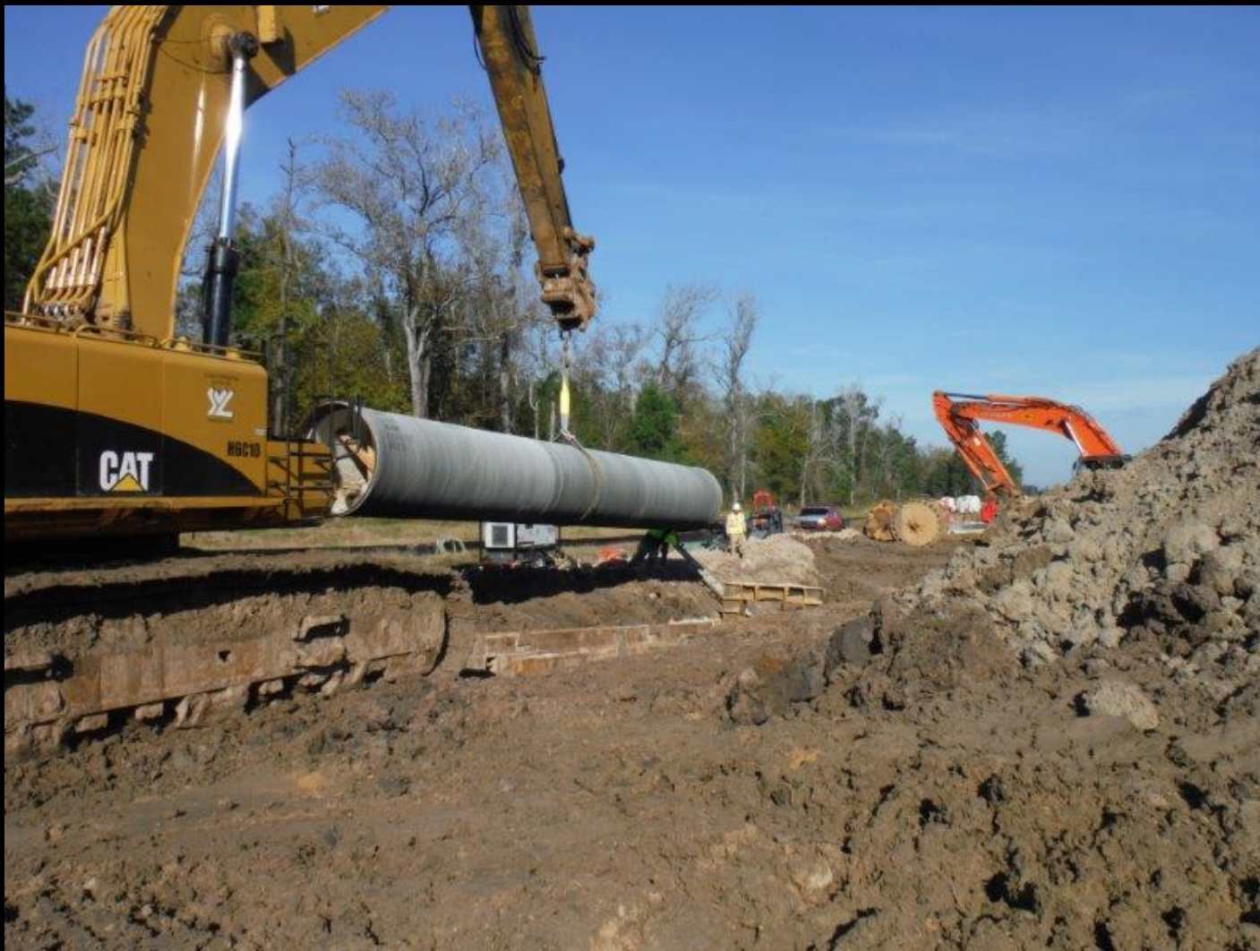
54 inch pipe installation along Fish Creek Thoroughfare near Lake Creek
