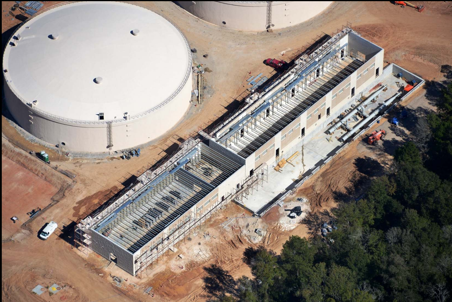
Aerial view of HSPS roof framing installation
