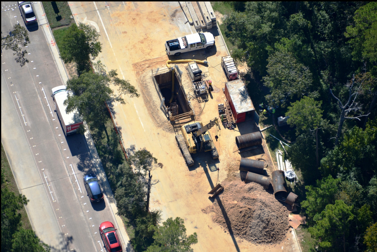
Tunnel operation utilizing 60 inch casing along Research Forest Drive at Shadowbend Place
