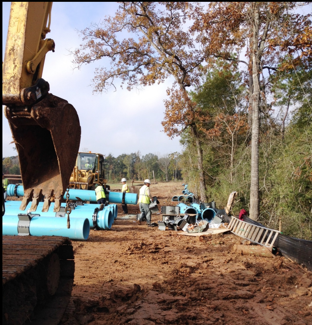
20 inch pipe installation along Tom Stinson Drive
