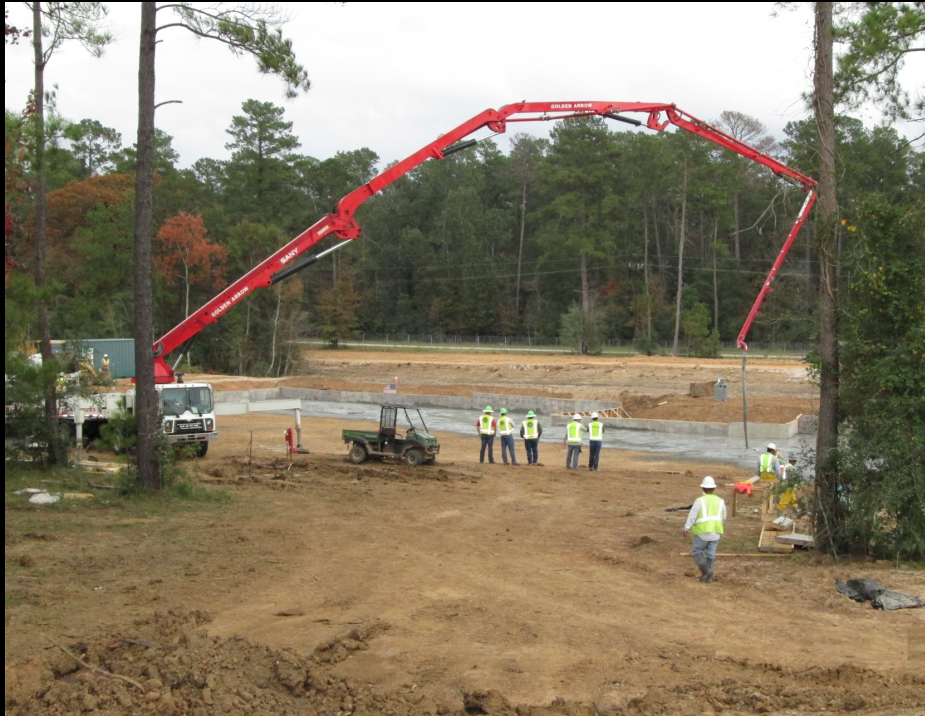
Structural backfill installation at Operations Building foundation
