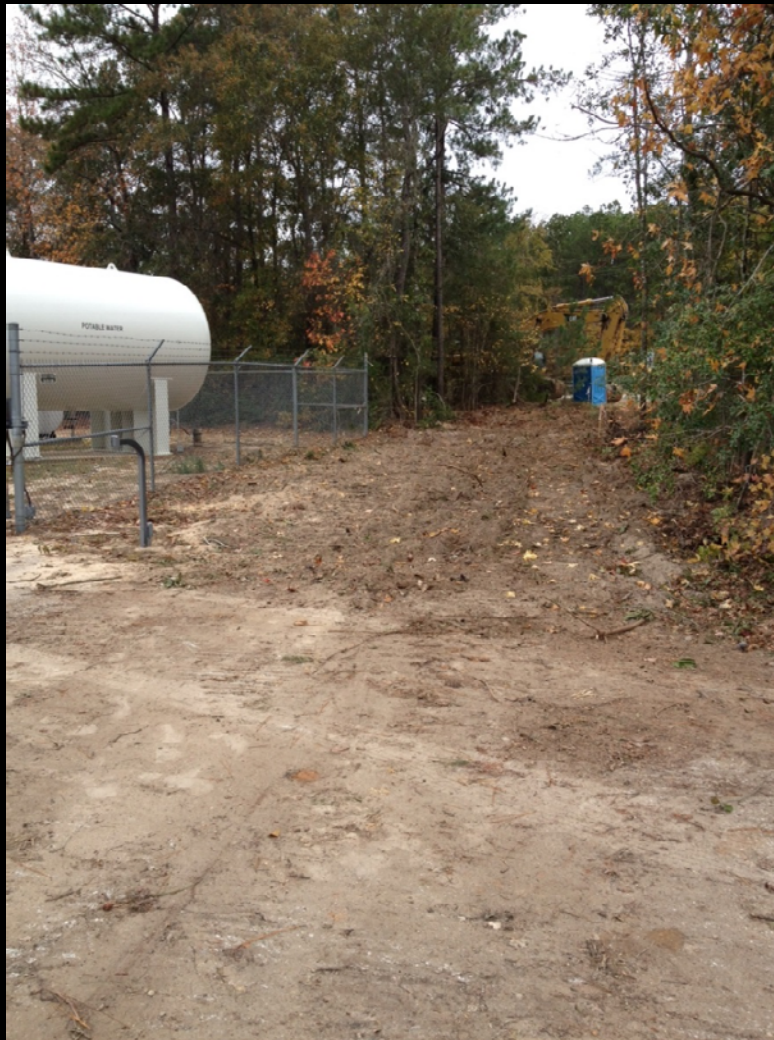
Tree clearing at City of Conroe Water Plant #15
