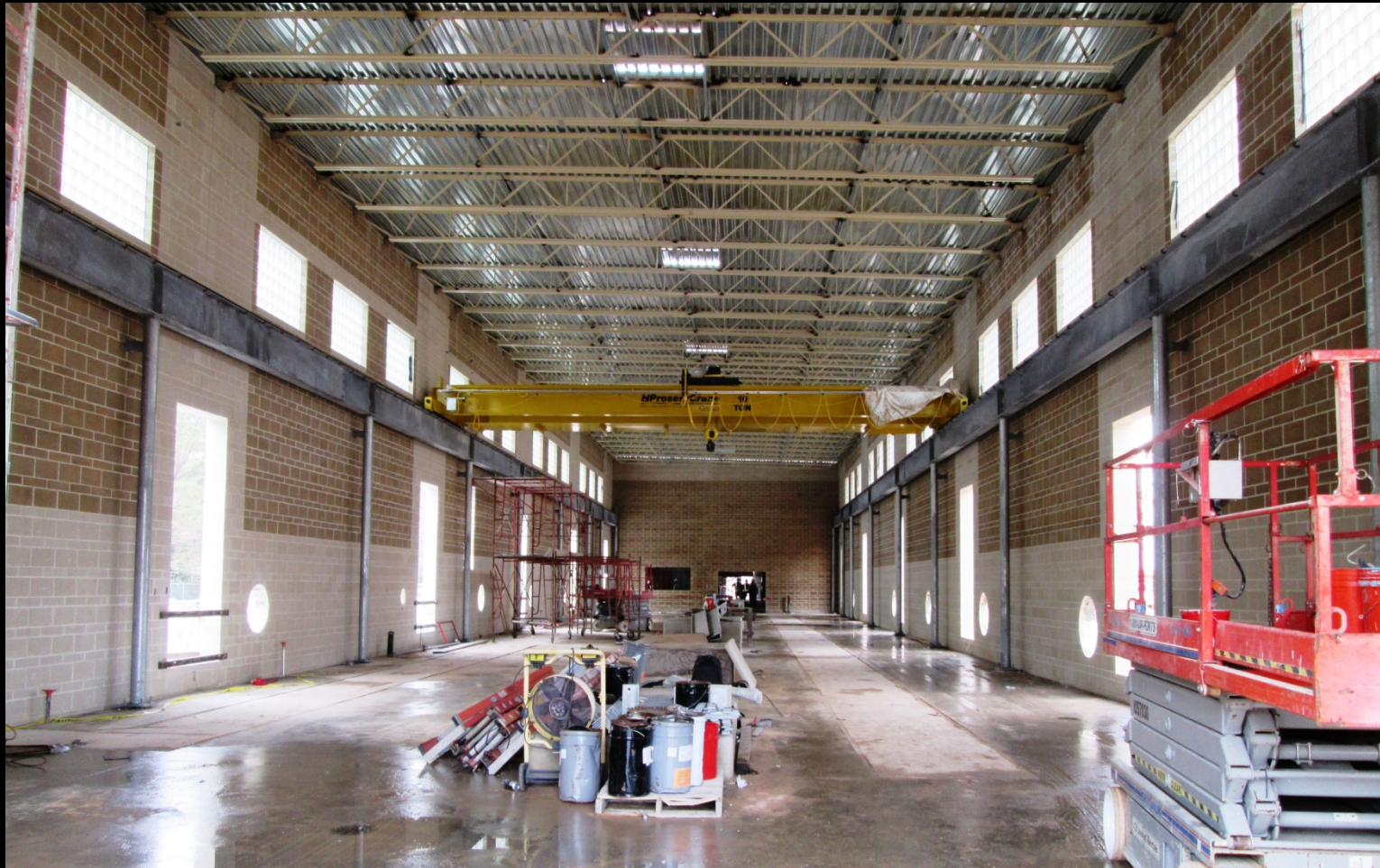
Interior view of Pump Room
