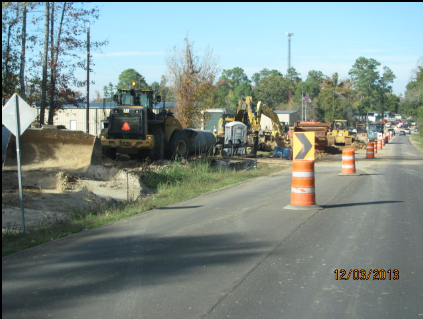
60 inch pipe installation along McCaleb Road
