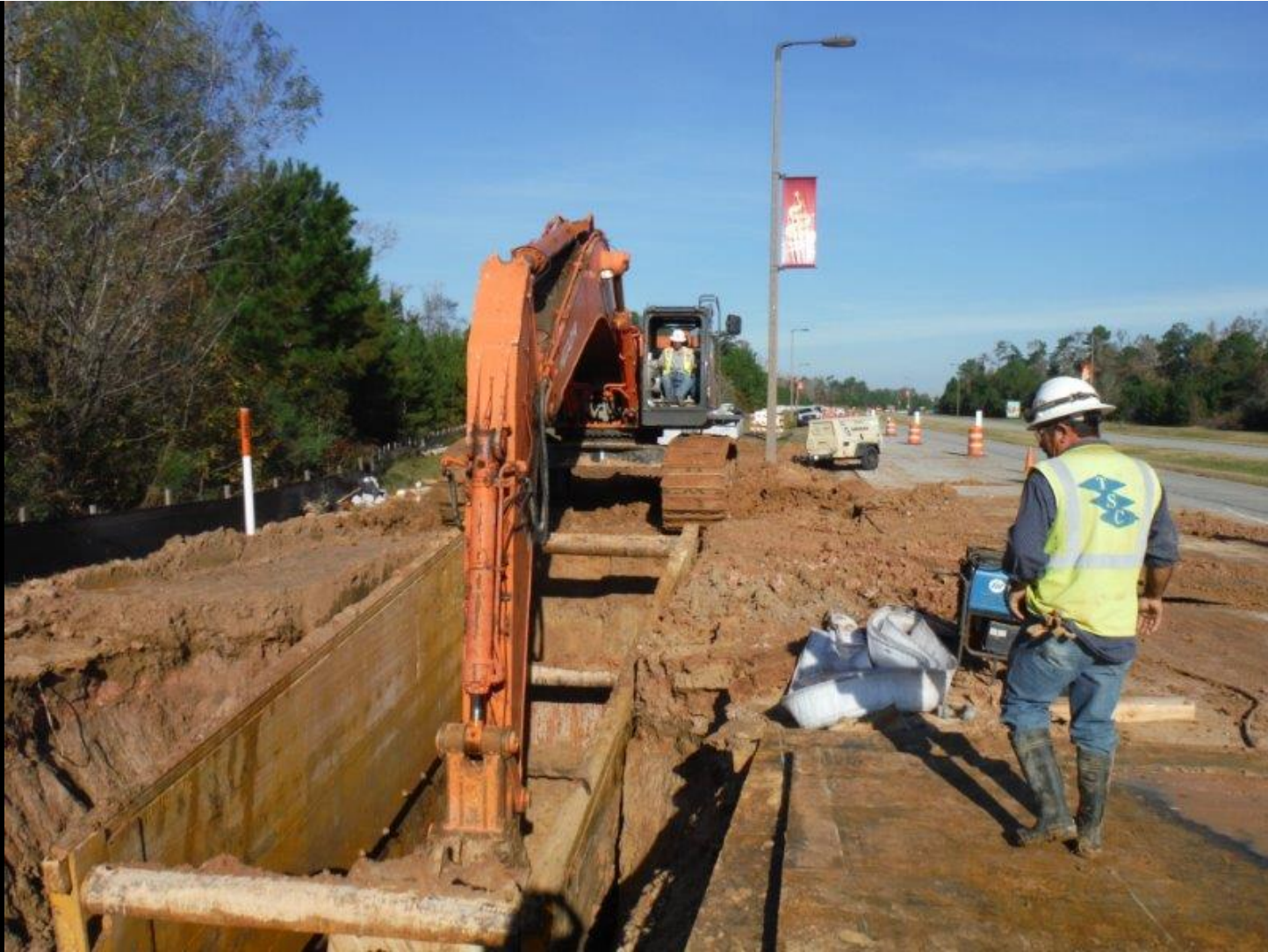
54 inch pipe installation along Fish Creek Thoroughfare
