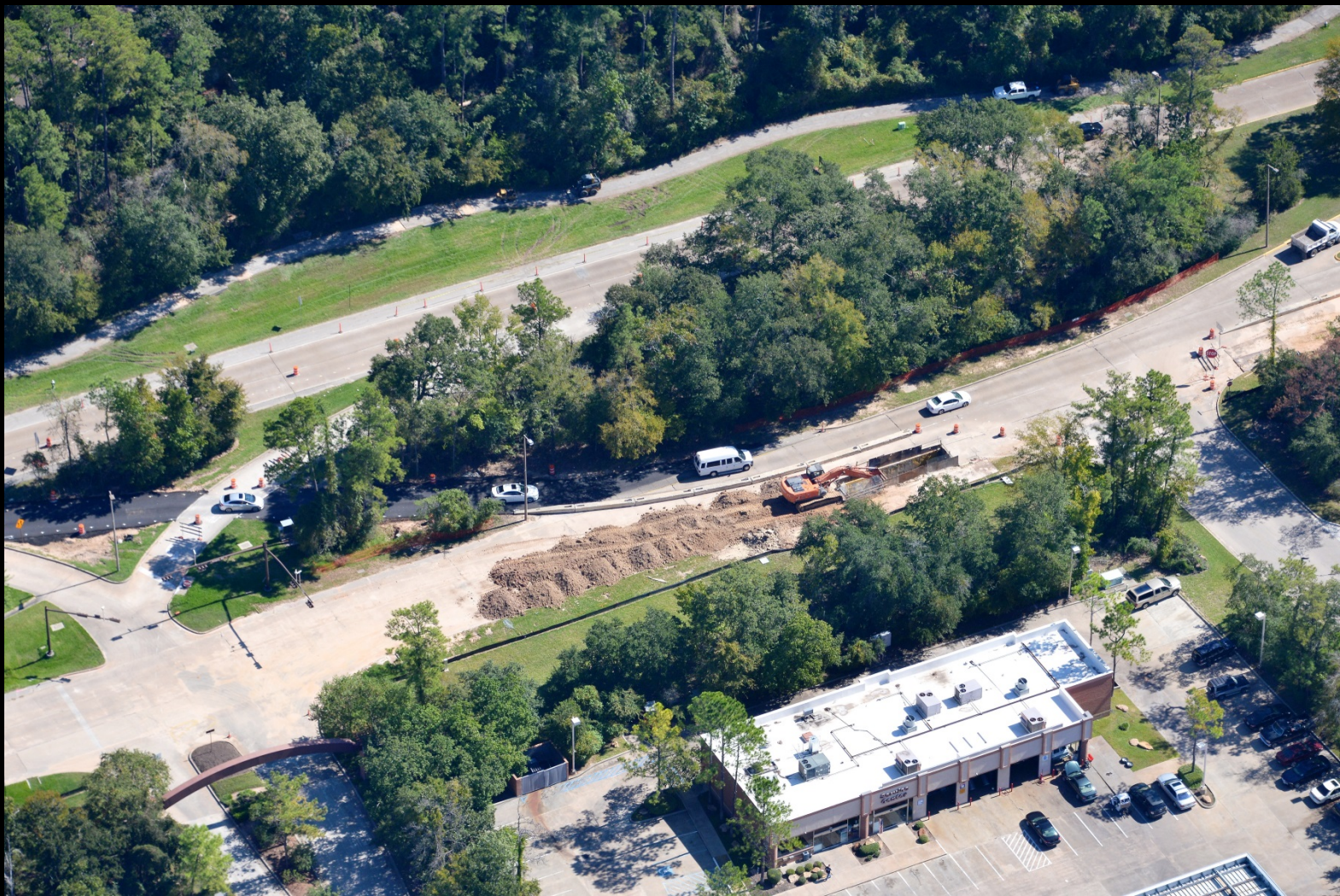
Traffic diversion and tunnel operation along Grogan's Mill Road at South Millbend Drive
