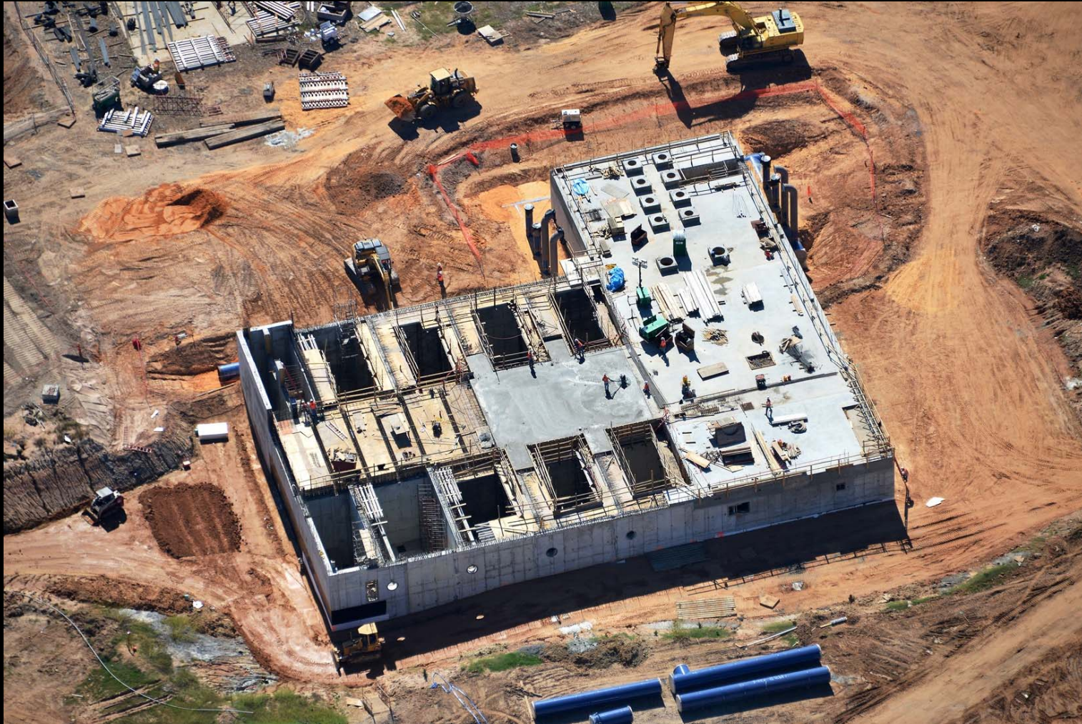
Aerial of GAC 2 nd Floor concrete deck installation
