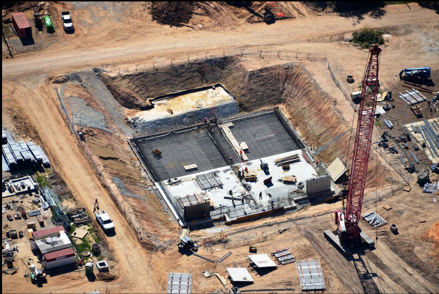
Aerial view, Backwash Equalization Basin foundation installation
