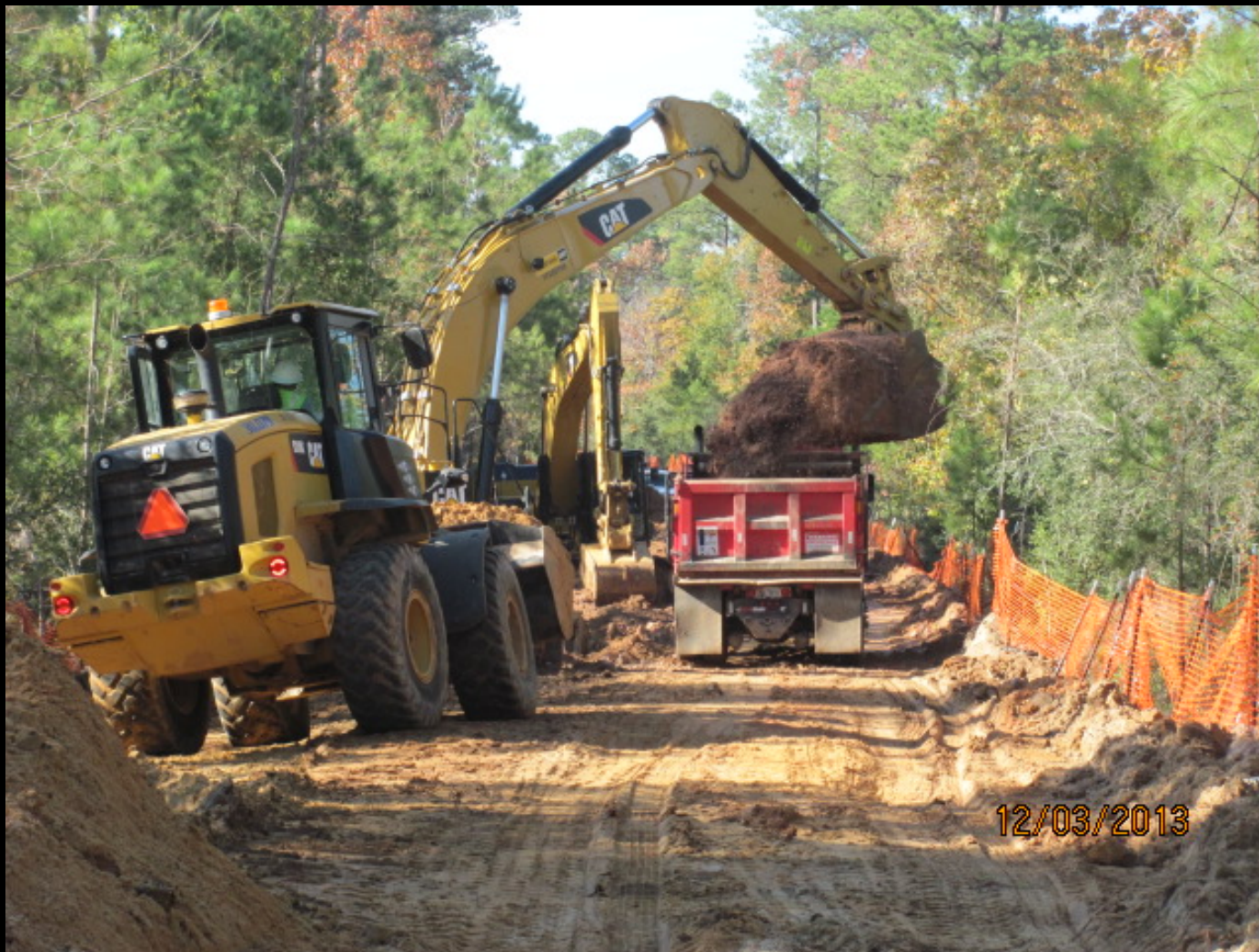
Open cut operation along future Research Forest Drive
