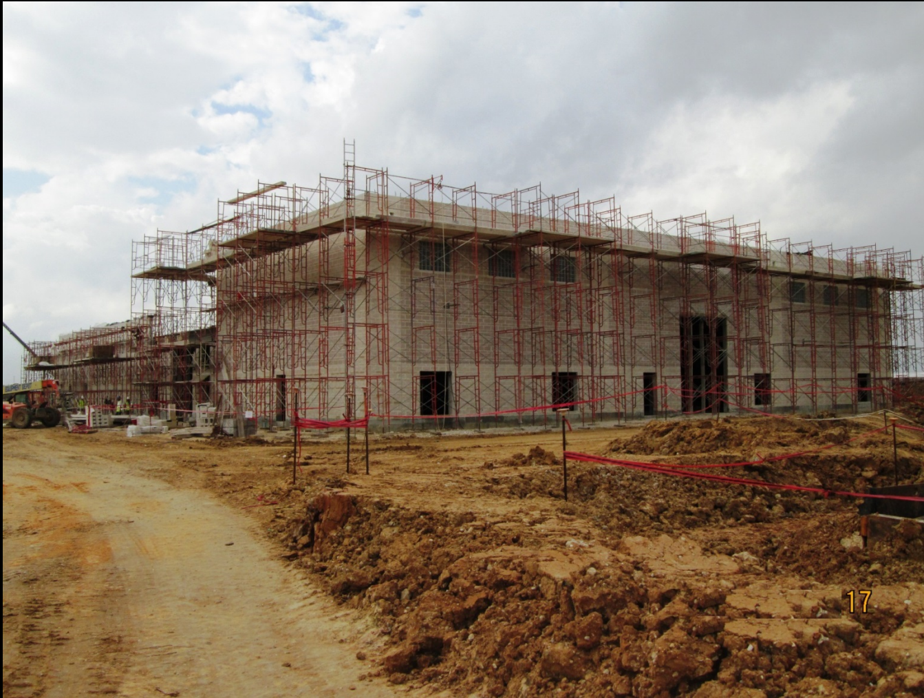
Masonry installation in progress
