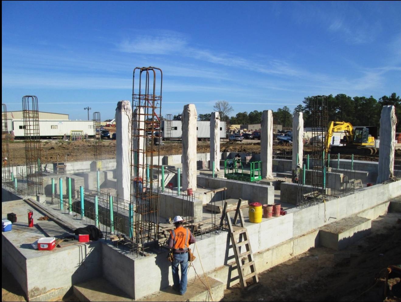
Installation of cast-in-place concrete columns
