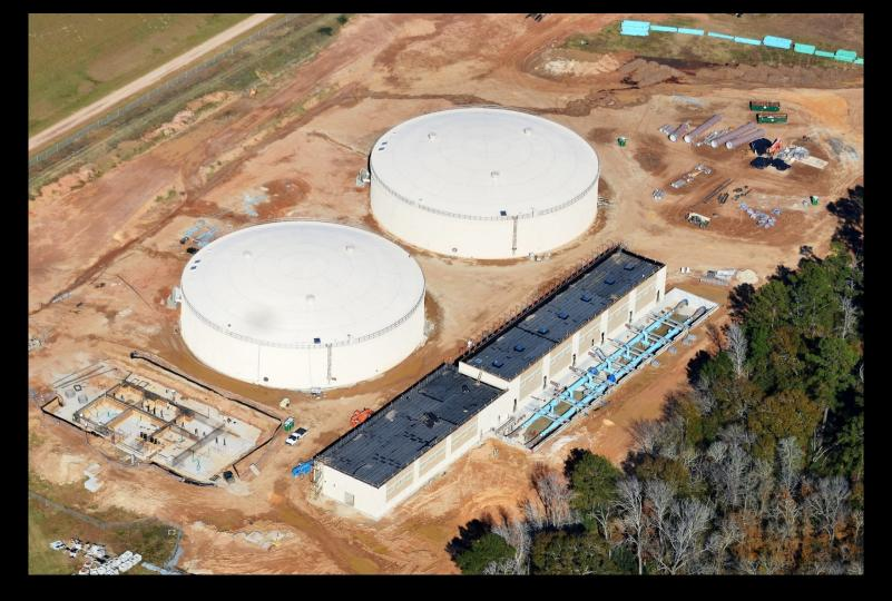
Initial leak testing complete at GSTs and HSPS dried in
