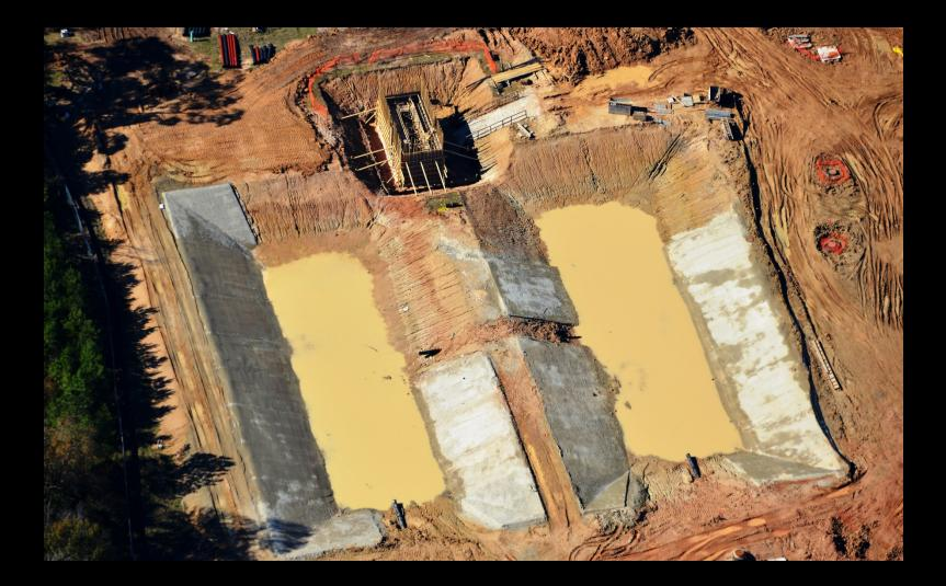
Water recovery basins and pump station foundations underway
