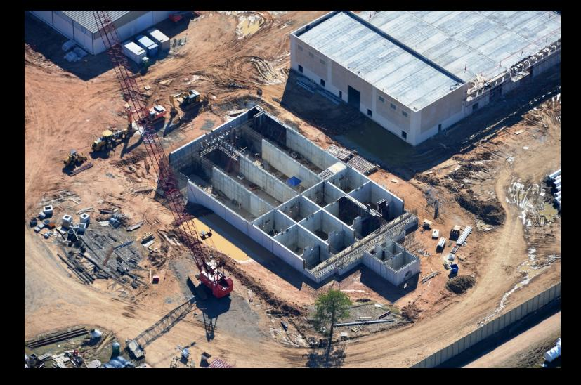
Pretreatment Facilities - Installation of intermediate concrete walls
