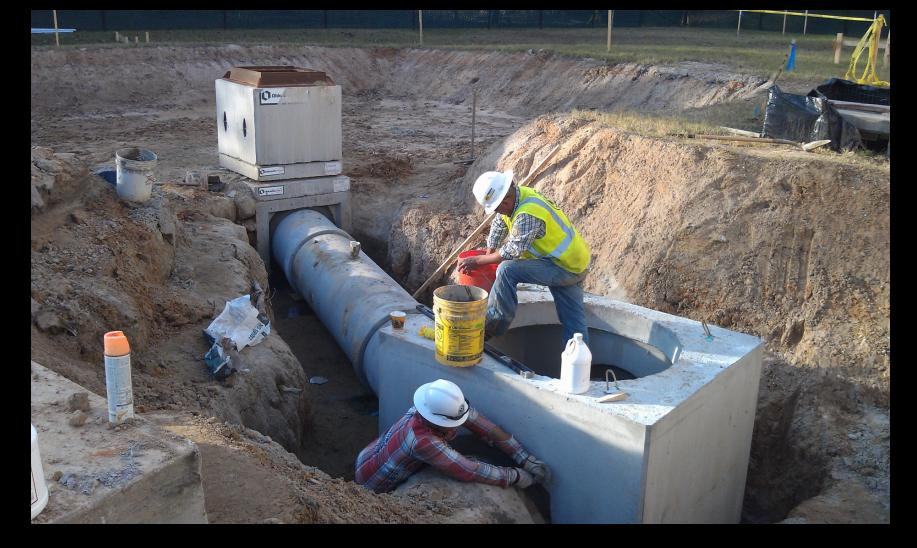
Stormwater pipe installation at SJRA Water Plant No. 4
